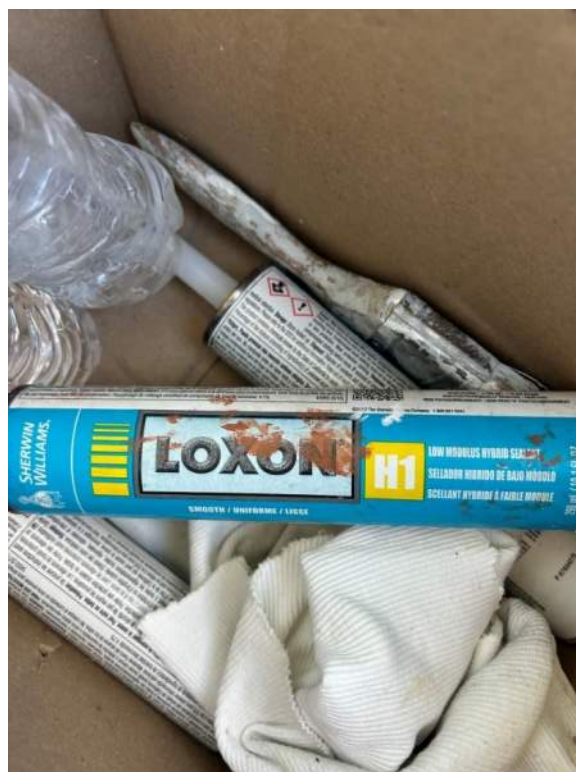
Figure 11: Sherwin Williams Loxon hybrid sealant was observed on site for application.
