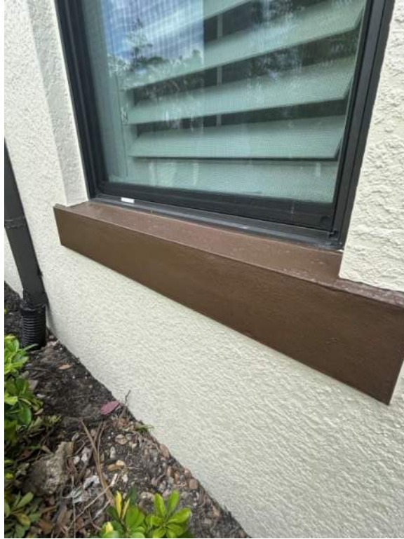
Figure 3: Paint application was completed on the brown window ledges.
