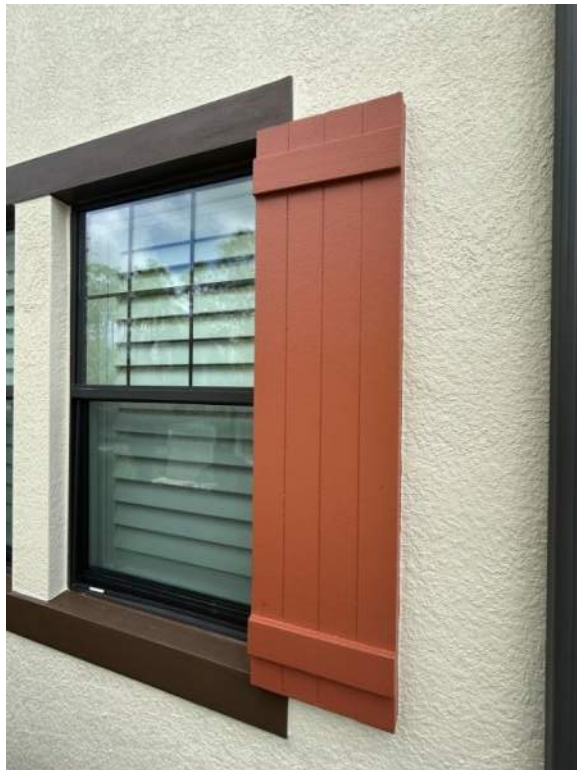
Figure 2: Paint application was completed on the red details on the sides of the windows.
