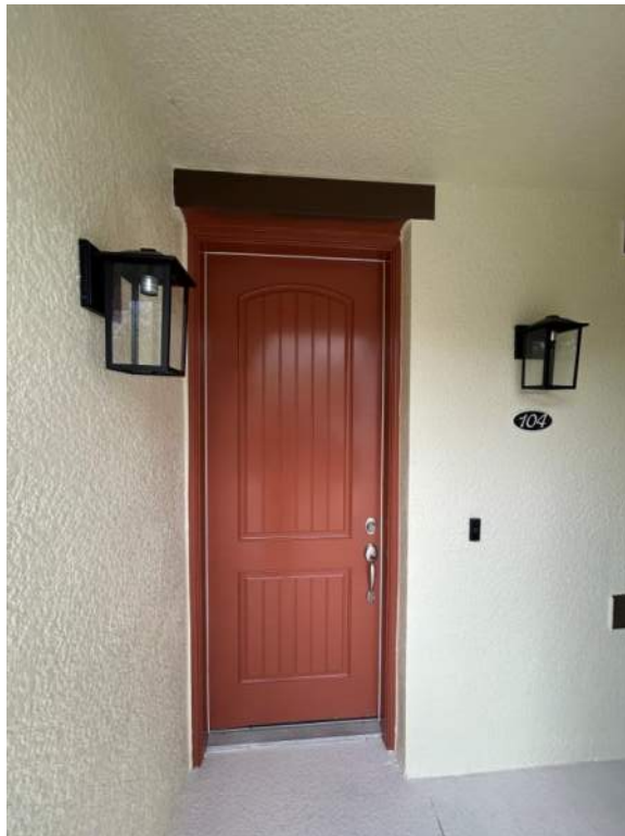
Figure 4: Paint application was completed on the red entry unit doors.
