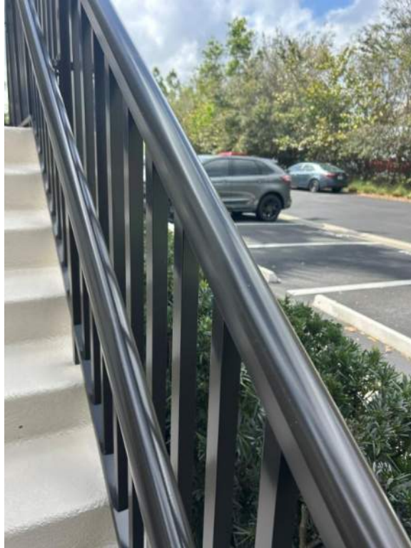
Figure 5: Paint application was completed on the guardrails of both staircases.
