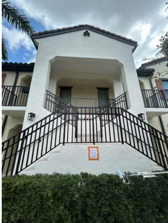
Figure 1: Paint application was completed on the exterior wall of the building.
