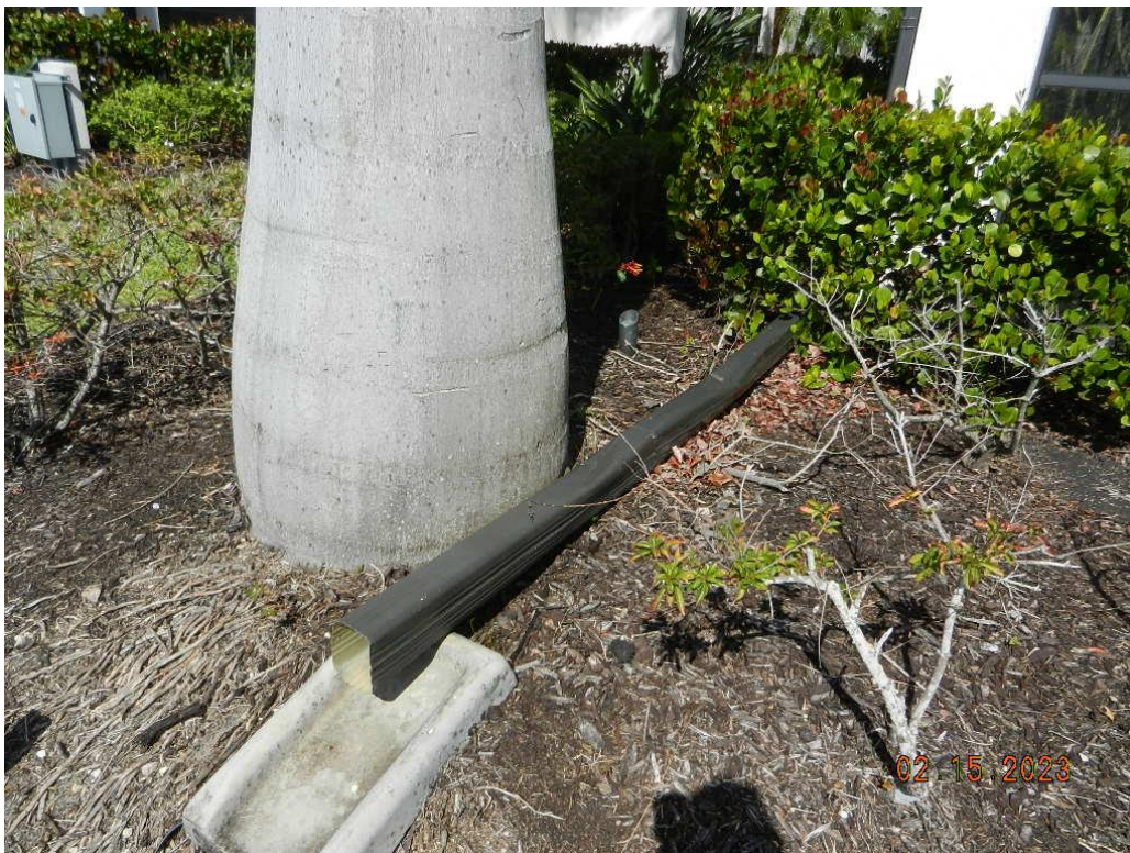
Damaged Down Spout with Negative Pitch
