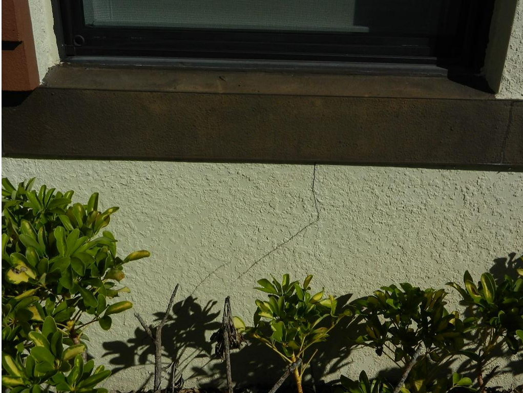
Stucco Delamination at 15110 Unit #105
