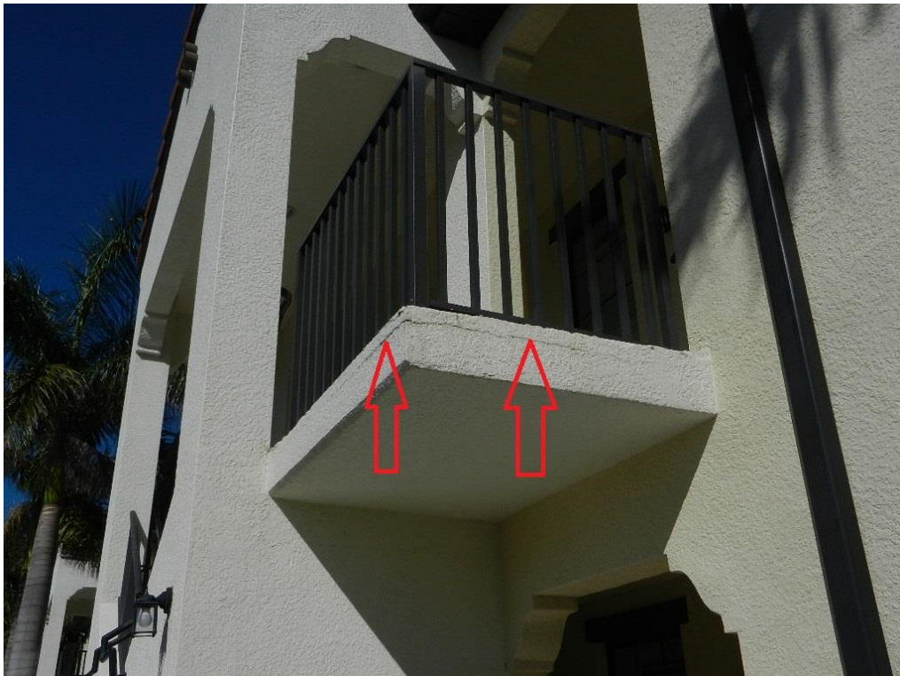
Stucco Delamination at Building 15110 with Potential Concrete / Rebar Damage
