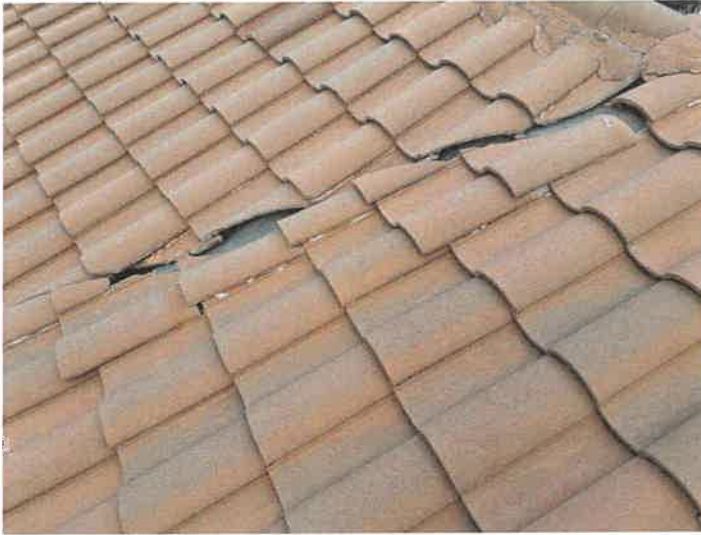
Pool House: Displaced/Missing Roof Tile
