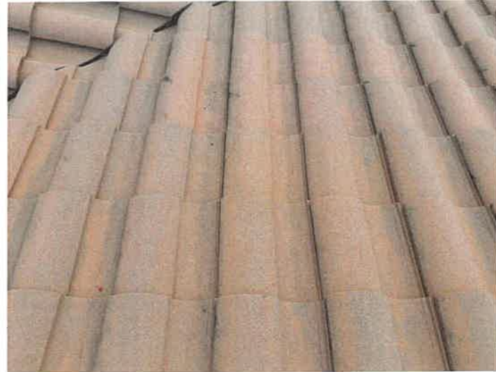
Pool House: Repaired Cracked Roof Tiles The cracked roof tiles were repaired with Titebond sealant.
