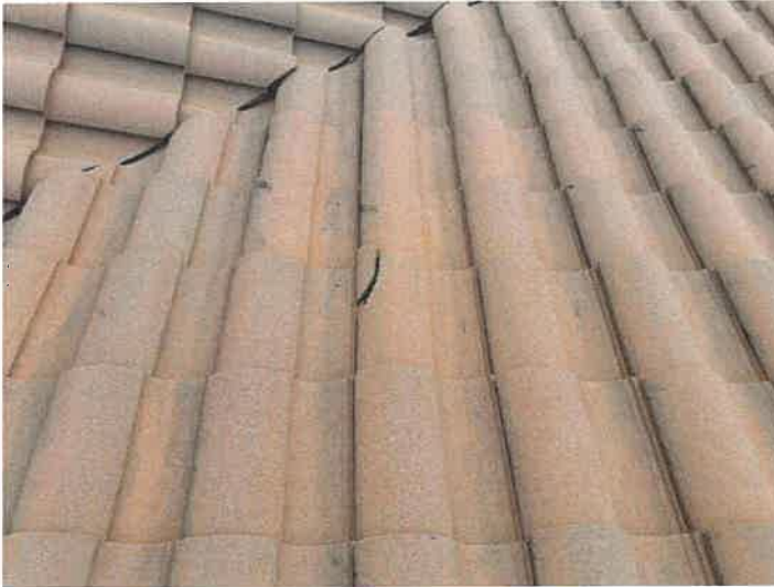
Pool House: Identified Cracked Roof Tiles Cracked roof tiles can allow premature underlayment deterioration from excessive UV exposure.
