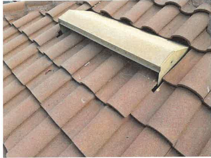
Pool House: Repaired Displaced/Missing Roof Tile
