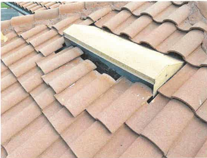
Pool House: Displaced/Missing Roof Tile
