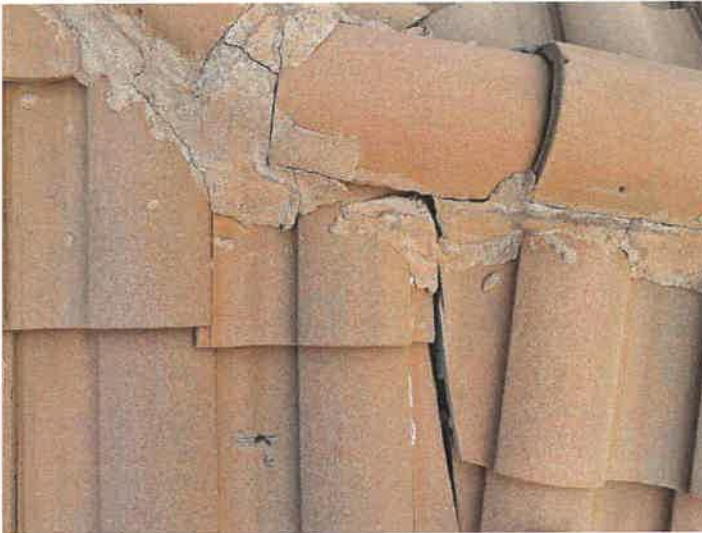
Pool House: Identified Cracked Roof Tiles Cracked roof tiles can allow premature underlayment deterioration from excessive UV exposure.
