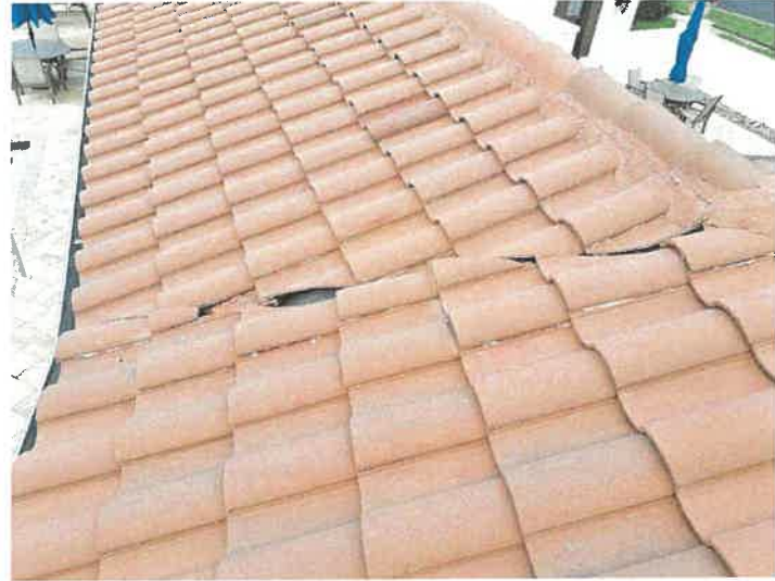
Pool House: Repaired Displaced/Missing Roof Tile
