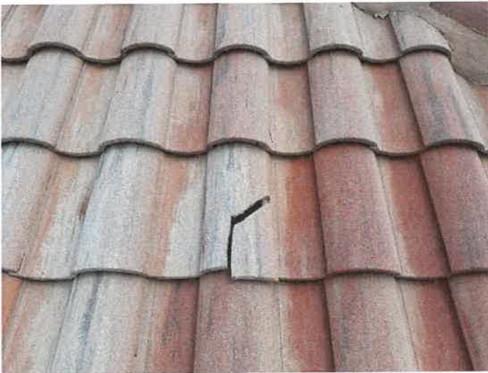
Building 15197: Identified Cracked Roof Tiles
