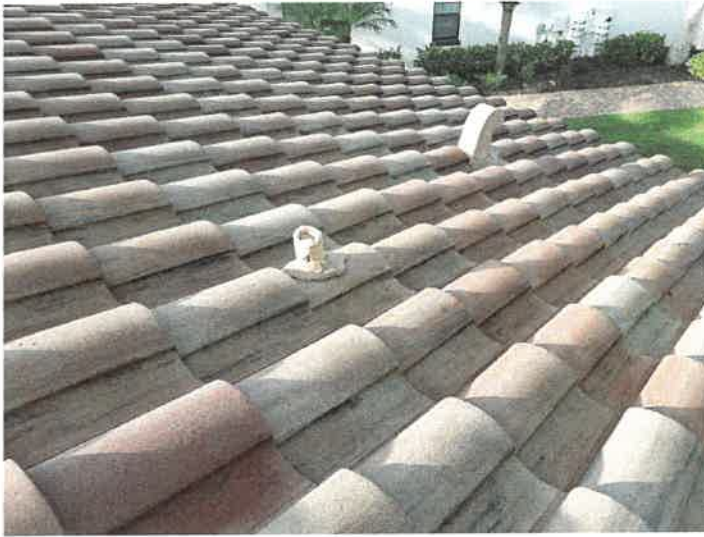
Building 15177: Lead Boots Lead boots appear to be in good condition.
