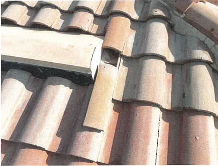
Building 15201: Displaced/Missing Roof Tile
