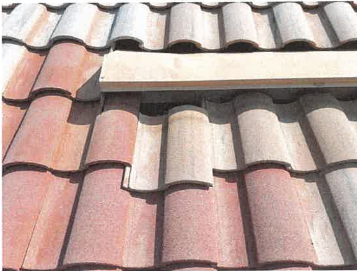
Building 15205: Displaced/Missing Roof Tile
