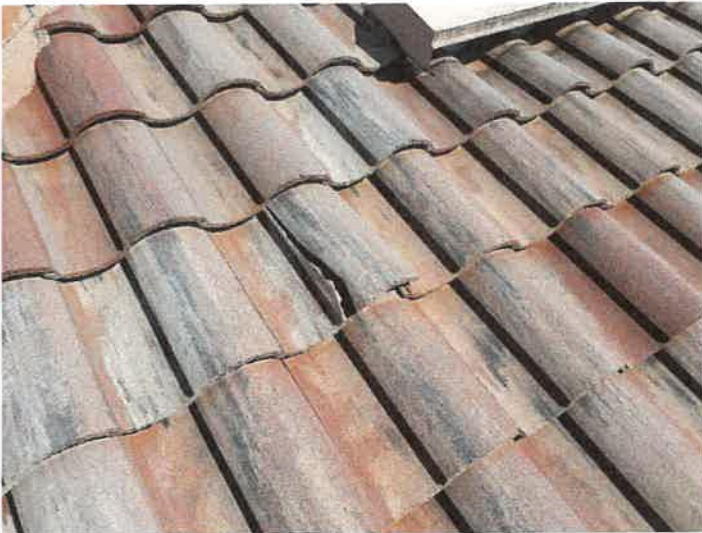
Building 15161: Identified Cracked Roof Tiles
