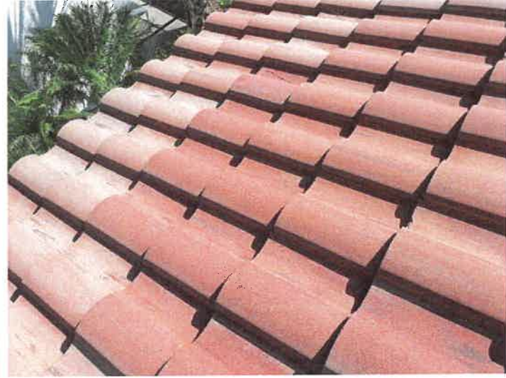
Building 15188: Repaired Cracked Roof Tiles
