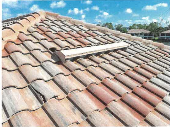
Building 15161: Roof Vents
