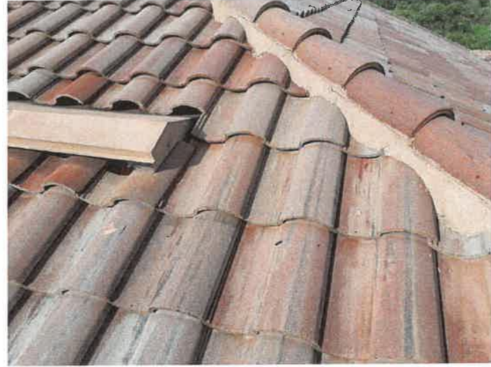
Building 15177: Repaired Displaced/Missing Roof Tile Replaced and secured the missing roof tile.
