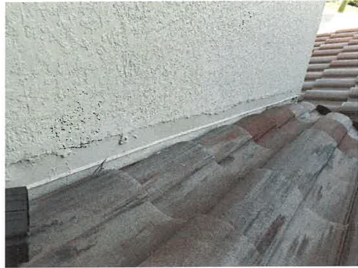
Building 15161: Counter Flashings The counter flashing appears to be in good condition.
