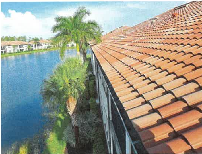
Building 15201: Gutters The gutters appear to be in good condition.
