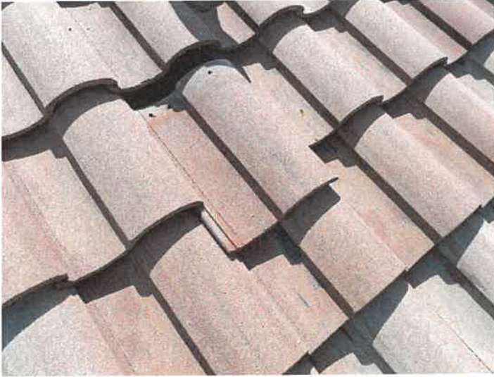
Building 15188: Displaced/Missing Roof Tile
