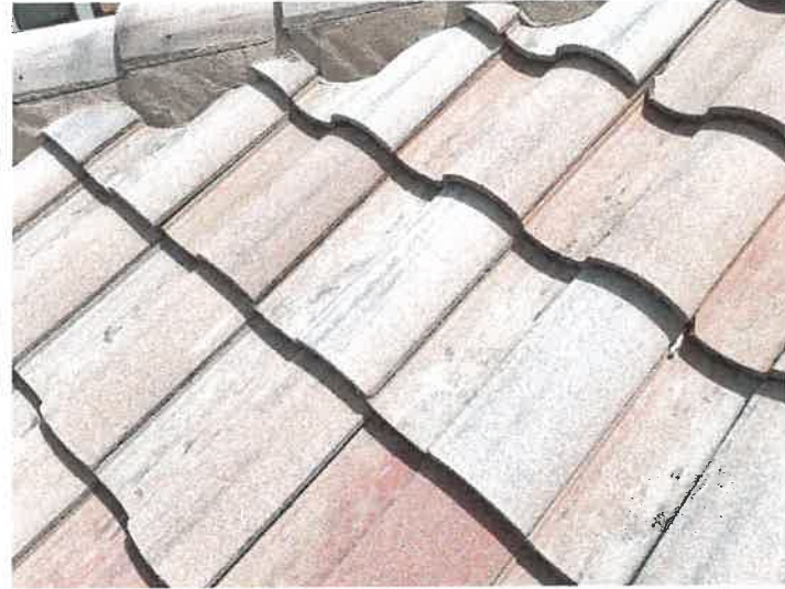
Building 15169: Repaired Displaced/Missing Roof Tile
