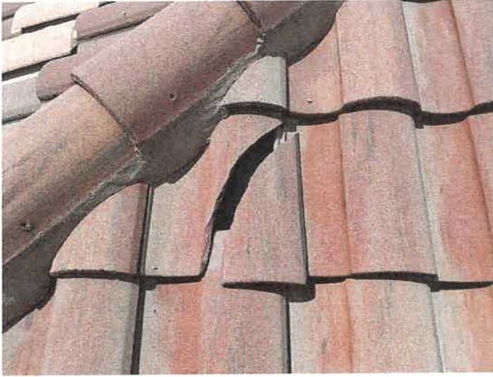
Building 15197: Identified Cracked Roof Tiles
