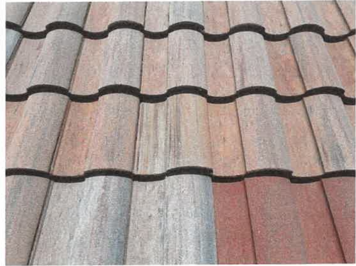
Building 15213: Repaired Displaced/Missing Roof Tile
