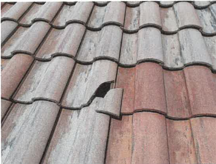
Building 15209: Identified Cracked Roof Tiles
