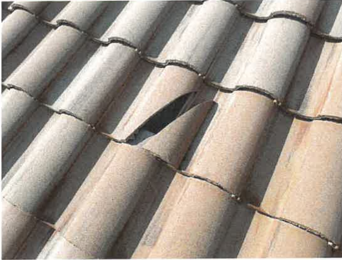
Building 15201: Identified Cracked Roof Tiles
