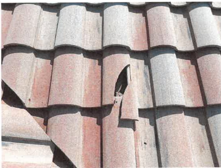
Building 15188: Identified Cracked Roof Tiles
