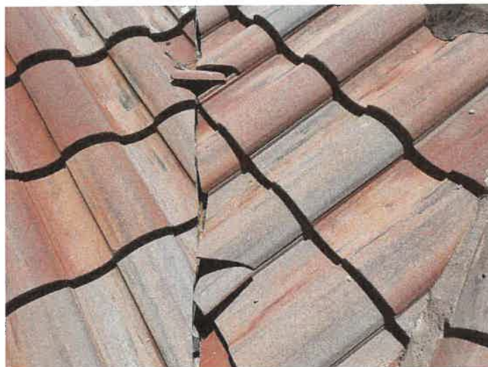
Building 15184: Identified Cracked Roof Tiles Cracked roof tiles can allow premature underlayment deterioration from excessive UV exposure.
