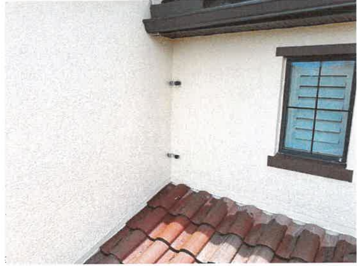
Building 15169: Downspout- missing
