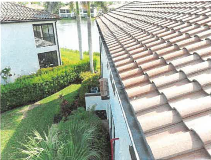
Building 15161: Gutters The gutters appear to be in good condition.
