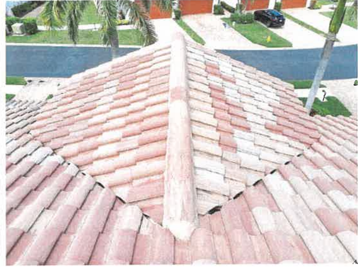
Building 15184: Valley The valley tiles appear to be in good condition.
