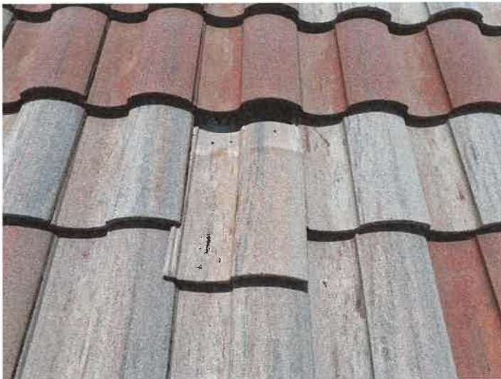
Building 15213: Displaced/Missing Roof Tile
