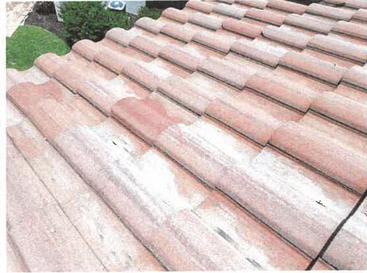
Building 15173: Repaired Cracked Roof Tiles
