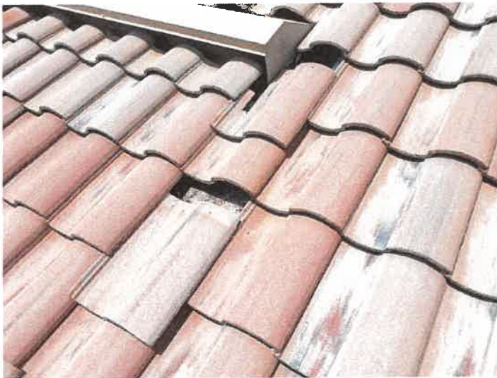
Building 15184: Identified Cracked Roof Tiles Cracked roof tiles can allow premature underlayment deterioration from excessive UV exposure.
