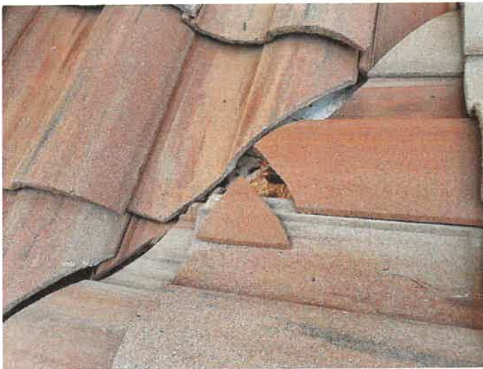
Building 15197: Identified Cracked Roof Tiles Cracked roof tiles can allow premature underlayment deterioration from excessive UV exposure.
