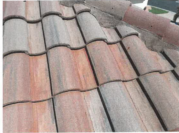
Building 15185: Repaired Cracked Roof Tiles The cracked roof tiles were repaired with Titebond sealant.
