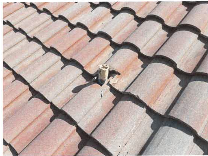
Building 15185: Missing Mortar Identified missing mortar around of lead boot. Crowther Roofing suggests installing mortar.
