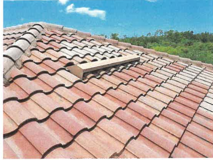
Building 15173: Roof Vents Roof vents appear to be in good condition.
