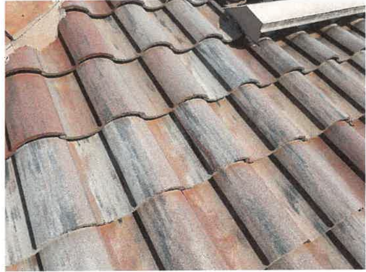
Building 15161: Repaired Cracked Roof Tiles
