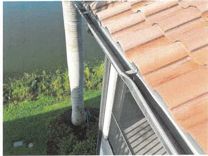
Building 15201: Gutter Metal- Broken Gutter is broken and needs to be replaced. (1ft.6" residential model).
