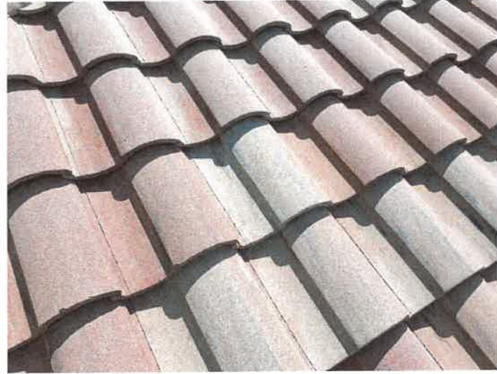
Building 15185: Repaired Displaced/Missing Roof Tile Replaced and secured the missing roof tile.
