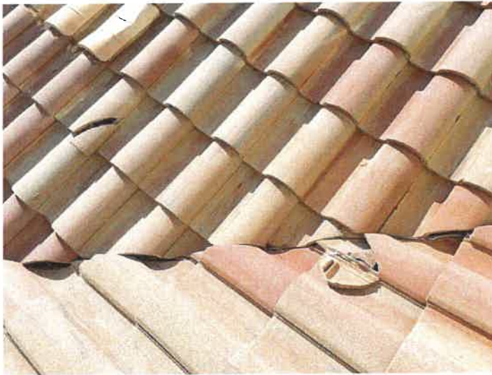
Building 15189: Identified Cracked Roof Tiles Cracked roof tiles can allow premature underlayment deterioration from excessive UV exposure.
