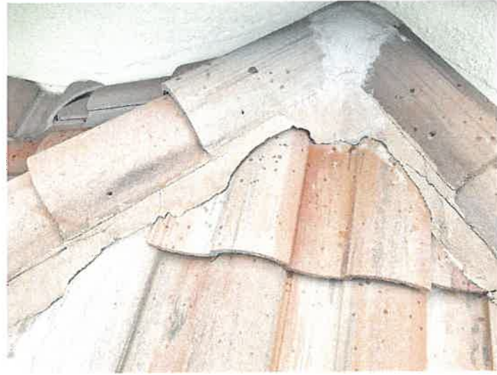
Building 15169: Repaired Displaced/Missing Roof Tile
