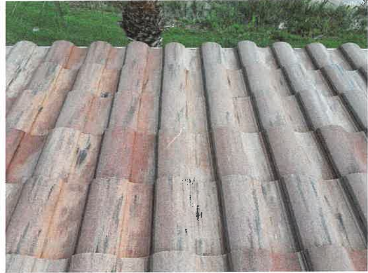
Building 15161: Repaired Cracked Roof Tiles The cracked roof tiles were repaired with Titebond sealant.
