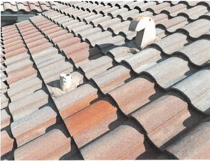
Building 15161: Lead Boots Lead boots appear to be in good condition.
