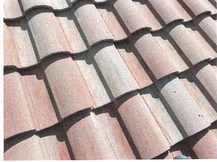
Building 15185: Repaired Displaced/Missing Roof Tile
