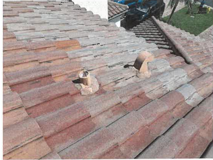
Building 15185: Lead Boots Lead boots appear to be in good condition.
