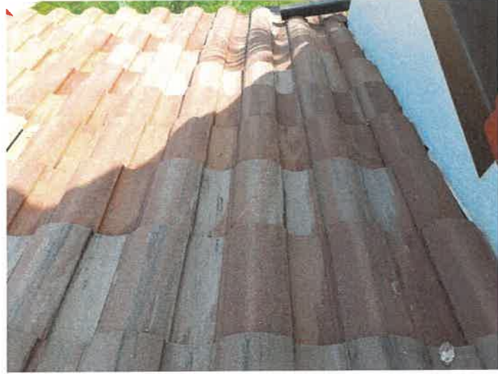
Building 15177: Repaired Cracked Roof Tiles
