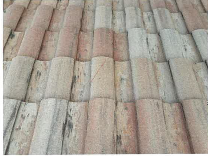
Building 15169: Repaired Cracked Roof Tiles
