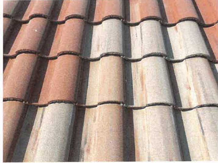
Building 15201: Repaired Displaced/Missing Roof Tile
