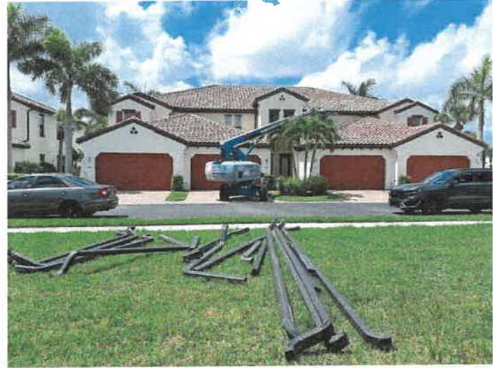
Building 15197: Downspout- missing
