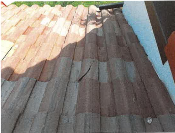
Building 15177: Identified Cracked Roof Tiles
