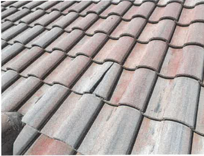
Building 15185: Identified Cracked Roof Tiles Cracked roof tiles can allow premature underlayment deterioration from excessive UV exposure.
