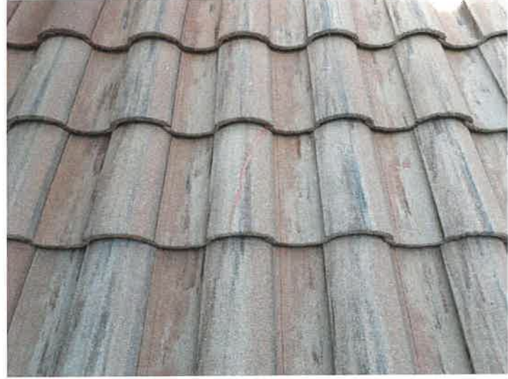
Building 15177: Repaired Cracked Roof Tiles The cracked roof tiles were repaired with Titebond sealant.
