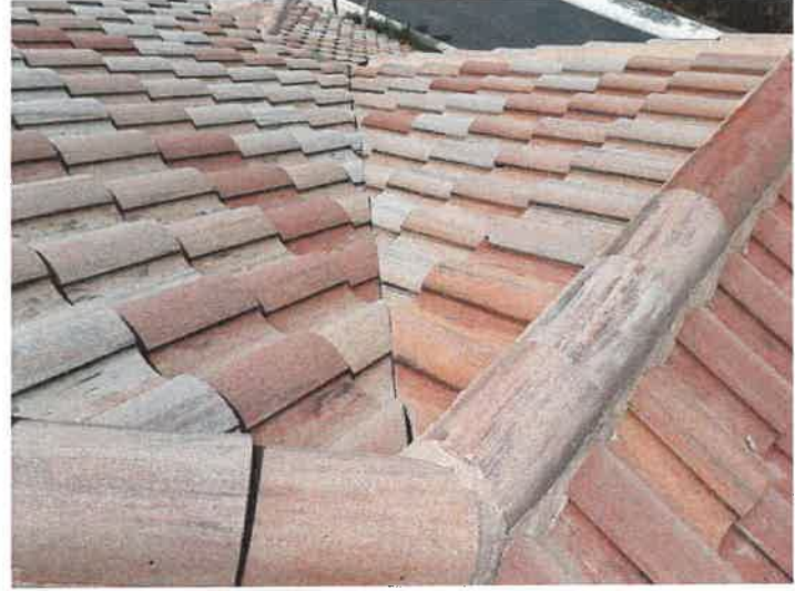
Building 15169: Valley The valley tiles appear to be in good condition.
