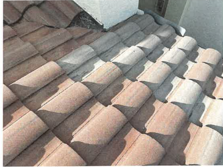
Building 15177: Repaired Cracked Roof Tiles
