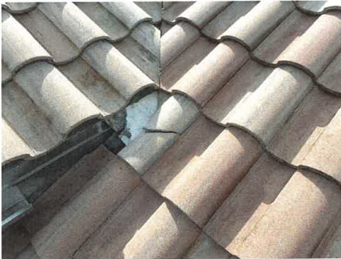
Building 15177: Identified Cracked Roof Tiles Cracked roof tiles can allow premature underlayment deterioration from excessive UV exposure.
