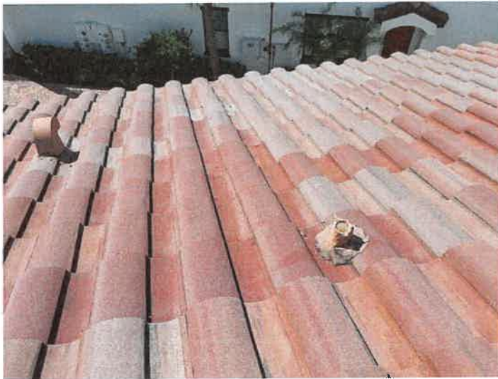
Building 15185: Lead Boots Lead boots appear to be in good condition.
