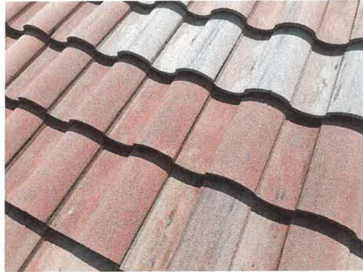
Building 15165: Repaired Cracked Roof Tiles
