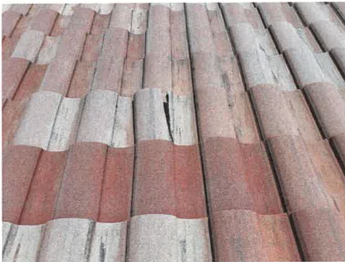
Building 15193: Identified Cracked Roof Tiles
