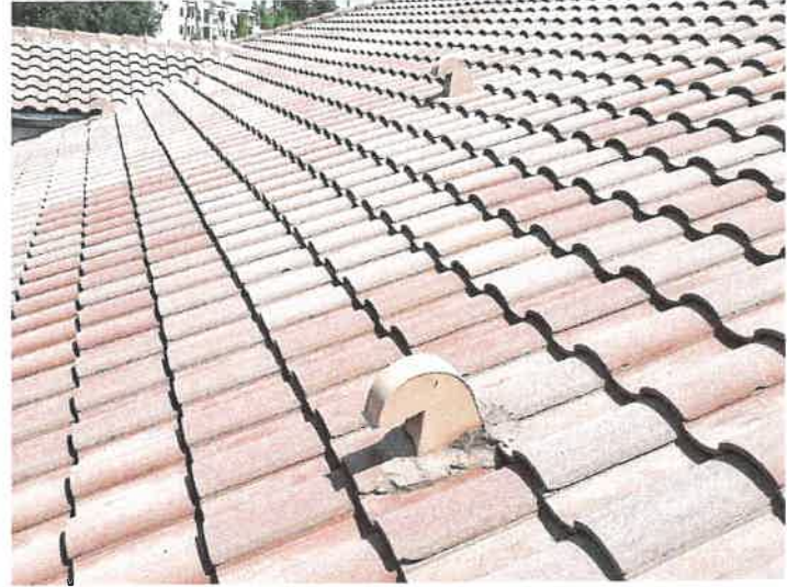
Building 15184: Roof Vents Roof vents appear to be in good condition.
