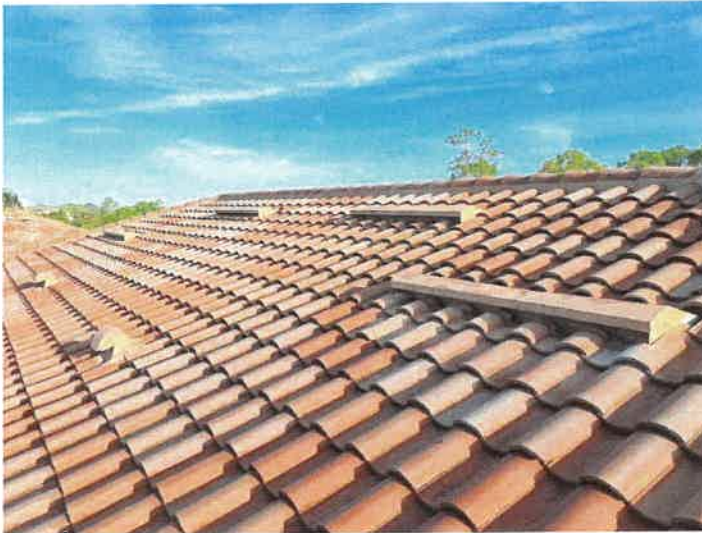
Building 15181: Roof Vents
