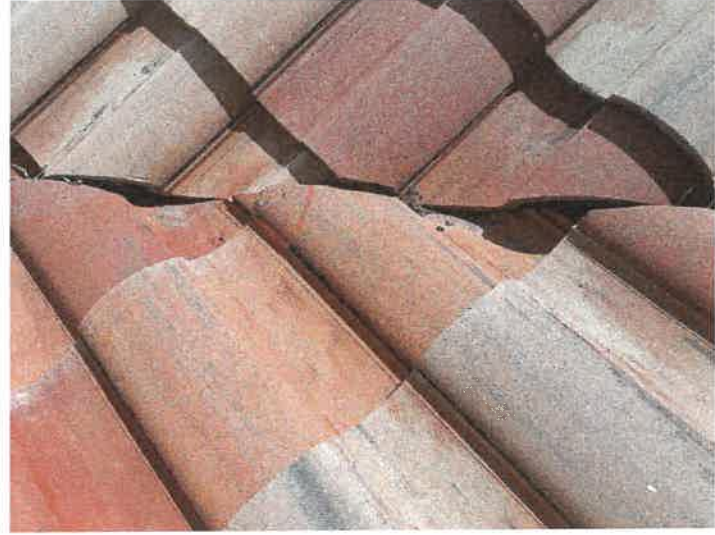
Building 15205: Repaired Cracked Roof Tiles The cracked roof tiles were repaired with Titebond sealant.
