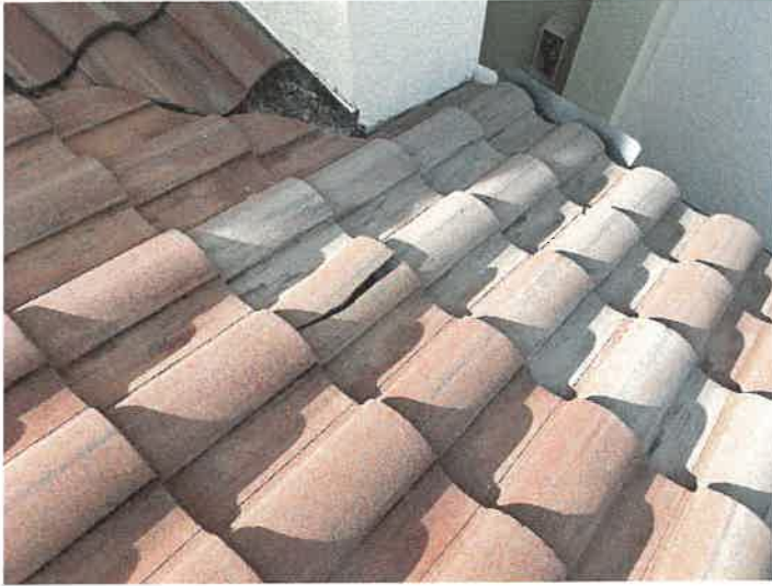
Building 15177: Identified Cracked Roof Tiles
