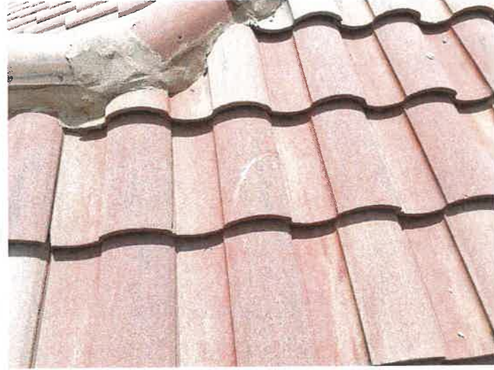
Building 15197: Repaired Cracked Roof Tiles
