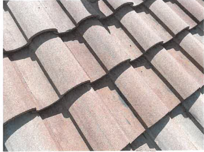
Building 15188: Repaired Displaced/Missing Roof Tile
