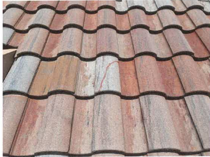
Building 15213: Repaired Cracked Roof Tiles
