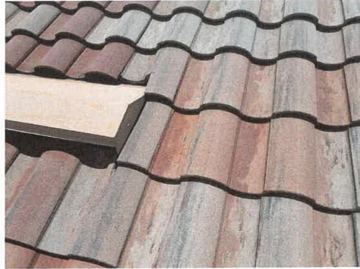
Building 15213: Repaired Displaced/Missing Roof Tile
