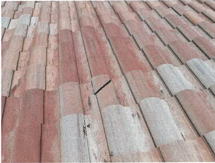
Building 15165: Identified Cracked Roof Tiles
