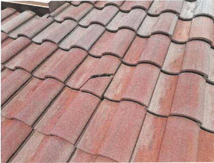
Building 15165: Identified Cracked Roof Tiles Cracked roof tiles can allow premature underlayment deterioration from excessive UV exposure.
