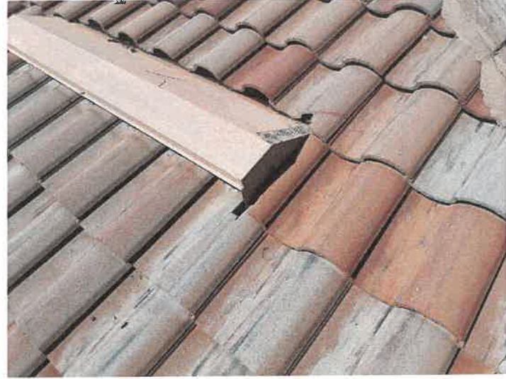
Building 15188: Repaired Displaced/Missing Roof Tile
