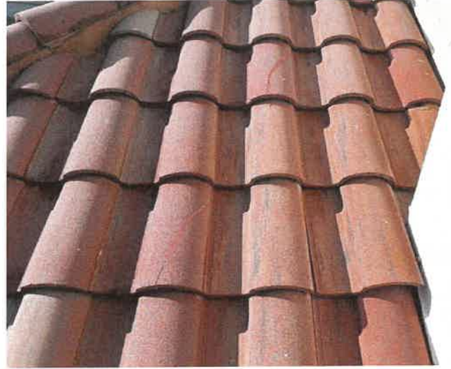
Building 15189: Repaired Cracked Roof Tiles
