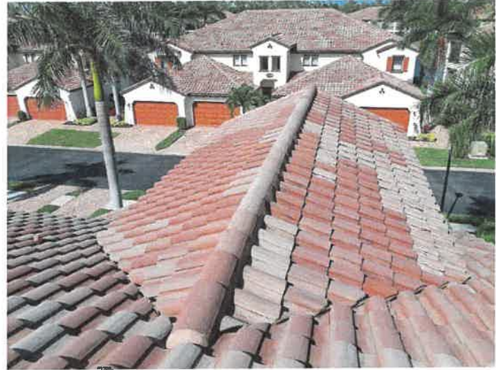
Building 15188: Valley The valley tiles appear to be in good condition.
