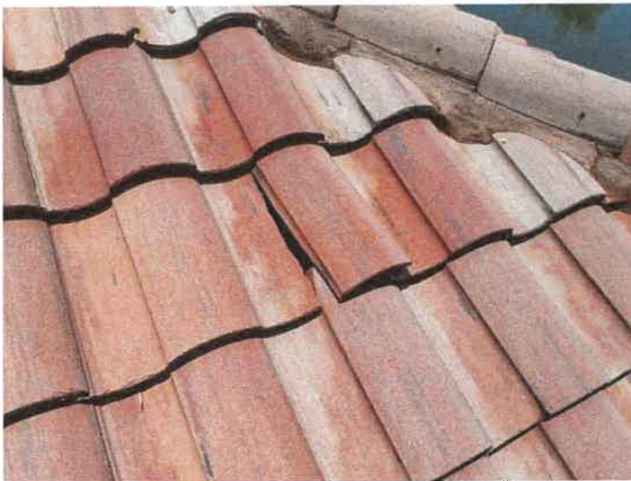
Building 15173: Identified Cracked Roof Tiles
