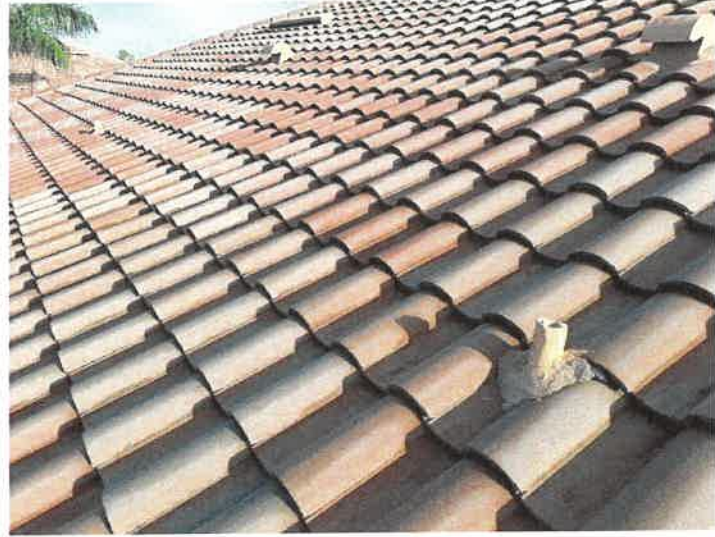
Building 15181: Lead Boots Lead boots appear to be in good condition.
