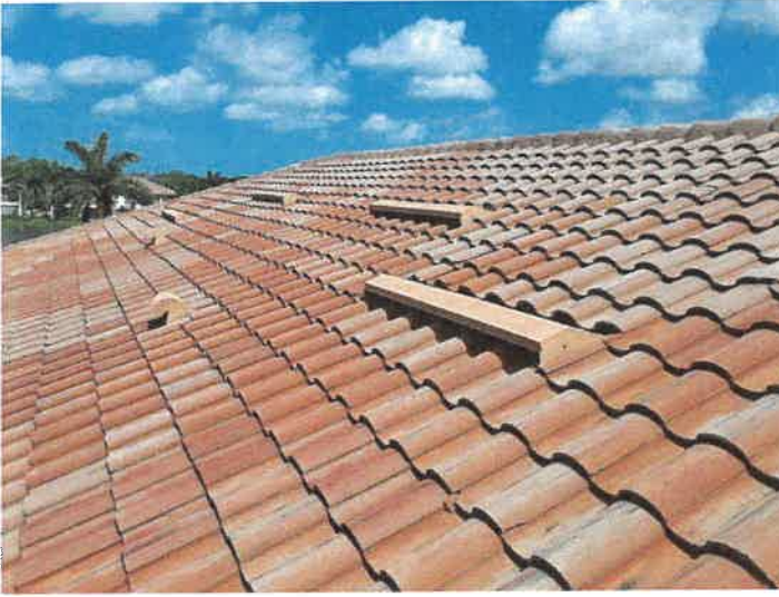
Building 15197: Roof Vents
