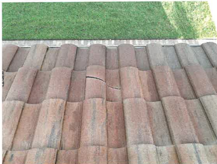
Building 15181: Identified Cracked Roof Tiles Cracked roof tiles can allow premature underlayment deterioration from excessive UV exposure.
