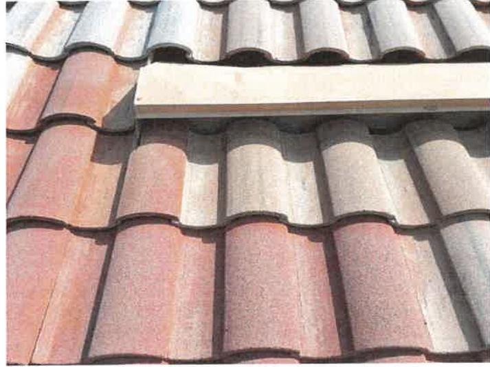
Building 15205: Repaired Displaced/Missing Roof Tile
