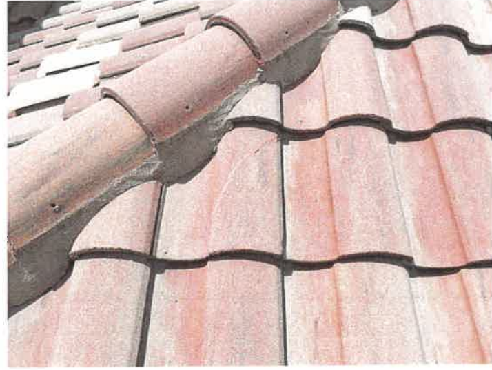
Building 15197: Repaired Cracked Roof Tiles
