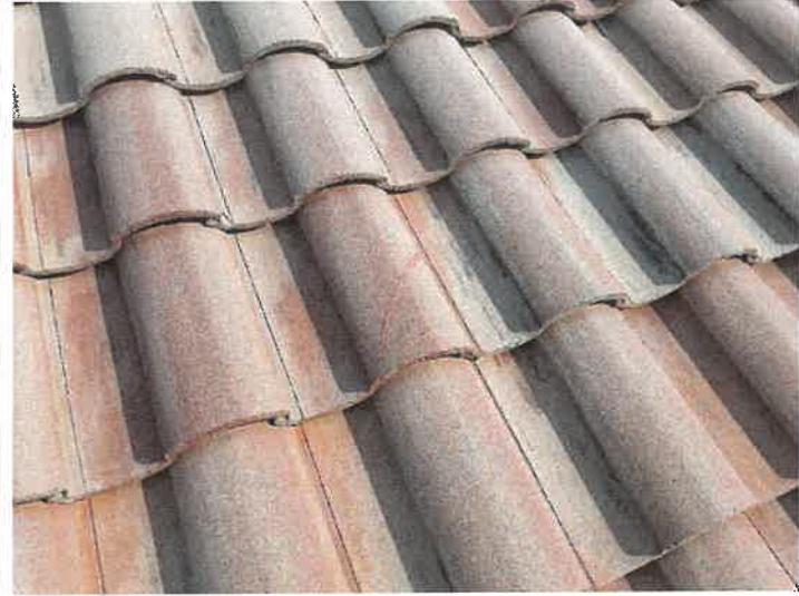
Building 15177: Repaired Cracked Roof Tiles
