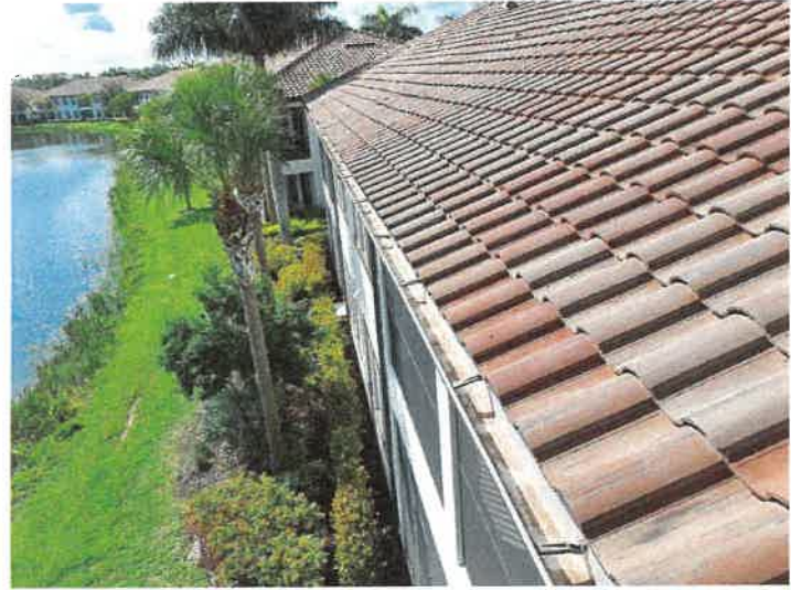
Building 15161: Gutters The gutters appear to be in good condition.
