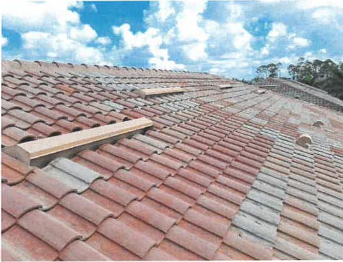
Building 15165: Roof Vents Roof vents appear to be in good condition.
