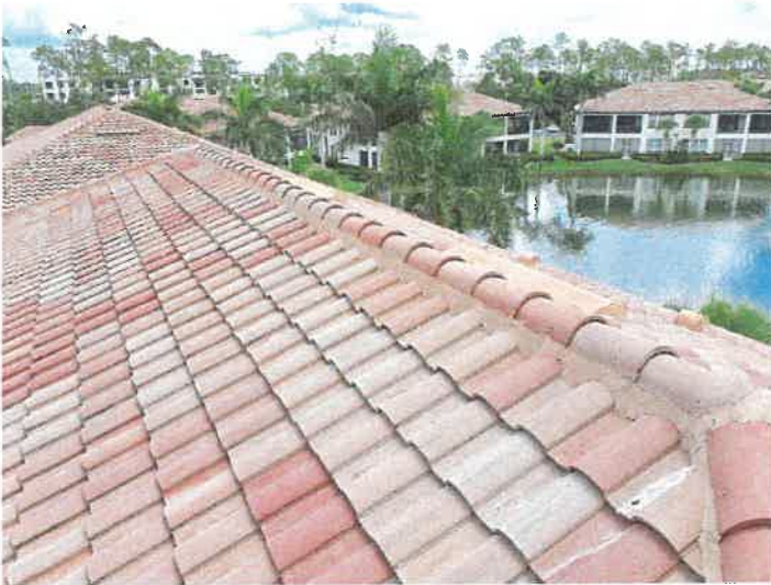
Building 15169: Ridge Tiles Ridge tiles appear to be in good condition.
