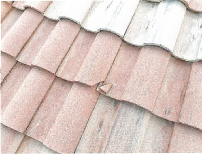
Building 15165: Identified Cracked Roof Tiles
