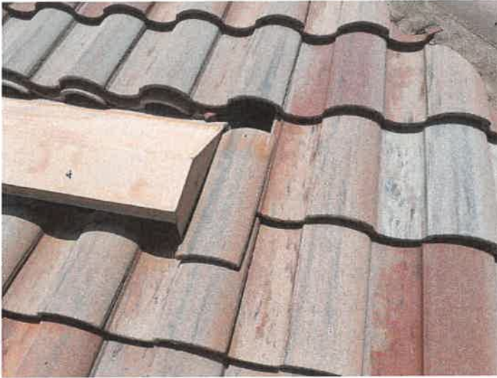
Building 15213: Displaced/Missing Roof Tile
