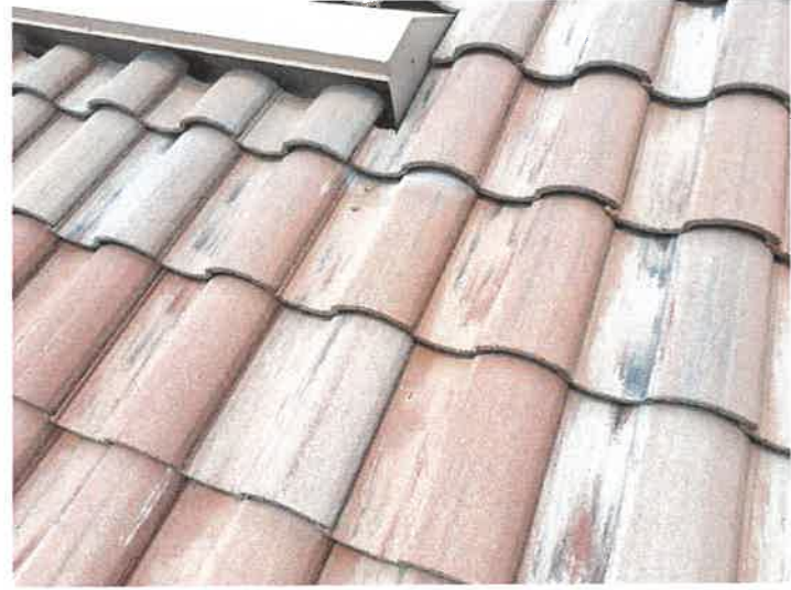
Building 15184: Repaired Displaced/Missing Roof Tile Replaced and secured the missing roof tile.
