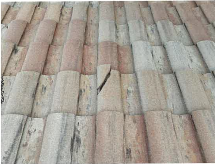
Building 15169: Identified Cracked Roof Tiles
