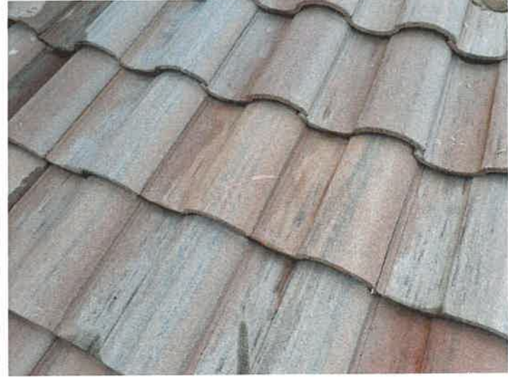
Building 15188: Repaired Cracked Roof Tiles
