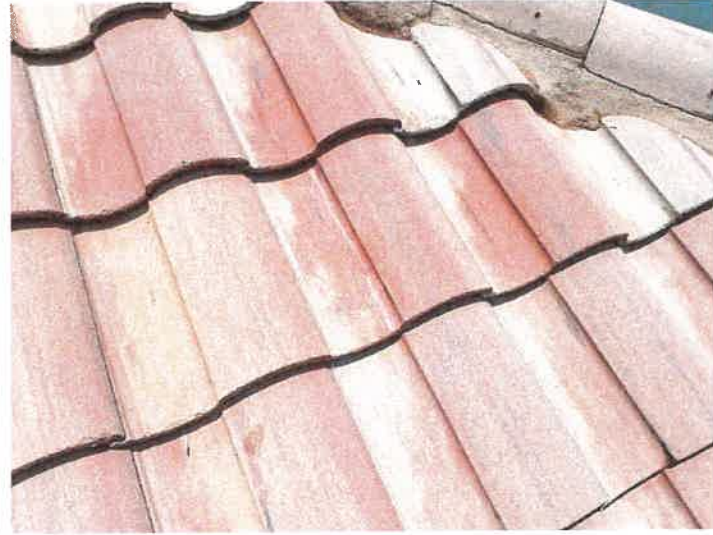
Building 15173: Repaired Cracked Roof Tiles
