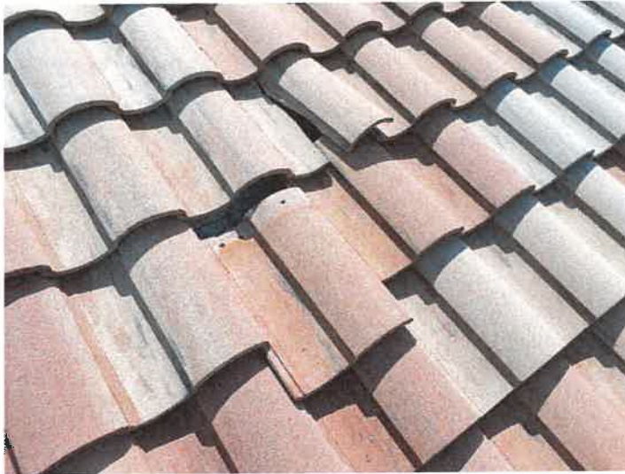
Building 15188: Displaced/Missing Roof Tile
