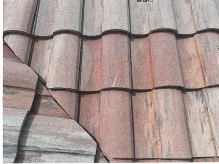
Building 15197: Repaired Cracked Roof Tiles The cracked roof tiles were repaired with Titebond sealant.
