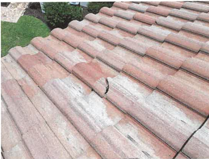
Building 15173: Identified Cracked Roof Tiles
