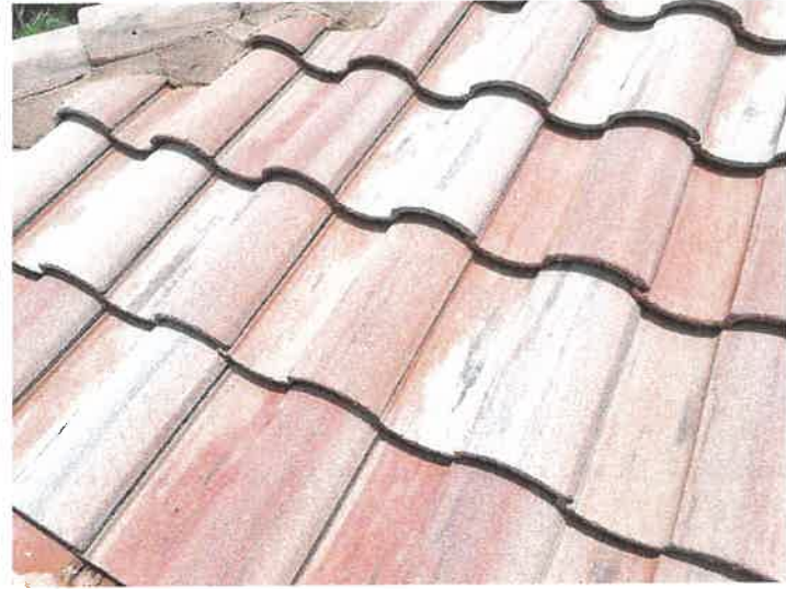
Building 15173: Repaired Displaced/Missing Roof Tile
