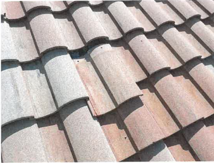
Building 15188: Displaced/Missing Roof Tile
