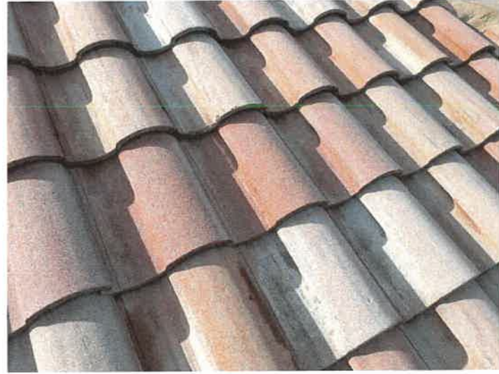
Building 15177: Repaired Cracked Roof Tiles
