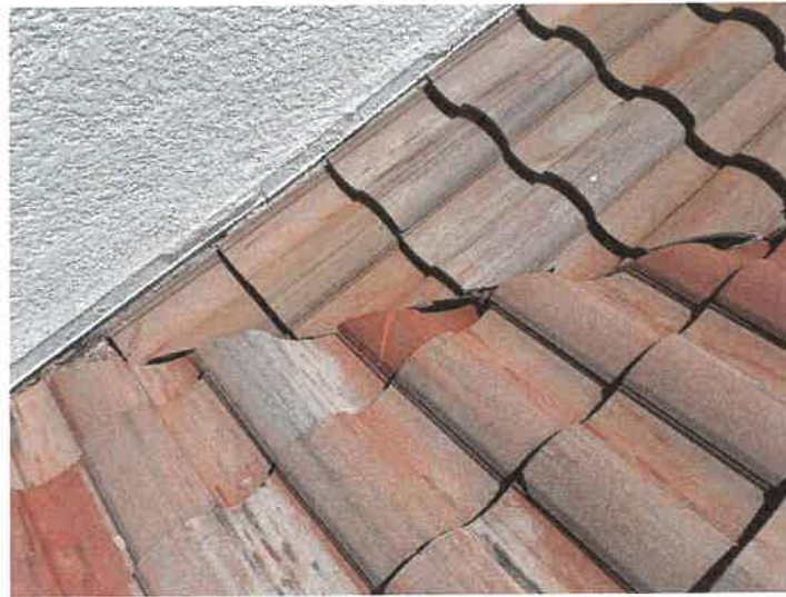
Building 15184: Repaired Cracked Roof Tiles
