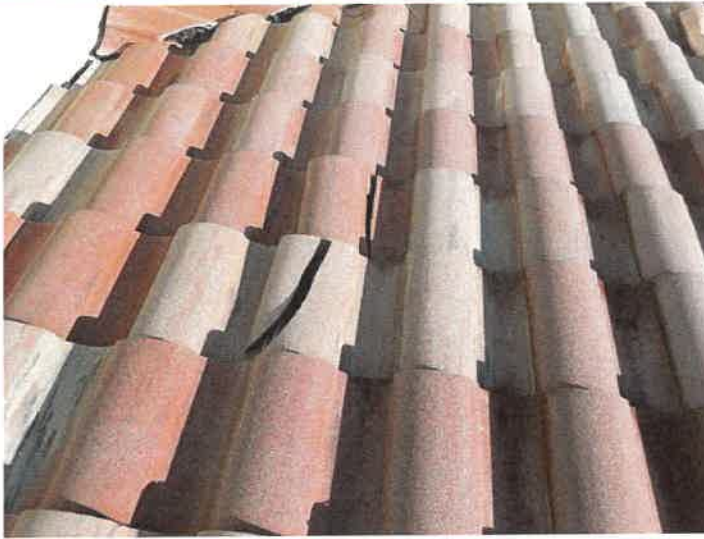
Building 15189: Identified Cracked Roof Tiles Cracked roof tiles can allow premature underlayment deterioration from excessive UV exposure.
