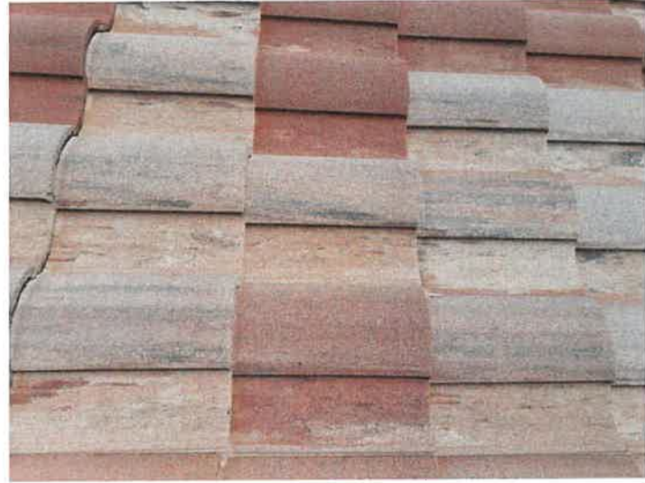
Building 15205: Repaired Displaced/Missing Roof Tile
