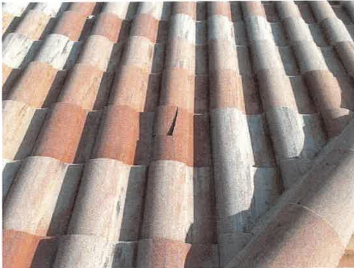
Building 15181: Identified Cracked Roof Tiles
