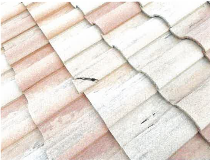
Building 15165: Identified Cracked Roof Tiles
