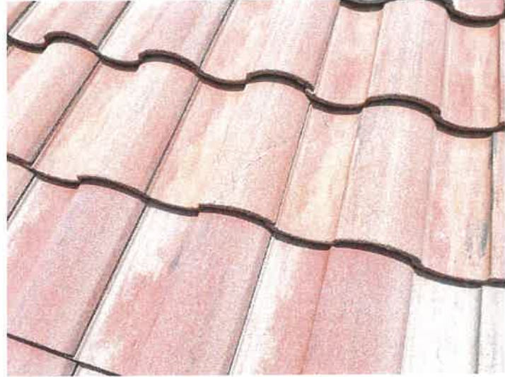
Building 15173: Repaired Cracked Roof Tiles
