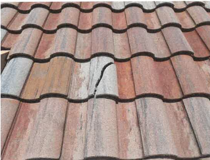
Building 15213: Identified Cracked Roof Tiles
