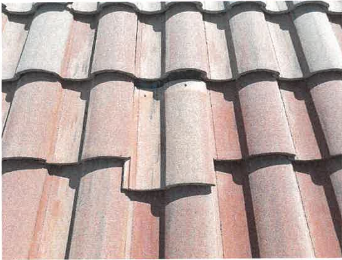
Building 15185: Displaced/Missing Roof Tile
