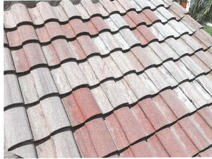
Building 15184: Repaired Cracked Roof Tiles
