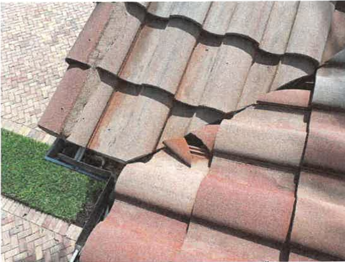
Building 15205: Identified Cracked Roof Tiles Cracked roof tiles can allow premature underlayment deterioration from excessive UV exposure.
