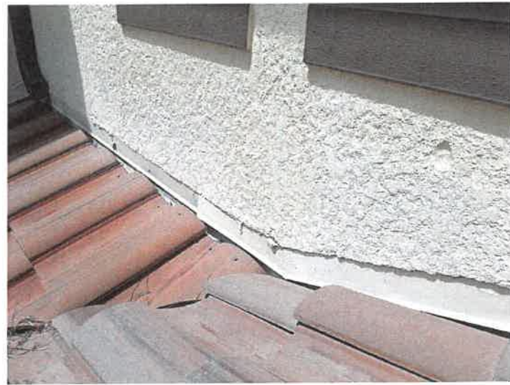
Building 15213: Counter Flashings
