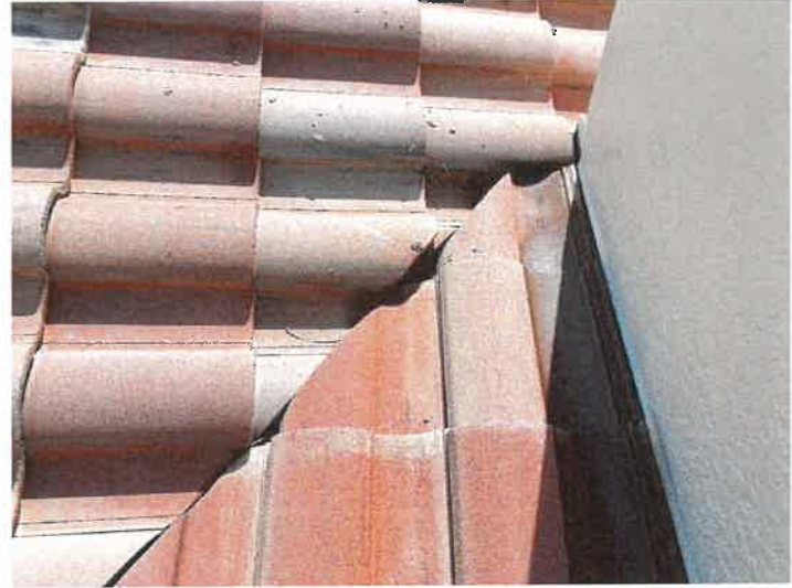
Building 15189: Repaired Cracked Roof Tiles The cracked roof tiles were repaired with Titebond sealant.
