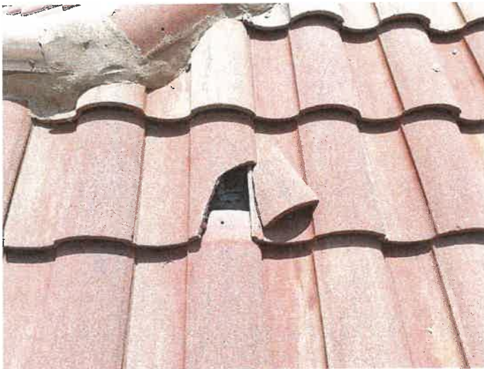
Building 15197: Identified Cracked Roof Tiles
