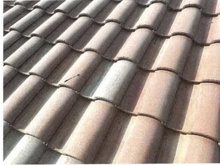
Building 15181: Repaired Displaced/Missing Roof Tile
