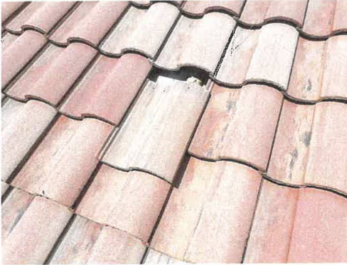
Displaced/Missing Roof Tile
