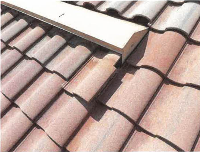
Building 15165: Displaced/Missing Roof Tile
