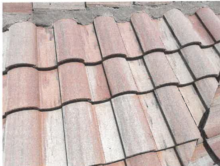
Building 15184: Repaired Displaced/Missing Roof Tile
