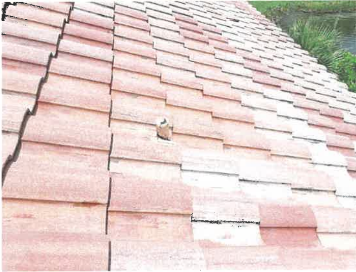
Building 15173: Lead Boots Lead boots appear to be in good condition.
