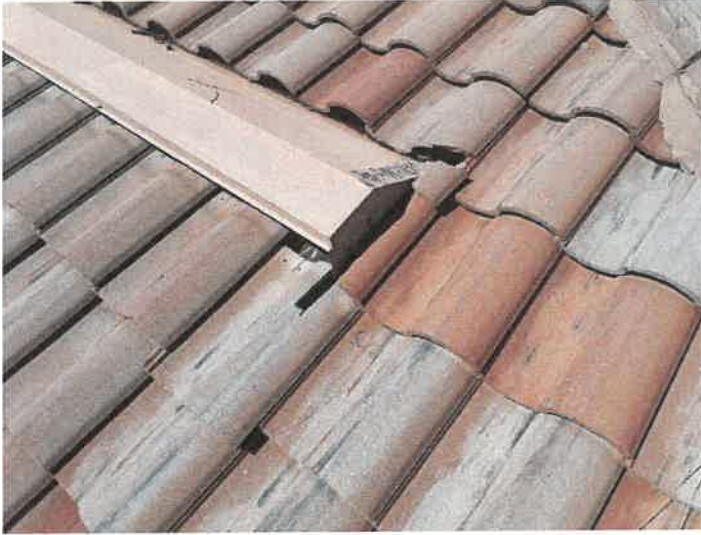
Building 15188: Displaced/Missing Roof Tile
