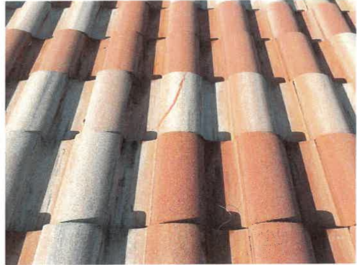
Building 15201: Repaired Cracked Roof Tiles
