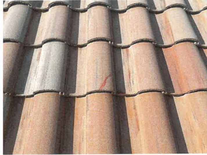
Building 15201: Repaired Cracked Roof Tiles The cracked roof tiles were repaired with Titebond sealant.
