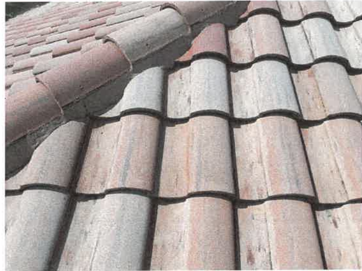
Building 15205: Repaired Displaced/Missing Roof Tile
