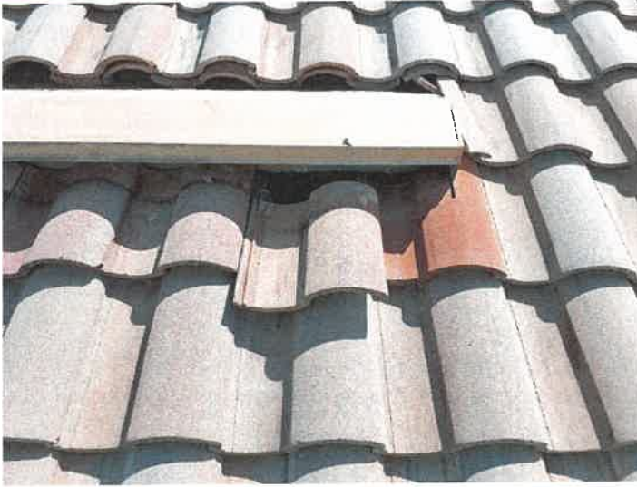
Building 15185: Displaced/Missing Roof Tile
