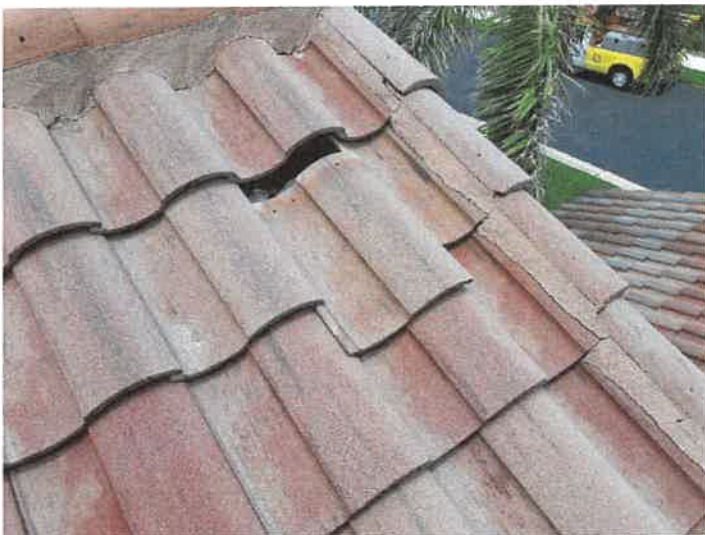
Building 15213: Displaced/Missing Roof Tile
