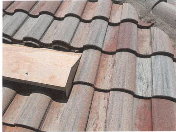
Building 15213: Repaired Displaced/Missing Roof Tile
