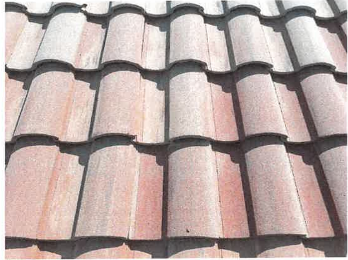
Building 15185: Repaired Displaced/Missing Roof Tile
