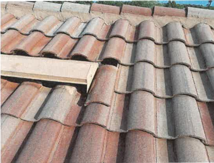
Building 15177: Displaced/Missing Roof Tile
