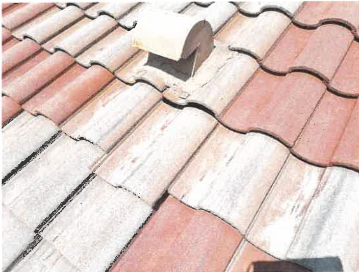
Building 15165: Displaced/Missing Roof Tile
