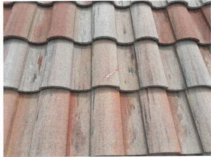
Building 15209: Repaired Cracked Roof Tiles
