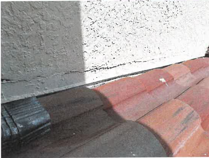
Building 15197: Counter Flashings
