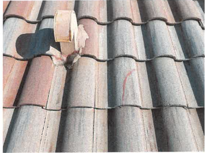
Building 15193: Repaired Displaced/Missing Roof Tile
