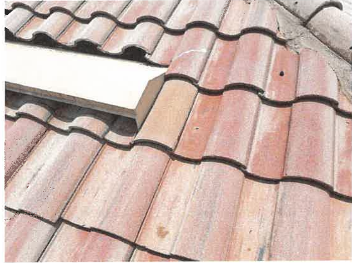
Building 15173: Repaired Displaced/Missing Roof Tile
