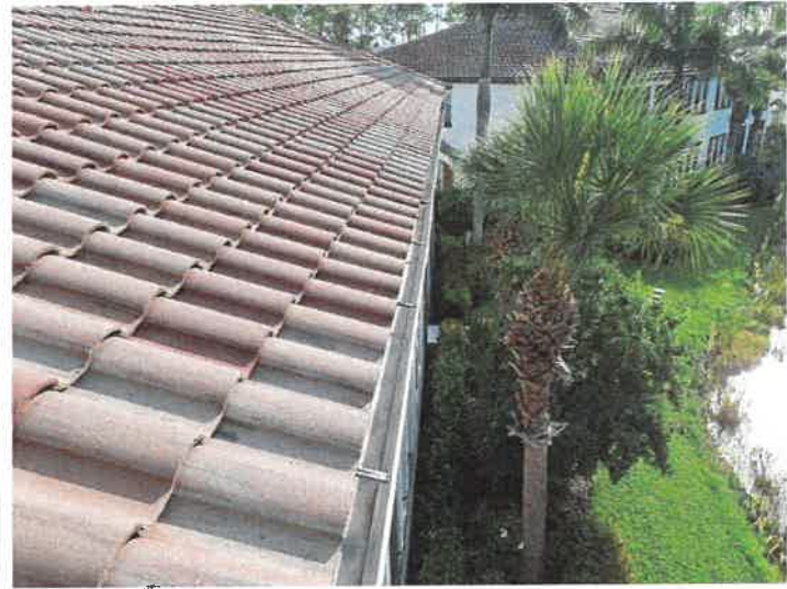
Building 15177: Gutters The gutters appear to be in good condition.
