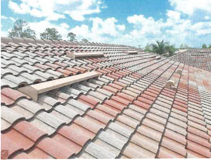
Building 15213: Roof Vents
