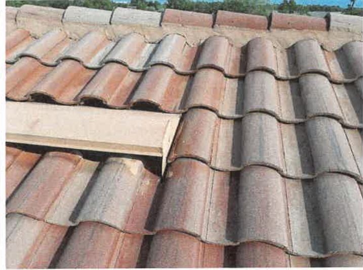
Building 15177: Repaired Displaced/Missing Roof Tile
