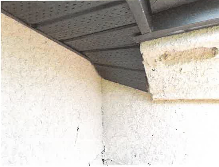
Building 15205: Loose Soffit Identified 2-feet of loose soffit.
