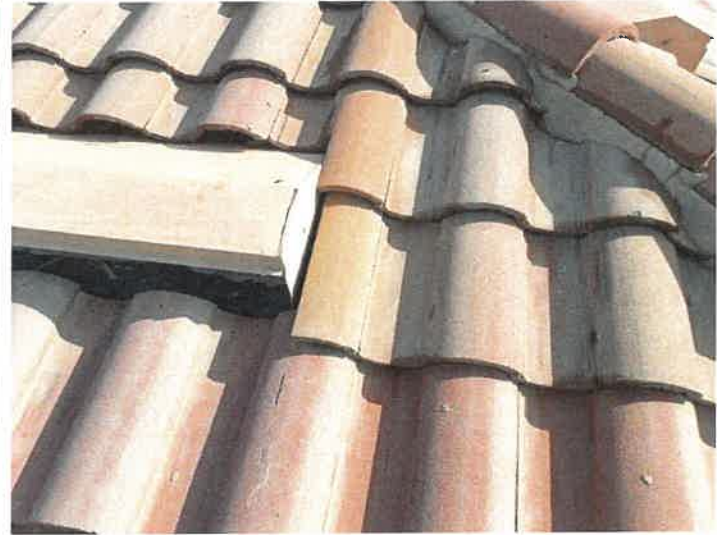
Building 15201: Repaired Displaced/Missing Roof Tile
