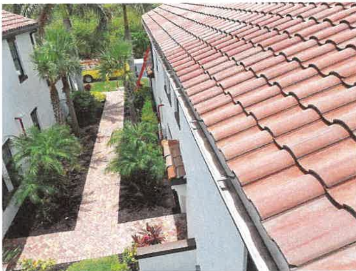
Building 15173: Gutters The gutters appear to be in good condition.
