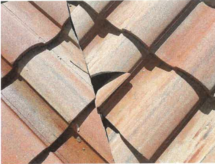
Building 15188: Identified Cracked Roof Tiles Cracked roof tiles can allow premature underlayment deterioration from excessive UV exposure.
