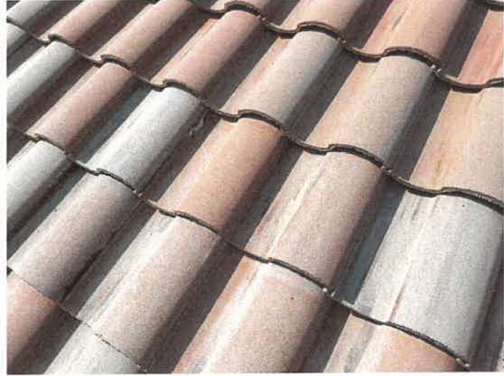
Building 15201: Repaired Displaced/Missing Roof Tile
