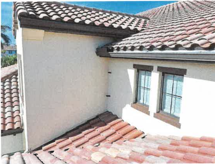
Building 15193: Identified Cracked Roof Tiles Cracked roof tiles can allow premature underlayment deterioration from excessive UV exposure.
