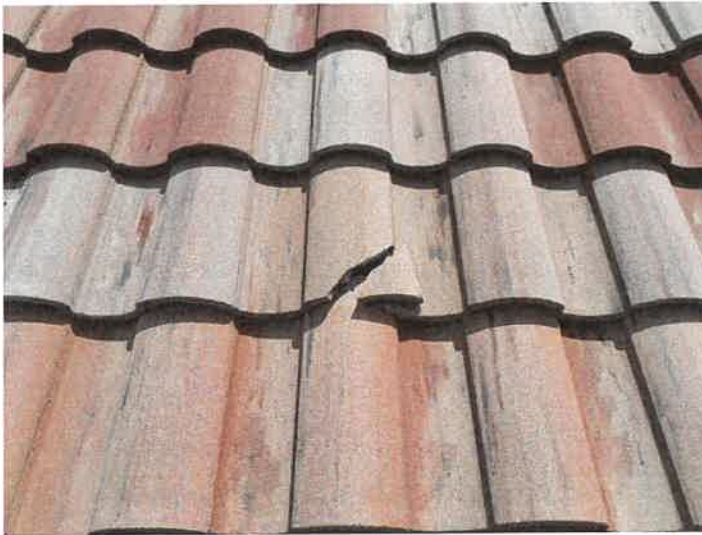
Building 15209: Identified Cracked Roof Tiles
