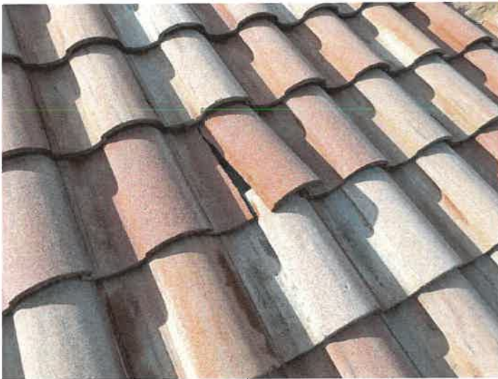
Building 15177: Identified Cracked Roof Tiles
