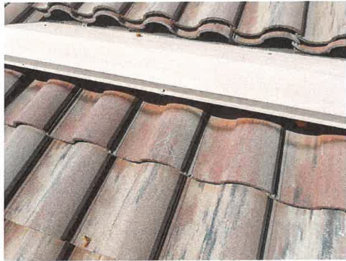
Building 15161: Repaired Displaced/Missing Roof Tile
