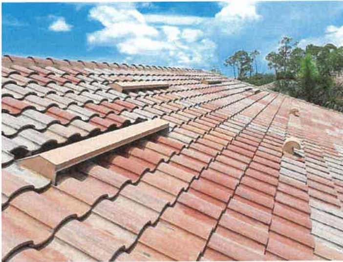
Building 15173: Identified Cracked Roof Tiles Cracked roof tiles can allow premature underlayment deterioration from excessive UV exposure.
