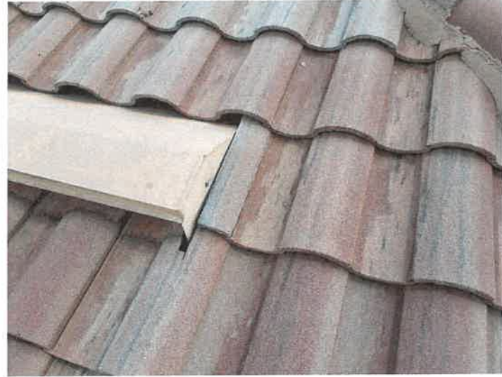
Building 15165: Repaired Displaced/Missing Roof Tile
