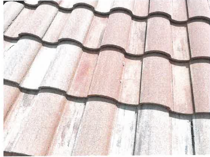
Building 15184: Repaired Displaced/Missing Roof Tile
