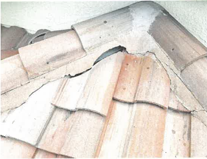
Building 15169: Displaced/Missing Roof Tile
