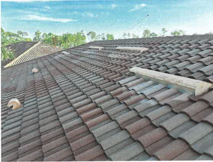
Building 15189: Roof Vents Roof vents appear to be in good condition.
