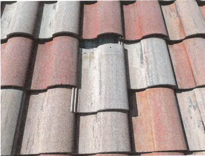
Building 15205: Displaced/Missing Roof Tile
