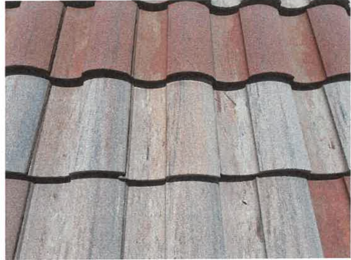
Building 15213: Repaired Displaced/Missing Roof Tile
