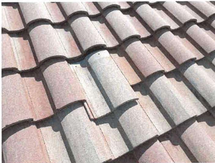
Building 15185: Identified Cracked Roof Tiles Cracked roof tiles can allow premature underlayment deterioration from excessive UV exposure.
