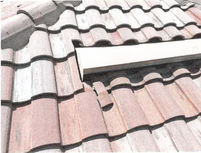
Building 15184: Identified Cracked Roof Tiles Cracked roof tiles can allow premature underlayment deterioration from excessive UV exposure.
