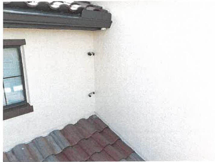
Building 15165: Downspout- missing
