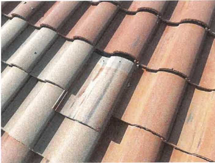
Building 15201: Displaced/Missing Roof Tile
