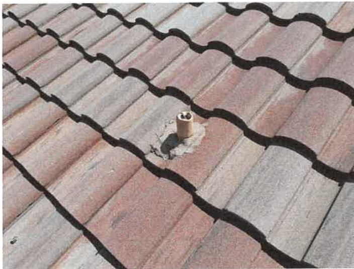
Building 15184: Lead Boots Lead boots appear to be in good condition.
