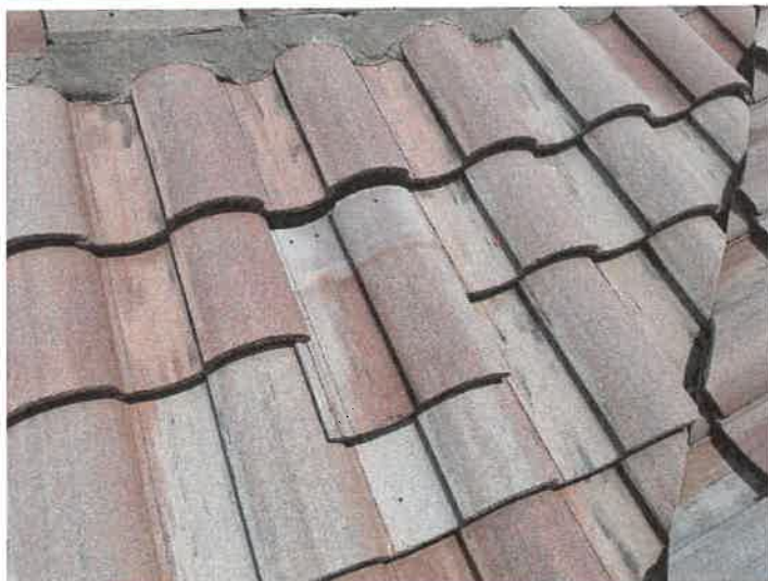
Building 15184: Displaced/Missing Roof Tile
