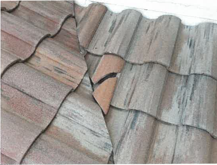
Building 15161: Identified Cracked Roof Tiles Cracked roof tiles can allow premature underlayment deterioration from excessive UV exposure.
