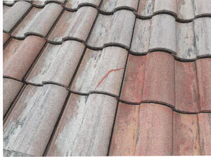
Building 15209: Repaired Cracked Roof Tiles
