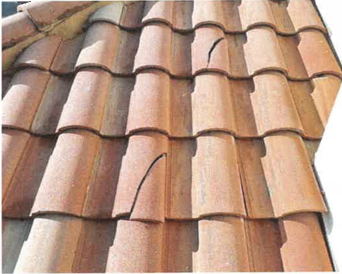
Building 15189: Identified Cracked Roof Tiles
