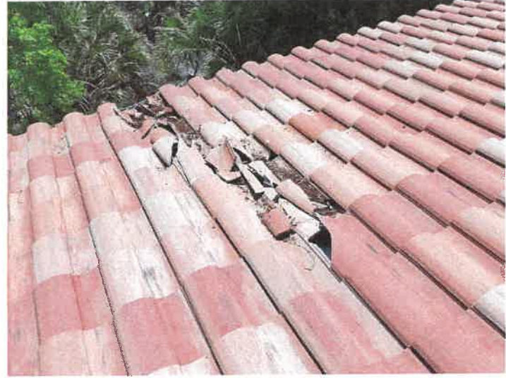
Building 15188: Broken Roof Tiles Crowther Roofing suggests replacing 15 cracked roof tiles.
