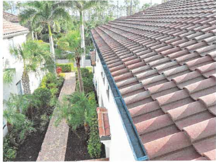
Building 15201: Gutter Metal- Broken Gutter is broken and needs to be replaced. (1ft.6" residential model).
