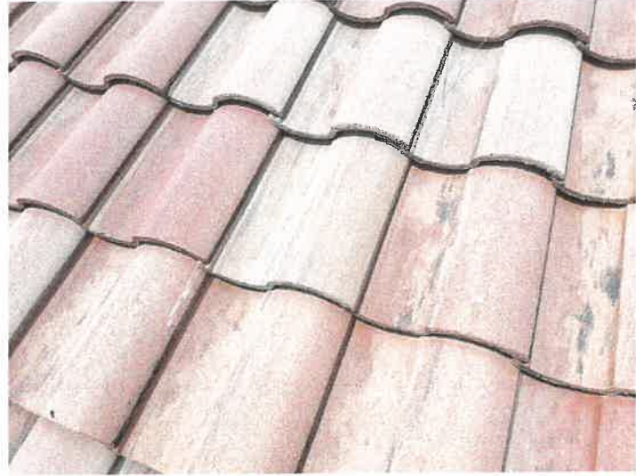
Repaired Displaced/Missing Roof Tile
