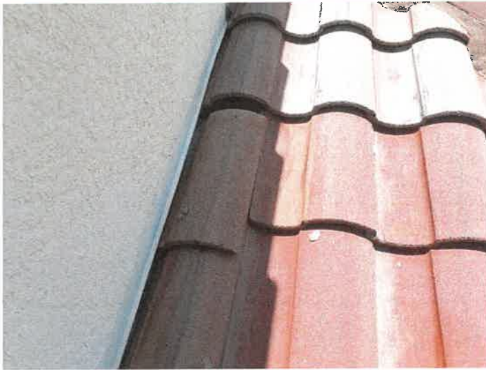
Building 15213: Displaced/Missing Roof Tile
