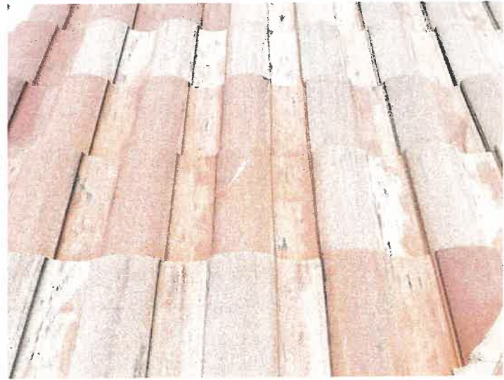
Building 15205: Repaired Cracked Roof Tiles
