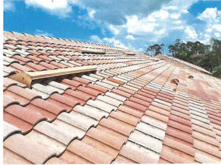
Building 15169: Roof Vents
