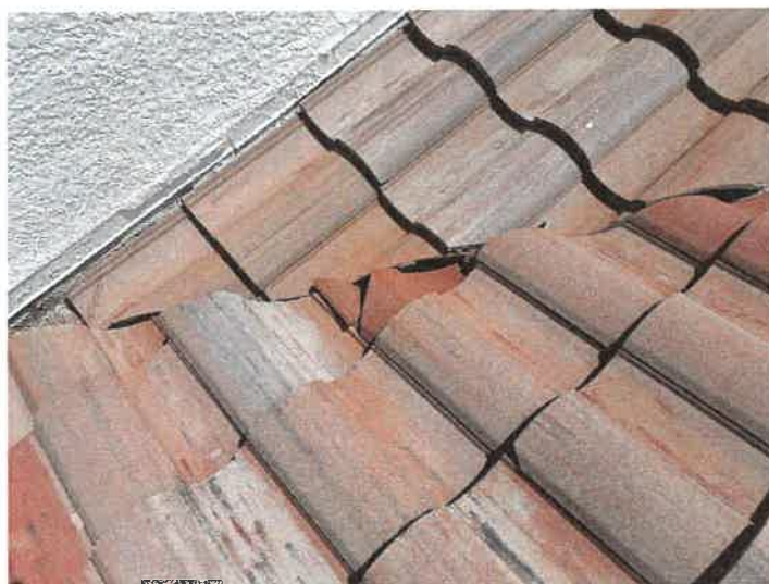
Building 15184: Identified Cracked Roof Tiles
