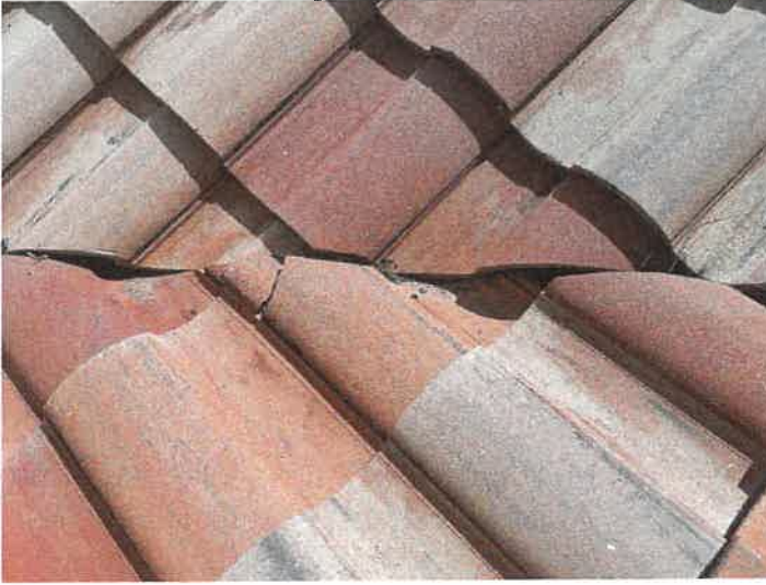
Building 15205: Identified Cracked Roof Tiles Cracked roof tiles can allow premature underlayment deterioration from excessive UV exposure.
