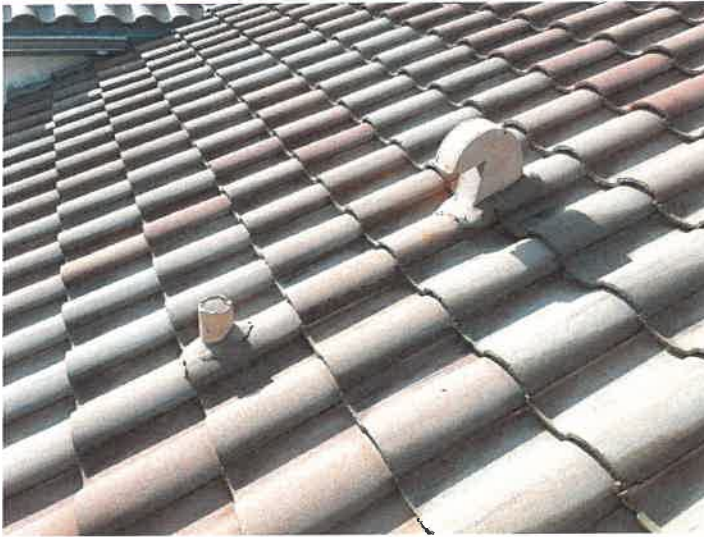
Building 15201: Lead Boots Lead boots appear to be in good condition.
