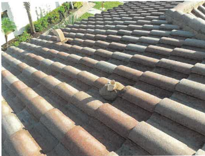
Building 15189: Lead Boots Lead boots appear to be in good condition.
