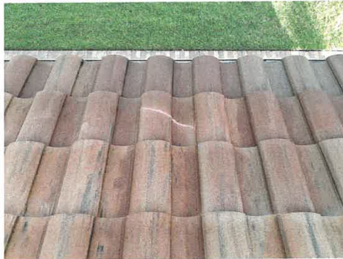
Building 15181: Repaired Cracked Roof Tiles The cracked roof tiles were repaired with Titebond sealant.
