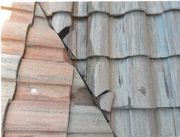
Building 15188: Identified Cracked Roof Tiles Cracked roof tiles can allow premature underlayment deterioration from excessive UV exposure.
