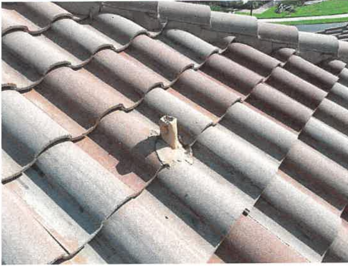
Building 15193: Lead Boots Lead boots appear to be in good condition.
