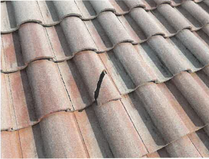
Building 15177: Identified Cracked Roof Tiles
