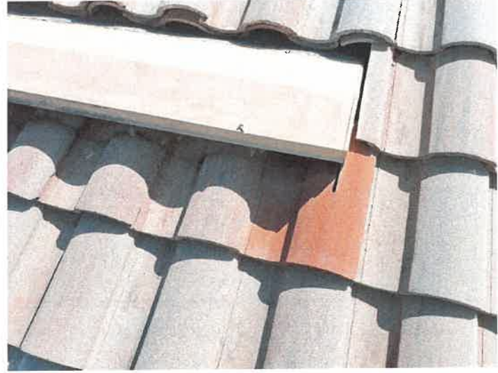
Building 15185: Repaired Displaced/Missing Roof Tile
