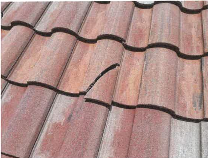
Building 15173: Identified Cracked Roof Tiles
