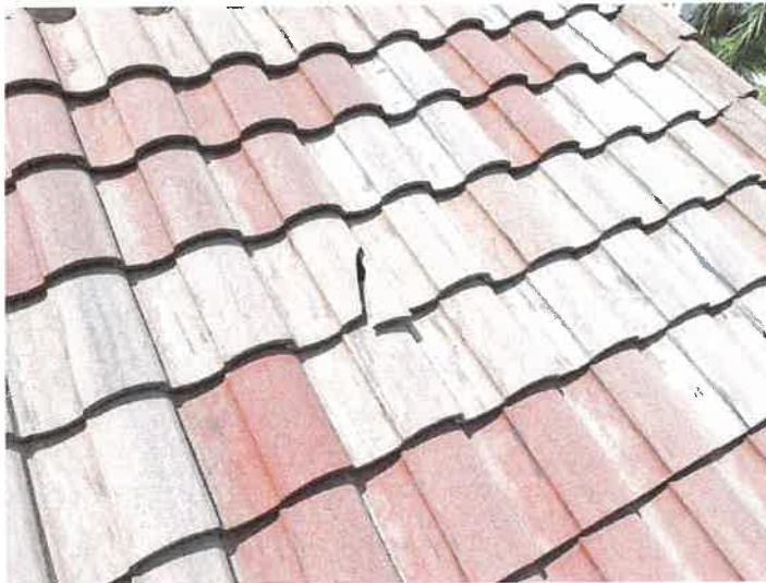
Building 15184: Identified Cracked Roof Tiles
