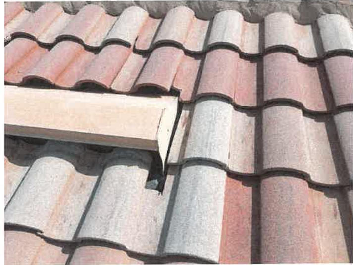
Building 15205: Repaired Displaced/Missing Roof Tile
