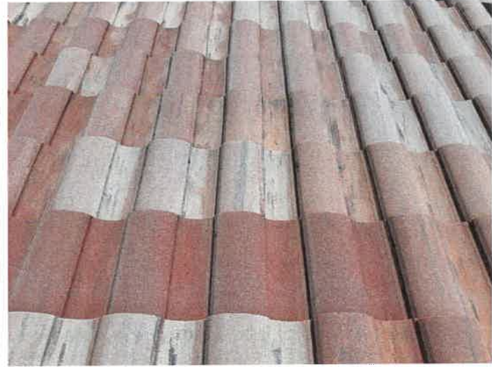
Building 15193: Repaired Cracked Roof Tiles
