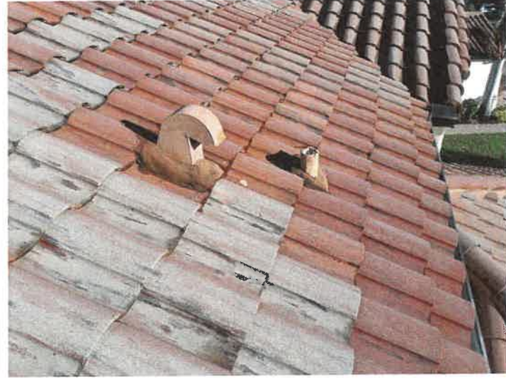
Building 15189: Lead Boots Lead boots appear to be in good condition.
