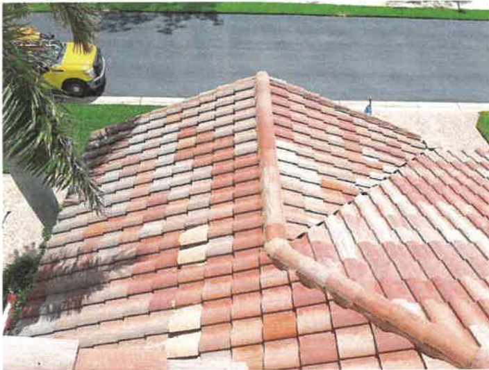
Building 15213: Surface Overview - Lower Roof The roof surface appears to be in good, maintainable condition at this time.
