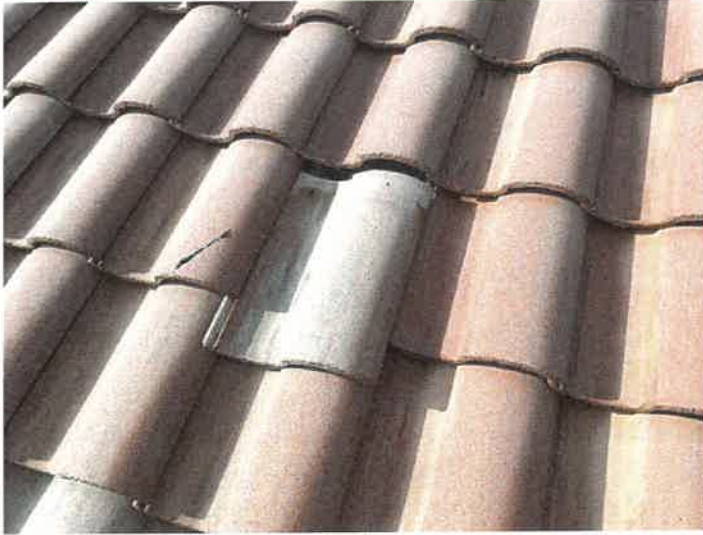
Building 15181: Displaced/Missing Roof Tile
