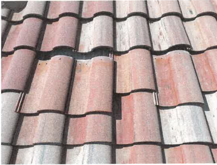
Building 15205: Displaced/Missing Roof Tile
