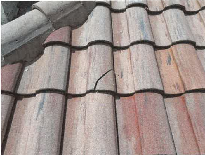
Building 15197: Identified Cracked Roof Tiles Cracked roof tiles can allow premature underlayment deterioration from excessive UV exposure.
