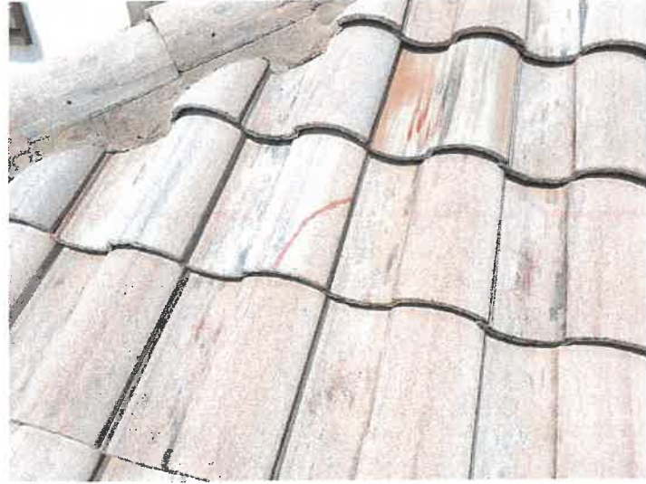
Building 15209: Repaired Cracked Roof Tiles Repaired cracked roof tiles with M1 sealant
