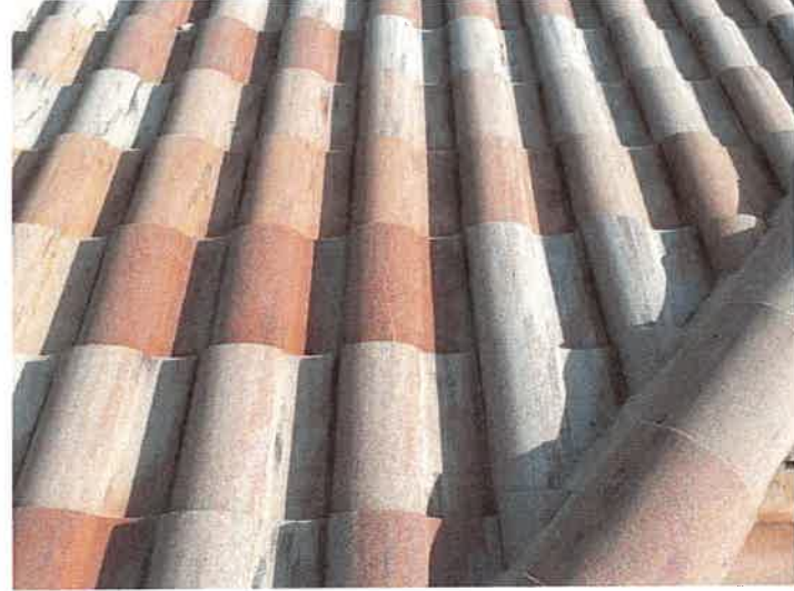
Building 15181: Repaired Cracked Roof Tiles
