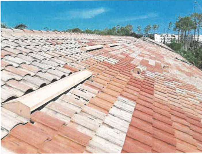
Building 15188: Roof Vents Roof vents appear to be in good condition.
