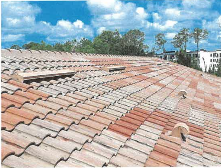
Building 15184: Roof Vents Roof vents appear to be in good condition.
