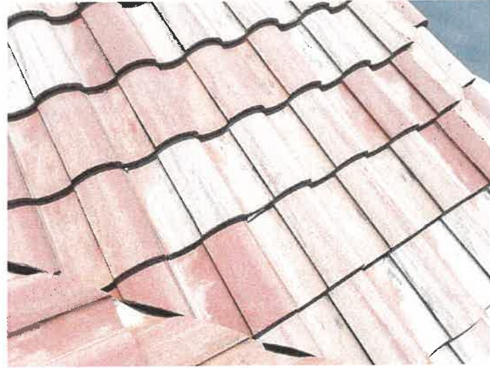
Building 15173: Repaired Cracked Roof Tiles The cracked roof tiles were repaired with Titebond sealant.
