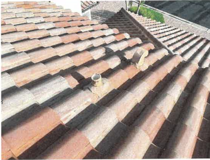
Building 15181: Lead Boots Lead boots appear to be in good condition.
