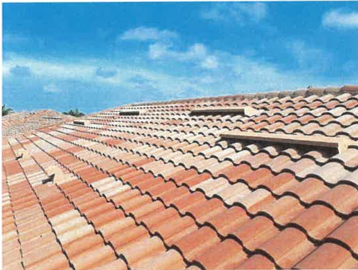
Building 15205: Roof Vents
