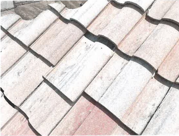
Building 15169: Displaced/Missing Roof Tile
