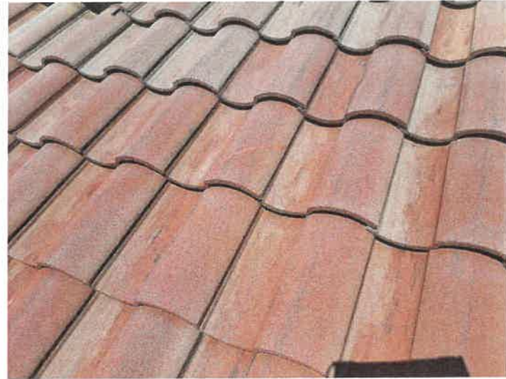
Building 15165: Repaired Cracked Roof Tiles The cracked roof tiles were repaired with Titebond sealant.
