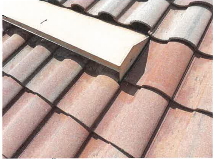
Building 15165: Repaired Displaced/Missing Roof Tile
