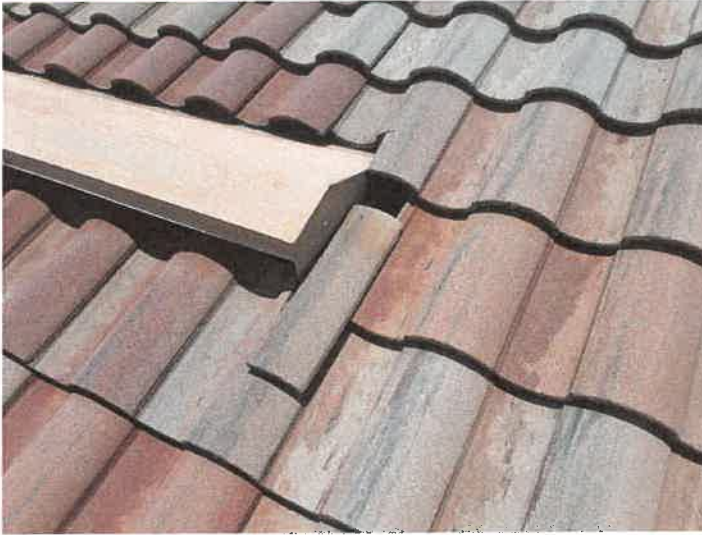
Building 15213: Displaced/Missing Roof Tile
