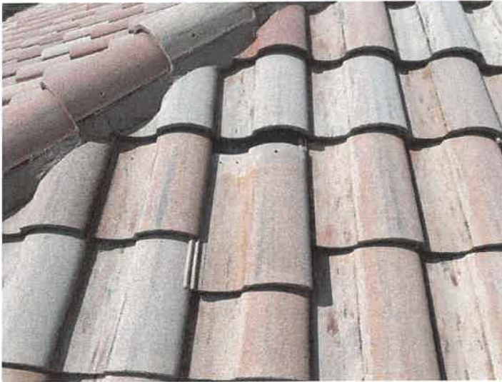
Building 15205: Displaced/Missing Roof Tile
