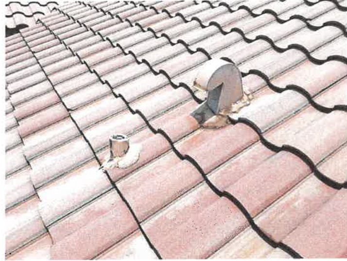
Building 15173: Lead Boots Lead boots appear to be in good condition.
