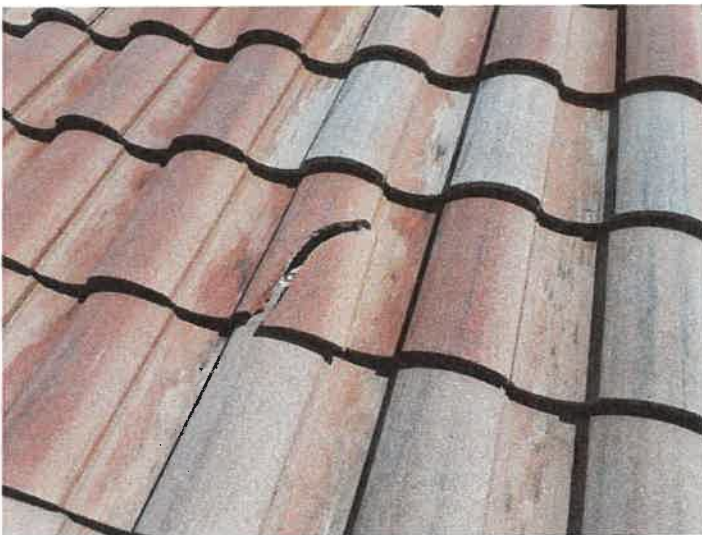
Building 15165: Identified Cracked Roof Tiles Cracked roof tiles can allow premature underlayment deterioration from excessive UV exposure.
