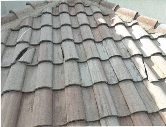
Building 15177: Identified Cracked Roof Tiles Cracked roof tiles can allow premature underlayment deterioration from excessive UV exposure.
