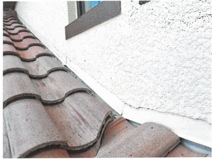
Building 15169: Counter Flashings
