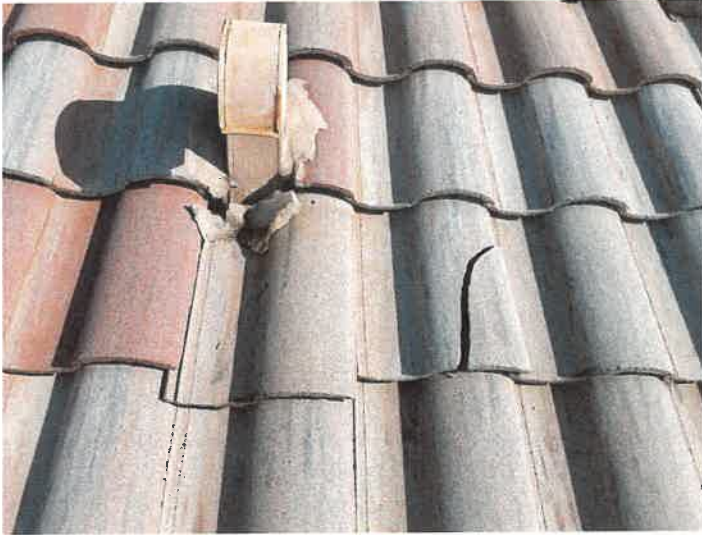
Building 15193: Displaced/Missing Roof Tile
