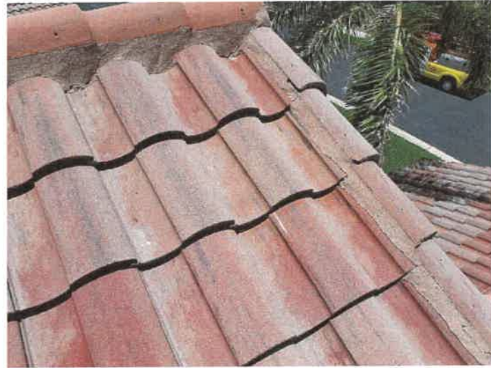
Building 15213: Repaired Displaced/Missing Roof Tile
