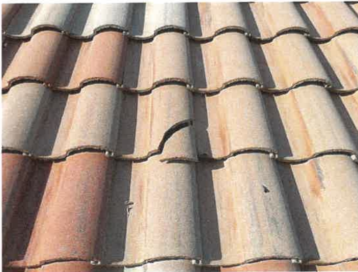
Building 15201: Identified Cracked Roof Tiles
