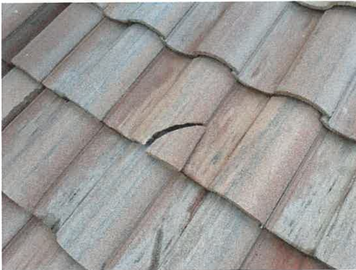
Building 15188: Identified Cracked Roof Tiles
