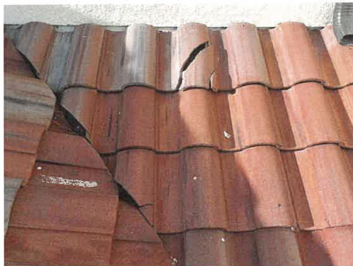
Building 15181: Identified Cracked Roof Tiles Cracked roof tiles can allow premature underlayment deterioration from excessive UV exposure.
