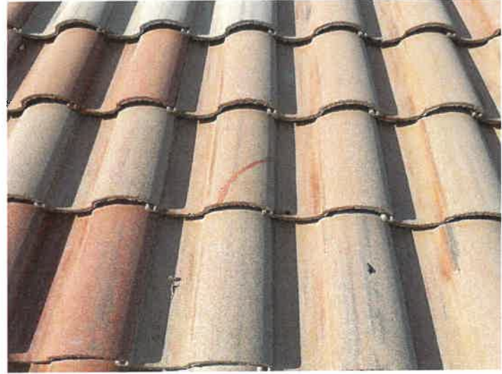
Building 15201: Repaired Cracked Roof Tiles
