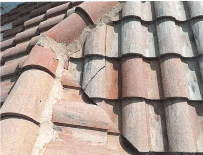
Building 15161: Identified Cracked Roof Tiles Cracked roof tiles can allow premature underlayment deterioration from excessive UV exposure.
