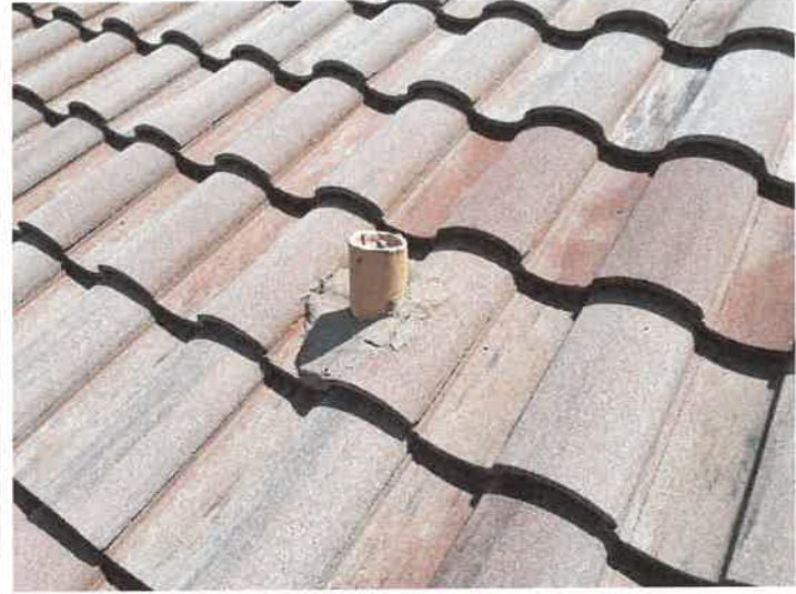
Building 15184: Lead Boots Lead boots appear to be in good condition.
