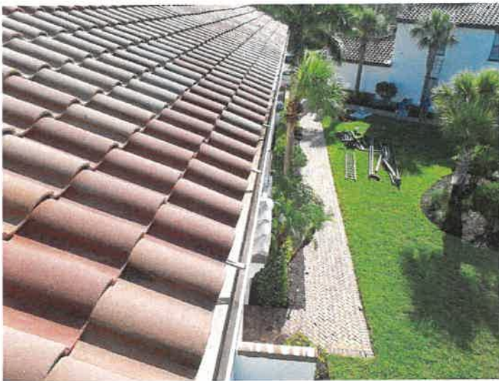
Building 15193: Gutters The gutters appear to be in good condition.
