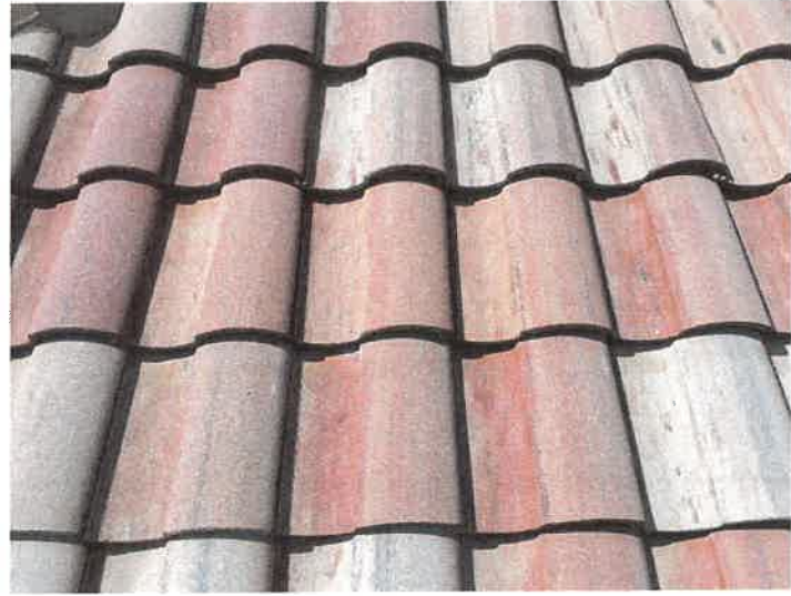
Building 15205: Repaired Displaced/Missing Roof Tile
