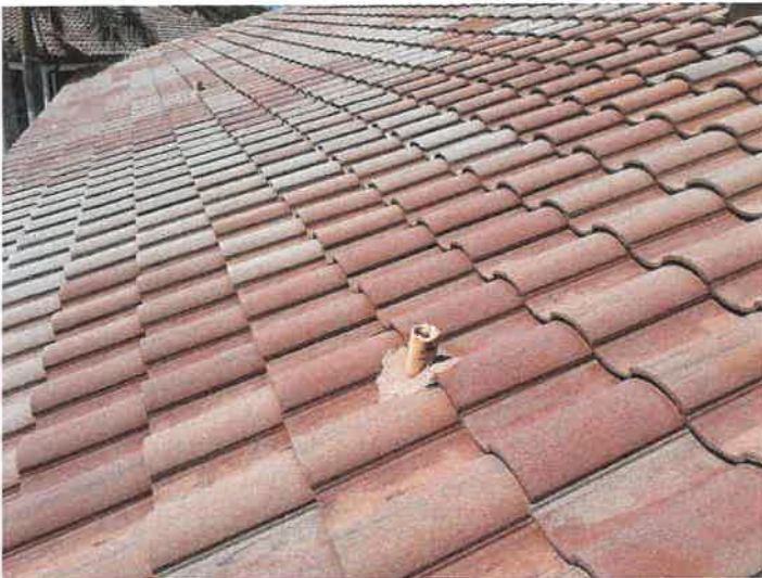
Building 15165: Lead Boots Lead boots appear to be in good condition.
