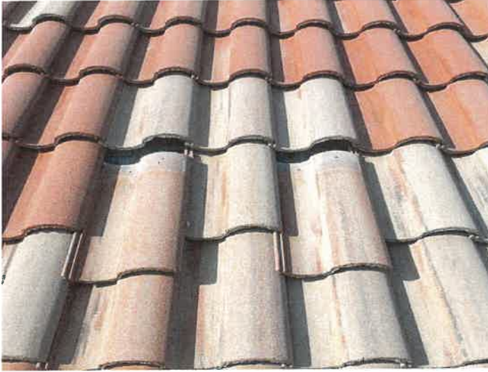
Building 15201: Displaced/Missing Roof Tile
