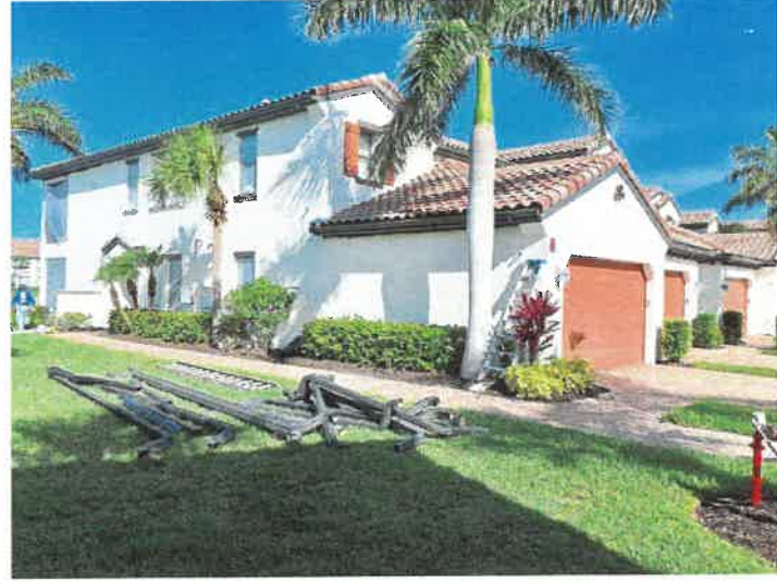
Building 15193: Downspout- missing Downspout is missing. The painting company that is painting the exteriors in Livingston Lakes has the missing downspouts.
