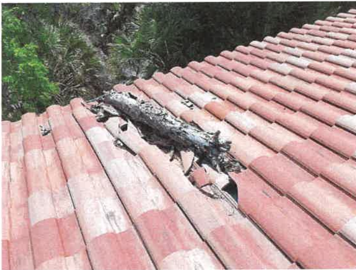
Building 15188: Debris on Roof Identified debris on the surface of the roof that could damage the membrane.
