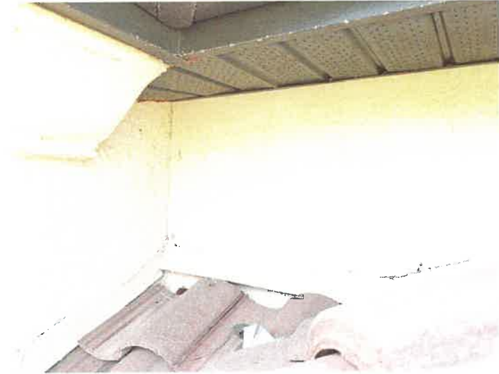
Building 15205: Completed Repair Soffit was properly secured back into place.
