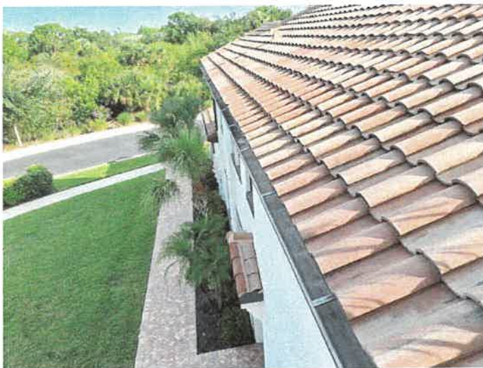
Building 15177: Gutters The gutters appear to be in good condition.
