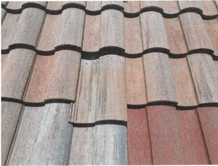
Building 15213: Displaced/Missing Roof Tile
