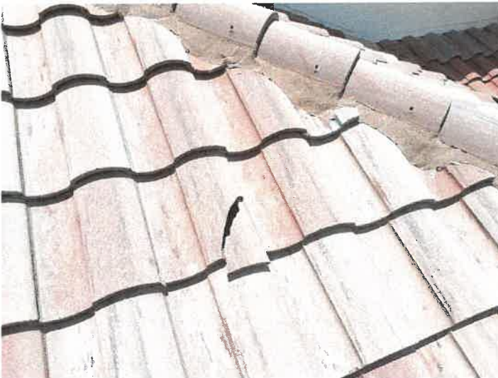
Building 15213: Identified Cracked Roof Tiles
