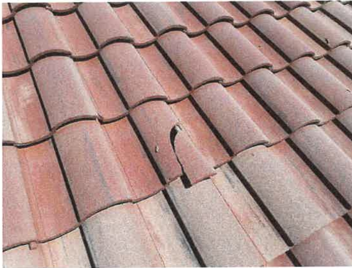
Building 15185: Identified Cracked Roof Tiles
