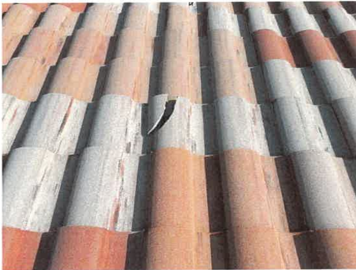
Building 15201: Identified Cracked Roof Tiles Cracked roof tiles can allow premature underlayment deterioration from excessive UV exposure.
