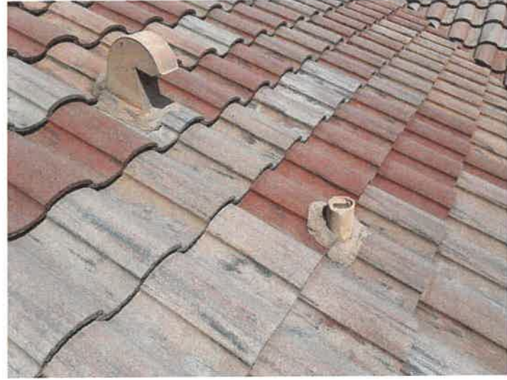
Building 15209: Lead Boots Lead boots appear to be in good condition.
