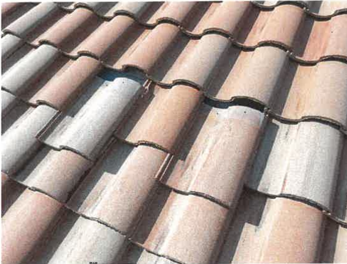
Building 15201: Displaced/Missing Roof Tile
