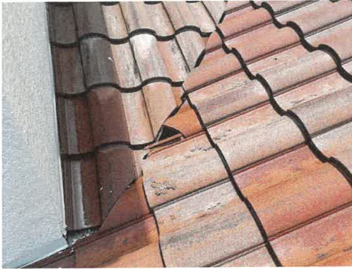
Building 15169: Identified Cracked Roof Tiles Cracked roof tiles can allow premature underlayment deterioration from excessive UV exposure.
