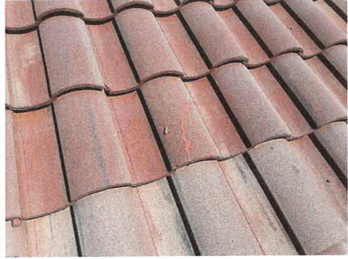
Building 15185: Repaired Cracked Roof Tiles
