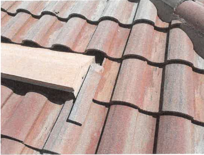
Building 15165: Displaced/Missing Roof Tile
