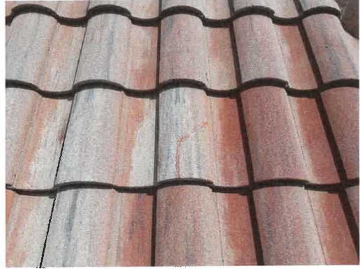
Building 15197: Repaired Cracked Roof Tiles
