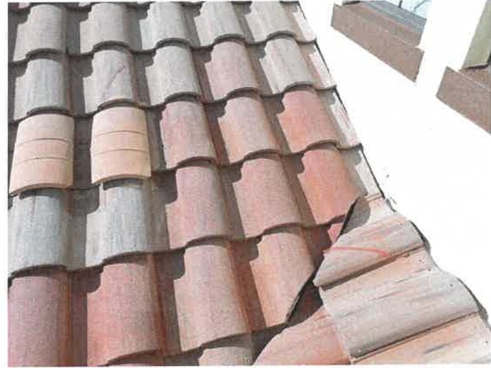
Building 15193: Repaired Cracked Roof Tiles The cracked roof tiles were repaired with Titebond sealant.
