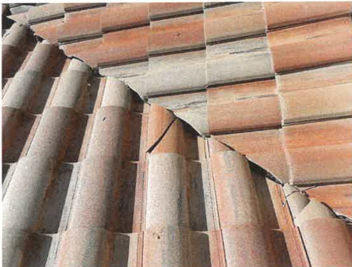
Building 15189: Identified Cracked Roof Tiles
