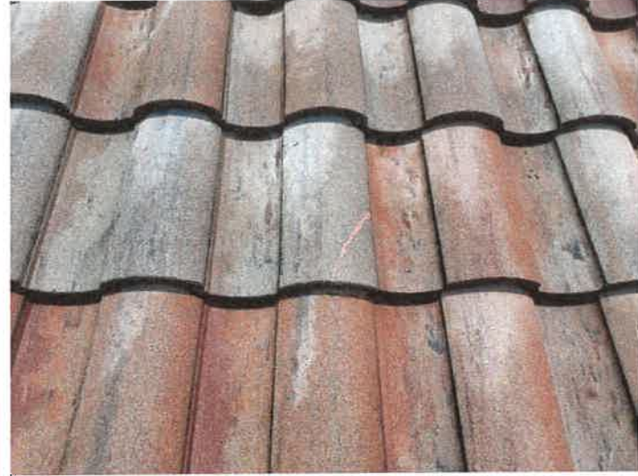
Building 15169: Repaired Cracked Roof Tiles The cracked roof tiles were repaired with Titebond sealant.
