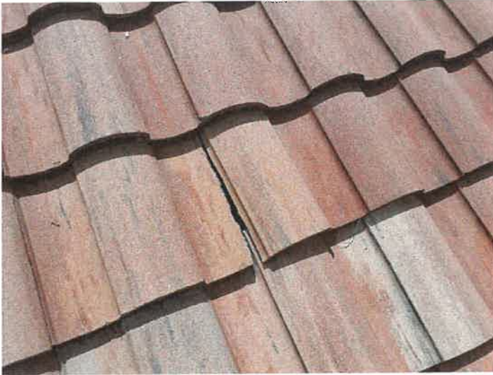
Building 15197: Identified Cracked Roof Tiles Cracked roof tiles can allow premature underlayment deterioration from excessive UV exposure.
