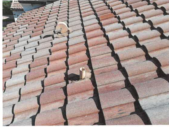
Building 15188: Lead Boots Lead boots appear to be in good condition.
