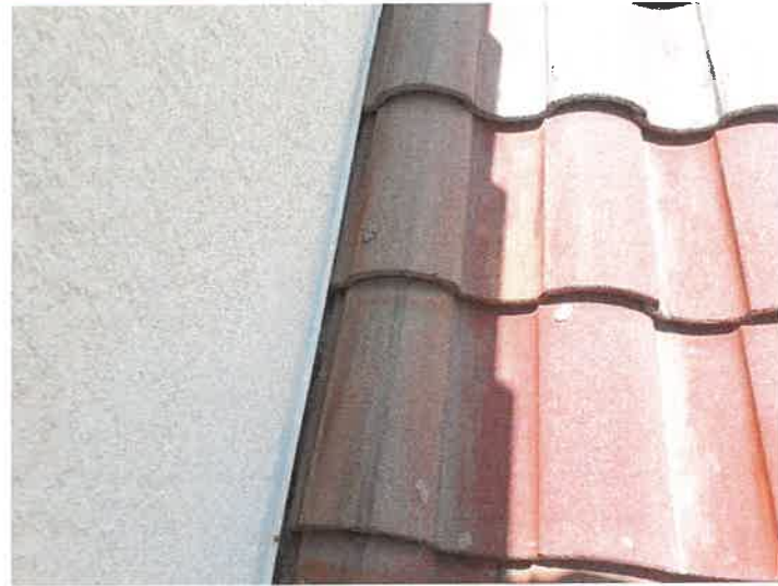
Building 15213: Repaired Displaced/Missing Roof Tile
