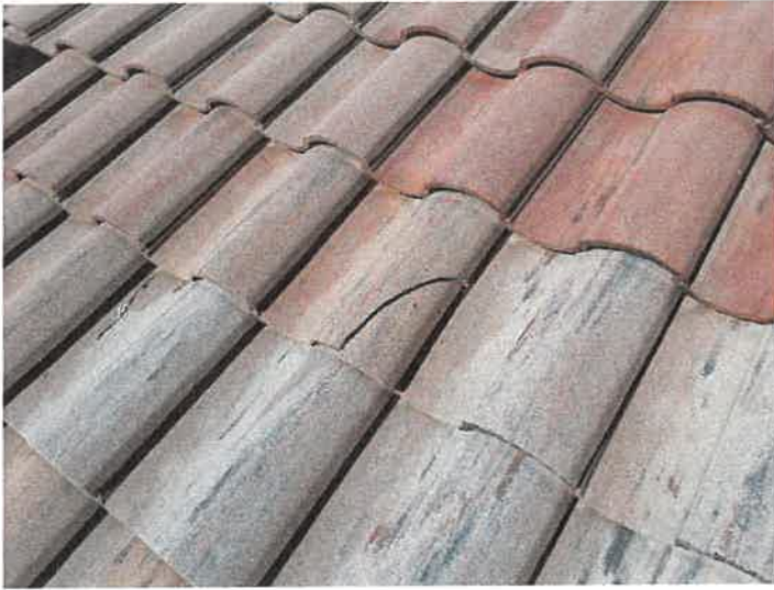
Building 15193: Identified Cracked Roof Tiles Cracked roof tiles can allow premature underlayment deterioration from excessive UV exposure.
