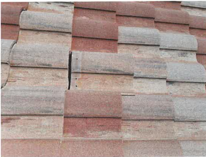
Building 15205: Displaced/Missing Roof Tile
