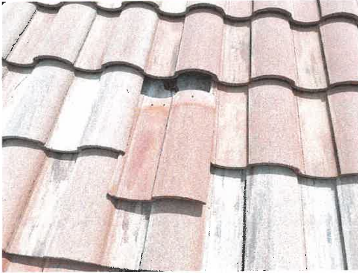
Building 15184: Displaced/Missing Roof Tile
