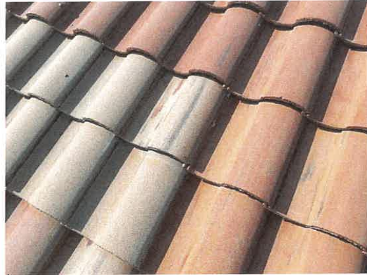
Building 15201: Repaired Displaced/Missing Roof Tile
