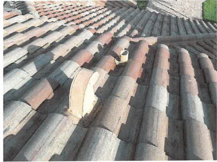
Building 15177: Lead Boots Lead boots appear to be in good condition.
