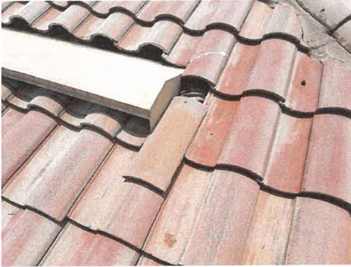
Building 15173: Displaced/Missing Roof Tile
