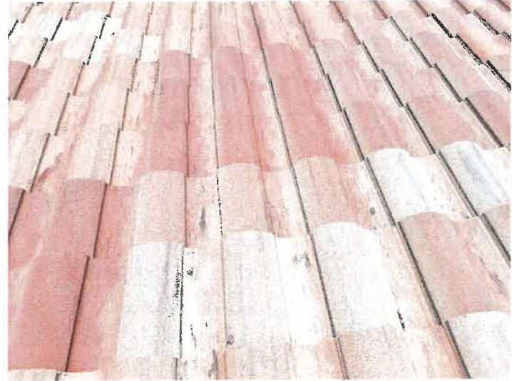
Building 15165: Repaired Cracked Roof Tiles
