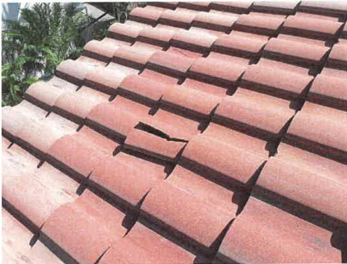
Building 15188: Identified Cracked Roof Tiles
