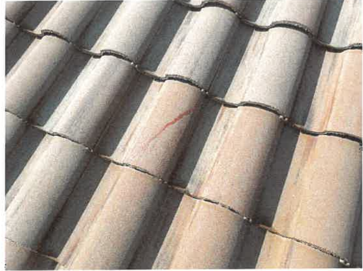
Building 15201: Repaired Cracked Roof Tiles
