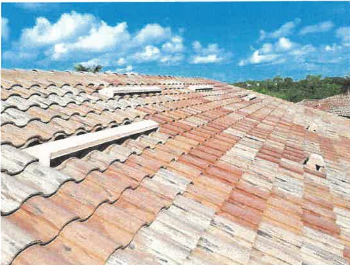
Building 15161: Roof Vents
