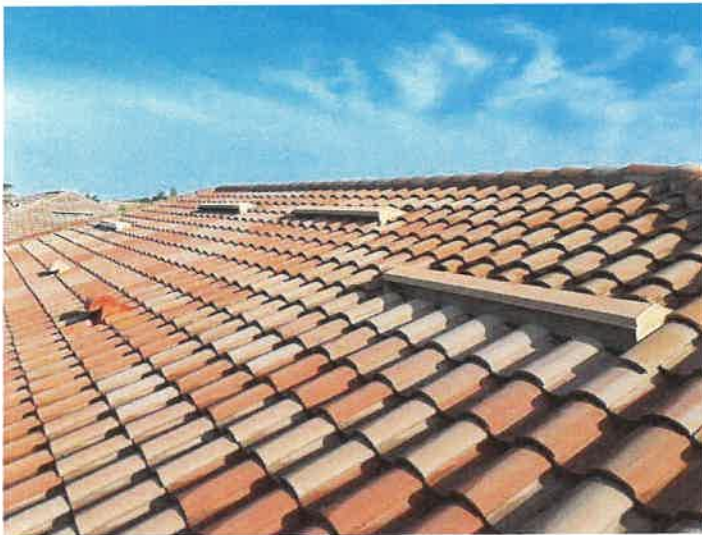
Building 15201: Roof Vents
