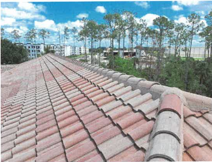
Building 15184: Ridge Tiles Ridge tiles appear to be in good condition.
