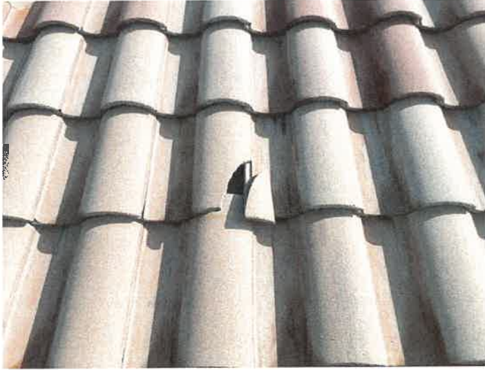
Building 15201: Identified Cracked Roof Tiles Cracked roof tiles can allow premature underlayment deterioration from excessive UV exposure.
