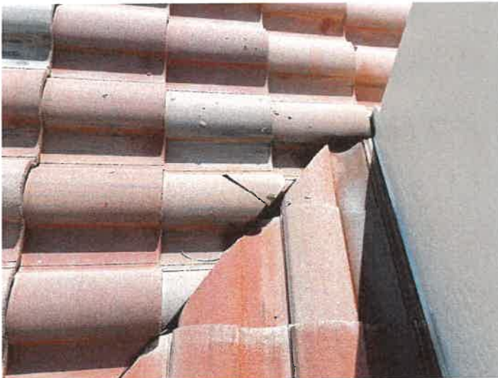
Building 15189: Identified Cracked Roof Tiles Cracked roof tiles can allow premature underlayment deterioration from excessive UV exposure.
