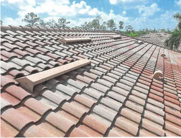
Building 15209: Roof Vents Roof vents appear to be in good condition.
