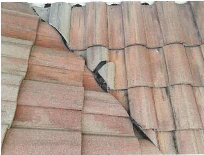
Building 15177: Identified Cracked Roof Tiles Cracked roof tiles can allow premature underlayment deterioration from excessive UV exposure.
