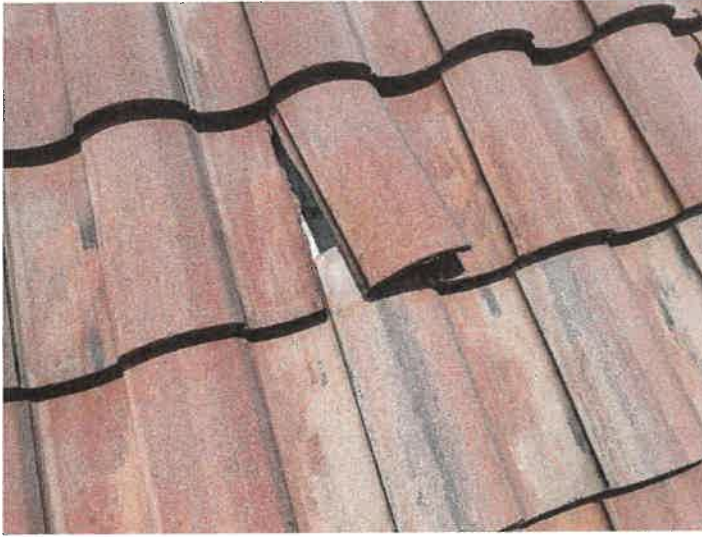
Building 15173: Identified Cracked Roof Tiles Cracked roof tiles can allow premature underlayment deterioration from excessive UV exposure.
