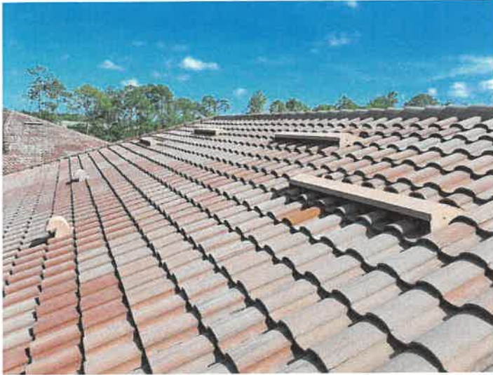
Building 15185: Roof Vents Roof vents appear to be in good condition.
