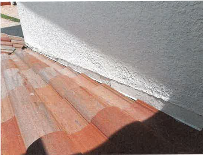
Building 15184: Counter Flashings
