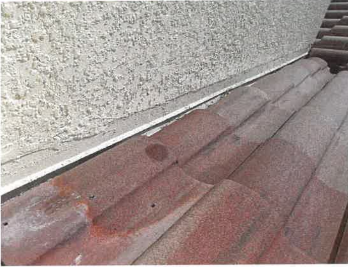
Building 15189: Counter Flashings
