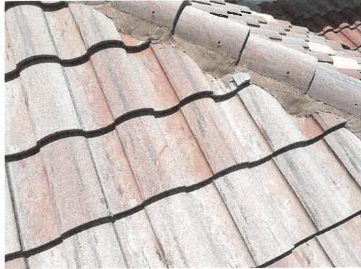
Building 15213: Repaired Cracked Roof Tiles
