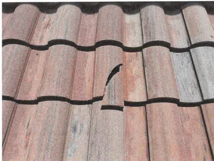
Building 15184: Identified Cracked Roof Tiles Cracked roof tiles can allow premature underlayment deterioration from excessive UV exposure.
