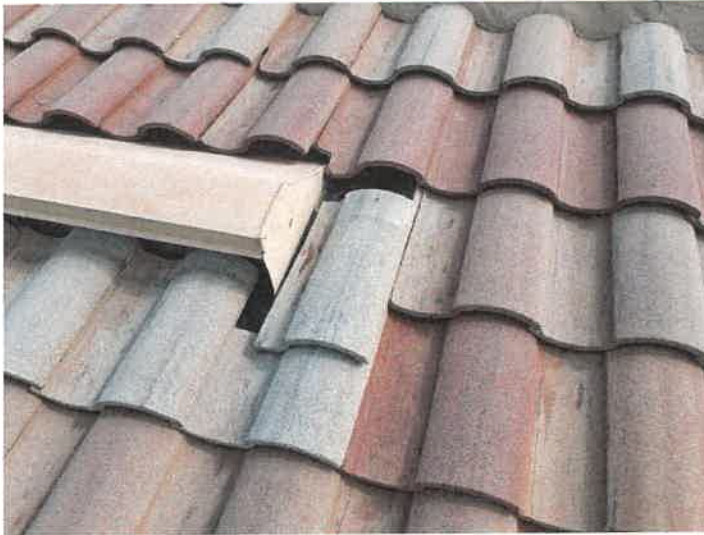
Building 15205: Displaced/Missing Roof Tile
