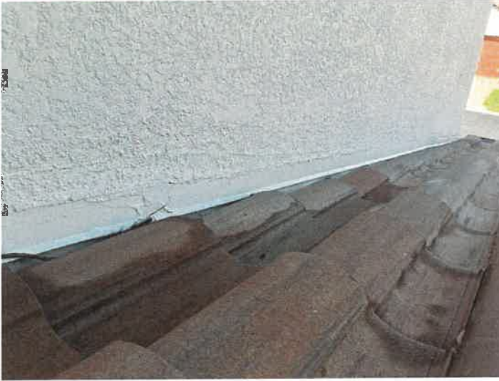
Building 15188: Counter Flashings
