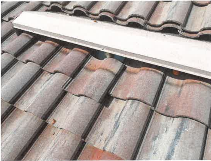
Building 15161: Displaced/Missing Roof Tile
