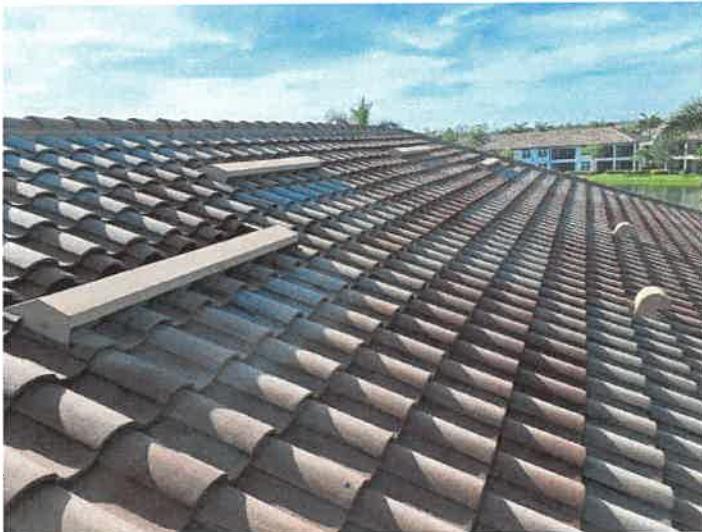
Building 15193: Roof Vents
