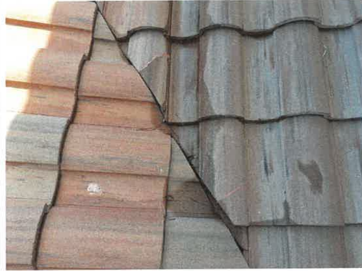
Building 15188: Repaired Cracked Roof Tiles The cracked roof tiles were repaired with Titebond sealant.
