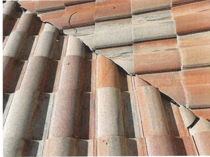
Building 15189: Repaired Cracked Roof Tiles
