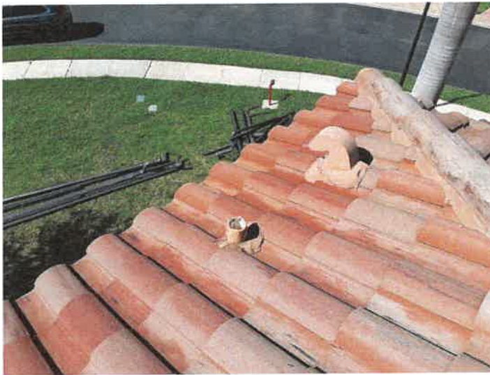
Building 15188: Lead Boots Lead boots appear to be in good condition.
