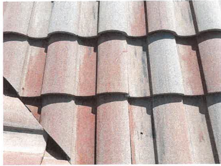
Building 15188: Repaired Cracked Roof Tiles
