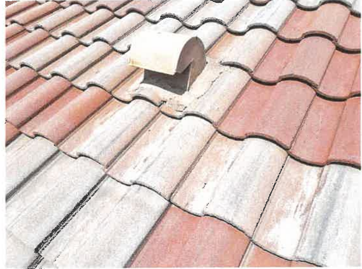
Building 15165: Repaired Displaced/Missing Roof Tile
