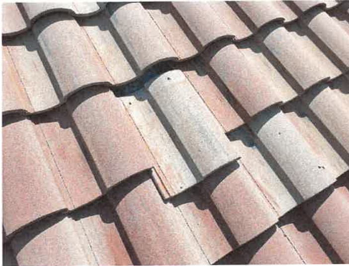
Building 15185: Displaced/Missing Roof Tile
