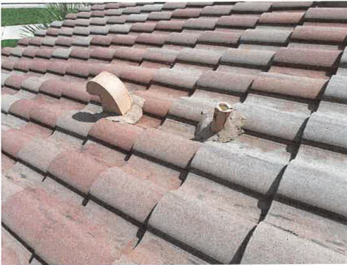
Building 15209: Lead Boots Lead boots appear to be in good condition.
