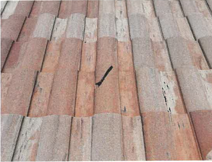
Building 15205: Identified Cracked Roof Tiles
