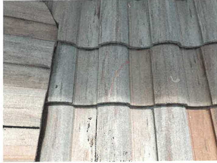
Building 15184: Repaired Cracked Roof Tiles The cracked roof tiles were repaired with Titebond sealant.
