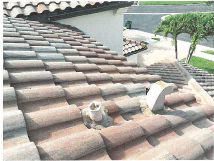
Building 15161: Lead Boots Lead boots appear to be in good condition.
