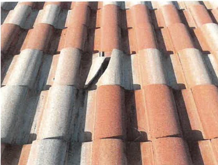
Building 15201: Identified Cracked Roof Tiles
