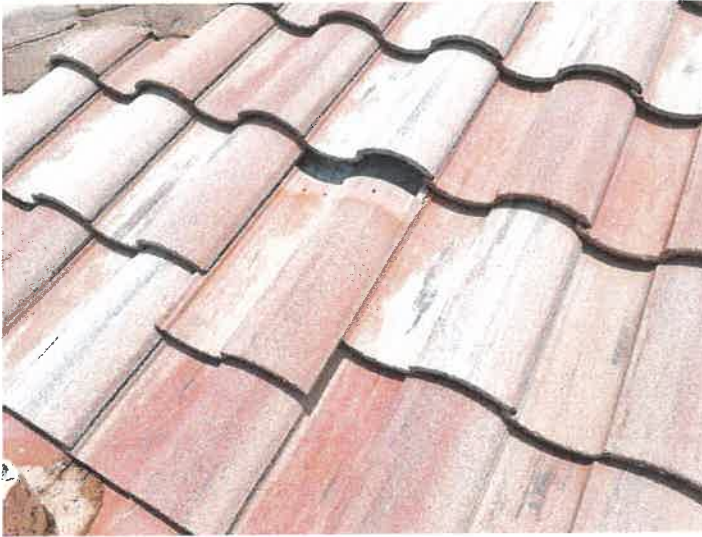
Building 15173: Displaced/Missing Roof Tile
