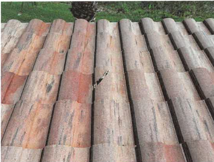
Building 15161: Identified Cracked Roof Tiles Cracked roof tiles can allow premature underlayment deterioration from excessive UV exposure.
