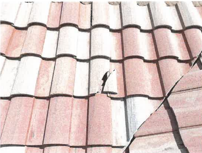
Building 15165: Identified Cracked Roof Tiles
