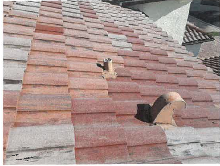
Building 15193: Lead Boots Lead boots appear to be in good condition.
