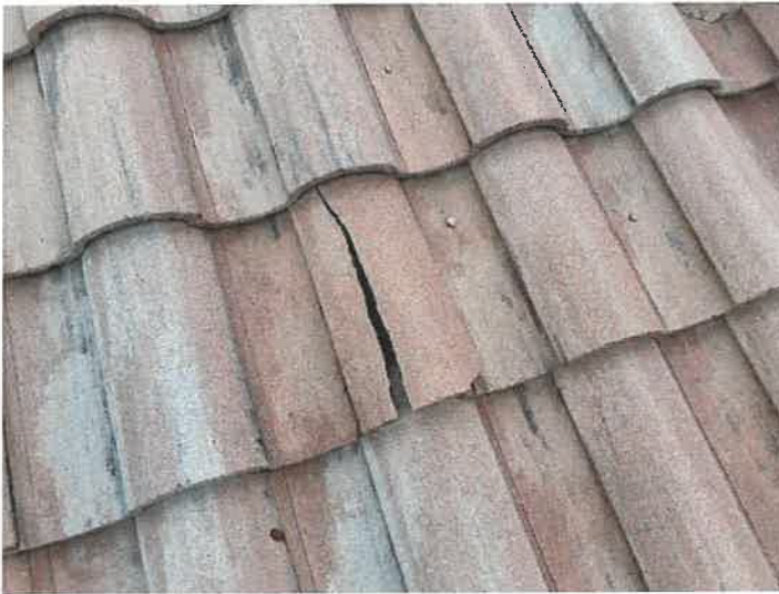
Building 15152: Identified Cracked Roof Tiles Cracked roof tiles can allow premature underlayment deterioration from excessive UV exposure.
