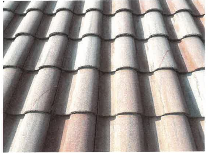
Building 15145: Repaired Cracked Roof Tiles
