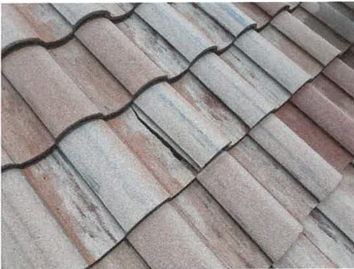
Building 15153: Identified Cracked Roof Tiles Cracked roof tiles can allow premature underlayment deterioration from excessive UV exposure.
