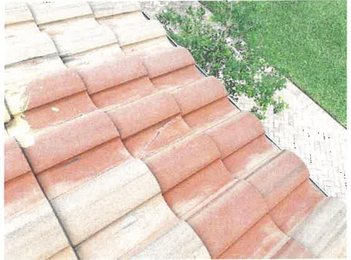
Building 15156: Repaired Cracked Roof Tiles
