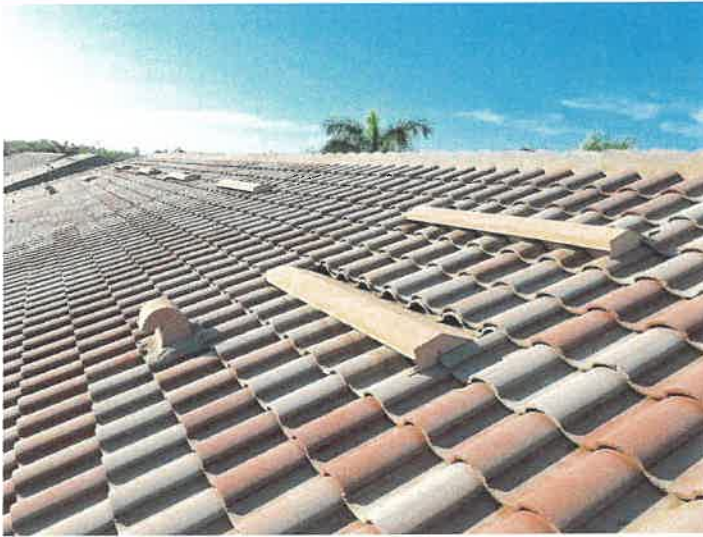
Building 15157: Roof Vents Roof vents appear to be in good condition.
