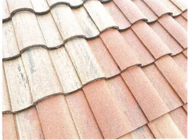
Building 15136: Repaired Cracked Roof Tiles
