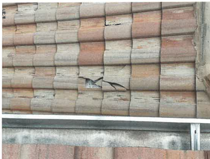
Building 15153: Broken Roof Tiles Crowther Roofing suggests replacing two (2) broken roof tiles.
