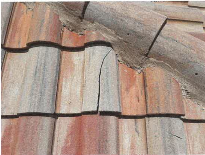
Building 15156: Identified Cracked Roof Tiles
