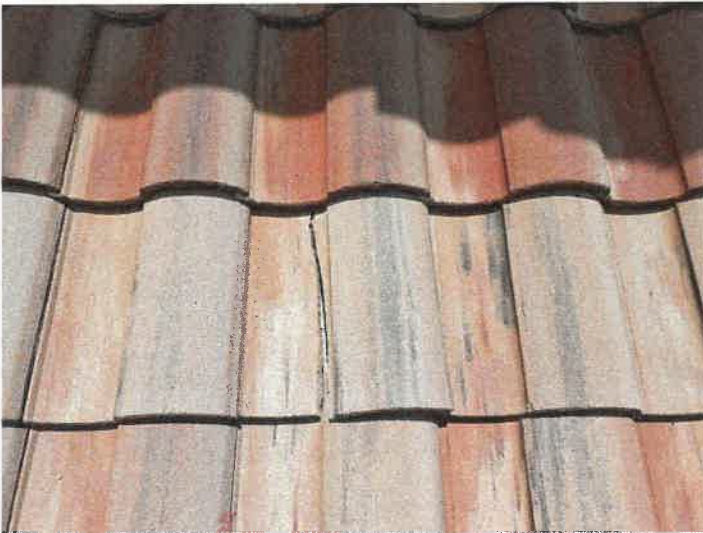
Building 15156: Identified Cracked Roof Tiles
