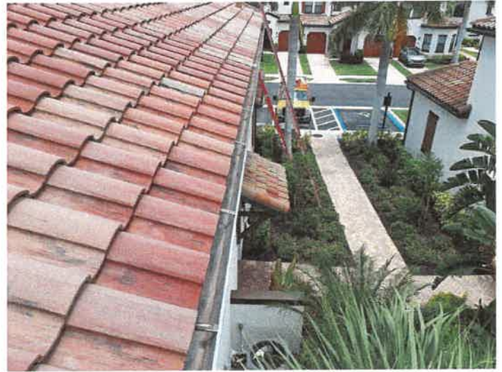
Building 15156: Gutters The gutters appear to be in good condition.
