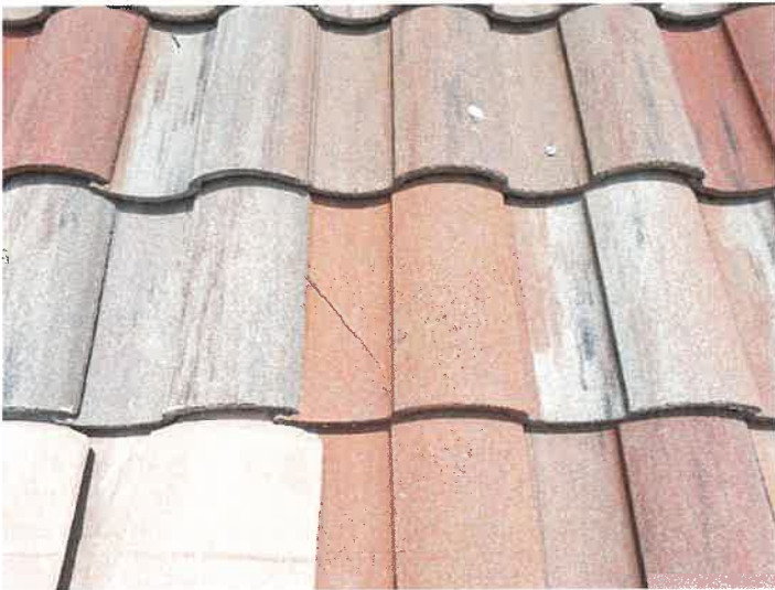
Building 15144: Identified Cracked Roof Tiles
