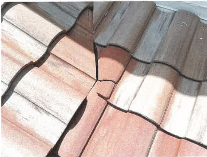
Building 15148: Identified Cracked Roof Tiles
