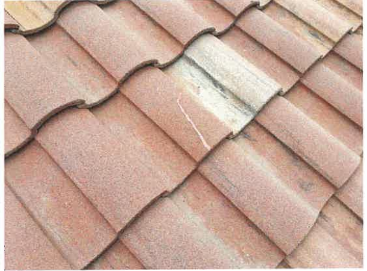
Building 15137: Repaired Cracked Roof Tiles
