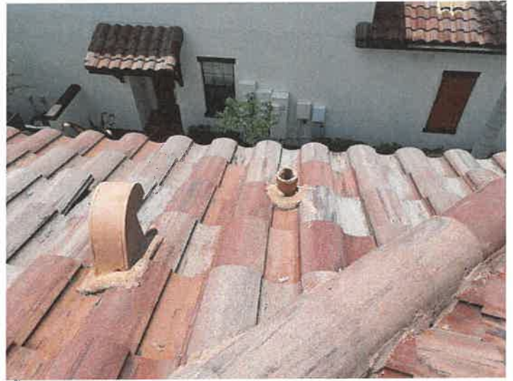
Building 15152: Lead Boots Lead boots appear to be in good condition.
