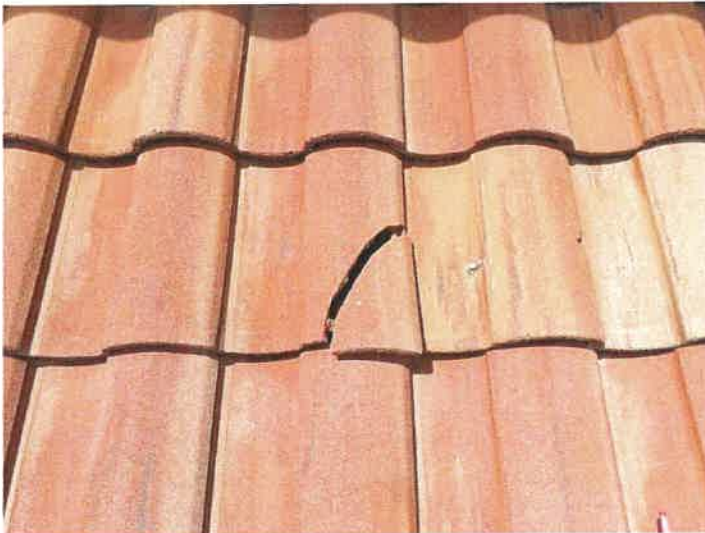
Building 15148: Identified Cracked Roof Tiles
