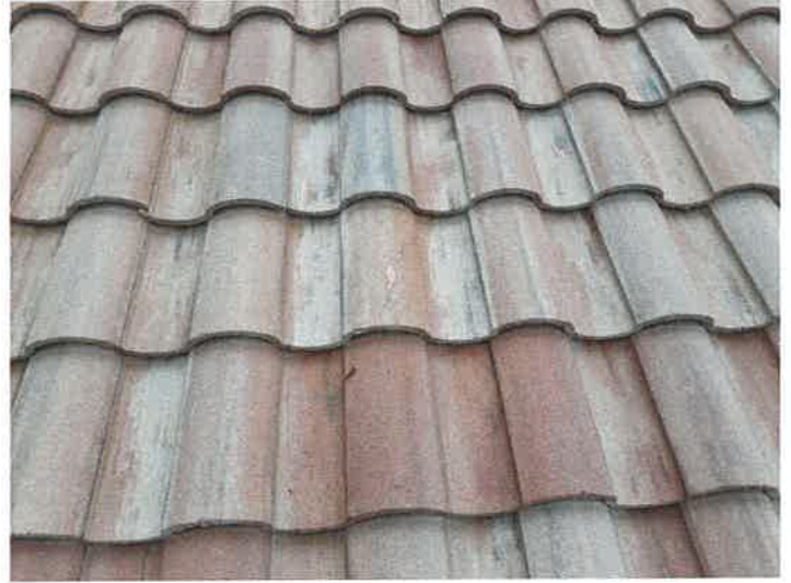
Building 15153: Repaired Cracked Roof Tiles
