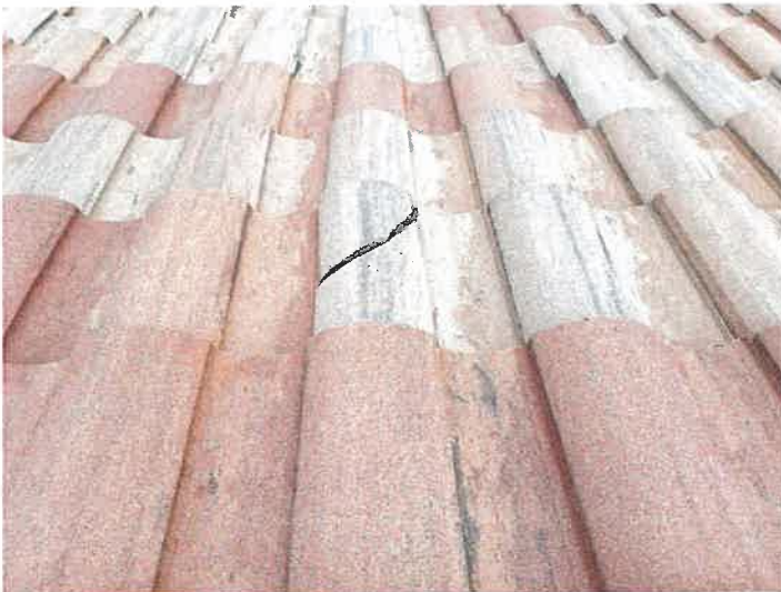
Building 15140: Identified Cracked Roof Tiles
