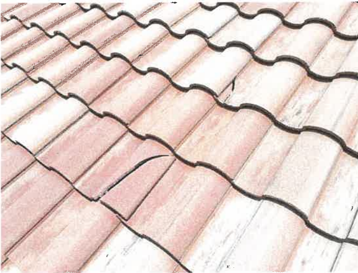
Building 15153: Identified Cracked Roof Tiles
