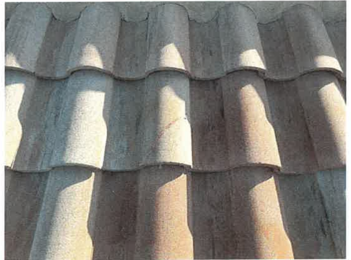
Building 15157: Repaired Cracked Roof Tiles
