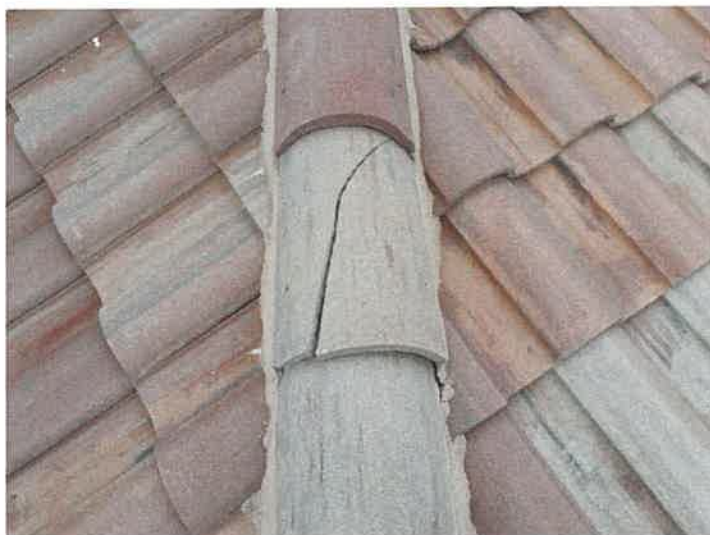
Building 15153: Identified Cracked Roof Tiles
