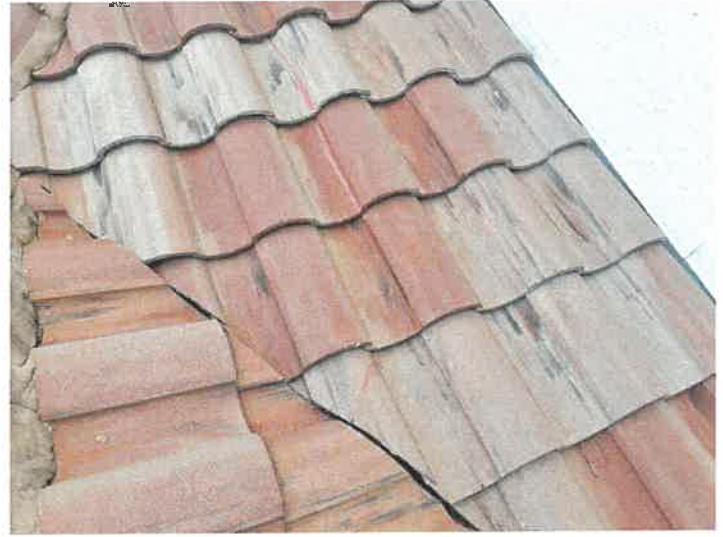
Building 15149: Repaired Cracked Roof Tiles
