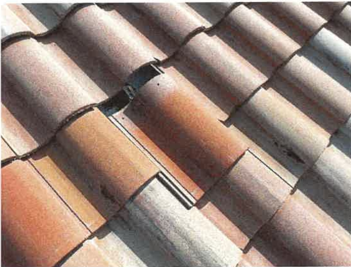
Building 15145: Displaced/Missing Roof Tile
