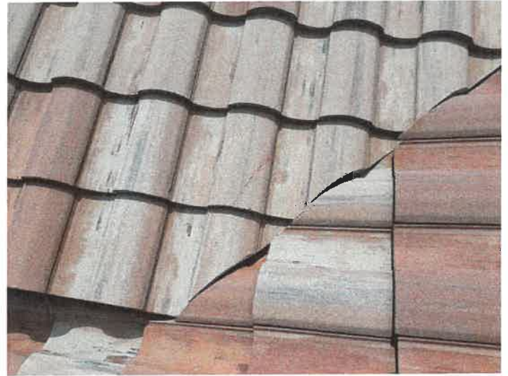
Building 15153: Repaired Cracked Roof Tiles
