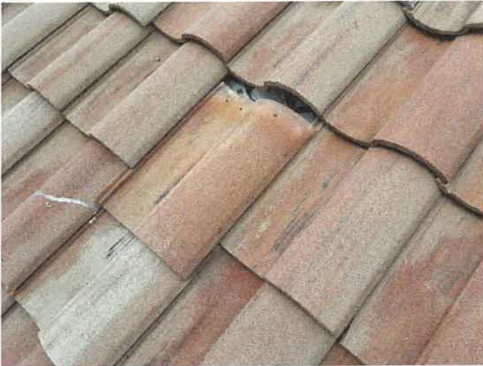
Building 15152: Displaced/Missing Roof Tile
