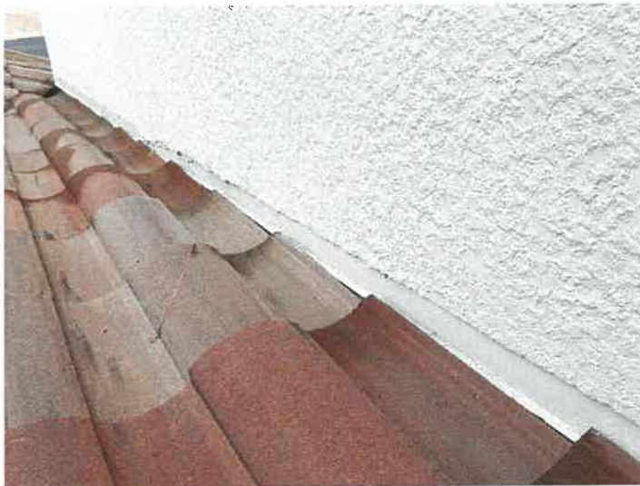
Building 15136: Counter Flashings
