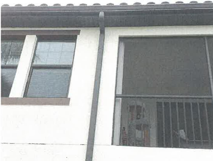
Building 15137: Gutter- Interior gutter issue (Location) Interior gutter has issues that will/have lead to water penetration. Remove and replace waterproofing material immediately.
