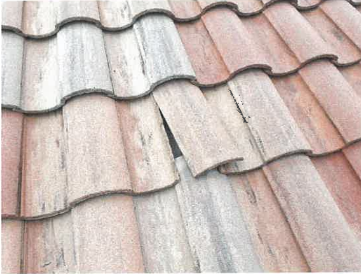
Building 15140: Identified Cracked Roof Tiles
