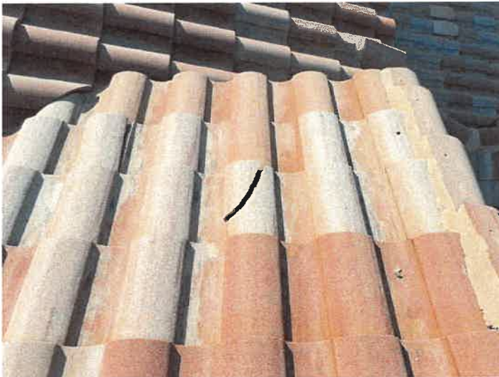
Building 15157: Identified Cracked Roof Tiles
