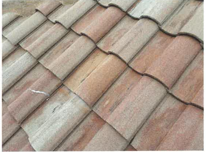
Building 15152: Repaired Displaced/Missing Roof Tile
