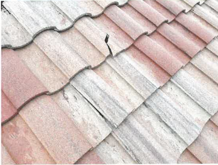
Building 15140: Identified Cracked Roof Tiles
