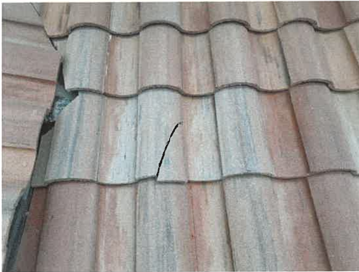
Building 15153: Identified Cracked Roof Tiles
