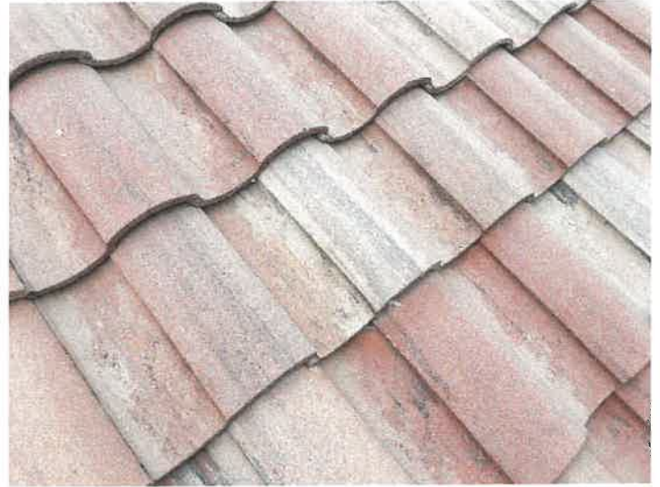
Building 15140: Repaired Displaced/Missing Roof Tile
