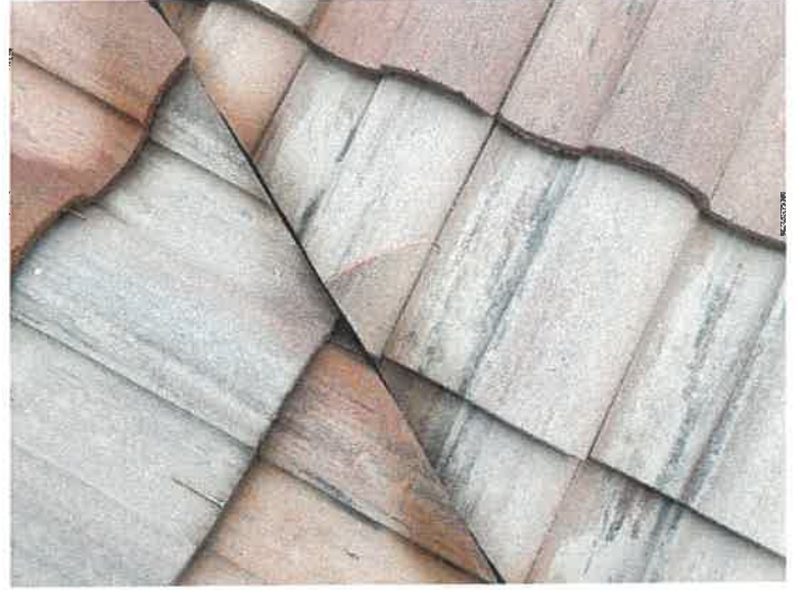
Building 15136: Repaired Cracked Roof Tiles
