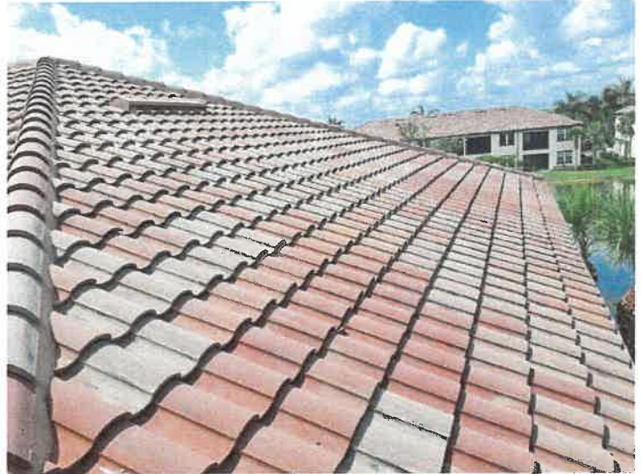
Building 15148: Surface Overview The roof surface appears to be in good, maintainable condition at this time.
