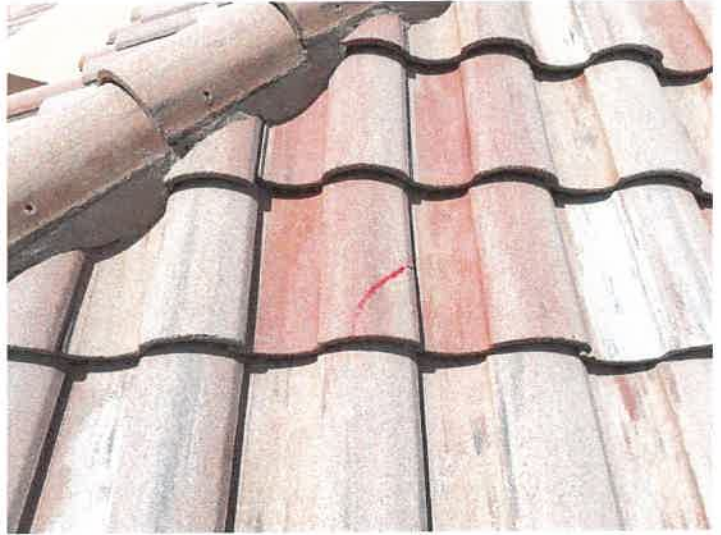
Building 15148: Repaired Cracked Roof Tiles The cracked roof tiles were repaired with Titebond sealant.
