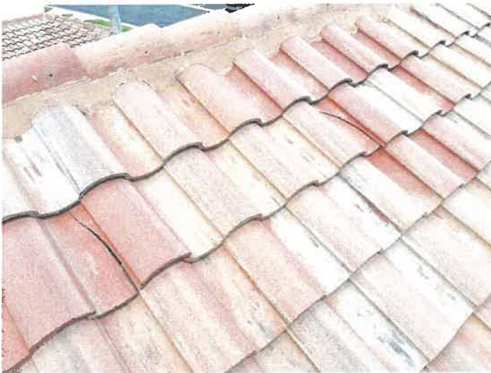
Building 15153: Identified Cracked Roof Tiles
