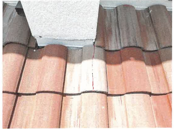
Building 15148: Repaired Cracked Roof Tiles
