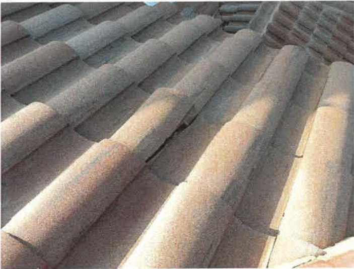
Building 15145: Identified Cracked Roof Tiles Cracked roof tiles can allow premature underlayment deterioration from excessive UV exposure.
