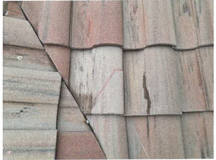
Building 15137: Repaired Cracked Roof Tiles
