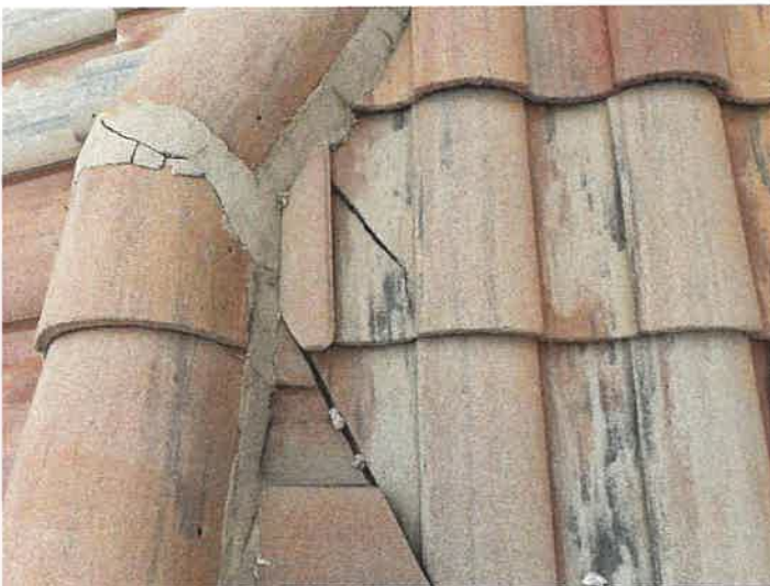
Building 15141: Identified Cracked Roof Tiles Cracked roof tiles can allow premature underlayment deterioration from excessive UV exposure.
