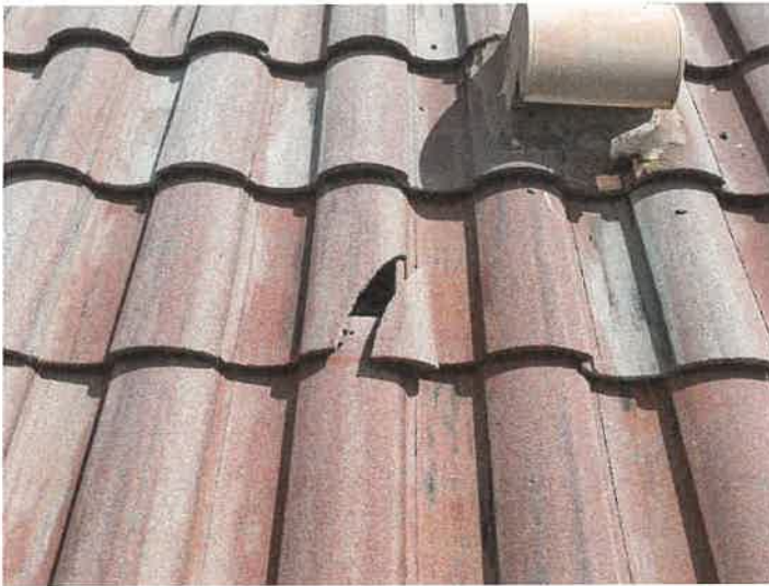
Building 15152: Identified Cracked Roof Tiles
