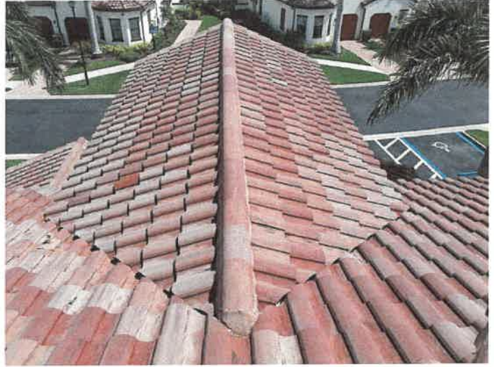
Building 15148: Valley The valley tiles appear to be in good condition.
