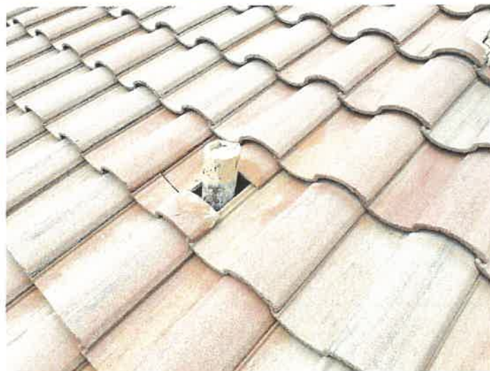
Building 15153: Missing Mortar
