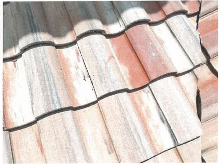
Building 15156: Repaired Cracked Roof Tiles
