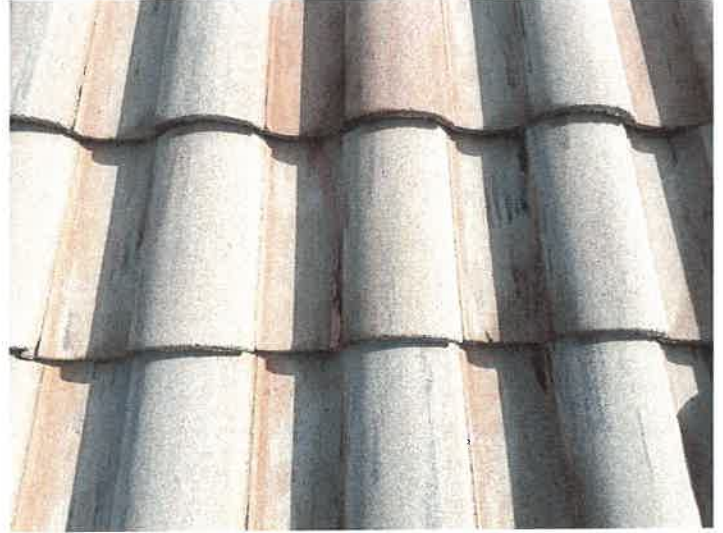
Building 15145: Repaired Cracked Roof Tiles
