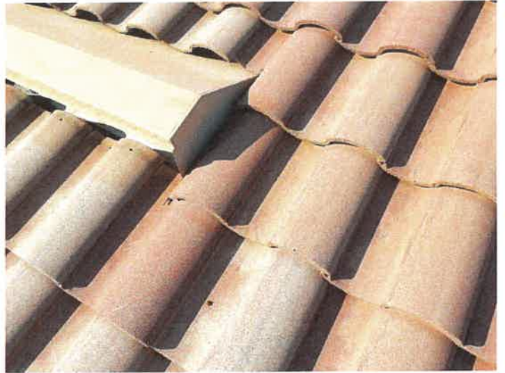
Repaired Displaced/Missing Roof Tile
