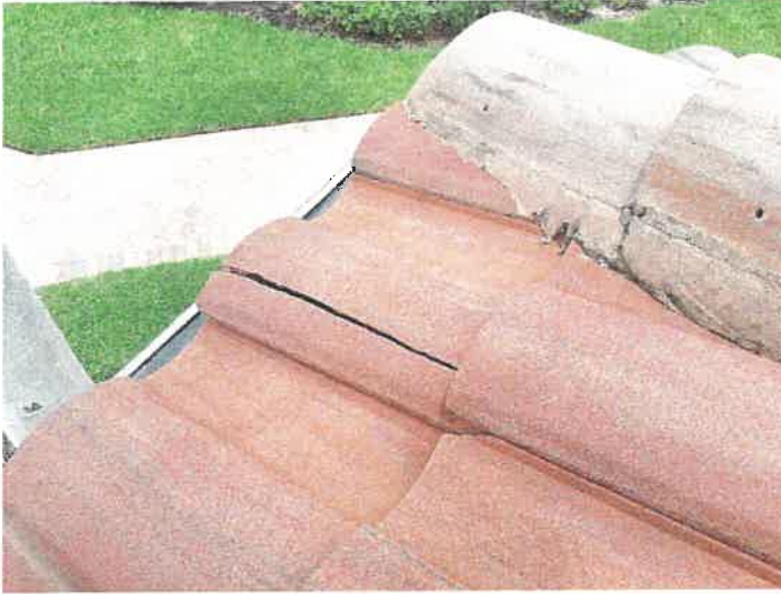
Building 15144: Identified Cracked Roof Tiles
