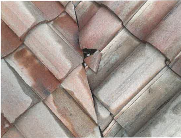
Building 15152: Identified Cracked Roof Tiles
