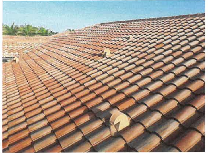
Building 15145: Roof Vents Roof vents appear to be in good condition.
