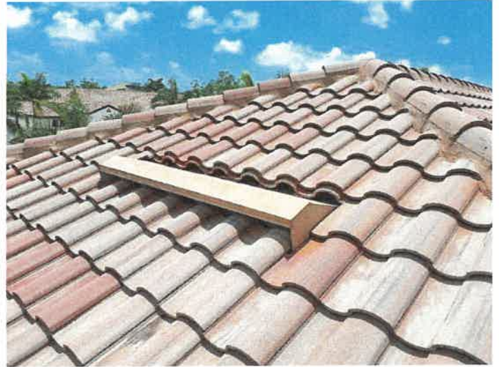
Building 15153: Roof Vents
