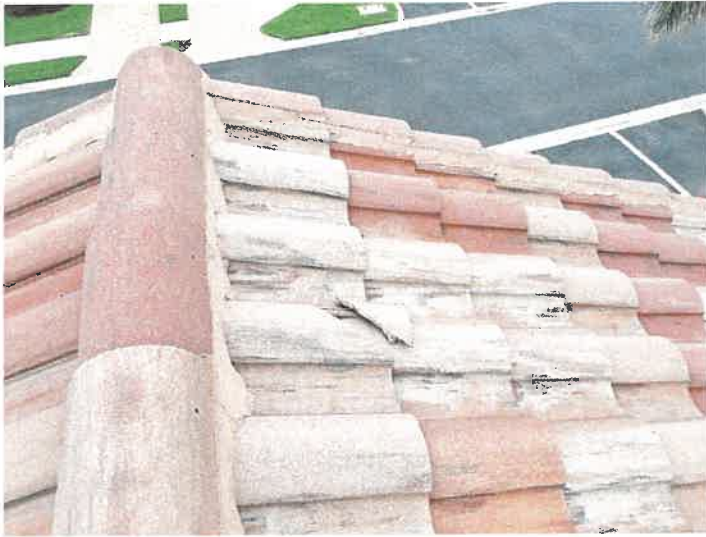
Building 15144: Identified Cracked Roof Tiles
