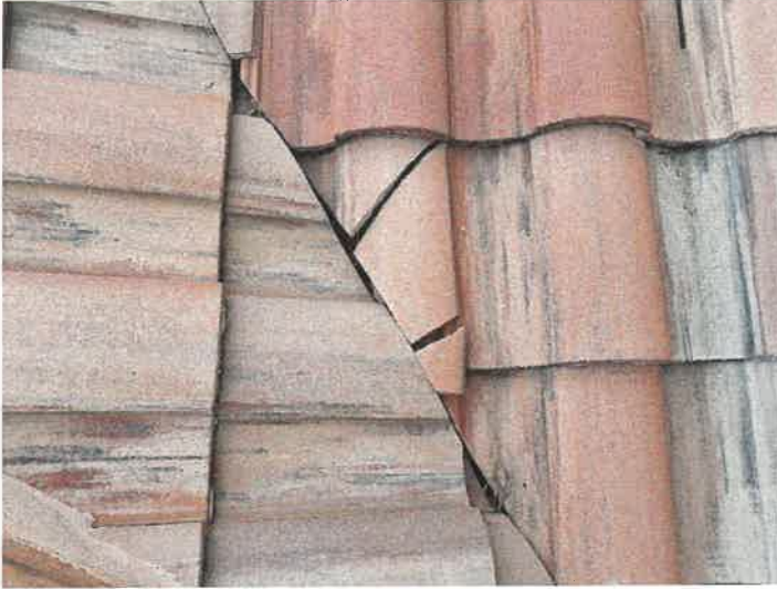
Building 15140: Identified Cracked Roof Tiles
