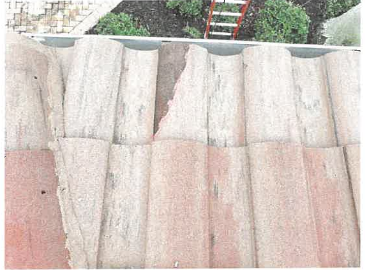
Building 15137: Repaired Cracked Roof Tiles
