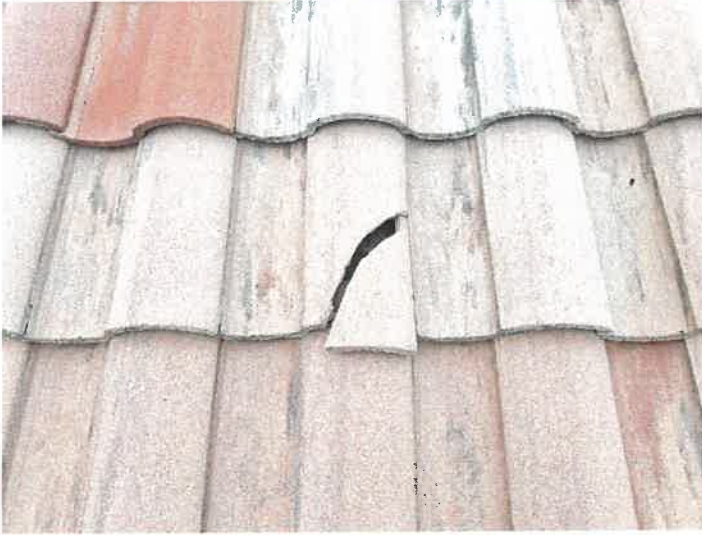
Building 15140: Identified Cracked Roof Tiles
