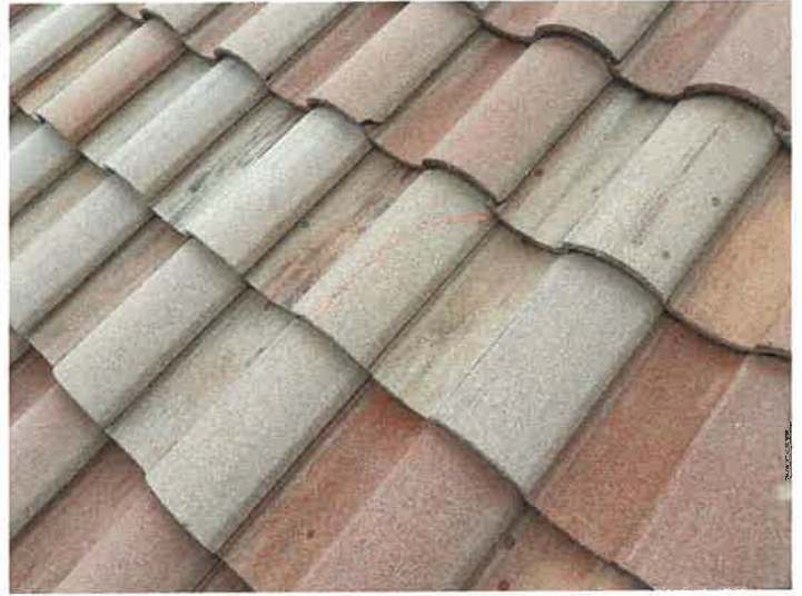
Building 15152: Repaired Cracked Roof Tiles
