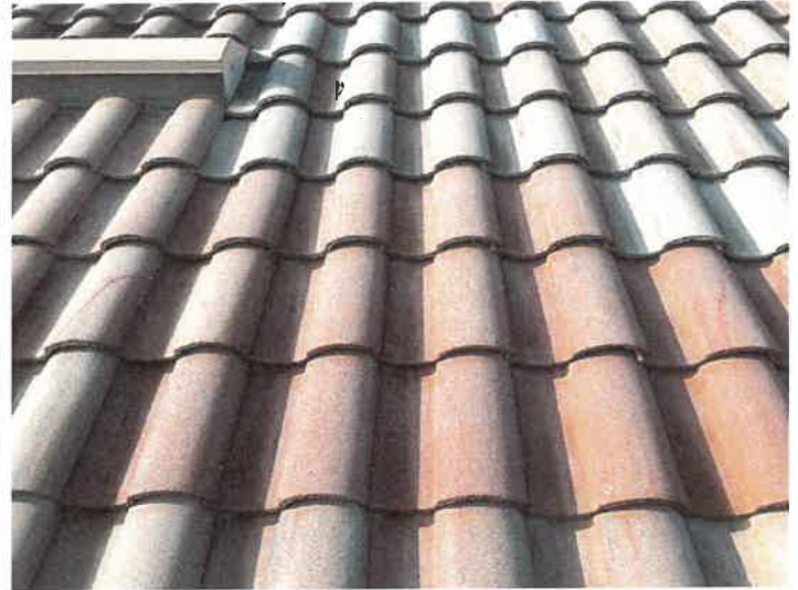
Building 15145: Repaired Cracked Roof Tiles
