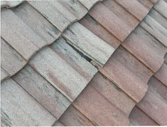
Building 15145: Identified Cracked Roof Tiles Cracked roof tiles can allow premature underlayment deterioration from excessive UV exposure.
