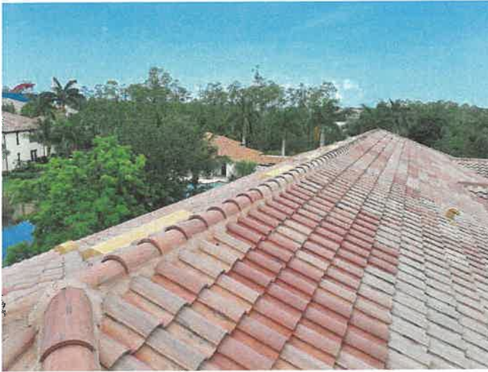
Building 15156: Ridge Tiles Ridge tiles appear to be in good condition.
