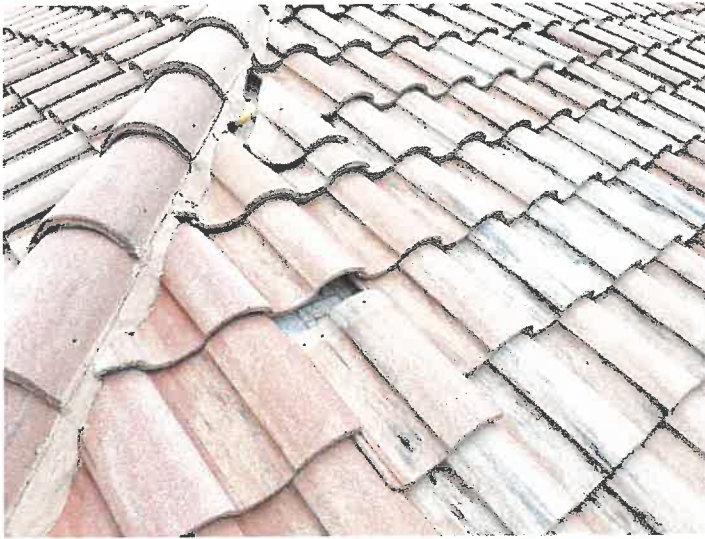
Building 15144: Displaced/Missing Roof Tile
