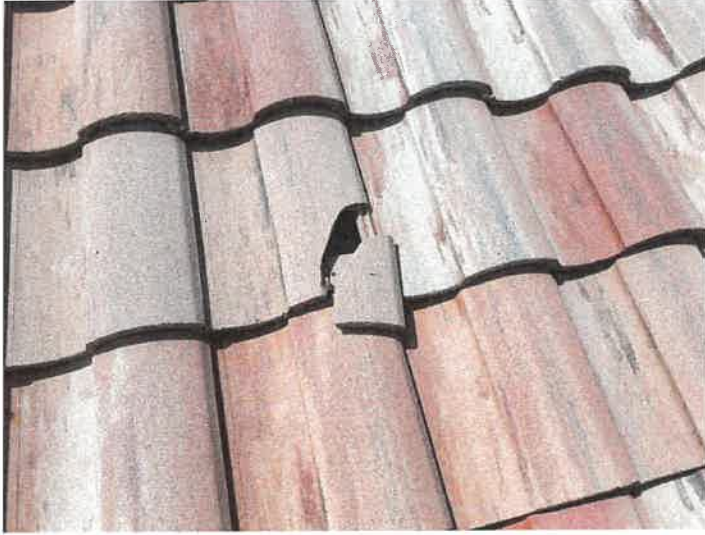
Building 15148: Identified Cracked Roof Tiles
