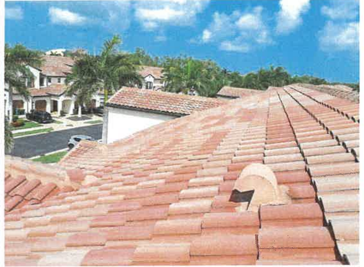
Building 15149: Roof Vents
