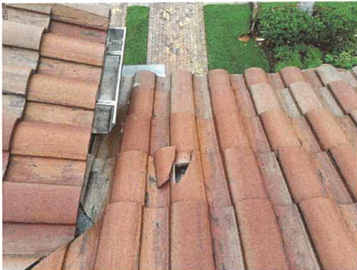
Building 15136: Identified Cracked Roof Tiles
