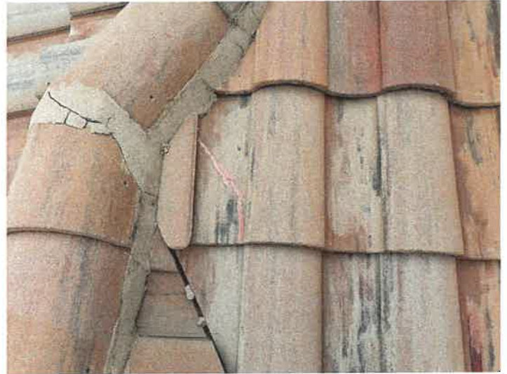
Building 15141: Repaired Cracked Roof Tiles The cracked roof tiles were repaired with Titebond sealant.
