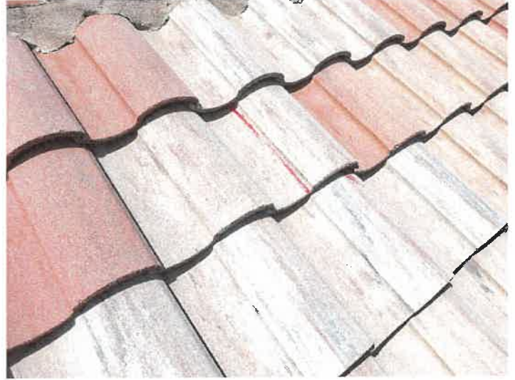
Building 15148: Repaired Cracked Roof Tiles
