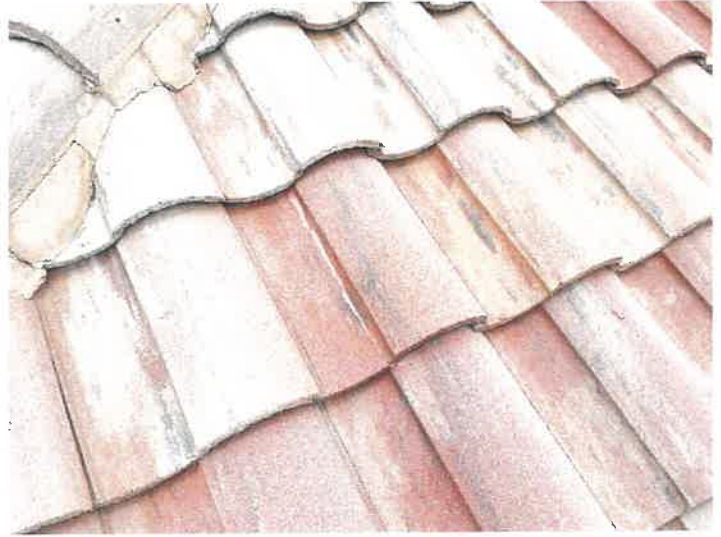
Building 15144: Repaired Cracked Roof Tiles
