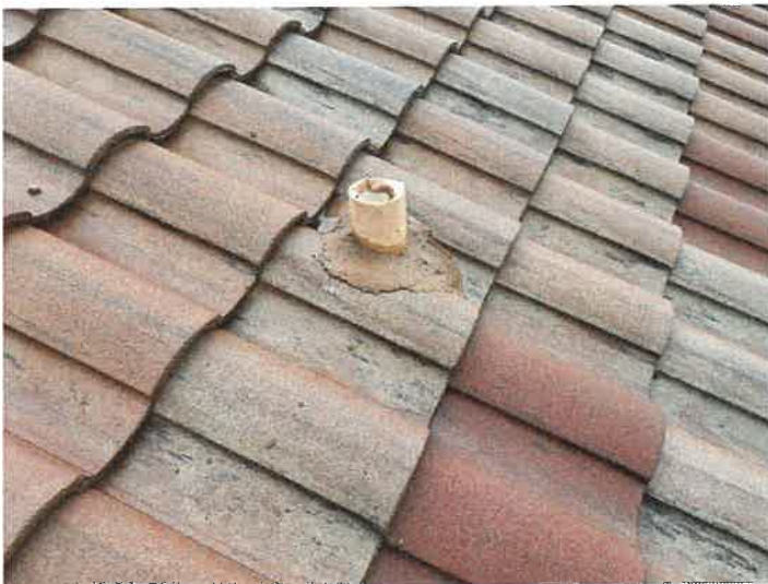
Building 15136: Lead Boots Lead boots appear to be in good condition.
