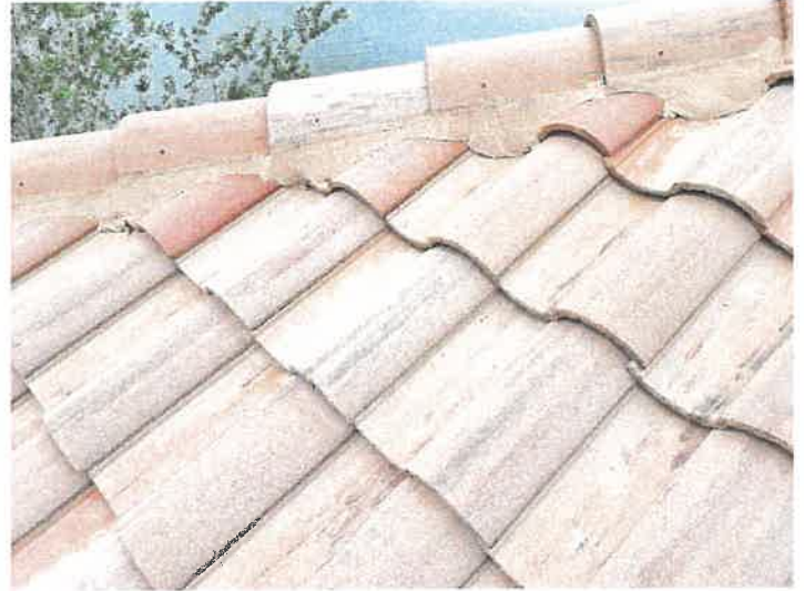
Building 15140: Repaired Displaced/Missing Roof Tile
