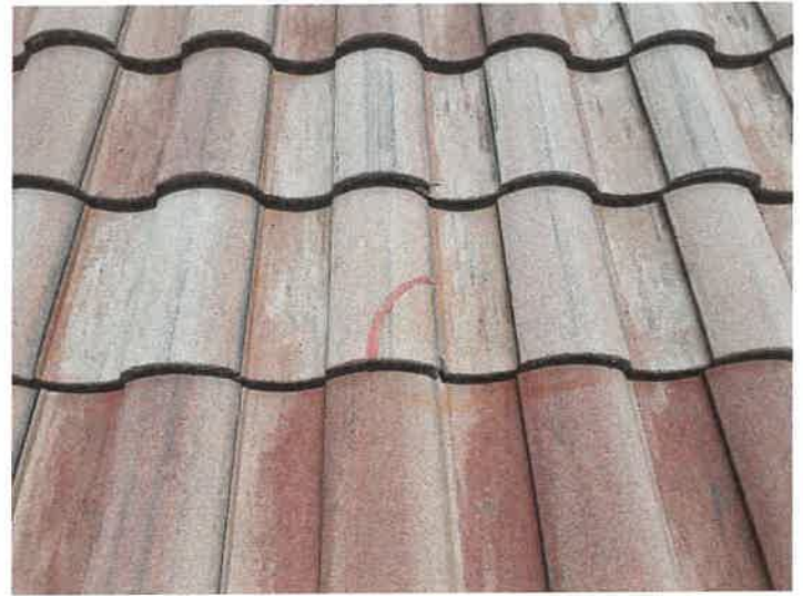
Building 15153: Repaired Cracked Roof Tiles
