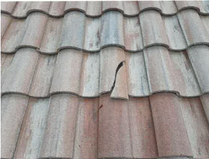
Building 15153: Identified Cracked Roof Tiles
