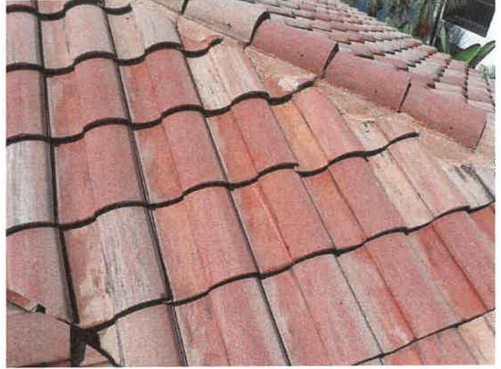
Building 15152: Repaired Cracked Roof Tiles
