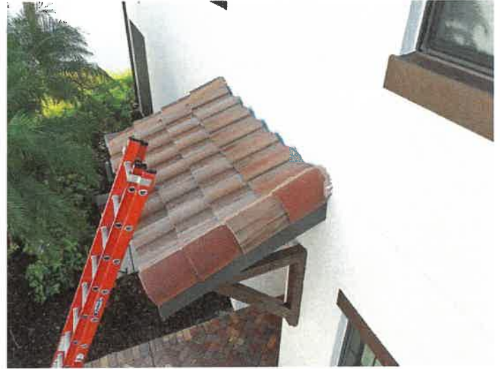
Building 15157: Repaired Displaced/Missing Roof Tile
