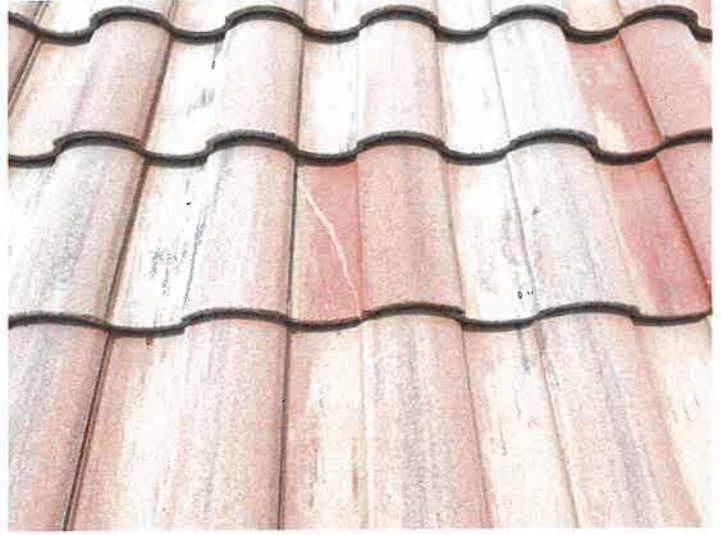
Building 15153: Repaired Cracked Roof Tiles
