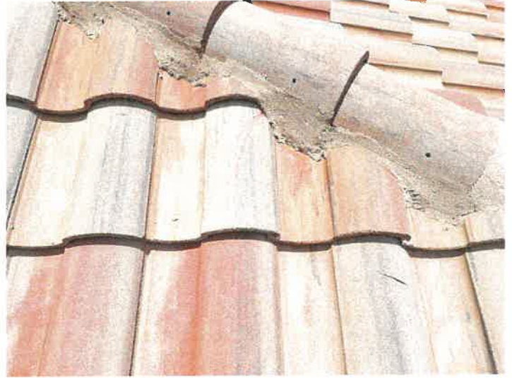
Building 15156: Repaired Cracked Roof Tiles
