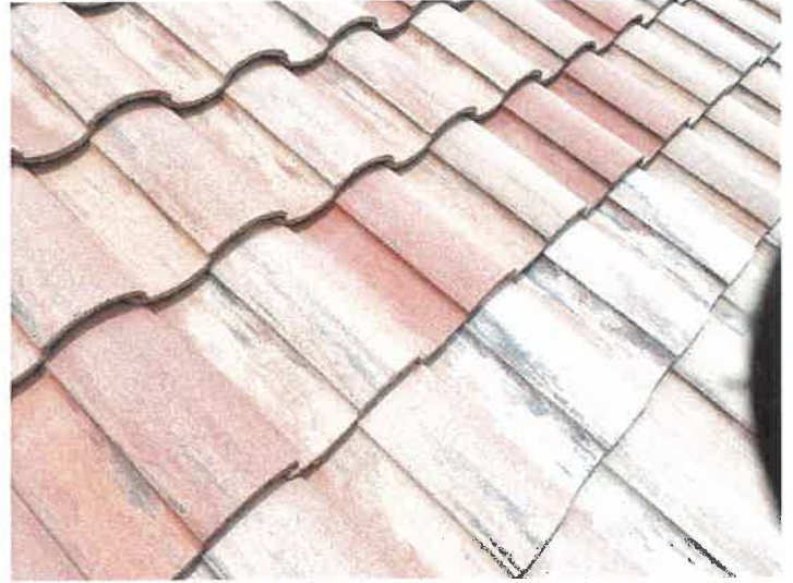
Building 15144: Repaired Displaced/Missing Roof Tile
