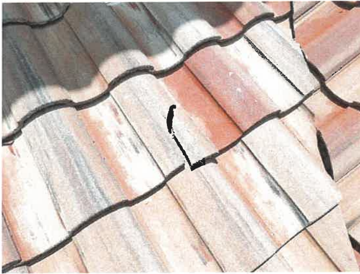
Building 15156: Identified Cracked Roof Tiles
