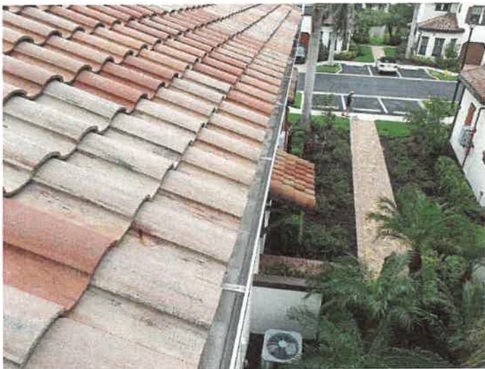
Building 15141: Gutters The gutters appear to be in good condition.
