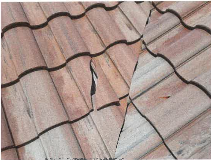
Building 15153: Identified Cracked Roof Tiles
