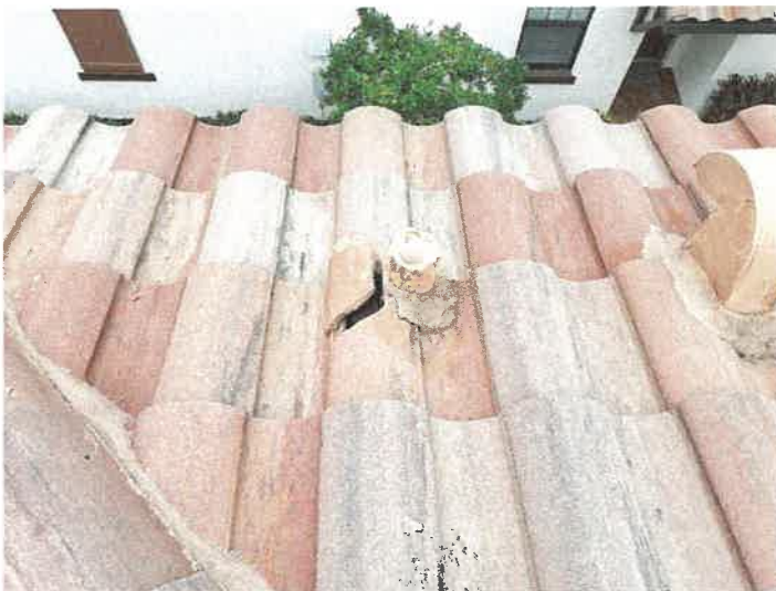
Building 15137: Identified Cracked Roof Tiles
