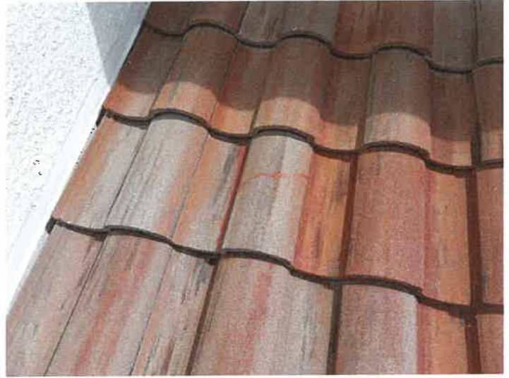
Building 15149: Repaired Cracked Roof Tiles
