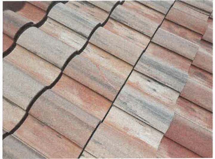
Building 15156: Repaired Cracked Roof Tiles
