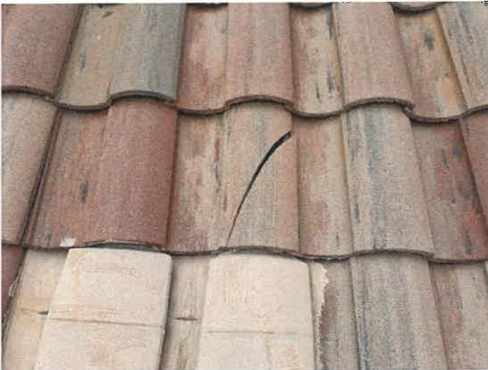
Building 15137: Identified Cracked Roof Tiles
