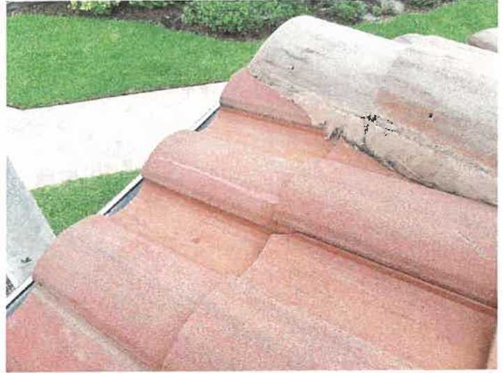
Building 15144: Repaired Cracked Roof Tiles
