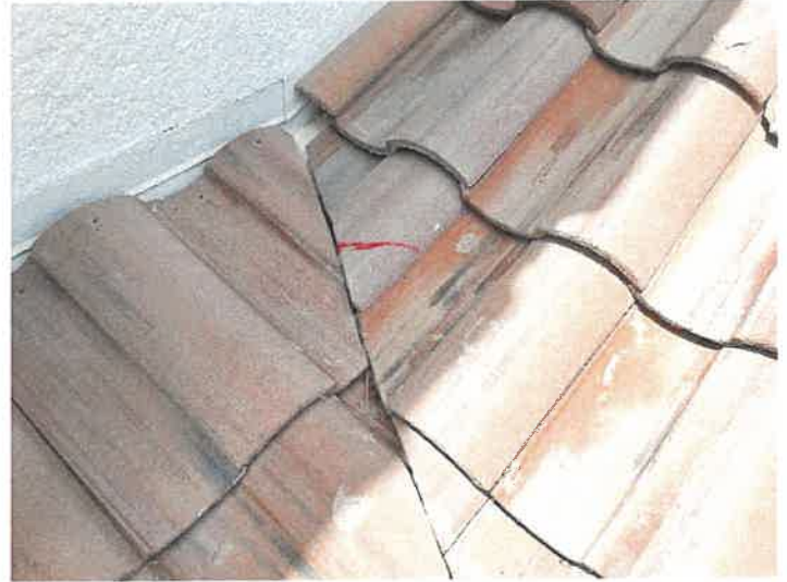
Building 15148: Repaired Cracked Roof Tiles
