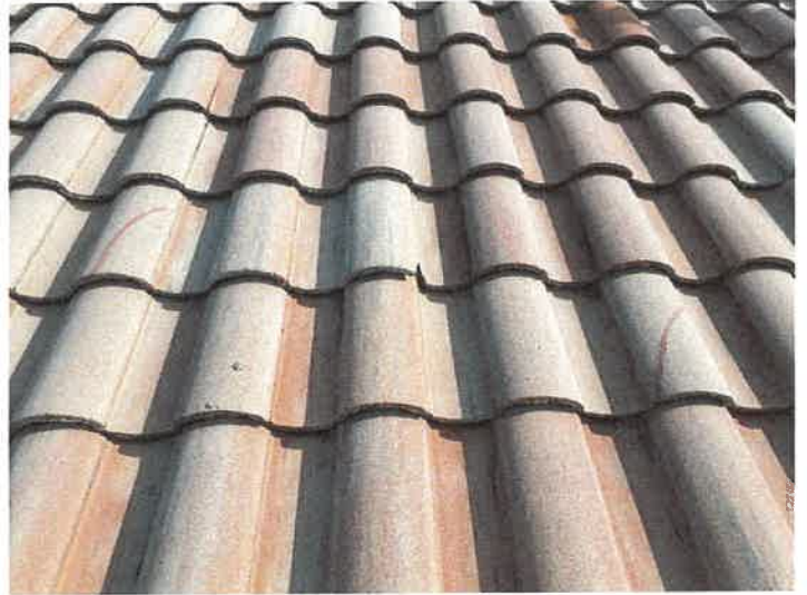
Building 15145: Repaired Cracked Roof Tiles
