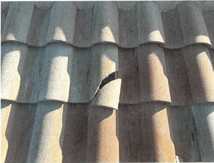
Building 15157: Identified Cracked Roof Tiles
