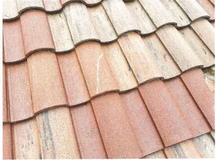
Building 15136: Repaired Cracked Roof Tiles The cracked roof tiles were repaired with Titebond sealant.
