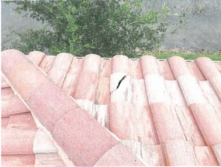
Building 15144: Identified Cracked Roof Tiles
