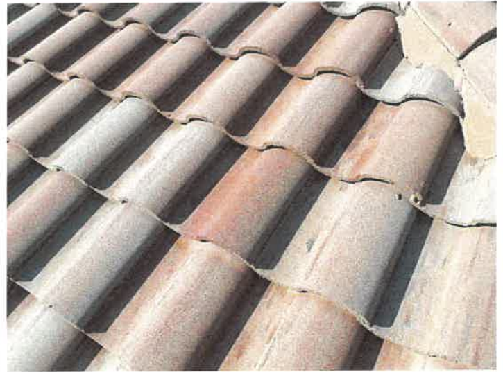
Building 15157: Repaired Displaced/Missing Roof Tile
