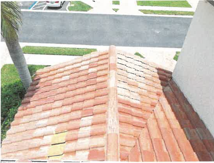
Building 15156: Appearance Overview - Lower Roof The roof appearance is in good, maintainable condition.
