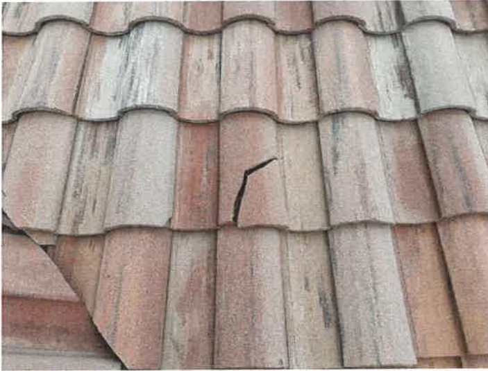
Building 15152: Identified Cracked Roof Tiles
