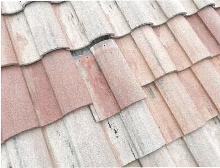
Displaced/Missing Roof Tile
