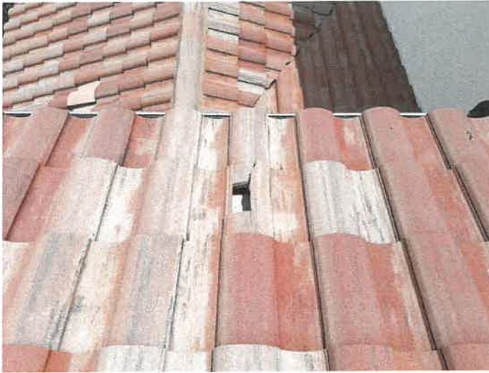
Building 15153: Broken Roof Tiles
