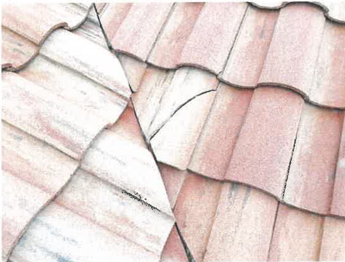
Building 15144: Identified Cracked Roof Tiles
