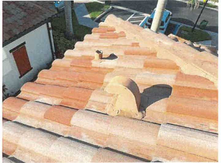
Building 15157: Lead Boots Lead boots appear to be in good condition.
