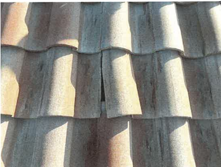
Building 15157: Identified Cracked Roof Tiles
