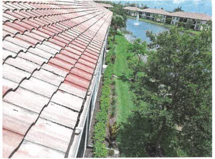
Building 15152: Gutters The gutters appear to be in good condition.
