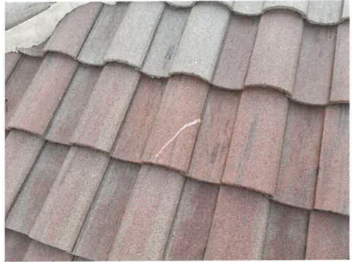
Building 15145: Repaired Cracked Roof Tiles
