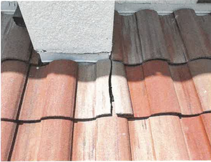
Building 15148: Identified Cracked Roof Tiles
