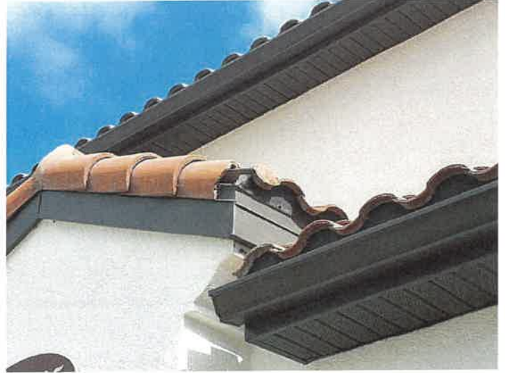
Building 15145: Broken Ridge Tile
