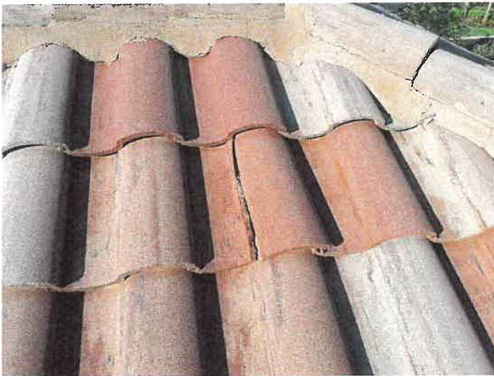
Building 15157: Identified Cracked Roof Tiles
