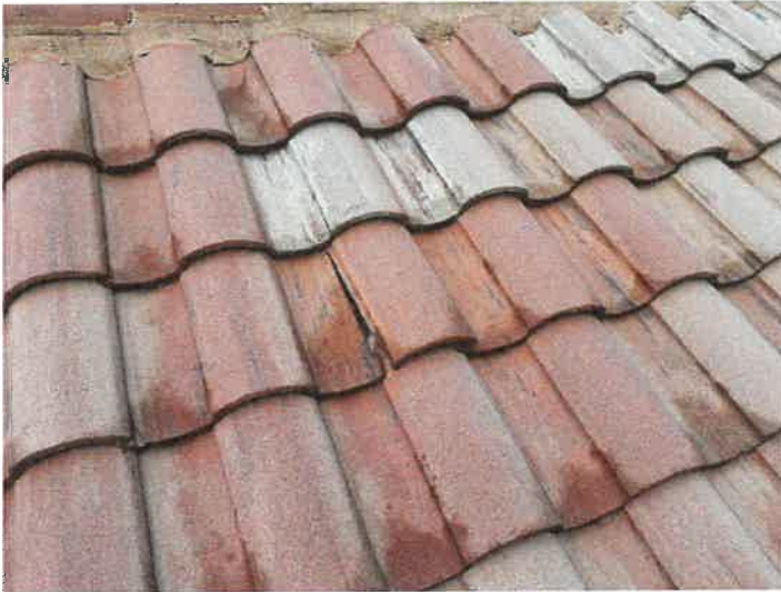
Building 15152: Identified Cracked Roof Tiles
