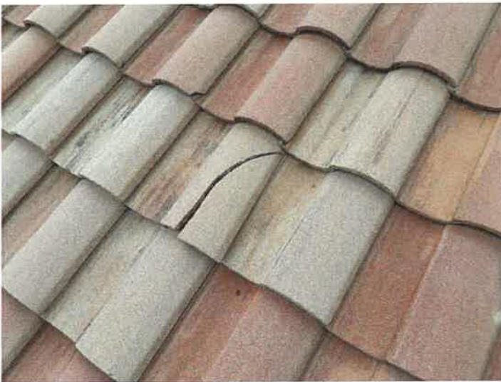
Building 15152: Identified Cracked Roof Tiles
