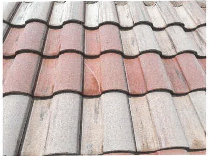
Building 15152: Repaired Cracked Roof Tiles
