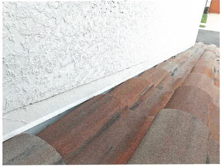
Building 15149: Counter Flashings
