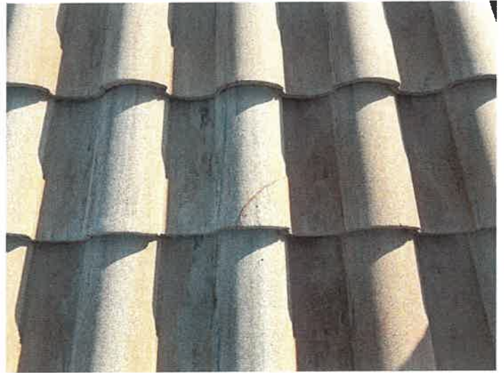
Building 15157: Repaired Cracked Roof Tiles
