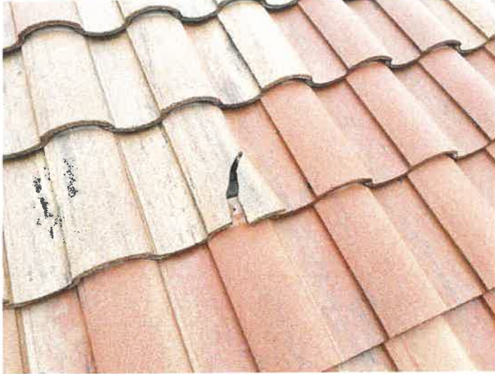
Building 15136: Identified Cracked Roof Tiles
