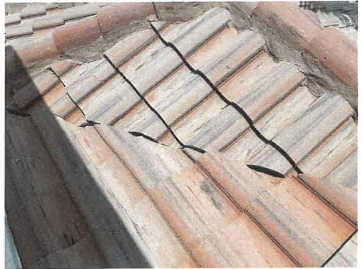
Building 15156: Repaired Cracked Roof Tiles
