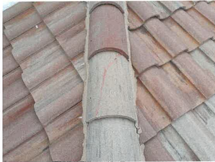
Building 15153: Repaired Cracked Roof Tiles
