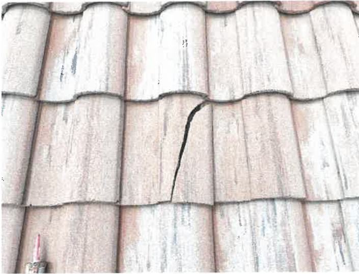
Building 15148: Identified Cracked Roof Tiles
