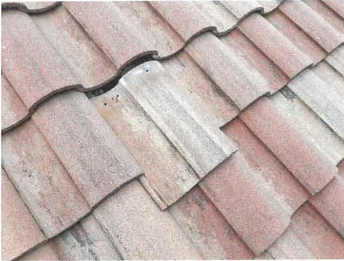
Building 15140: Displaced/Missing Roof Tile
