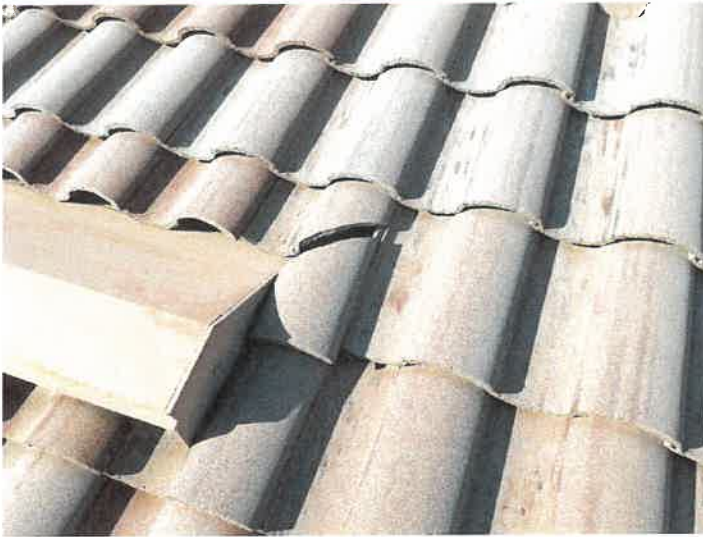
Building 15157: Identified Cracked Roof Tiles
