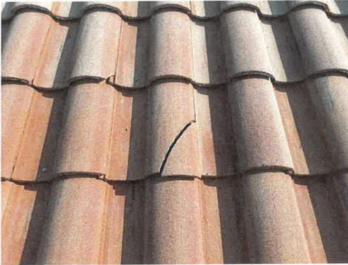
Building 15145: Identified Cracked Roof Tiles
