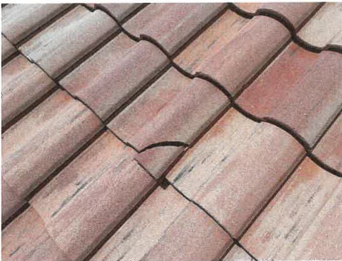
Building 15152: Identified Cracked Roof Tiles
