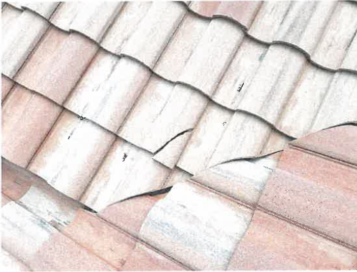
Building 15153: Identified Cracked Roof Tiles
