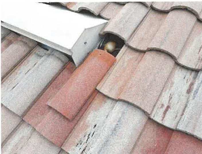
Building 15141: Displaced/Missing Roof Tile
