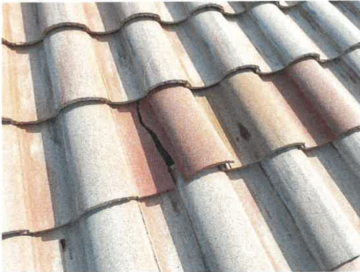
Building 15145: Identified Cracked Roof Tiles
