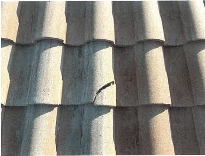
Building 15157: Identified Cracked Roof Tiles
