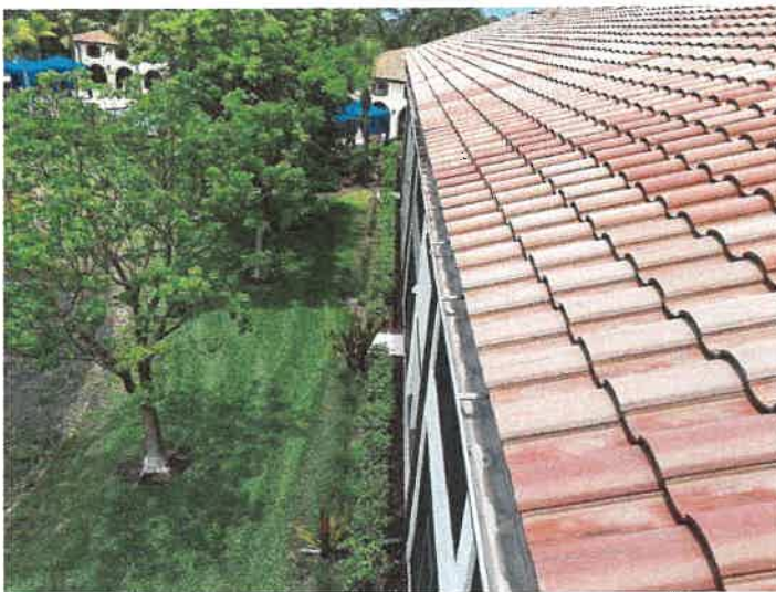
Building 15156: Gutters The gutters appear to be in good condition.
