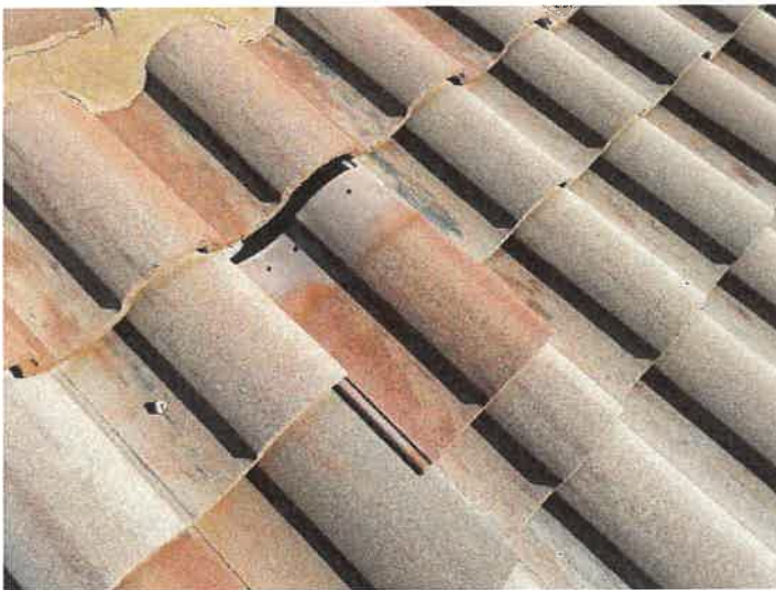
Building 15157: Displaced/Missing Roof Tile
