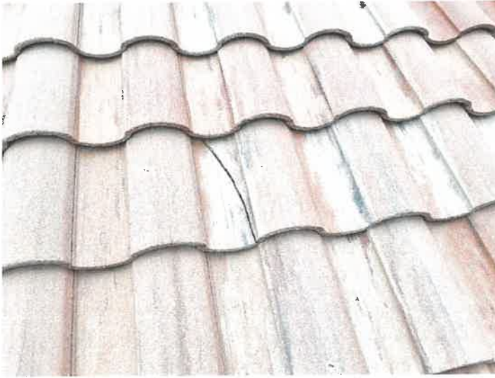
Building 15153: Identified Cracked Roof Tiles
