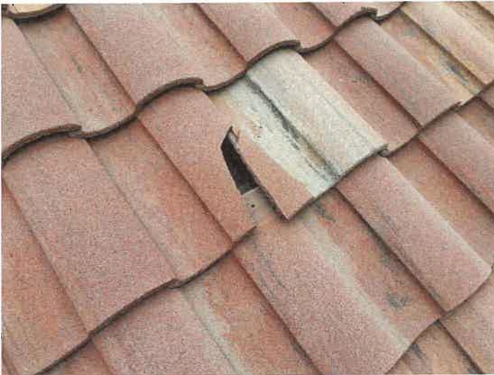
Building 15137: Identified Cracked Roof Tiles
