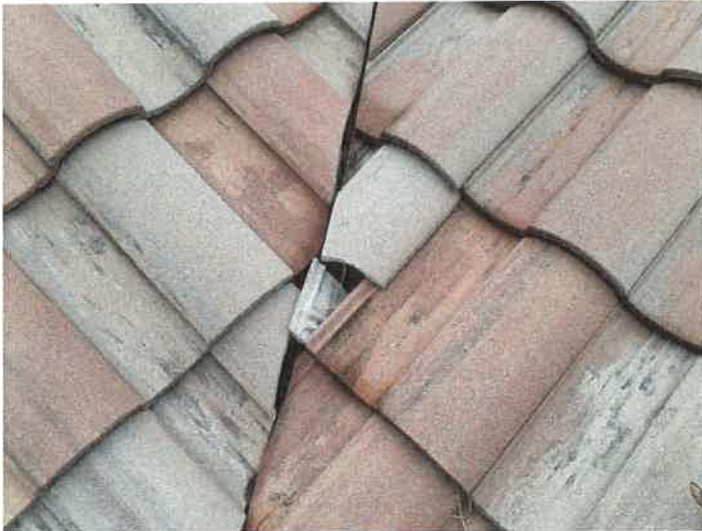
Building 15136: Identified Cracked Roof Tiles
