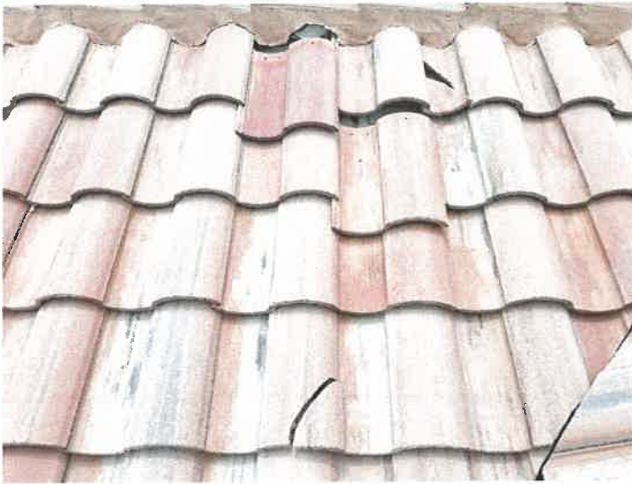
Identified Cracked Roof Tiles
