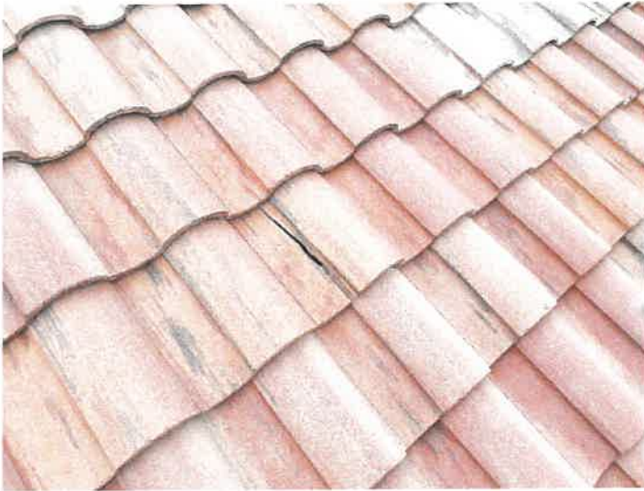
Building 15144: Identified Cracked Roof Tiles
