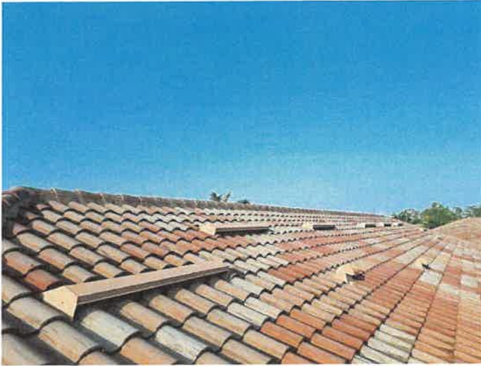
Building 15145: Roof Vents Roof vents appear to be in good condition.
