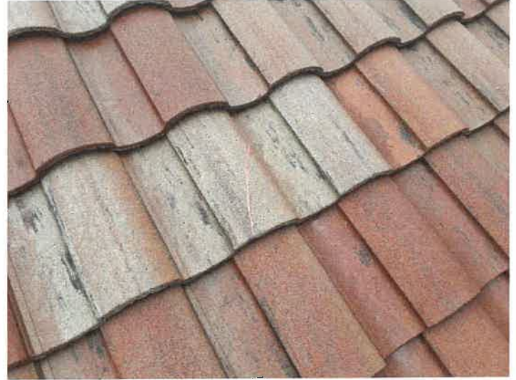
Building 15136: Repaired Cracked Roof Tiles
