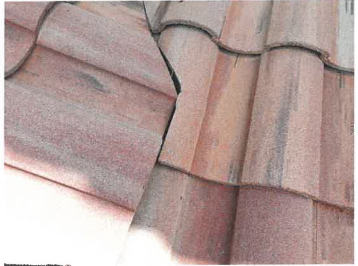
Building 15149: Repaired Cracked Roof Tiles
