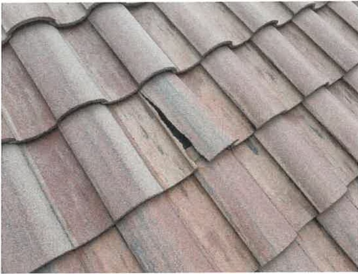
Building 15153: Identified Cracked Roof Tiles
