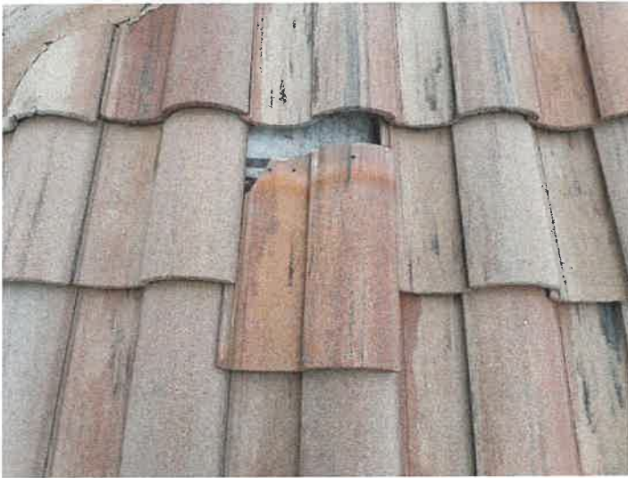
Building 15152: Displaced/Missing Roof Tile
