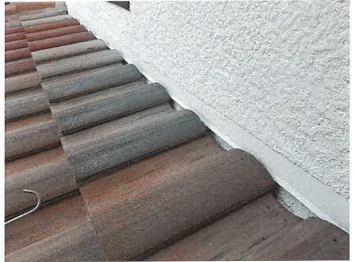
Building 15141: Counter Flashings The counter flashing appears to be in good condition.
