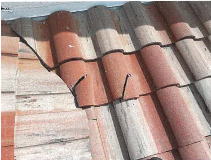
Building 15145: Identified Cracked Roof Tiles Cracked roof tiles can allow premature underlayment deterioration from excessive UV exposure.
