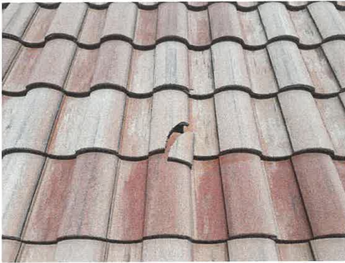
Building 15153: Identified Cracked Roof Tiles
