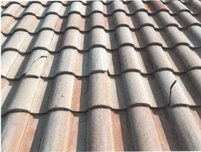
Building 15145: Identified Cracked Roof Tiles
