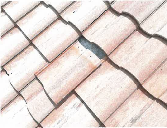
Building 15153: Displaced/Missing Roof Tile
