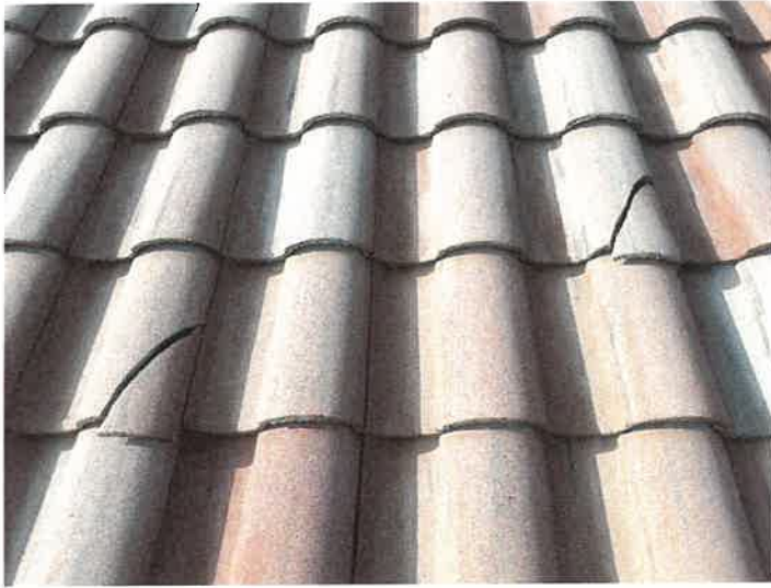
Building 15145: Identified Cracked Roof Tiles
