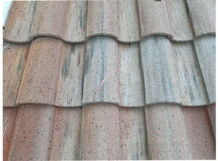
Building 15153: Repaired Cracked Roof Tiles
