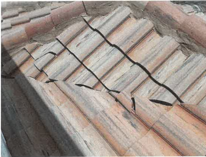
Building 15156: Identified Cracked Roof Tiles
