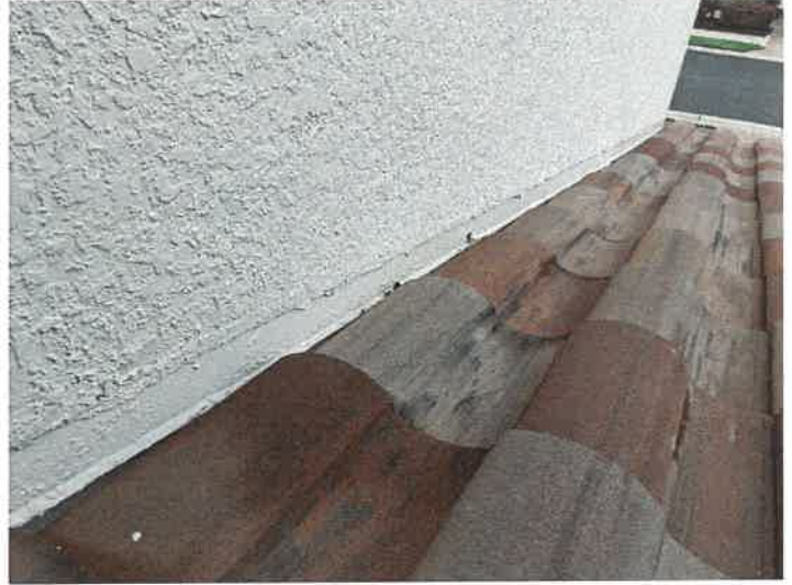
Building 15137: Counter Flashings The counter flashing appears to be in good condition.
