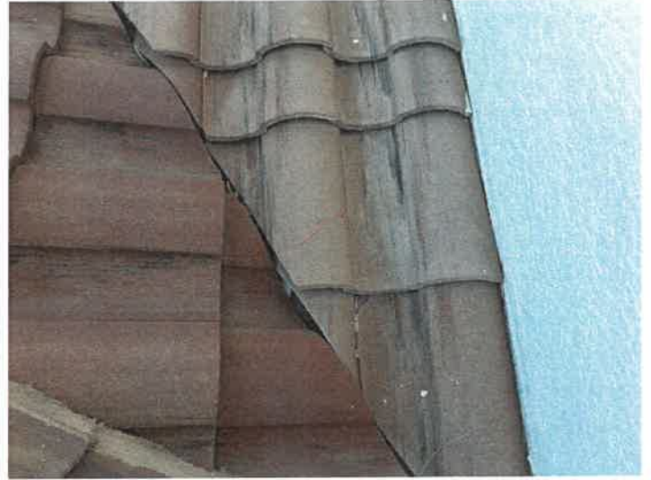
Building 15157: Repaired Cracked Roof Tiles
