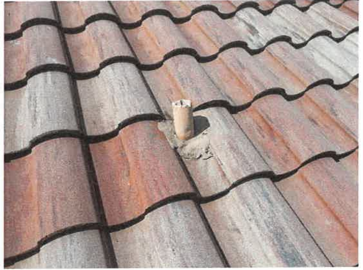
Building 15149: Lead Boots Lead boots appear to be in good condition.
