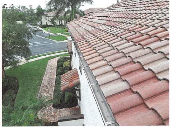
Building 15137: Gutters The gutters appear to be in good condition.
