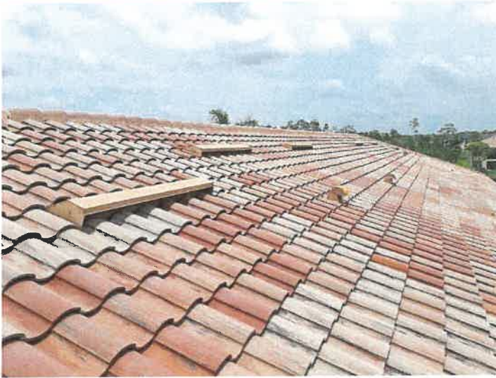
Building 15144: Roof Vents Roof vents appear to be in good condition.
