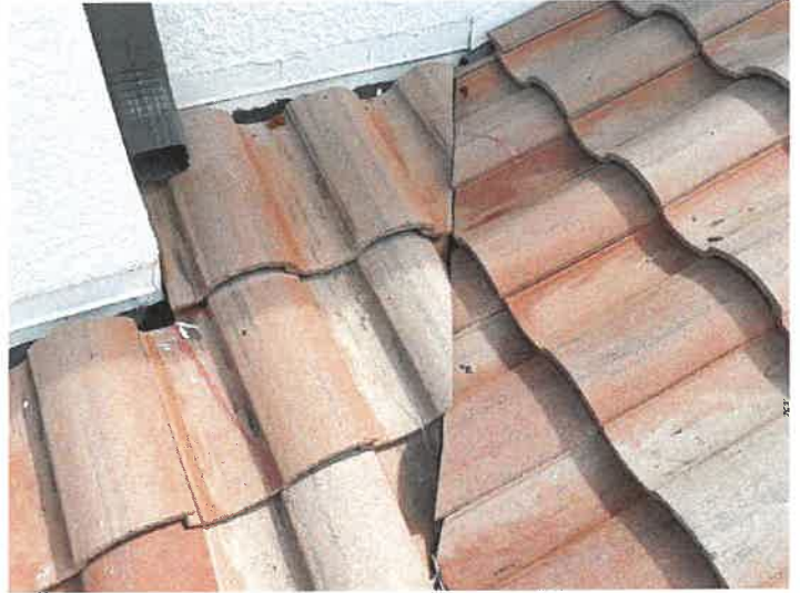
Building 15145: Repaired Cracked Roof Tiles
