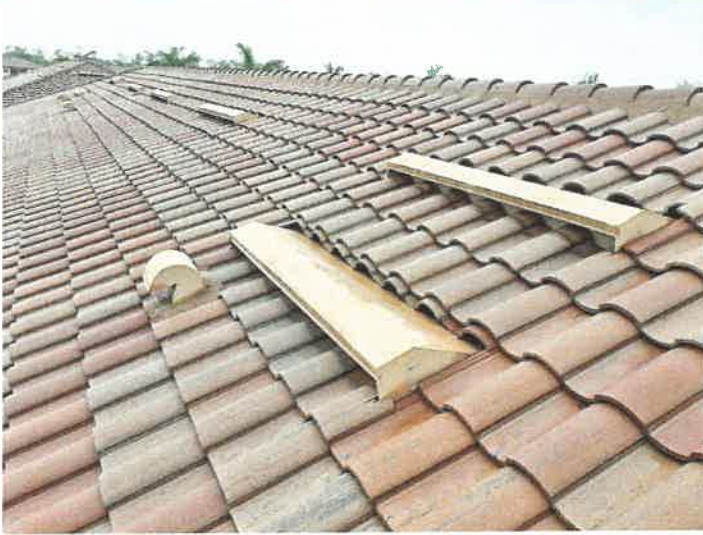
Building 15136: Roof Vents Roof vents appear to be in good condition.
