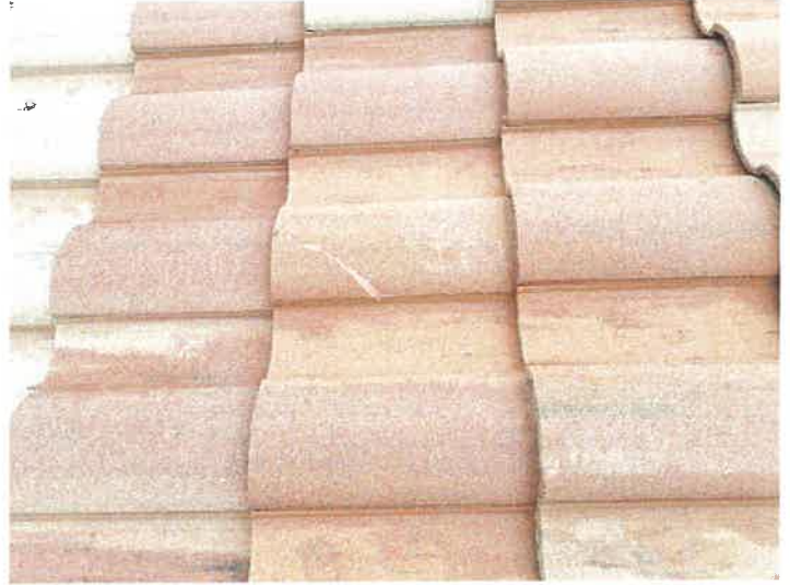
Building 15141: Repaired Cracked Roof Tiles
