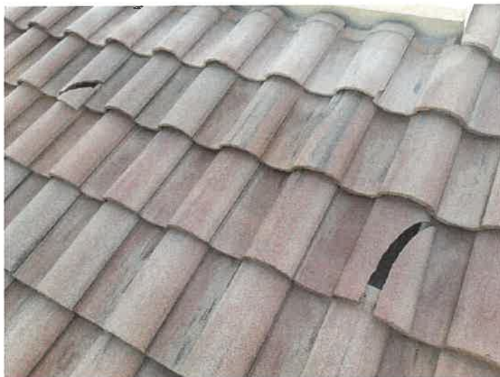
Building 15145: Identified Cracked Roof Tiles
