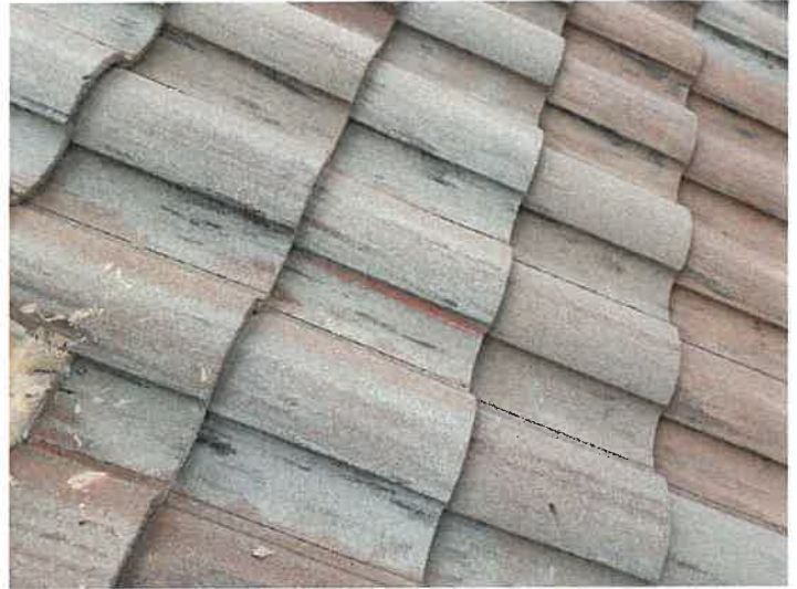
Building 15152: Repaired Cracked Roof Tiles
