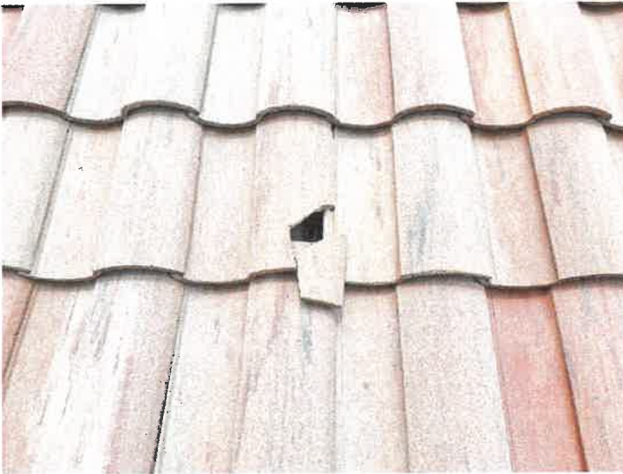
Building 15144: Identified Cracked Roof Tiles
