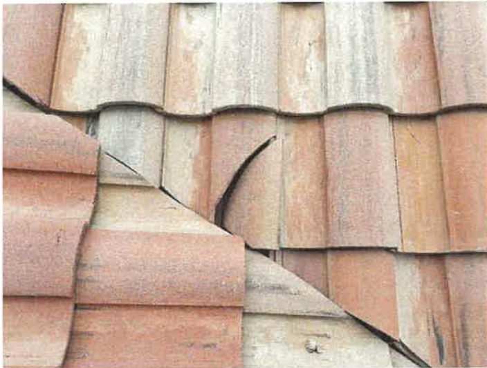
Building 15140: Identified Cracked Roof Tiles
