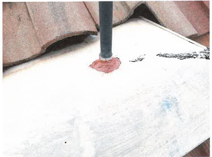
Building 15141: Roof Vents Roof vents appear to be in good condition.
