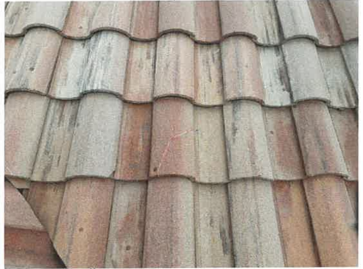
Building 15152: Repaired Cracked Roof Tiles
