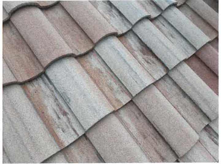
Building 15153: Repaired Cracked Roof Tiles The cracked roof tiles were repaired with Titebond sealant.
