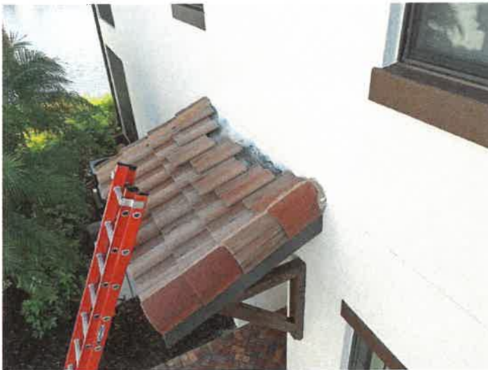
Building 15157: Displaced/Missing Roof Tile
