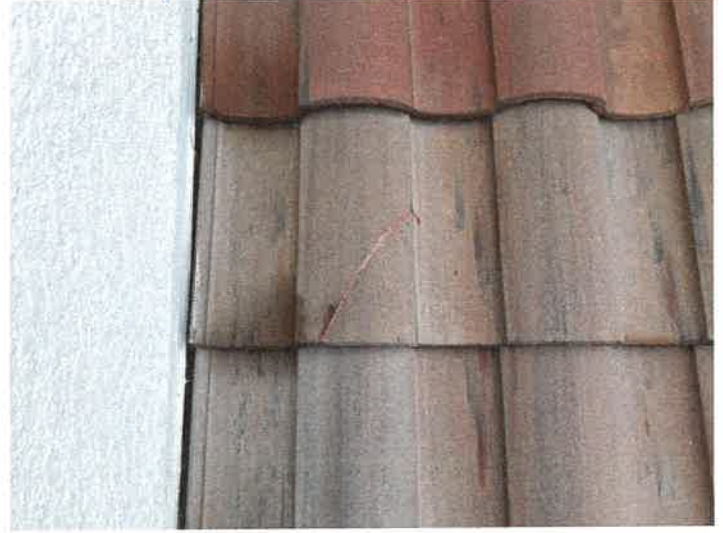
Building 15136: Repaired Cracked Roof Tiles
