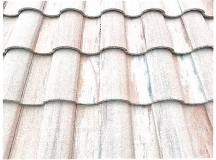
Building 15153: Repaired Cracked Roof Tiles
