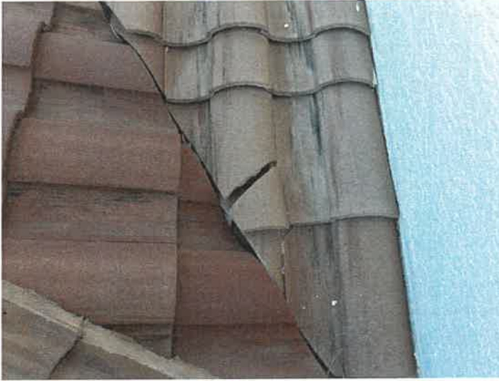
Building 15157: Identified Cracked Roof Tiles
