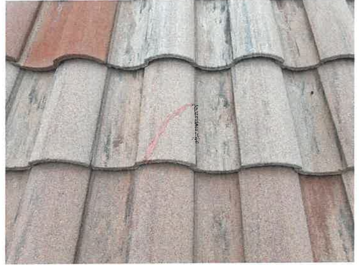
Building 15140: Repaired Cracked Roof Tiles
