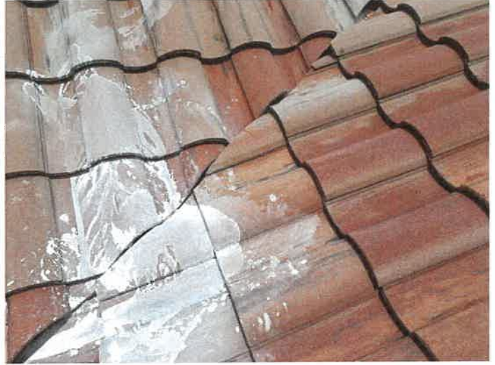
Building 15144: Repaired Cracked Roof Tiles
