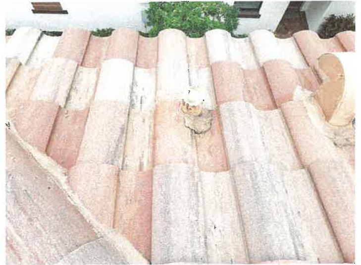
Building 15137: Repaired Cracked Roof Tiles
