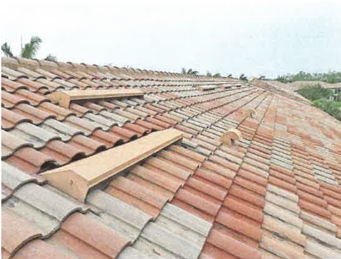
Building 15137: Roof Vents
