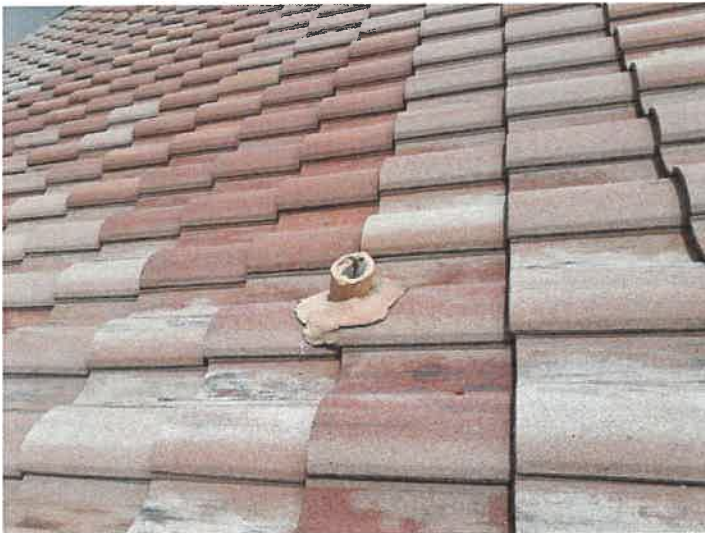
Building 15144: Lead Boots Lead boots appear to be in good condition.
