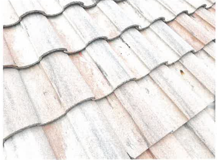
Building 15140: Repaired Cracked Roof Tiles
