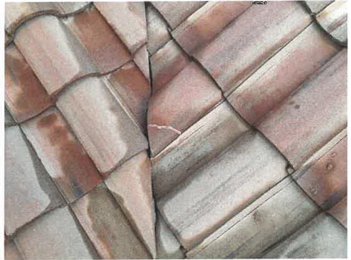
Building 15152: Repaired Cracked Roof Tiles
