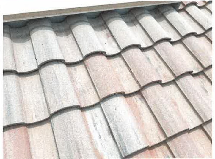
Building 15153: Repaired Cracked Roof Tiles
