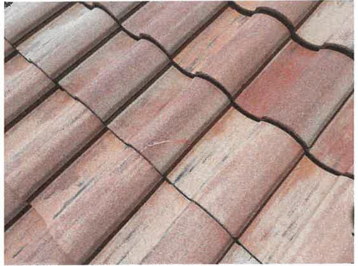
Building 15152: Repaired Cracked Roof Tiles
