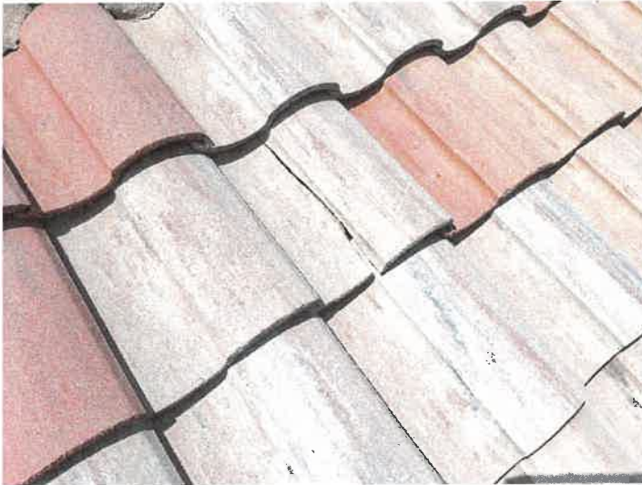
Building 15148: Identified Cracked Roof Tiles
