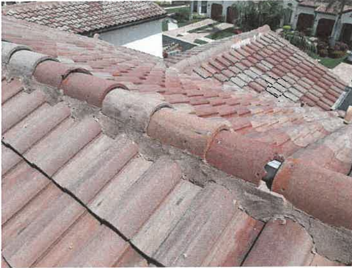
Building 15148: Broken Ridge Tiles
