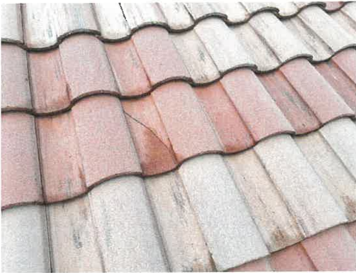
Building 15152: Identified Cracked Roof Tiles
