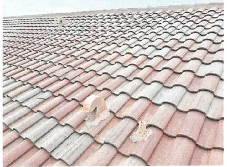
Building 15140: Roof Vents Roof vents appear to be in good condition.
