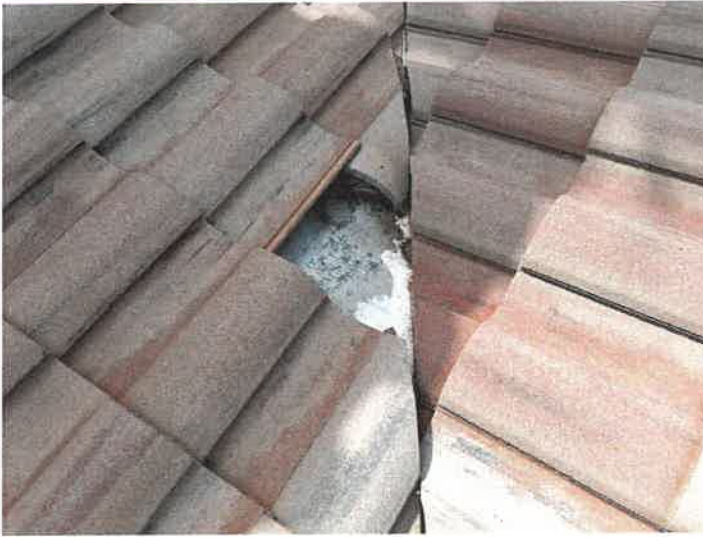
Building 15145: Missing Roof Tile
