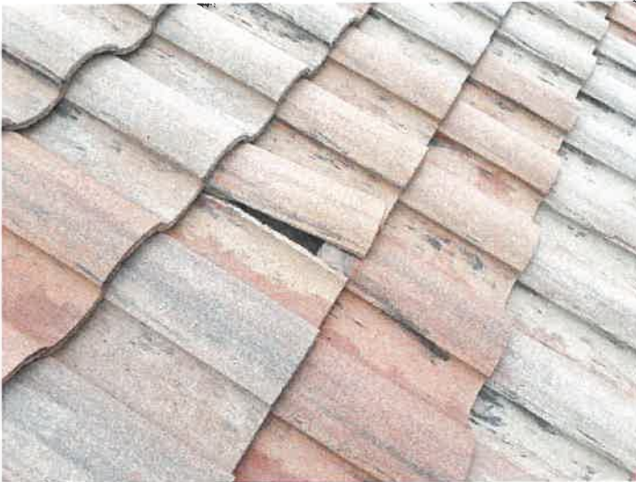
Building 15140: Identified Cracked Roof Tiles
