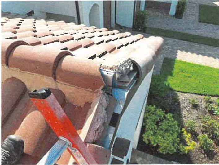
Building 15157: Cracked/Missing Ridge Tiles Crowther Roofing suggests replacing three (3) ridge tiles.
