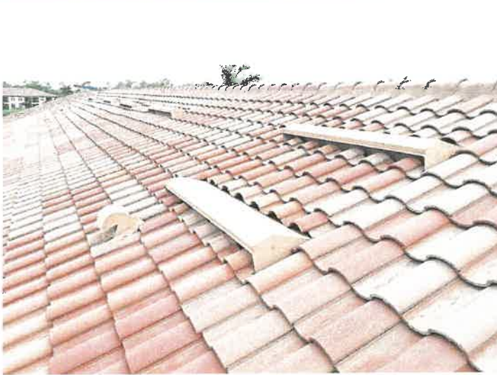
Building 15140: Roof Vents Roof vents appear to be in good condition.
