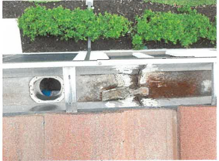
Building 15137: Gutter- Interior gutter issue Interior gutter has issues that will/have lead to water penetration. Remove and replace waterproofing material immediately.
