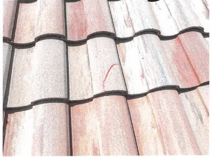
Building 15148: Repaired Cracked Roof Tiles
