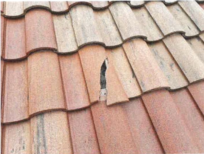
Building 15136: Identified Cracked Roof Tiles Cracked roof tiles can allow premature underlayment deterioration from excessive UV exposure.
