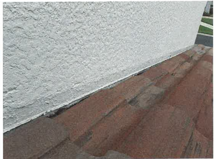
Building 15136: Counter Flashings
