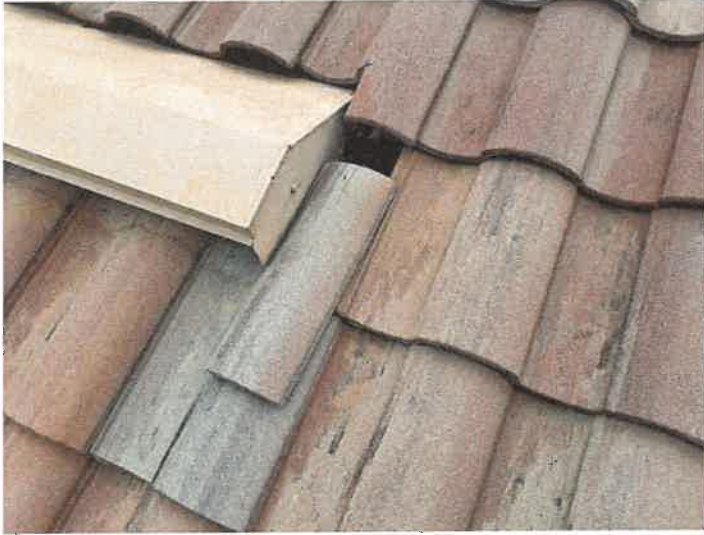
Building 15137: Displaced/Missing Roof Tile
