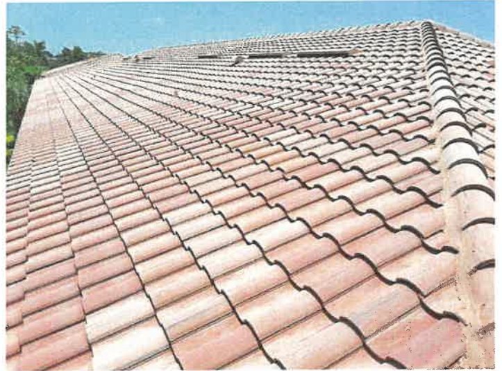
Building 15152: Surface Overview The roof surface appears to be in good, maintainable condition at this time.
