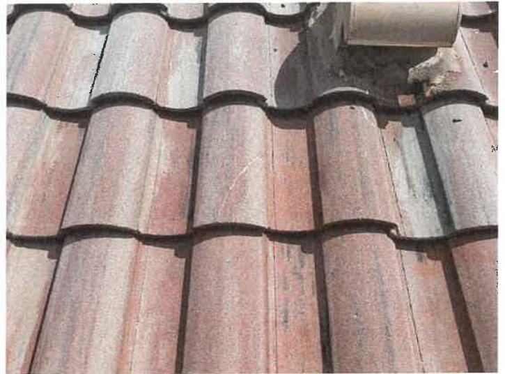
Building 15152: Repaired Cracked Roof Tiles
