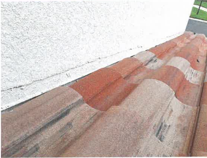
Building 15140: Counter Flashings
