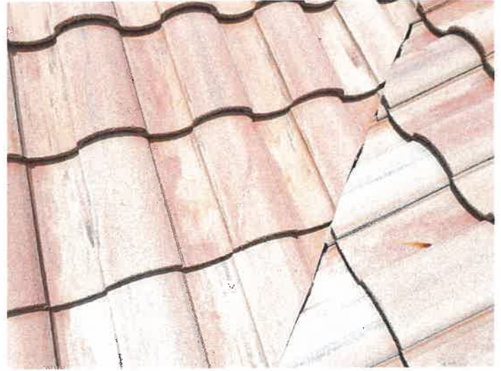
Building 15153: Repaired Cracked Roof Tiles
