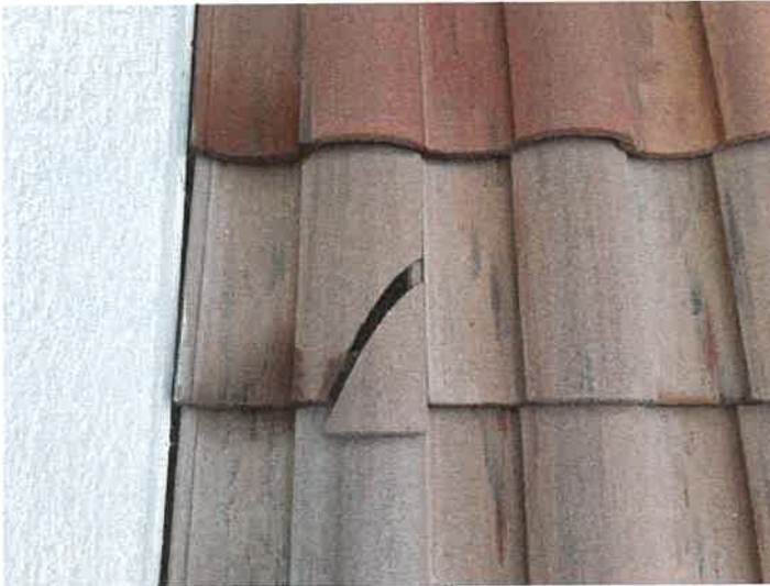
Building 15136: Identified Cracked Roof Tiles
