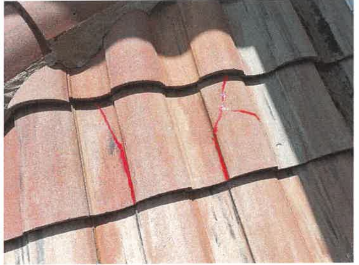
Building 15148: Repaired Cracked Roof Tiles
