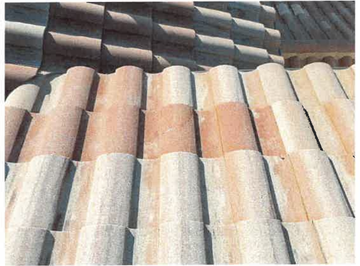
Building 15157: Repaired Cracked Roof Tiles
