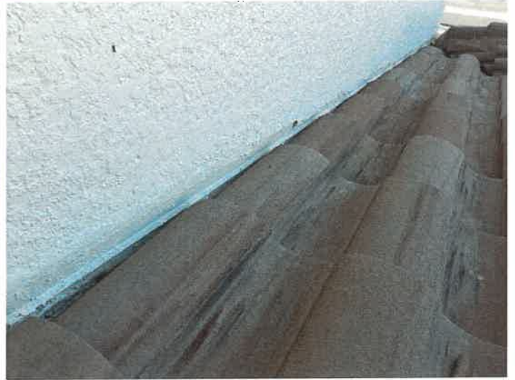
Building 15157: Counter Flashings The counter flashing appears to be in good condition.
