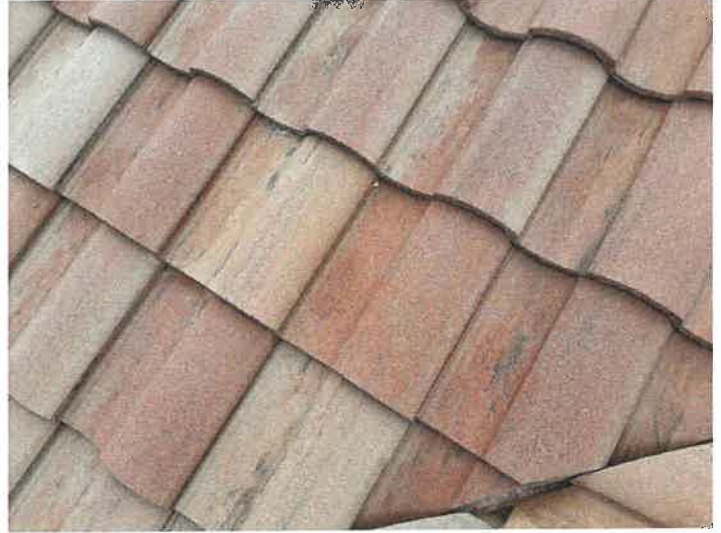
Building 15137: Repaired Displaced/Missing Roof Tile
