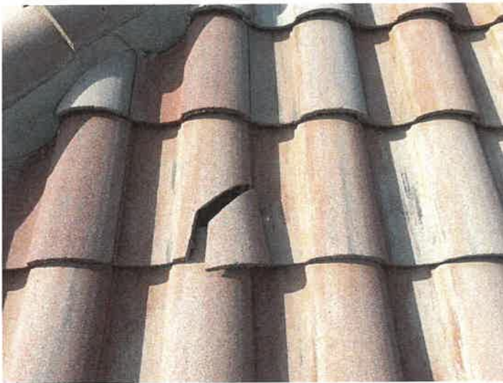
Building 15145: Identified Cracked Roof Tiles
