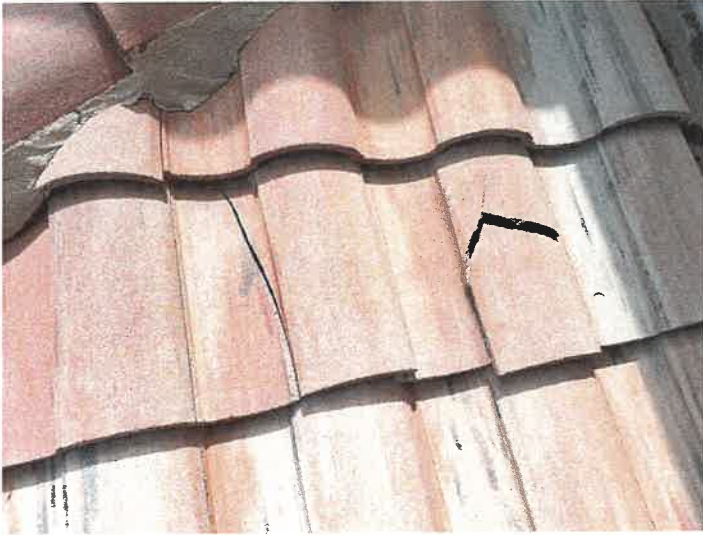
Building 15148: Identified Cracked Roof Tiles
