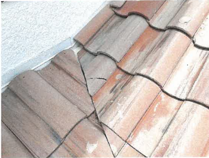
Building 15148: Identified Cracked Roof Tiles
