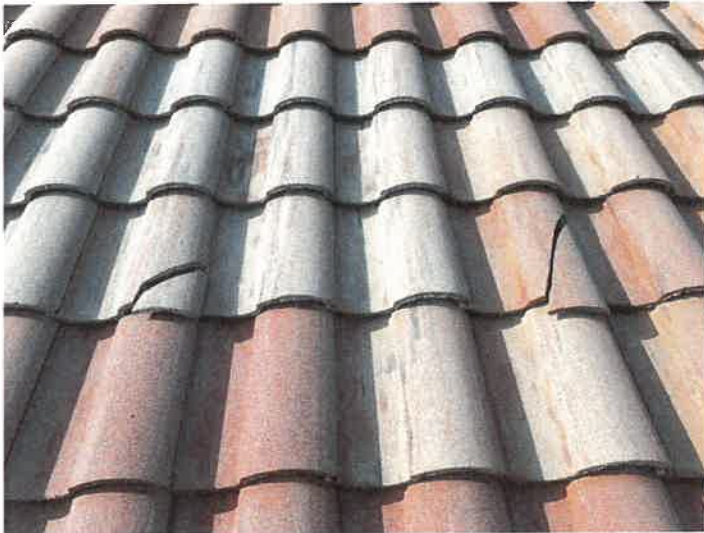
Building 15145: Identified Cracked Roof Tiles
