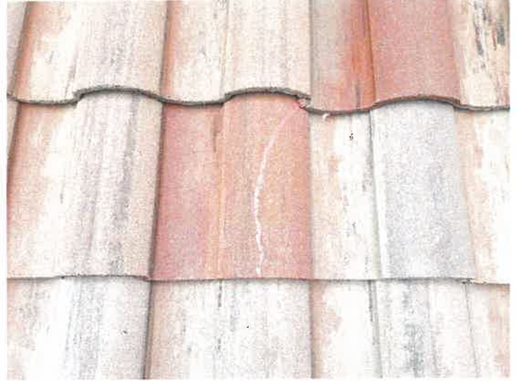
Building 15140: Repaired Cracked Roof Tiles
