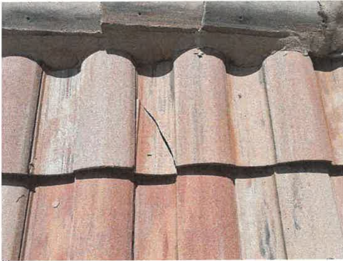
Building 15152: Identified Cracked Roof Tiles
