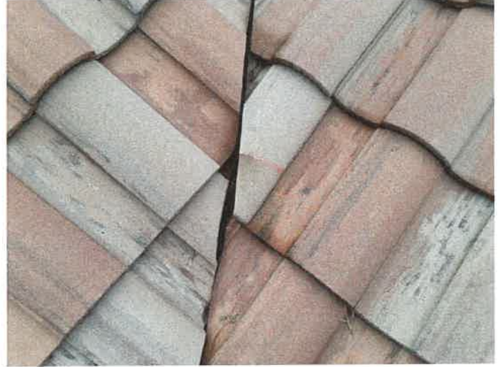
Building 15136: Repaired Cracked Roof Tiles
