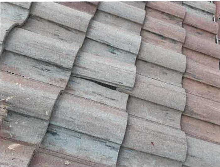
Building 15152: Identified Cracked Roof Tiles
