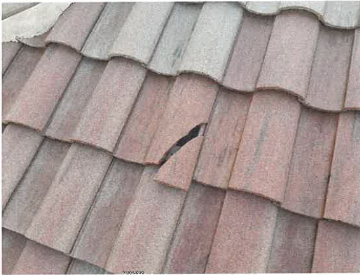
Building 15145: Identified Cracked Roof Tiles
