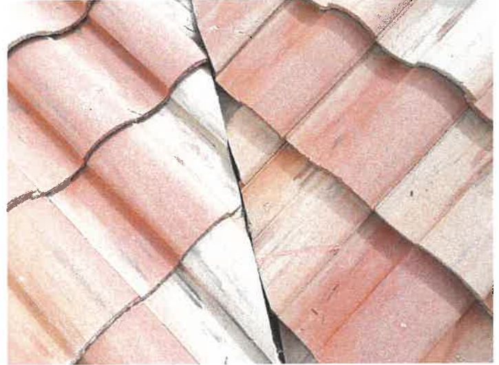
Building 15145: Repaired Cracked Roof Tiles The cracked roof tiles were repaired with Titebond sealant.
