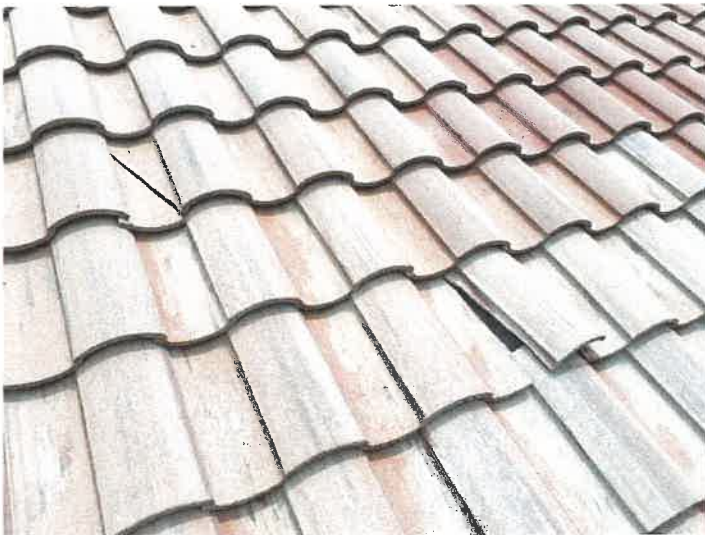
Building 15153: Identified Cracked Roof Tiles
