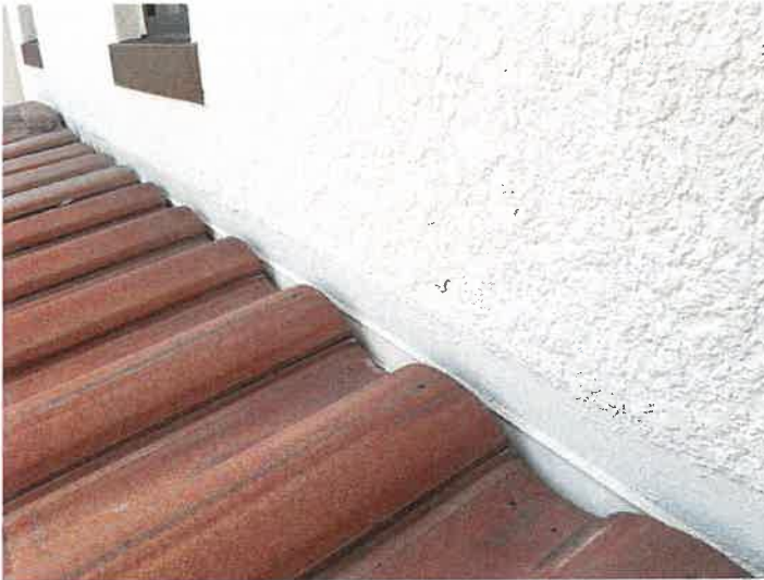
Building 15148: Counter Flashings
