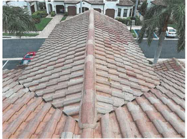
Building 15156: Valley The valley tiles appear to be in good condition.
