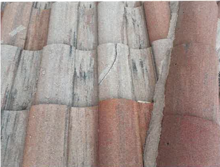
Building 15140: Identified Cracked Roof Tiles
