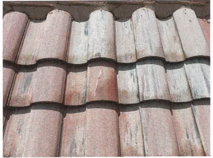
Building 15152: Repaired Cracked Roof Tiles
