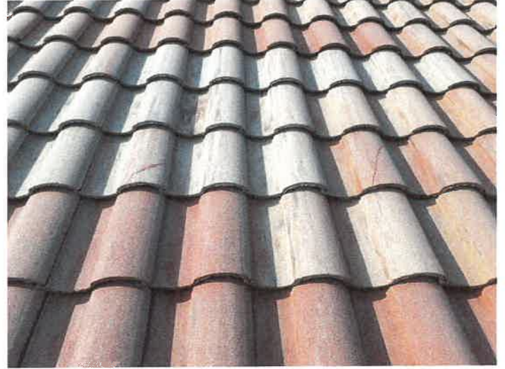
Building 15145: Repaired Cracked Roof Tiles
