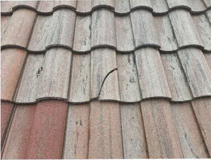
Building 15136: Identified Cracked Roof Tiles Cracked roof tiles can allow premature underlayment deterioration from excessive UV exposure.
