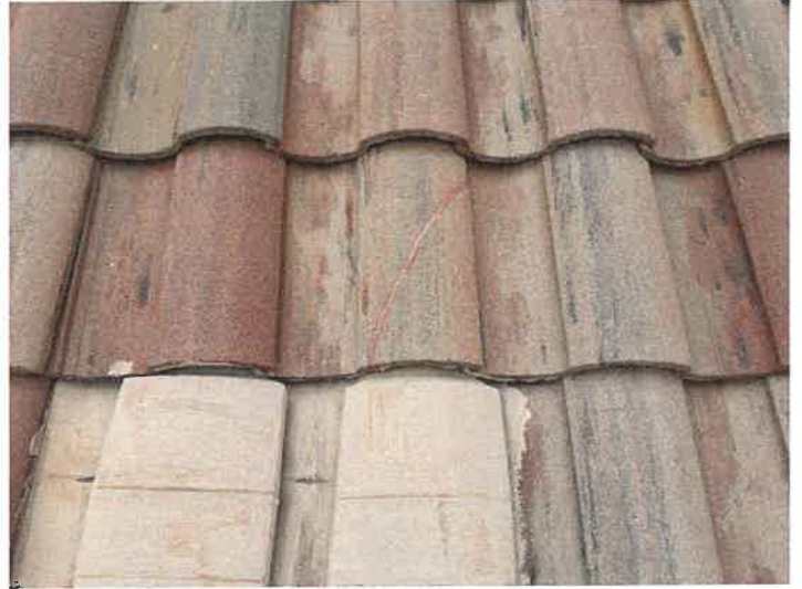
Building 15137: Repaired Cracked Roof Tiles
