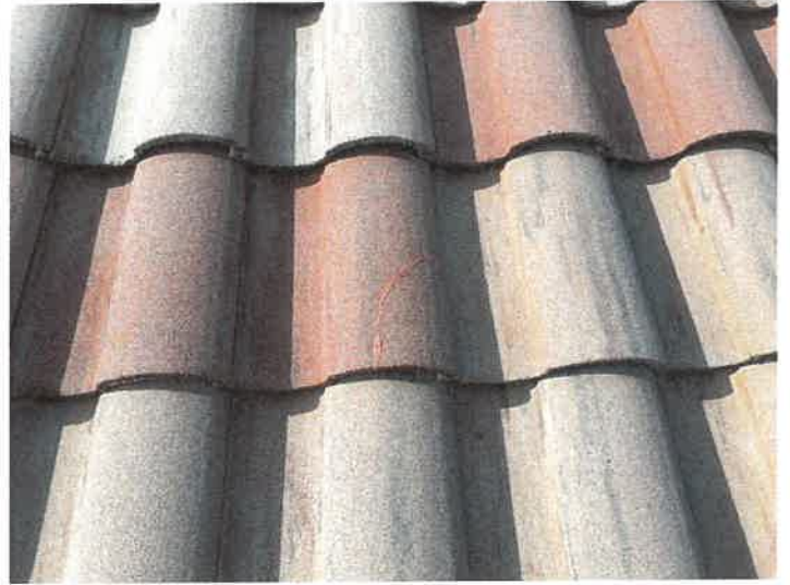
Building 15145: Repaired Cracked Roof Tiles
