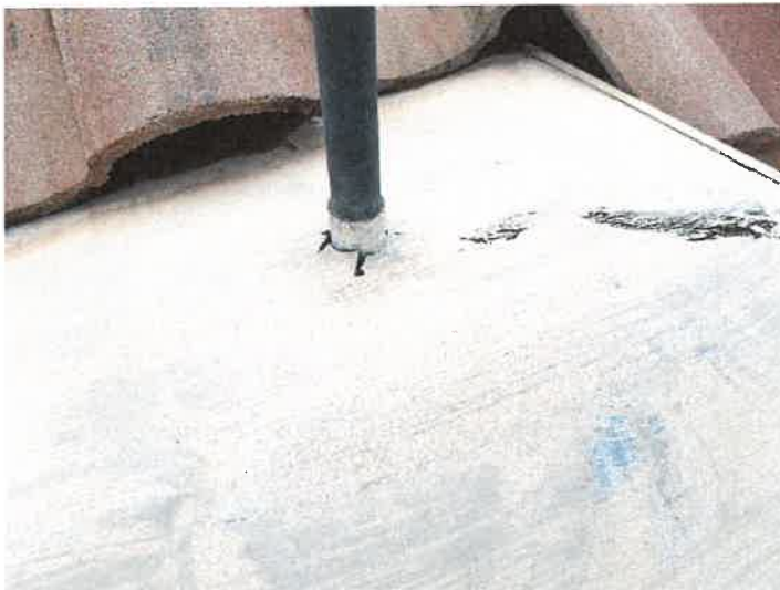
Building 15141: Sealant Failure Identified a void in the sealant.
