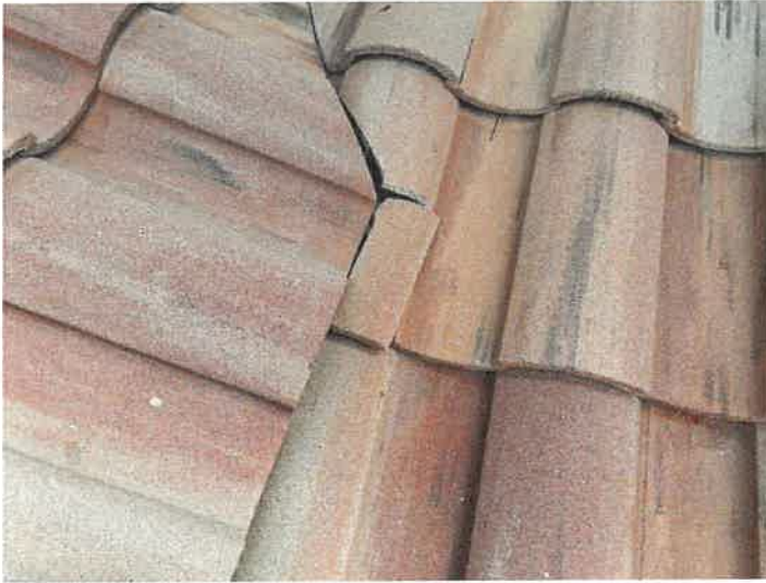
Building 15149: Identified Cracked Roof Tiles
