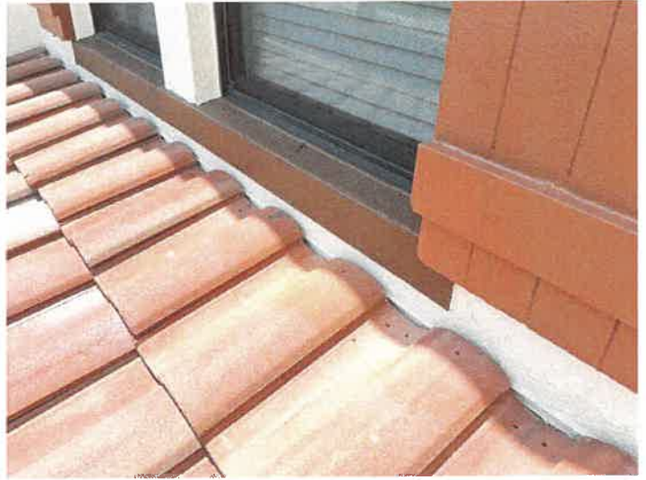
Building 15152: Counter Flashings
