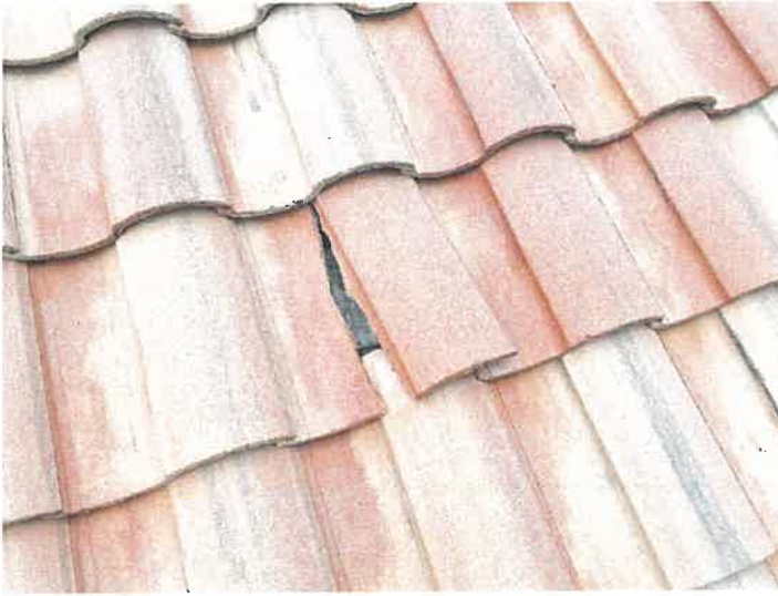
Building 15156: Identified Cracked Roof Tiles Cracked roof tiles can allow premature underlayment deterioration from excessive UV exposure.
