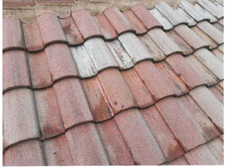
Building 15152: Repaired Cracked Roof Tiles
