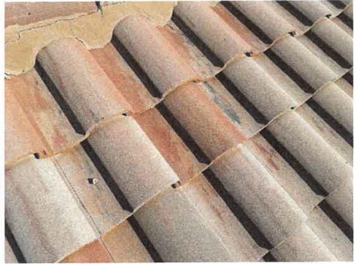
Building 15157: Repaired Displaced/Missing Roof Tile
