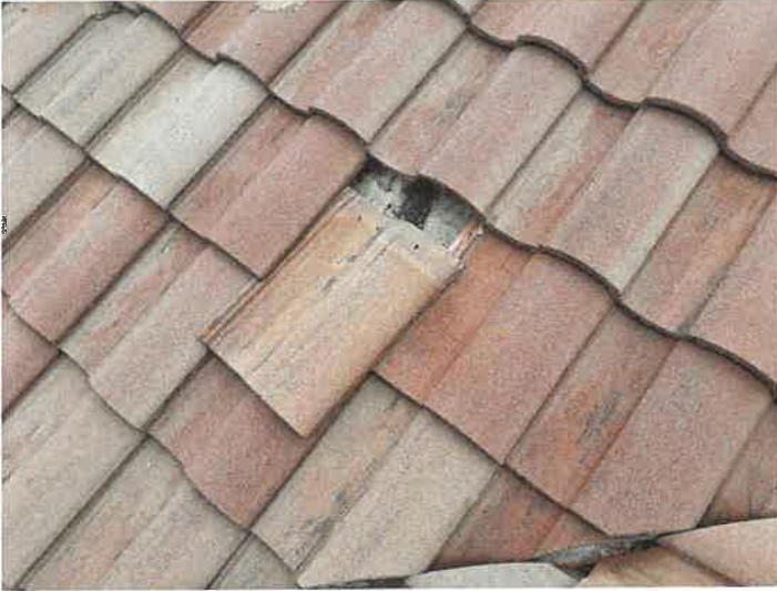
Building 15137: Displaced/Missing Roof Tile
