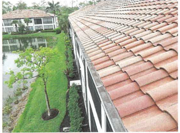
Building 15141: Gutters The gutters appear to be in good condition.
