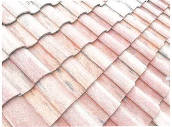
Building 15144: Repaired Cracked Roof Tiles
