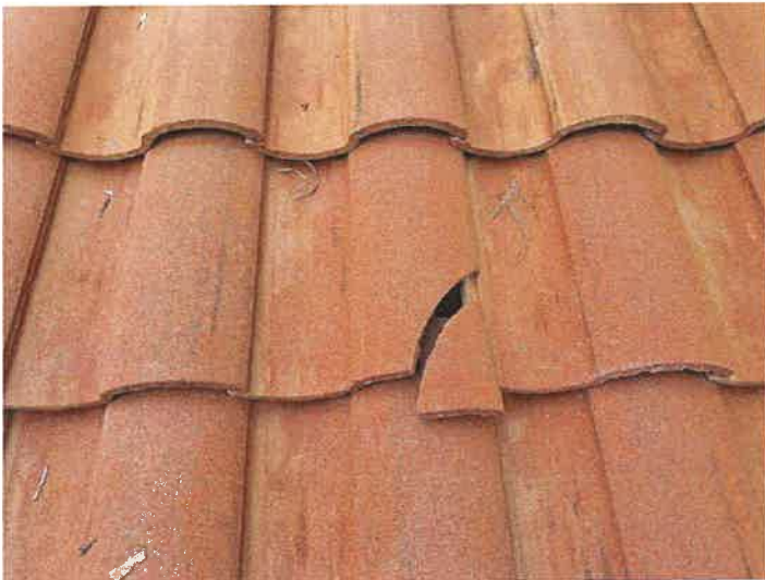
Building 15141: Identified Cracked Roof Tiles
