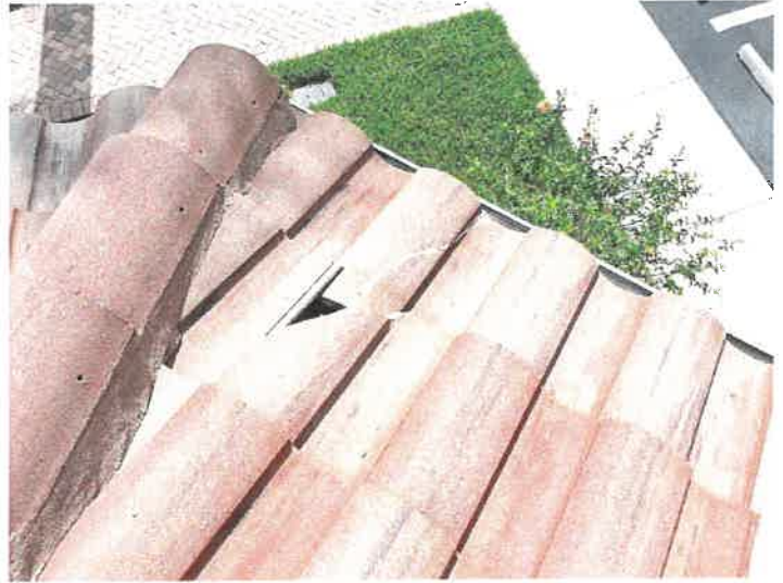
Building 15145: Broken Roof Tile
