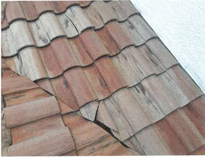
Building 15149: Identified Cracked Roof Tiles
