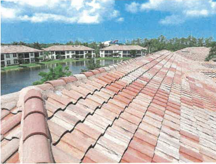
Building 15148: Ridge Tiles Ridge tiles appear to be in good condition.
