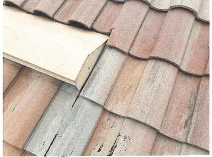
Building 15137: Repaired Displaced/Missing Roof Tile
