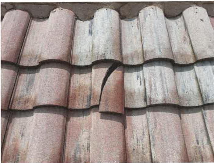
Building 15152: Identified Cracked Roof Tiles
