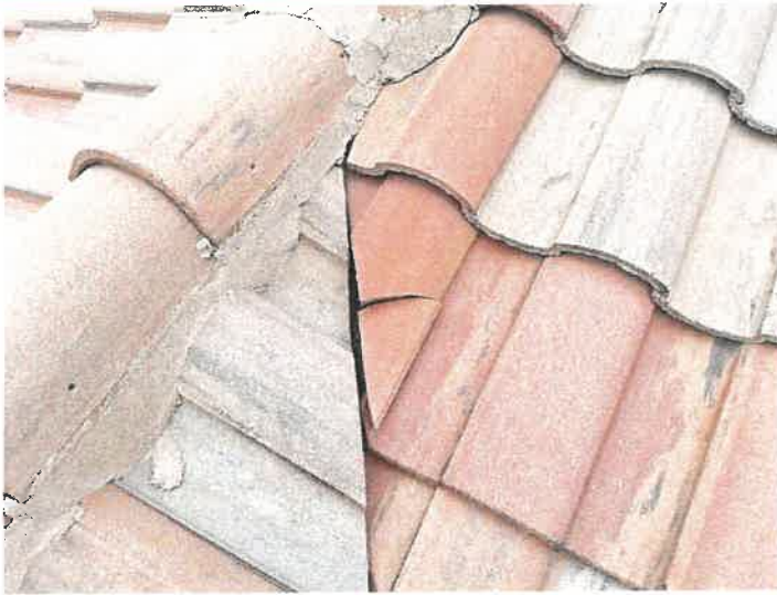
Building 15140: Identified Cracked Roof Tiles
