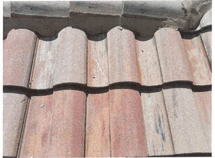
Building 15152: Repaired Cracked Roof Tiles
