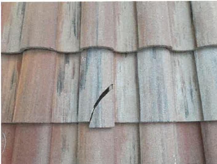
Building 15153: Identified Cracked Roof Tiles
