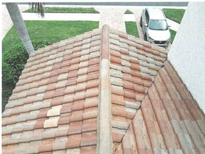
Building 15153: Appearance Overview - Lower Roof The roof appearance is in good, maintainable condition.
