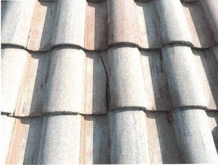
Building 15145: Identified Cracked Roof Tiles
