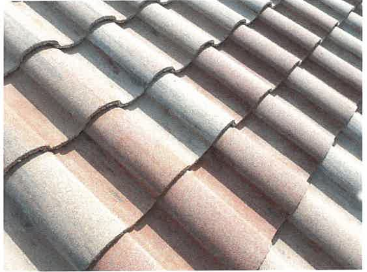
Building 15145: Repaired Displaced/Missing Roof Tile
