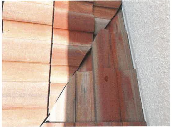
Building 15156: Repaired Cracked Roof Tiles
