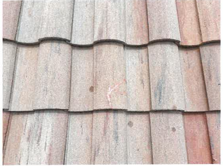
Building 15144: Repaired Cracked Roof Tiles
