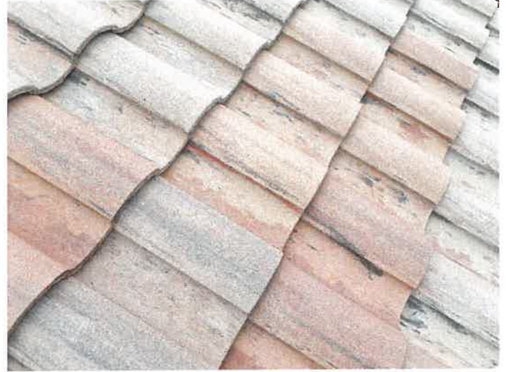
Building 15140: Repaired Cracked Roof Tiles
