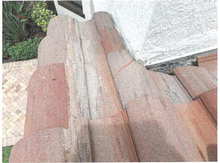
Building 15144: Repaired Cracked Roof Tiles
