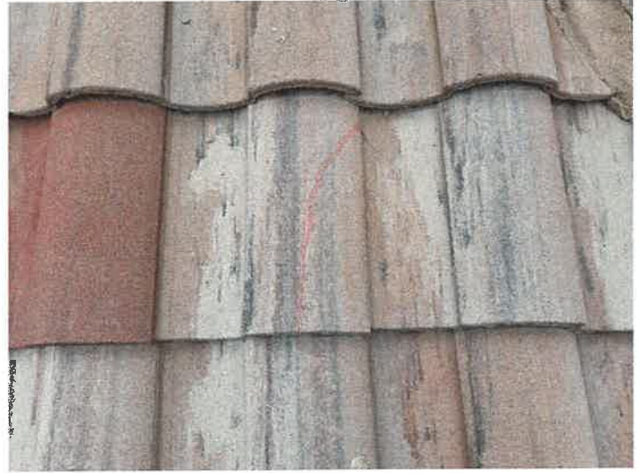
Building 15137: Repaired Cracked Roof Tiles
