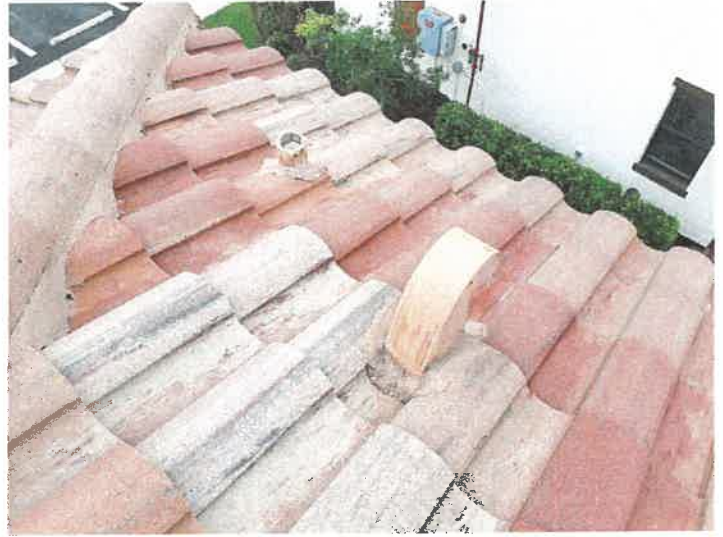
Building 15141: Lead Boots Lead boots appear to be in good condition.
