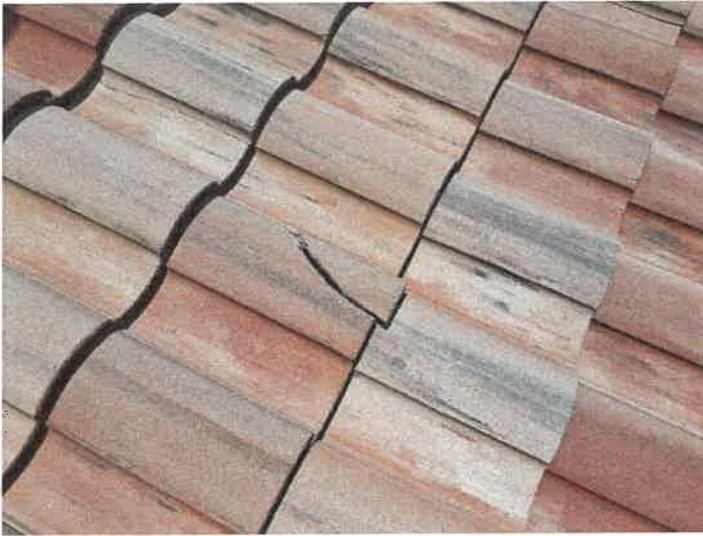
Building 15156: Identified Cracked Roof Tiles
