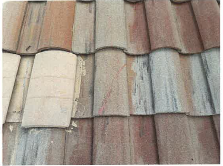
Building 15145: Repaired Cracked Roof Tiles
