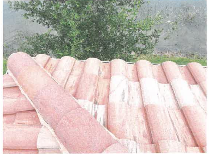
Building 15144: Repaired Cracked Roof Tiles
