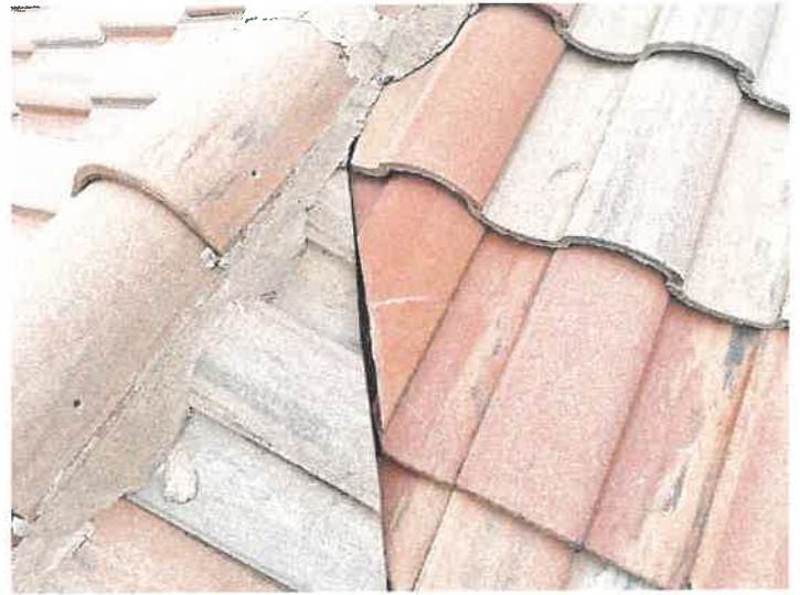
Building 15140: Repaired Cracked Roof Tiles
