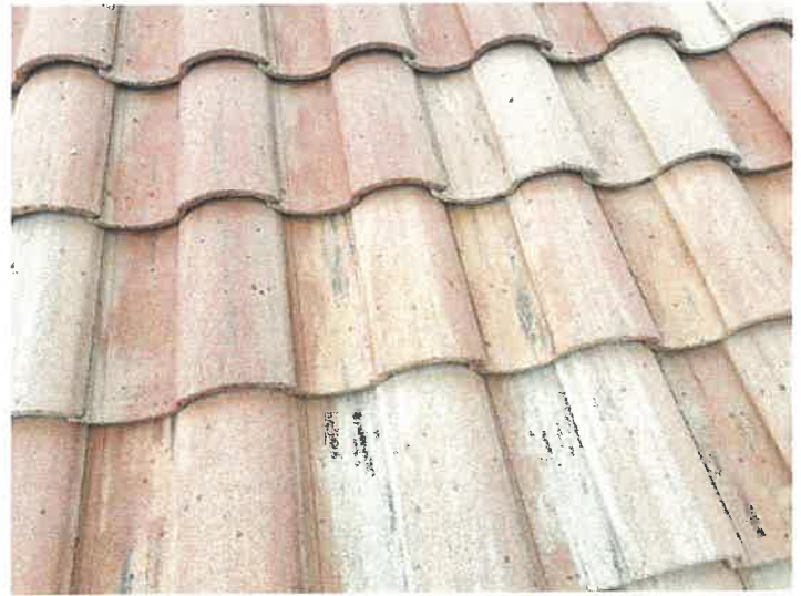
Building 15152: Repaired Cracked Roof Tiles The cracked roof tiles were repaired with Titebond sealant.
