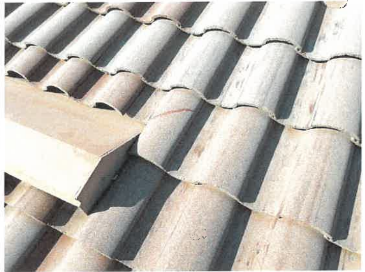
Building 15157: Repaired Cracked Roof Tiles
