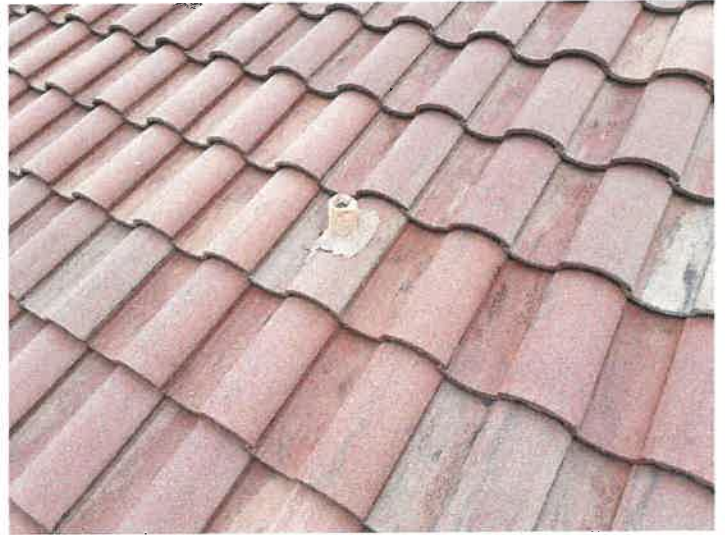
Building 15140: Lead Boots Lead boots appear to be in good condition.
