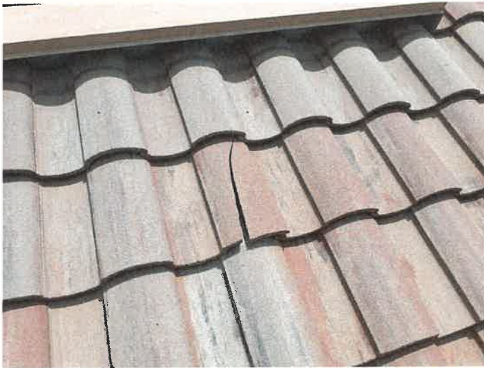
Building 15153: Identified Cracked Roof Tiles
