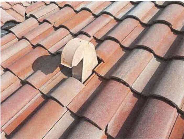
Building 15145: Missing Mortar Identified missing mortar around of the roof vent. Crowther Roofing suggests installing mortar.
