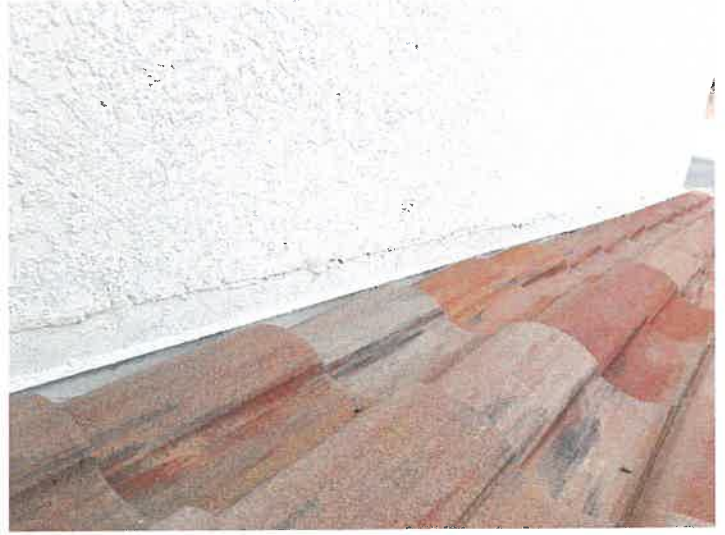
Building 15144: Counter Flashings
