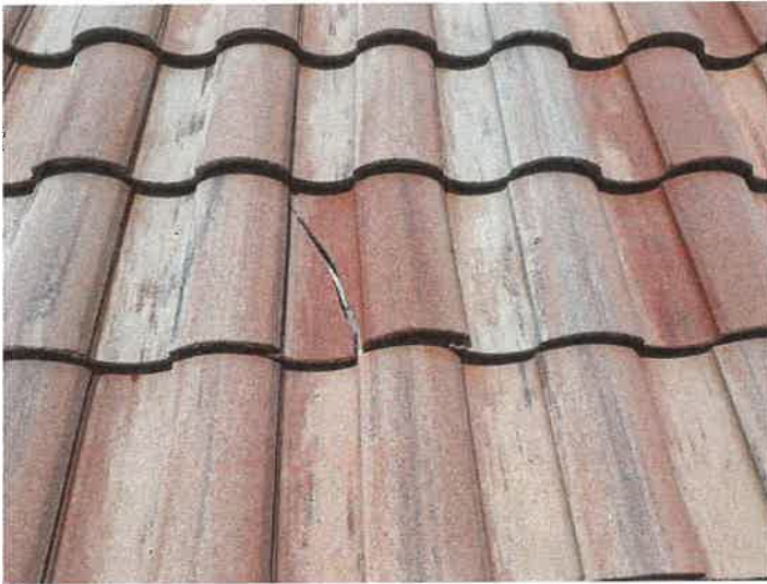
Building 15153: Identified Cracked Roof Tiles
