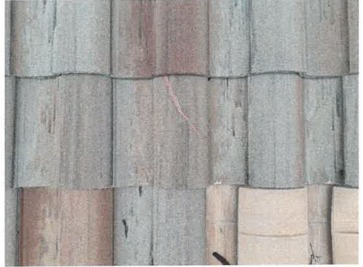
Building 15136: Repaired Cracked Roof Tiles
