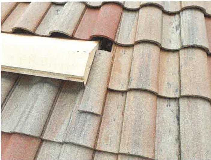
Building 15136: Displaced/Missing Roof Tile
