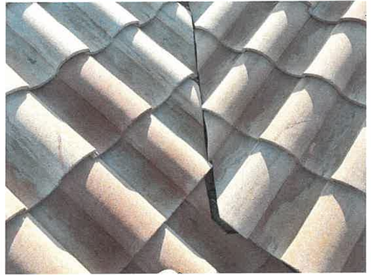
Building 15157: Repaired Cracked Roof Tiles
