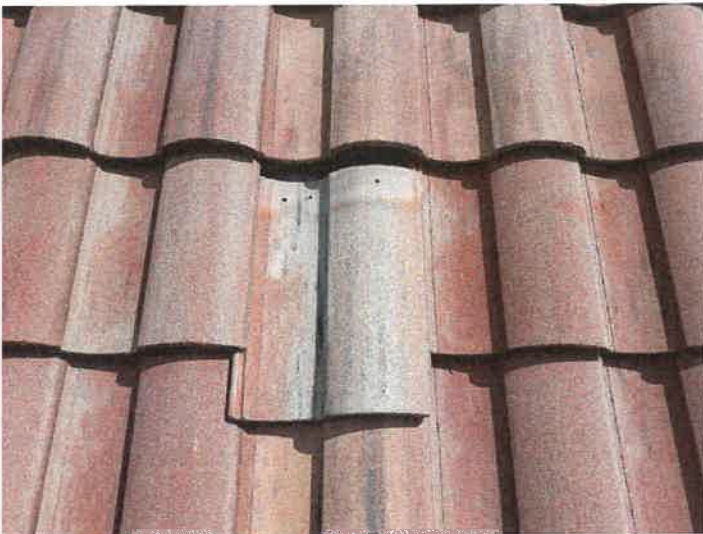
Building 15152: Displaced/Missing Roof Tile
