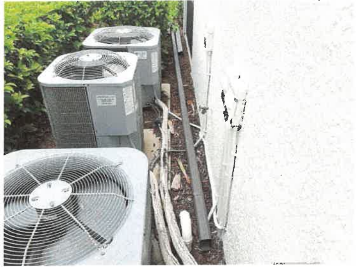
Building 15148: Location Crowther Roofing suggests reinstalling the downspout.
