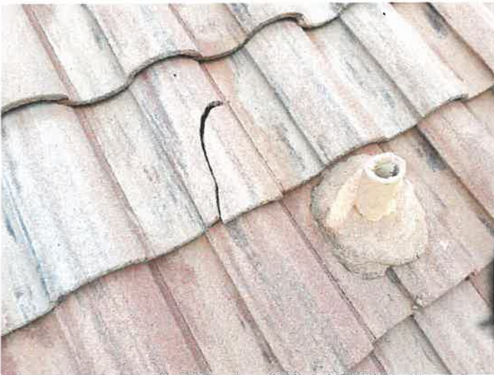
Building 15152: Identified Cracked Roof Tiles Cracked roof tiles can allow premature underlayment deterioration from excessive UV exposure.
