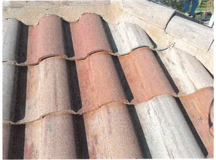
Building 15157: Repaired Cracked Roof Tiles
