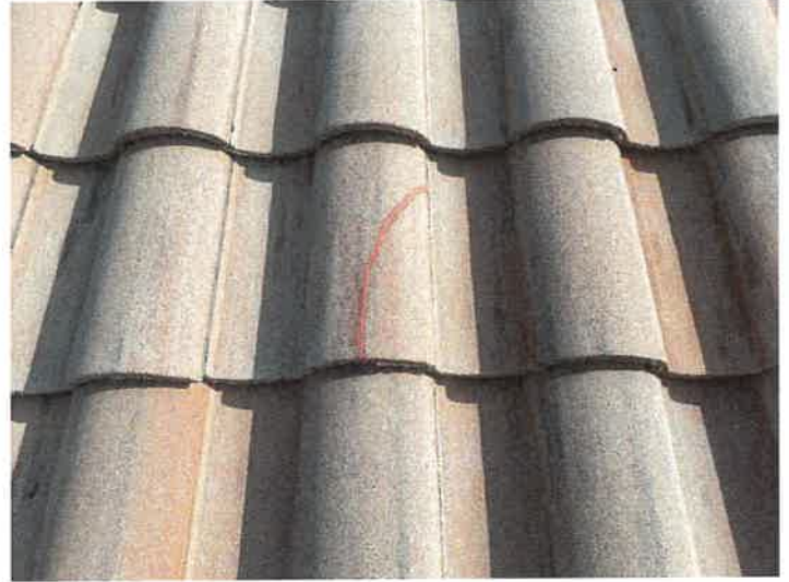
Building 15145: Repaired Cracked Roof Tiles
