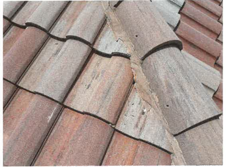
Building 15153: Repaired Displaced/Missing Roof Tile
