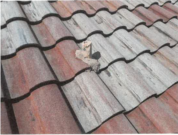
Building 15149: Lead Boots Lead boots appear to be in good condition.
