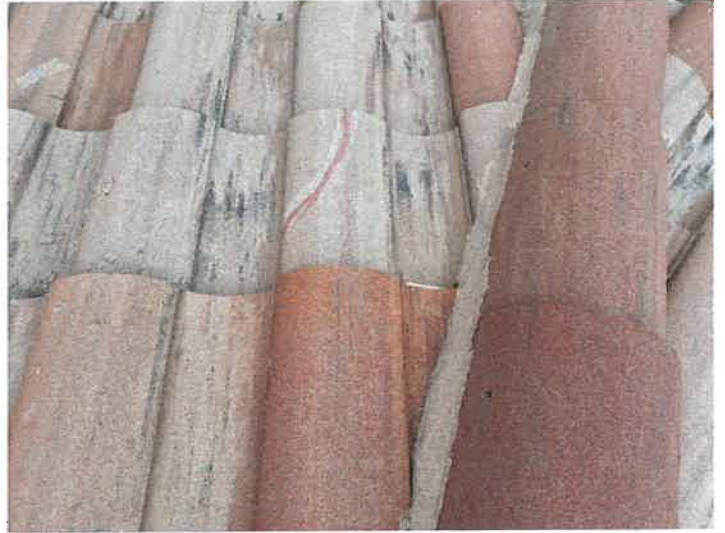
Building 15140: Repaired Cracked Roof Tiles
