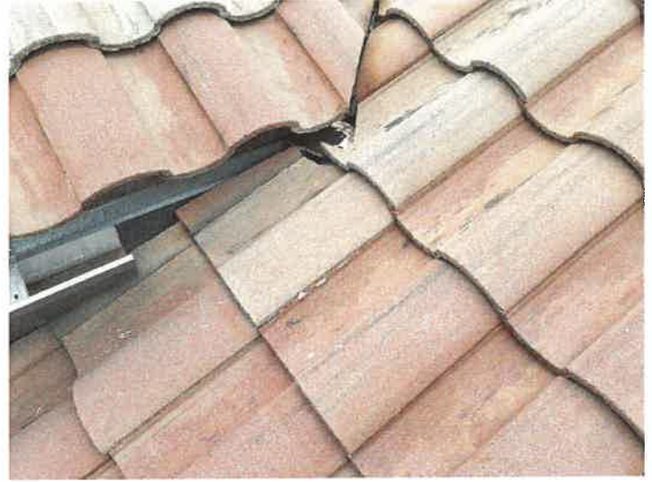
Building 15137: Repaired Displaced/Missing Roof Tile
