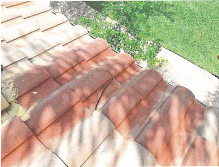
Building 15156: Identified Cracked Roof Tiles
