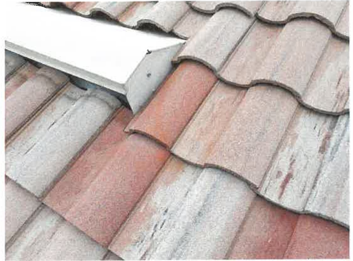
Building 15141: Repaired Displaced/Missing Roof Tile
