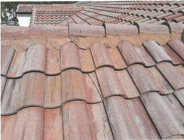
Building 15149: Identified Cracked Roof Tiles
