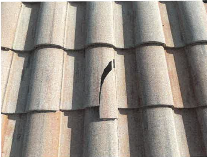
Building 15145: Identified Cracked Roof Tiles
