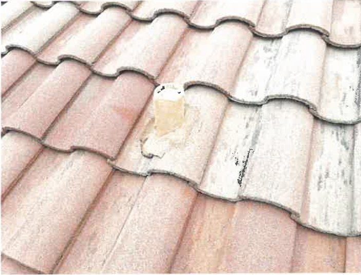
Building 15137: Lead Boots Lead boots appear to be in good condition.
