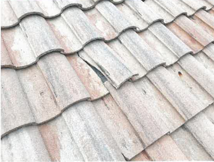
Building 15140: Identified Cracked Roof Tiles
