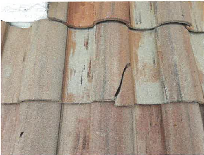
Building 15141: Identified Cracked Roof Tiles Cracked roof tiles can allow premature underlayment deterioration from excessive UV exposure.
