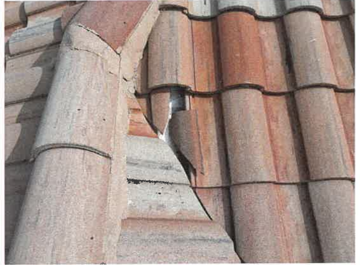
Building 15145: Broken Roof Tile
