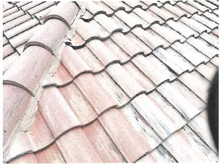
Building 15144: Repaired Displaced/Missing Roof Tile
