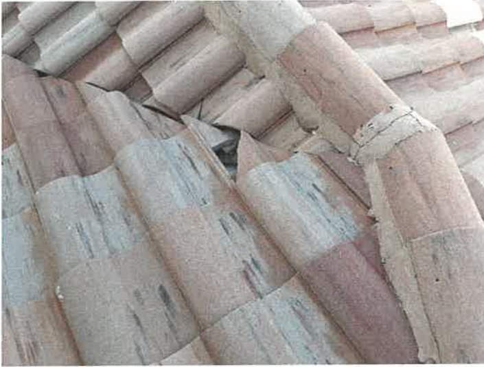
Building 15145: Broken Roof Tile
