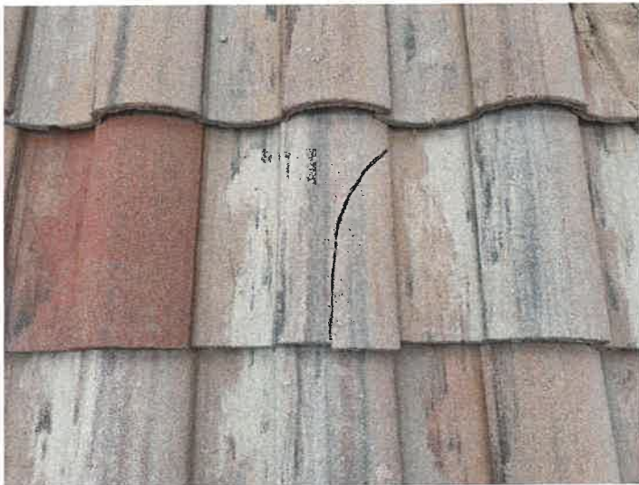
Building 15137: Identified Cracked Roof Tiles
