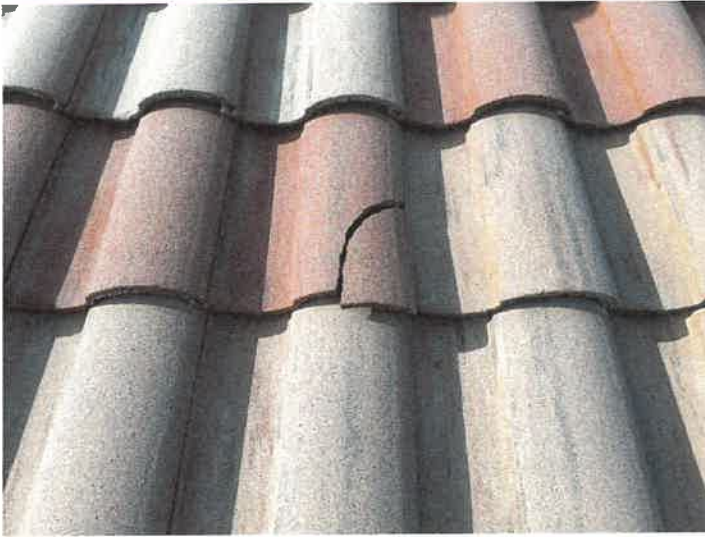
Building 15145: Identified Cracked Roof Tiles
