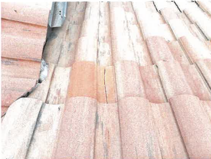
Building 15144: Identified Cracked Roof Tiles
