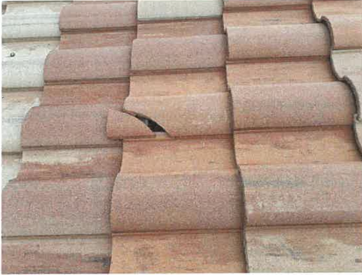
Building 15141: Identified Cracked Roof Tiles
