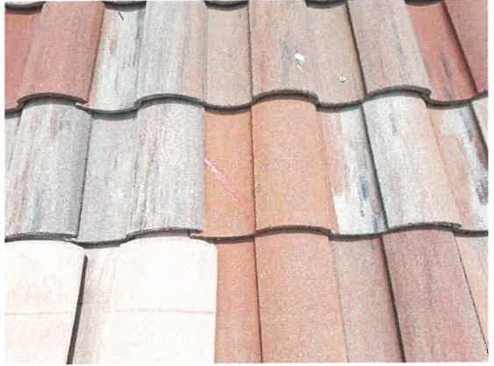
Building 15144: Repaired Cracked Roof Tiles
