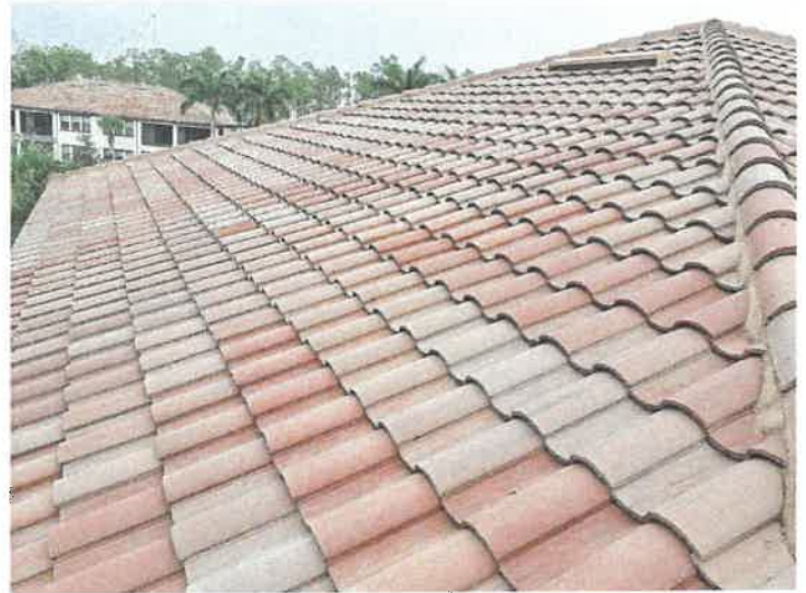
Building 15137: Surface Overview The roof surface appears to be in good, maintainable condition at this time.
