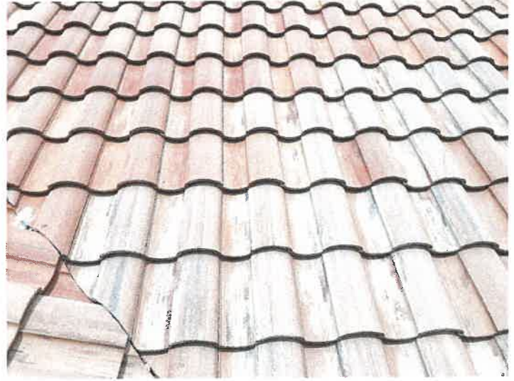
Building 15153: Repaired Cracked Roof Tiles
