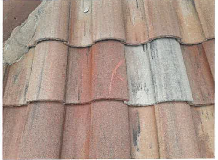
Building 15137: Repaired Cracked Roof Tiles
