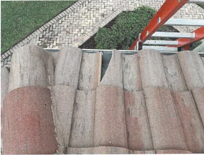
Building 15137: Identified Cracked Roof Tiles
