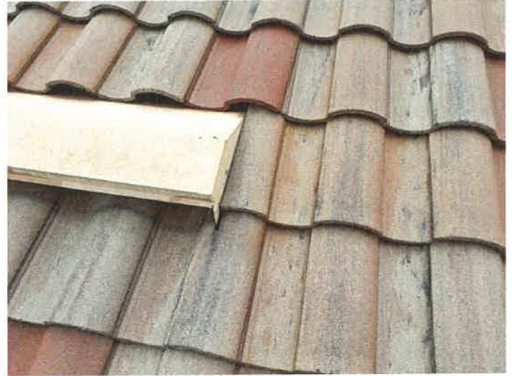
Building 15136: Repaired Displaced/Missing Roof Tile
