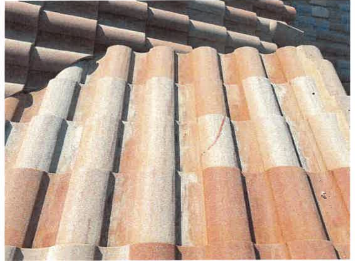
Building 15157: Repaired Cracked Roof Tiles
