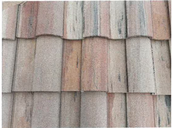
Building 15152: Repaired Displaced/Missing Roof Tile
