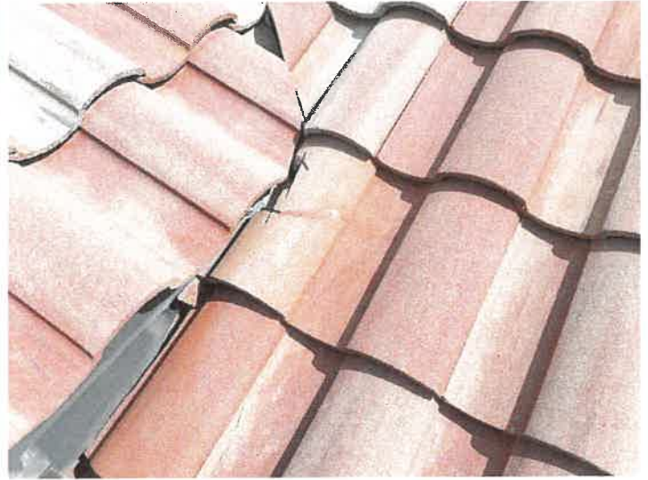
Building 15149: Repaired Cracked Roof Tiles
