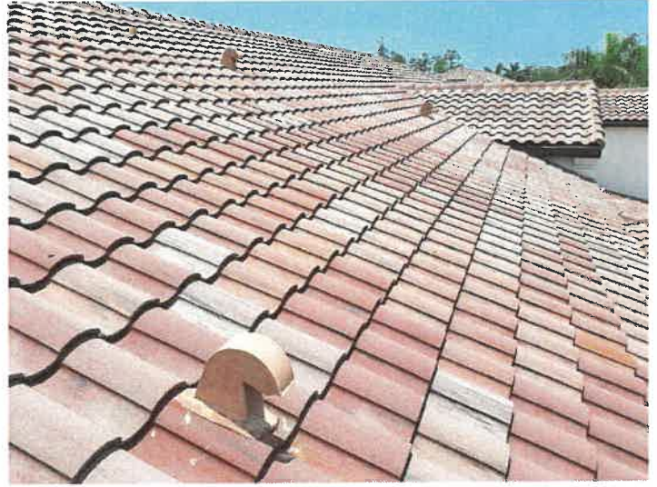
Building 15152: Roof Vents Roof vents appear to be in good condition.
