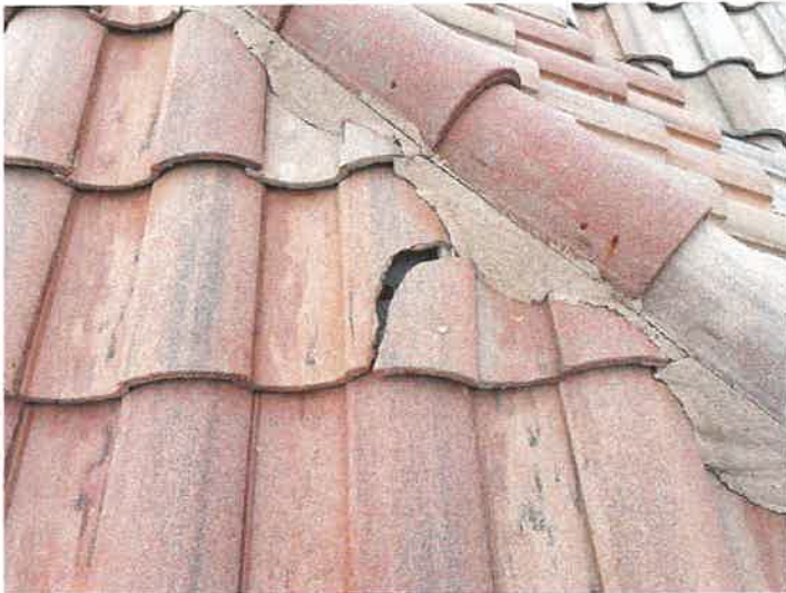
Building 15140: Identified Cracked Roof Tiles
