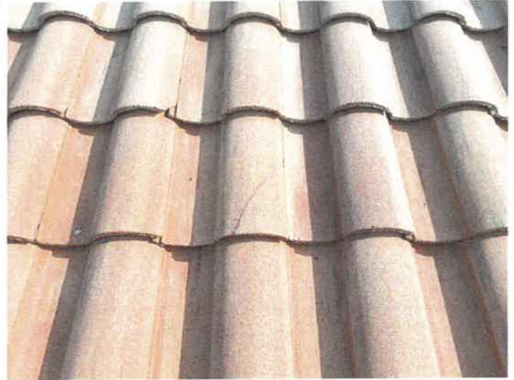
Building 15145: Repaired Cracked Roof Tiles
