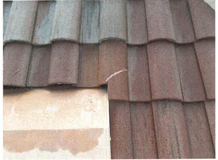
Building 15145: Repaired Cracked Roof Tiles
