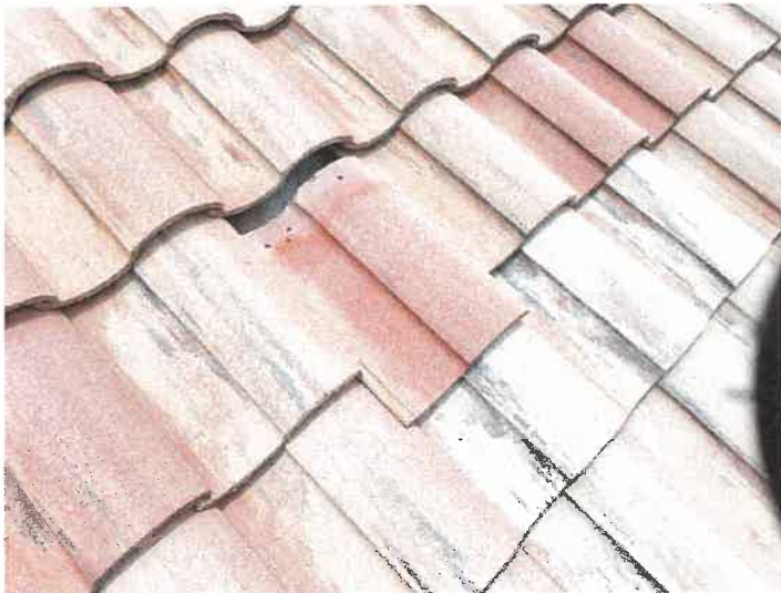
Building 15144: Displaced/Missing Roof Tile
