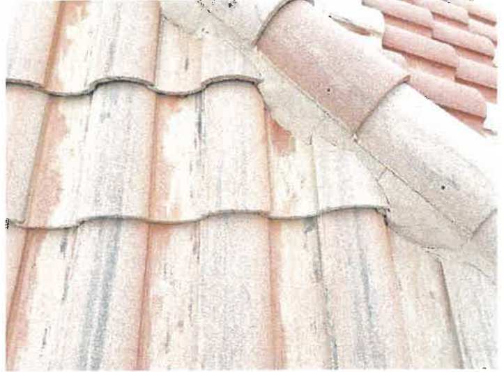
Building 15141: Repaired Cracked Roof Tiles
