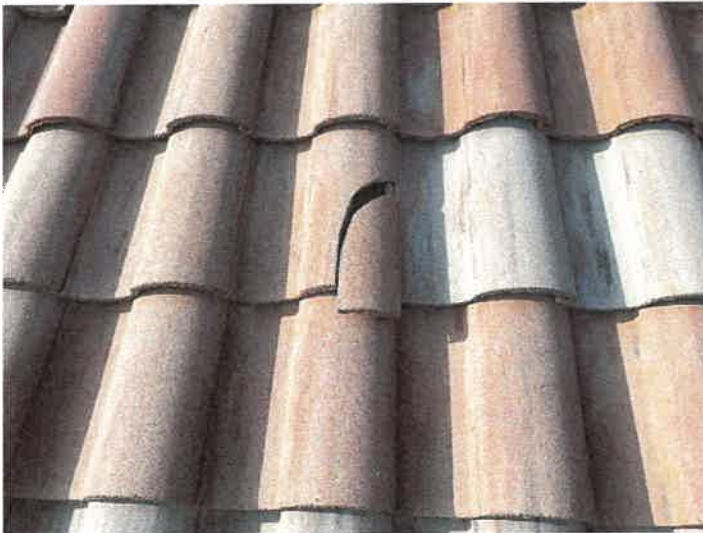
Building 15145: Identified Cracked Roof Tiles
