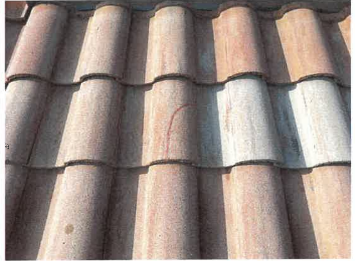
Building 15145: Repaired Cracked Roof Tiles
