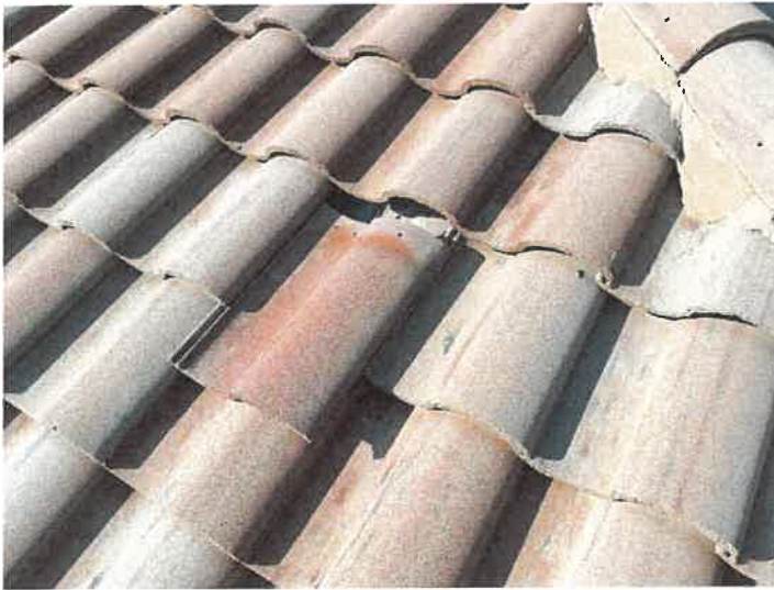
Building 15157: Displaced/Missing Roof Tile
