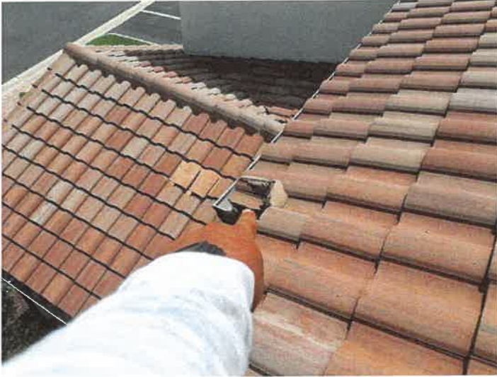
Building 15148: Broken Ridge Tile
