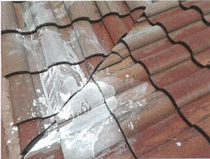
Building 15144: Identified Cracked Roof Tiles
