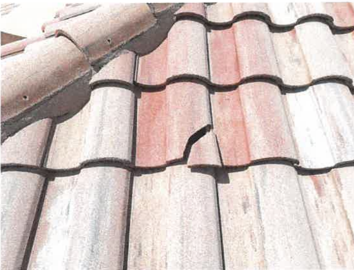
Building 15148: Identified Cracked Roof Tiles Cracked roof tiles can allow premature underlayment deterioration from excessive UV exposure.
