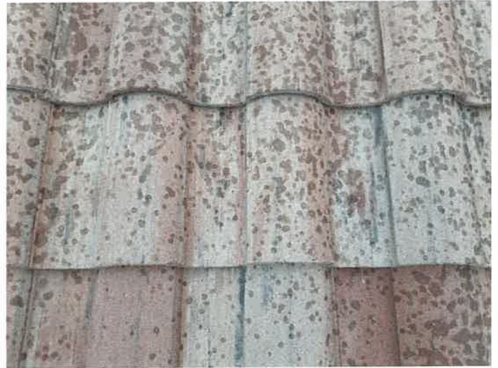
Building 15153: Repaired Cracked Roof Tiles
