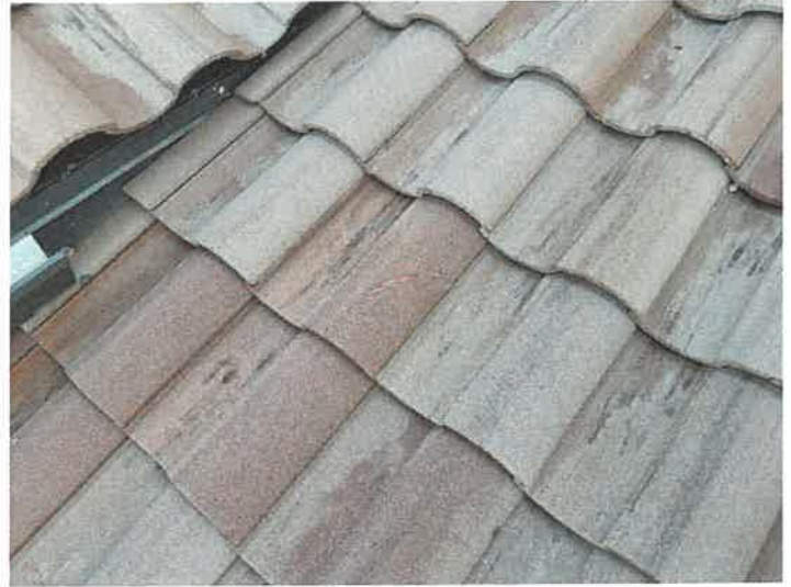
Building 15157: Repaired Cracked Roof Tiles The cracked roof tiles were repaired with Titebond sealant.
