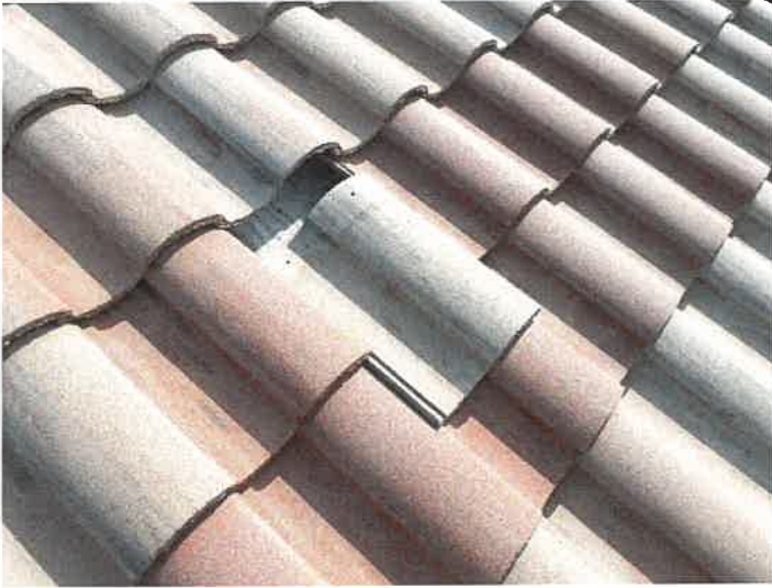
Building 15145: Displaced/Missing Roof Tile
