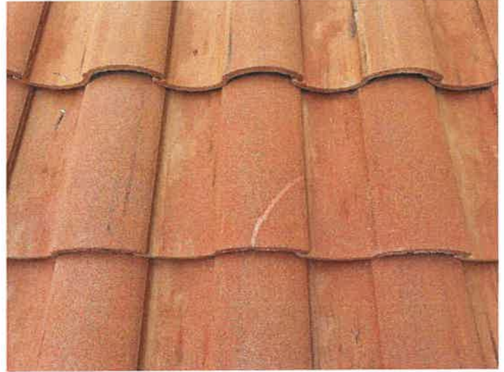
Building 15141: Repaired Cracked Roof Tiles
