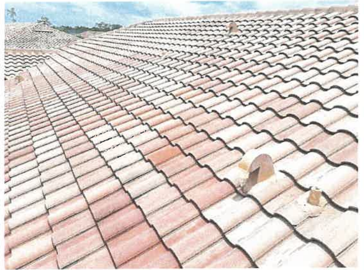
Building 15144: Roof Vents Roof vents appear to be in good condition.
