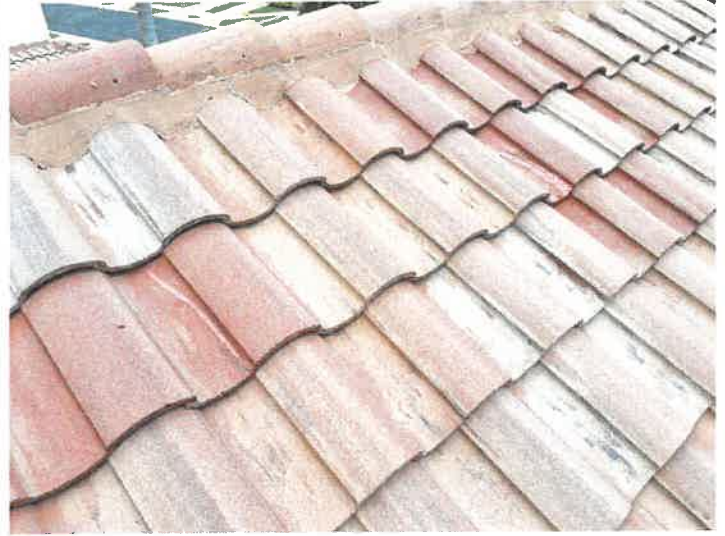
Building 15153: Repaired Cracked Roof Tiles
