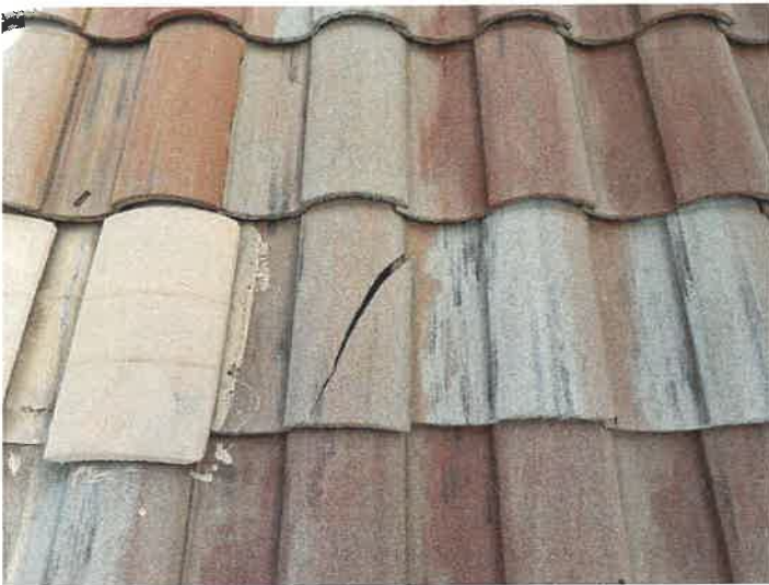
Building 15145: Identified Cracked Roof Tiles
