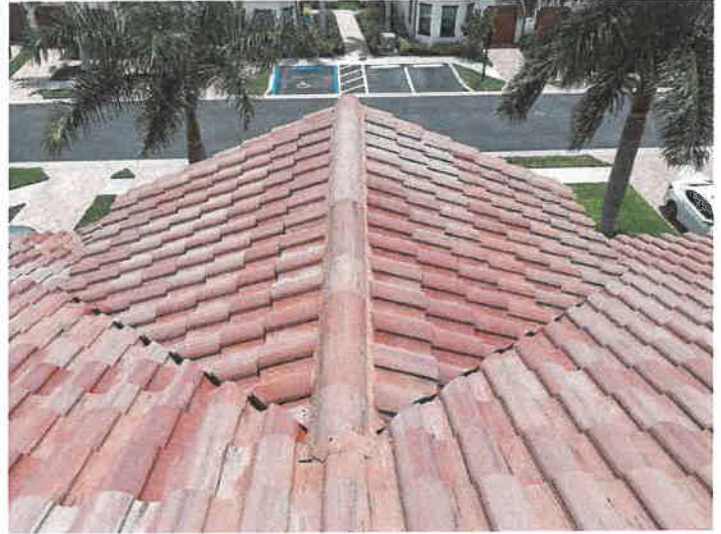
Building 15153: Valley The valley tiles appear to be in good condition.
