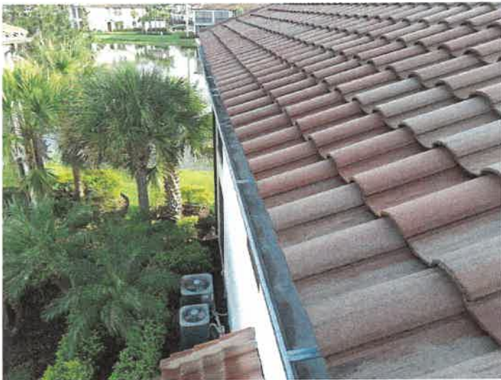
Building 15145: Gutters The gutters appear to be in good condition.
