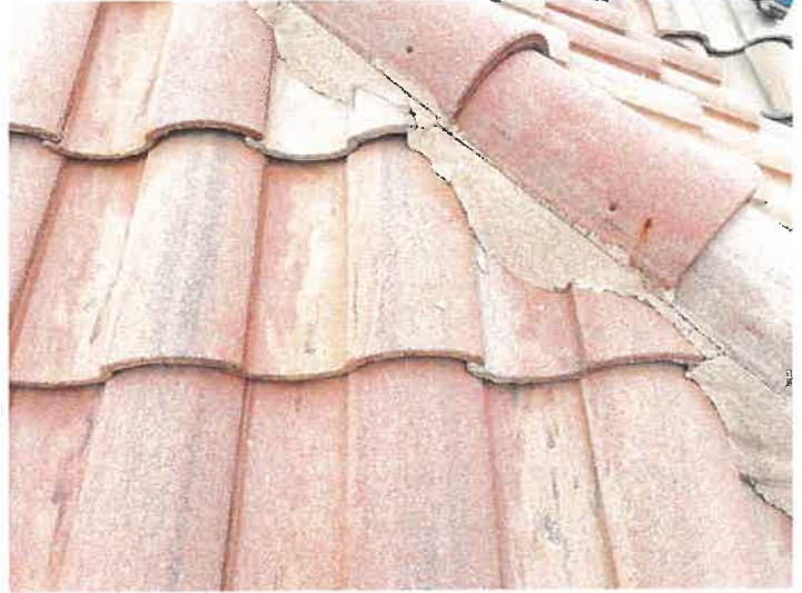
Building 15140: Repaired Cracked Roof Tiles
