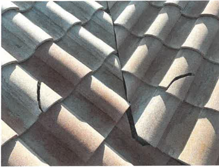
Building 15157: Identified Cracked Roof Tiles
