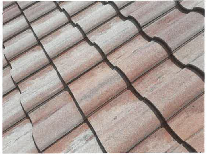
Building 15153: Repaired Displaced/Missing Roof Tile
