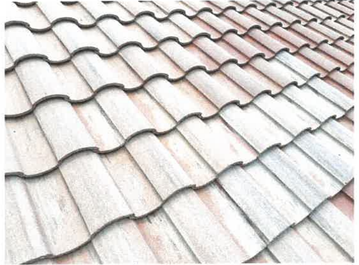
Building 15153: Repaired Cracked Roof Tiles
