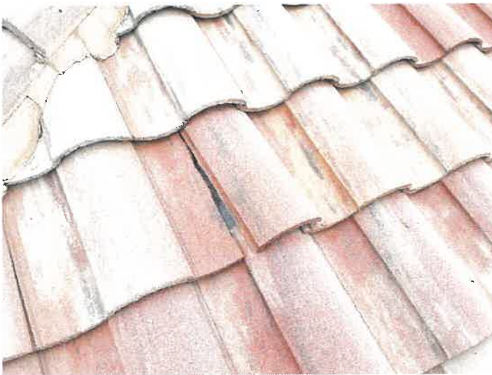
Building 15144: Identified Cracked Roof Tiles
