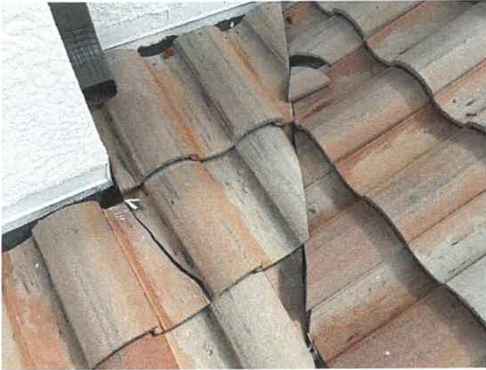
Building 15145: Identified Cracked Roof Tiles
