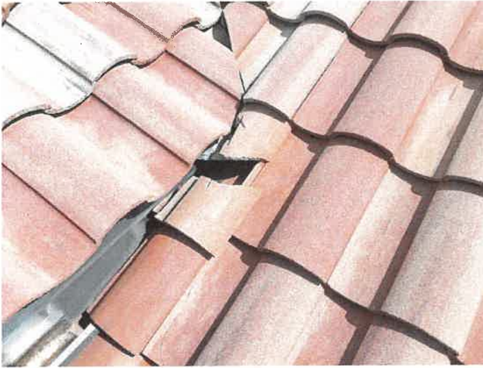
Building 15149: Identified Cracked Roof Tiles
