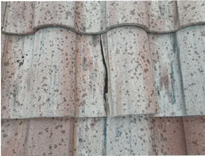
Building 15153: Identified Cracked Roof Tiles
