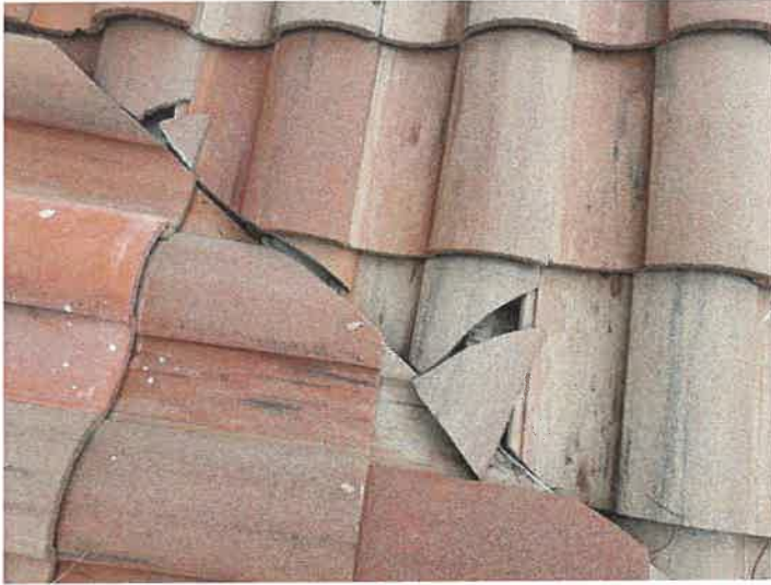
Building 15141: Identified Cracked Roof Tiles Cracked roof tiles can allow premature underlayment deterioration from excessive UV exposure.
