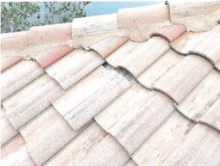
Building 15140: Displaced/Missing Roof Tile
