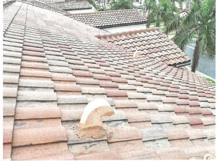
Building 15136: Roof Vents Roof vents appear to be in good condition.
