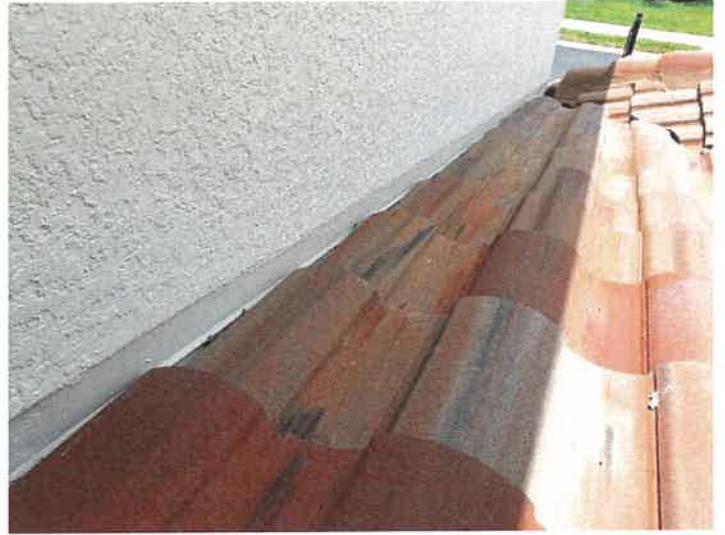
Building 15156: Counter Flashings
