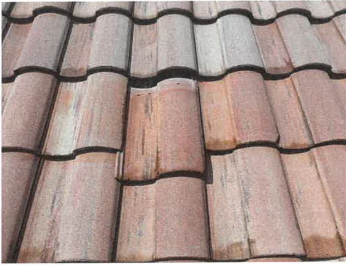
Building 15152: Displaced/Missing Roof Tile
