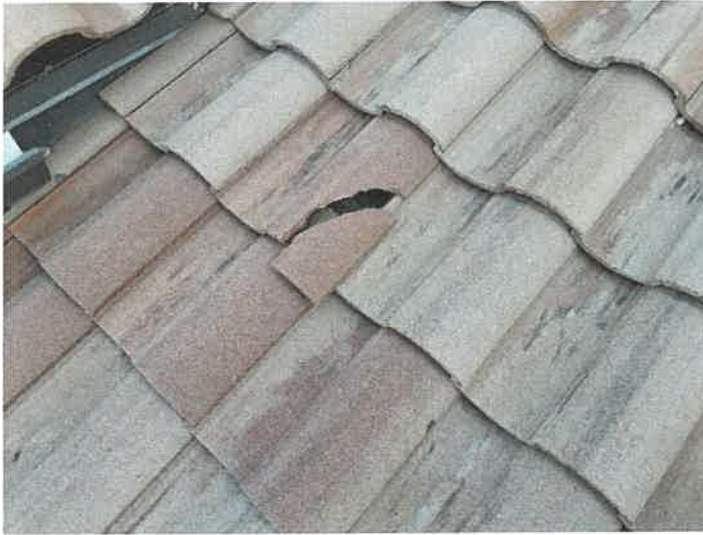
Building 15157: Identified Cracked Roof Tiles Cracked roof tiles can allow premature underlayment deterioration from excessive UV exposure.
