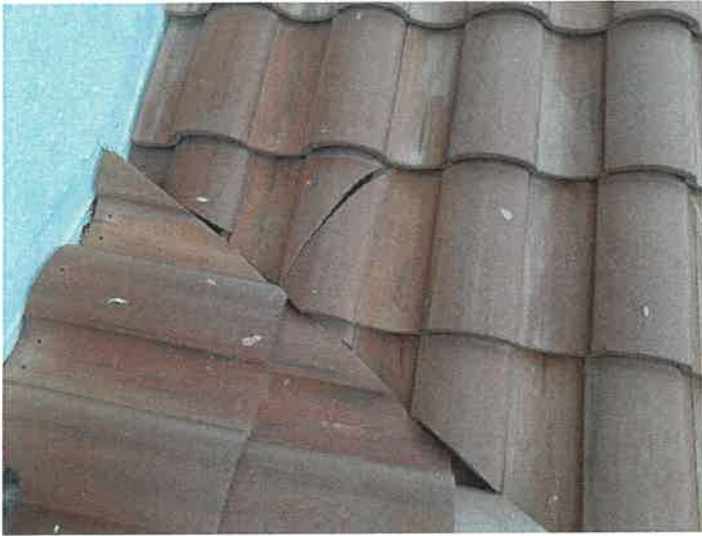
Building 15153: Identified Cracked Roof Tiles
