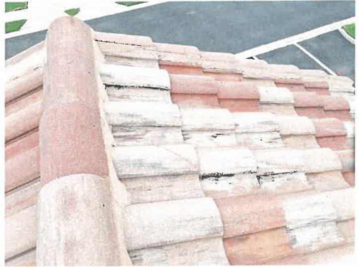
Building 15144: Repaired Cracked Roof Tiles
