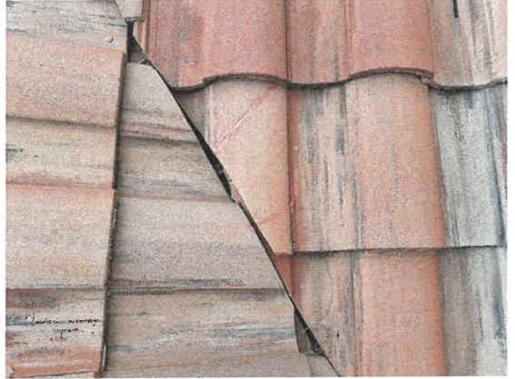
Building 15140: Repaired Cracked Roof Tiles
