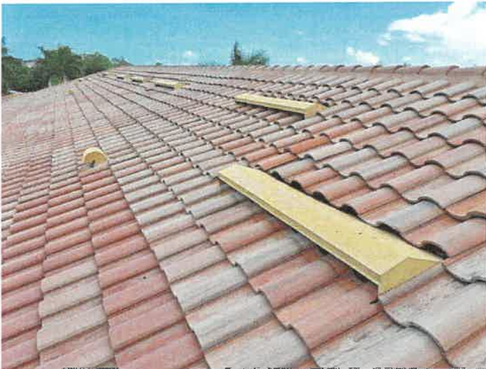
Building 15156: Identified Cracked Roof Tiles Cracked roof tiles can allow premature underlayment deterioration from excessive UV exposure.
