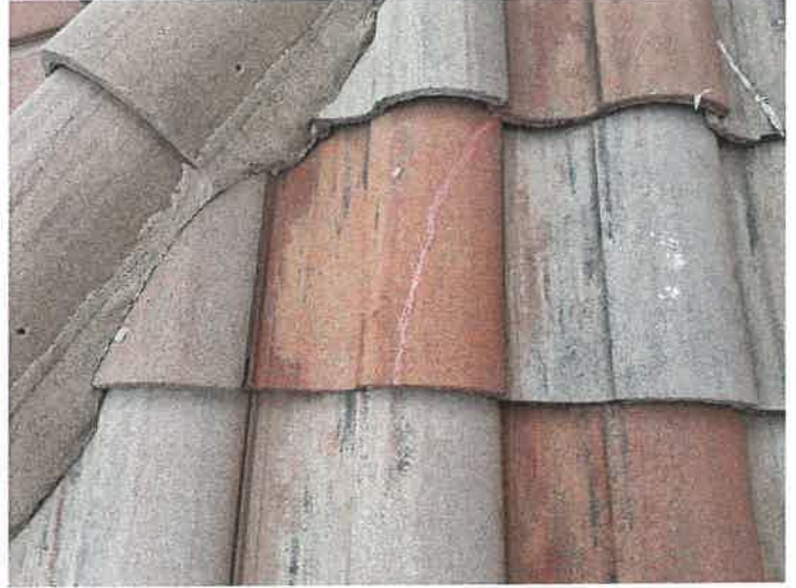
Building 15140: Repaired Cracked Roof Tiles
