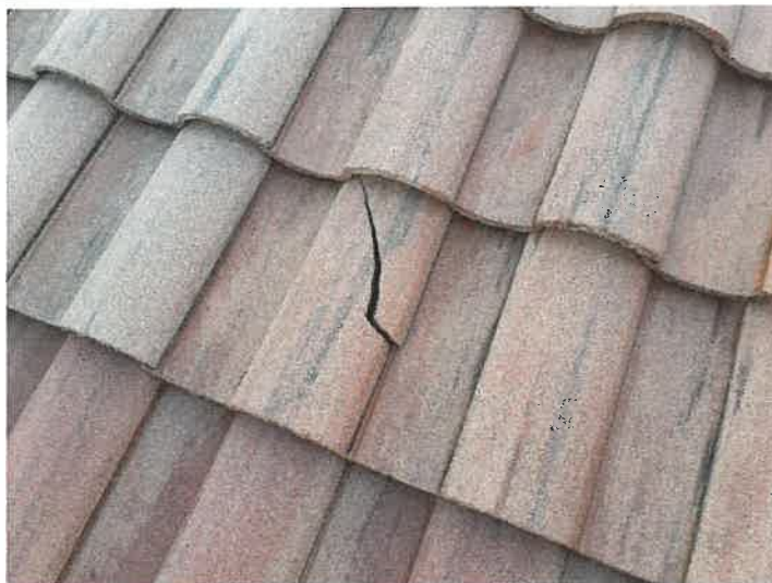
Building 15145: Identified Cracked Roof Tiles
