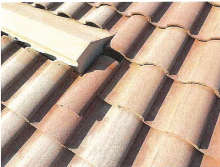
Displaced/Missing Roof Tile
