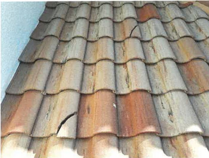
Building 15157: Identified Cracked Roof Tiles
