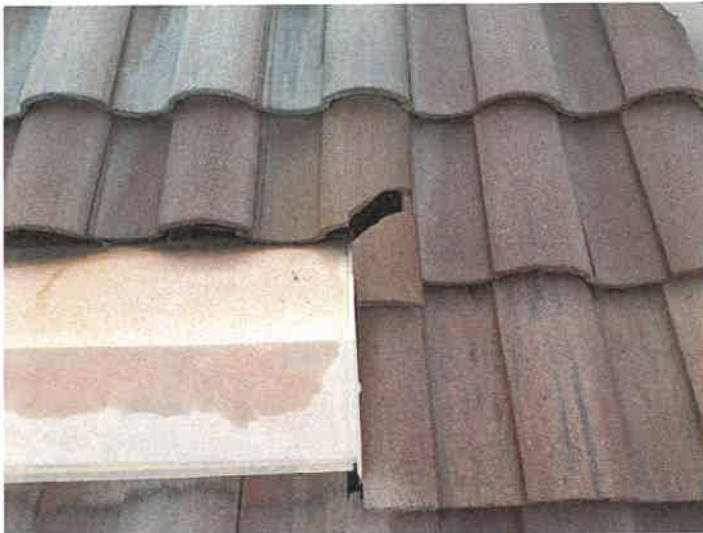
Building 15145: Identified Cracked Roof Tiles
