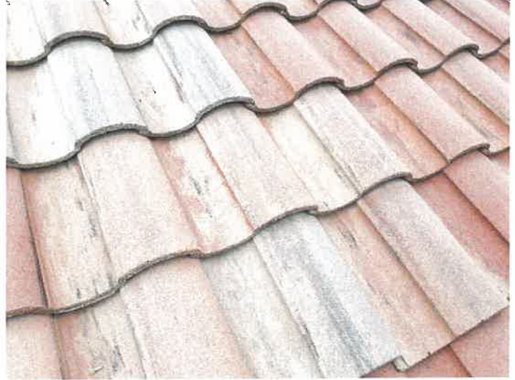
Building 15140: Repaired Cracked Roof Tiles
