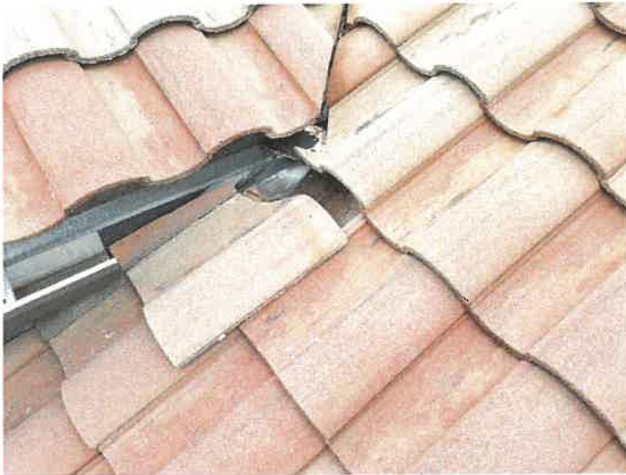
Building 15137: Displaced/Missing Roof Tile
