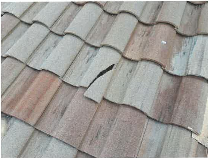
Building 15157: Identified Cracked Roof Tiles Cracked roof tiles can allow premature underlayment deterioration from excessive UV exposure.
