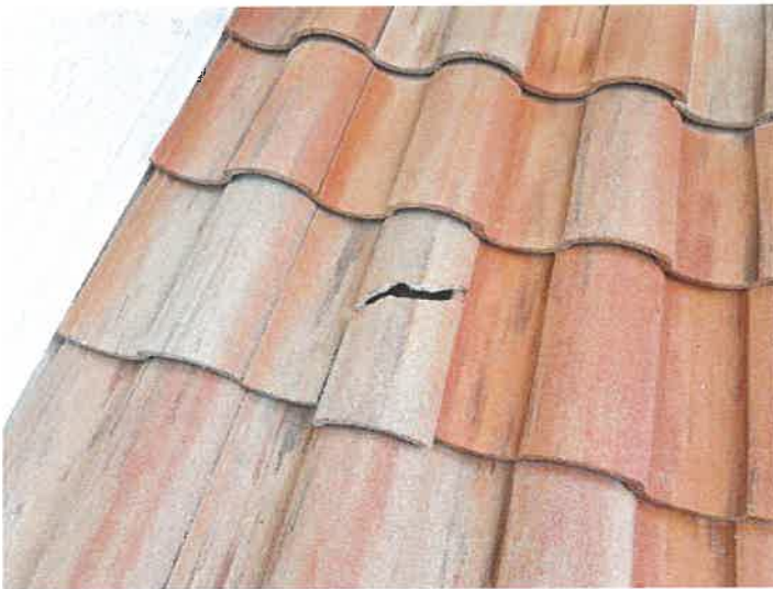
Building 15149: Identified Cracked Roof Tiles
