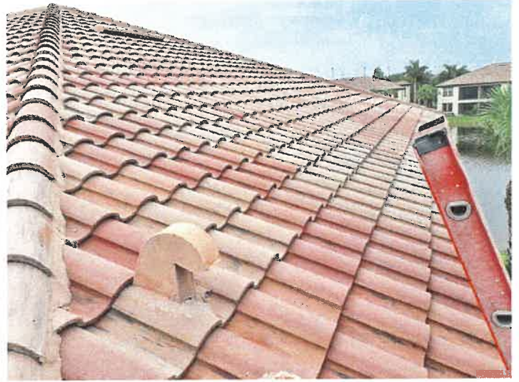
Building 15140: Surface Overview The roof surface appears to be in good, maintainable condition at this time.
