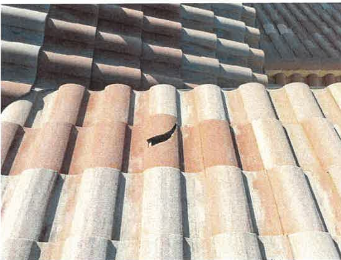
Building 15157: Identified Cracked Roof Tiles
