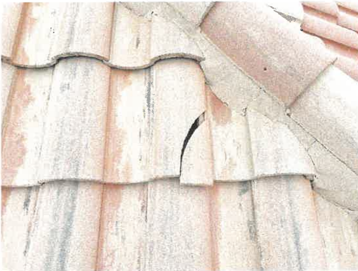
Building 15141: Identified Cracked Roof Tiles
