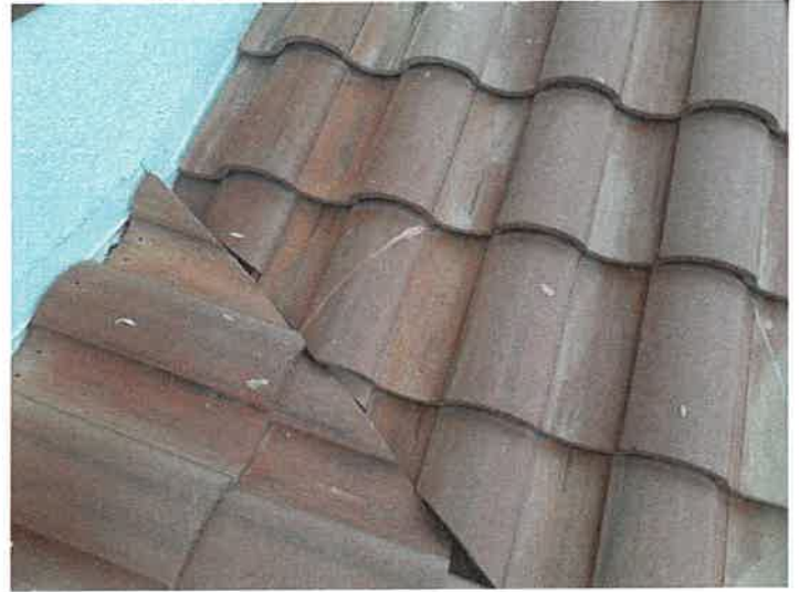
Building 15153: Repaired Cracked Roof Tiles
