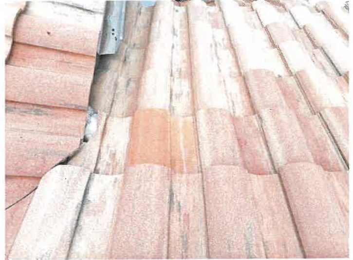
Building 15144: Repaired Cracked Roof Tiles
