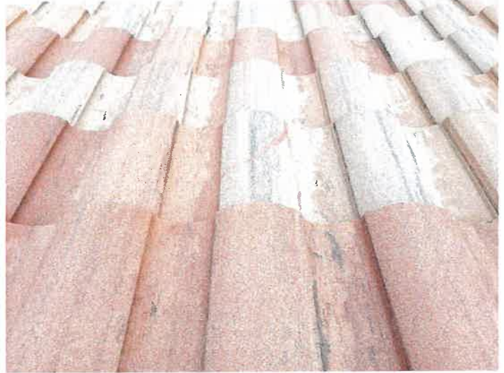
Building 15140: Repaired Cracked Roof Tiles
