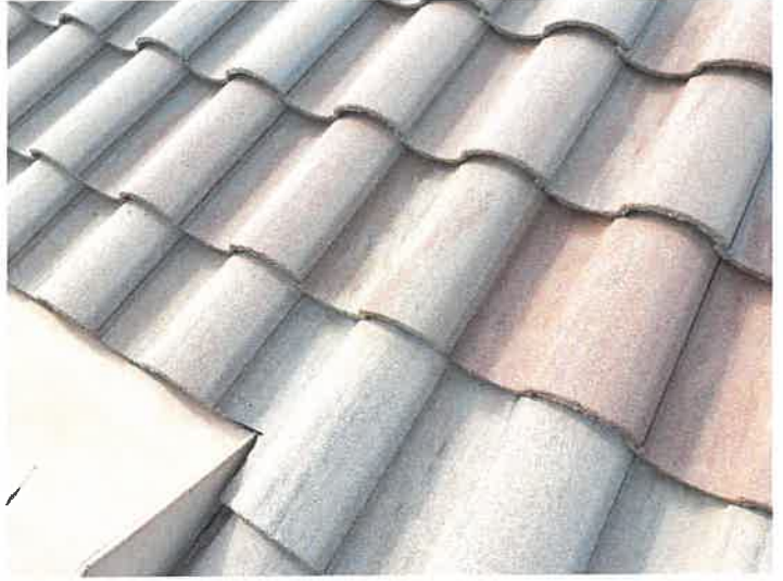
Building 15145: Repaired Displaced/Missing Roof Tile
