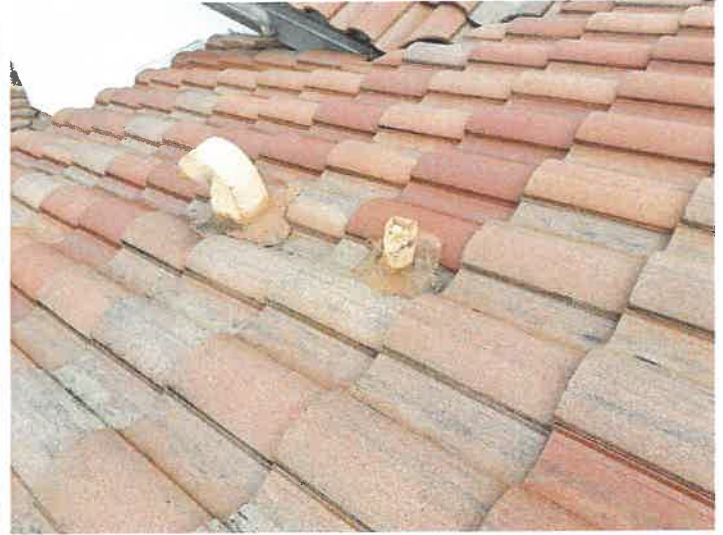
Building 15136: Lead Boots Lead boots appear to be in good condition.
