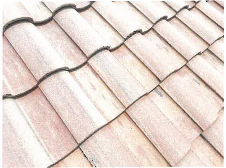
Building 15153: Repaired Cracked Roof Tiles
