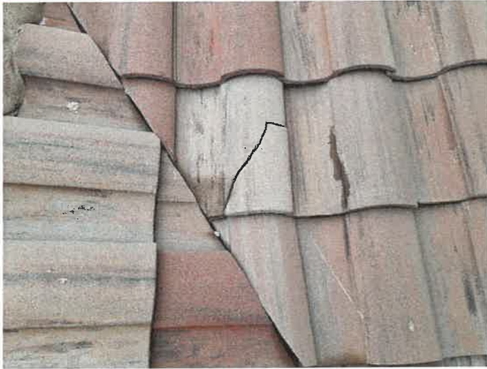
Building 15137: Identified Cracked Roof Tiles
