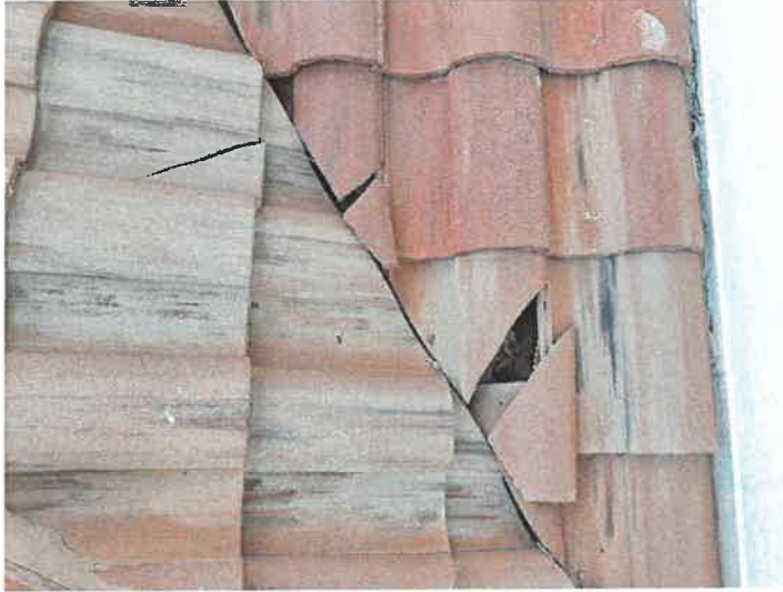
Building 15145: Identified Cracked Roof Tiles Cracked roof tiles can allow premature underlayment deterioration from excessive UV exposure.
