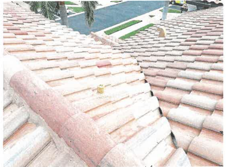
Building 15156: Lead Boots Lead boots appear to be in good condition.
