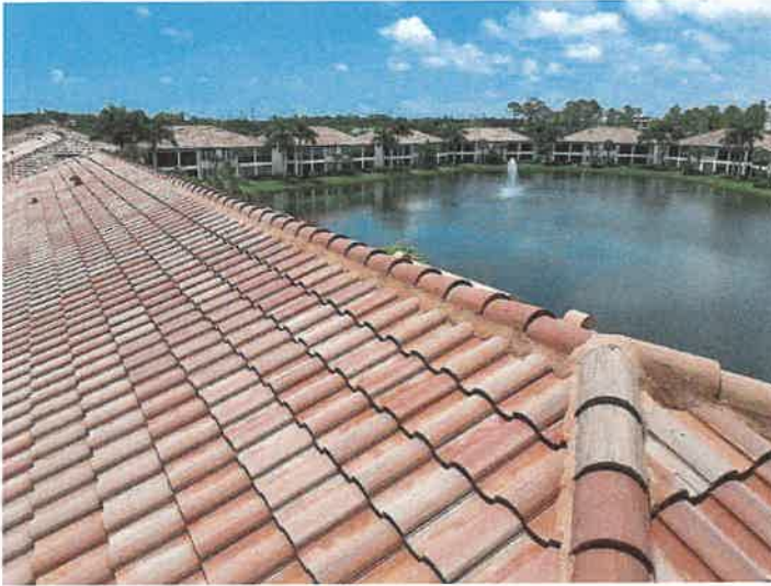
Building 15153: Ridge Tiles Ridge tiles appear to be in good condition.
