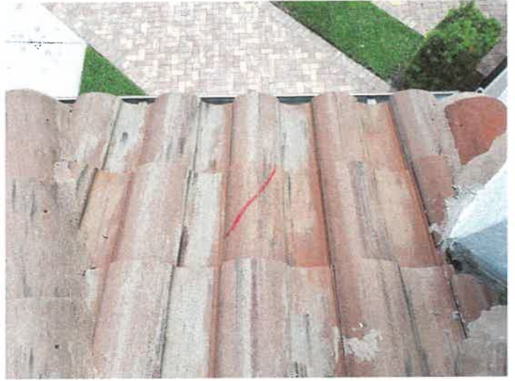
Building 15148: Repaired Cracked Roof Tiles
