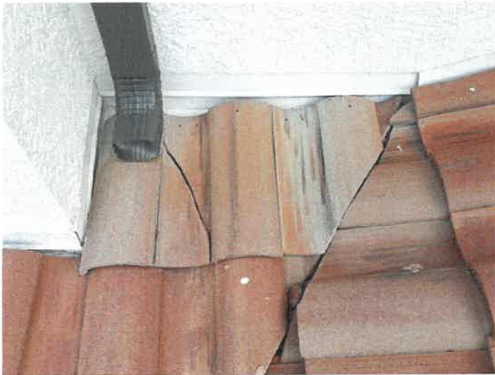
Building 15149: Identified Cracked Roof Tiles
