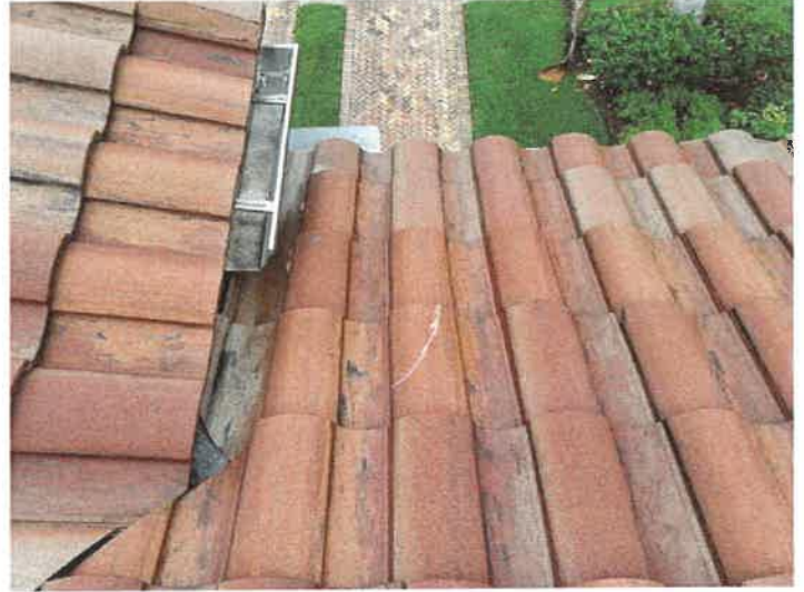
Building 15136: Repaired Cracked Roof Tiles
