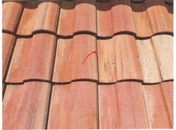
Building 15148: Repaired Cracked Roof Tiles
