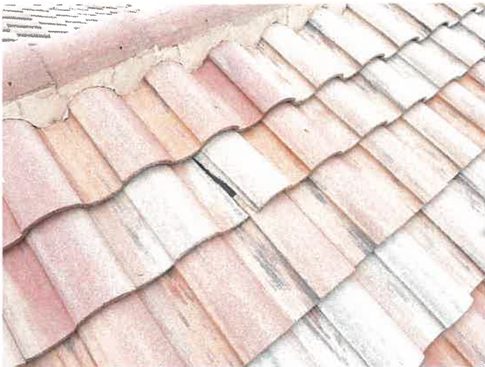
Building 15144: Identified Cracked Roof Tiles
