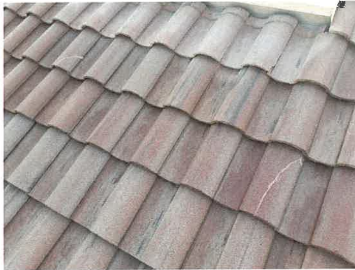
Building 15145: Repaired Cracked Roof Tiles
