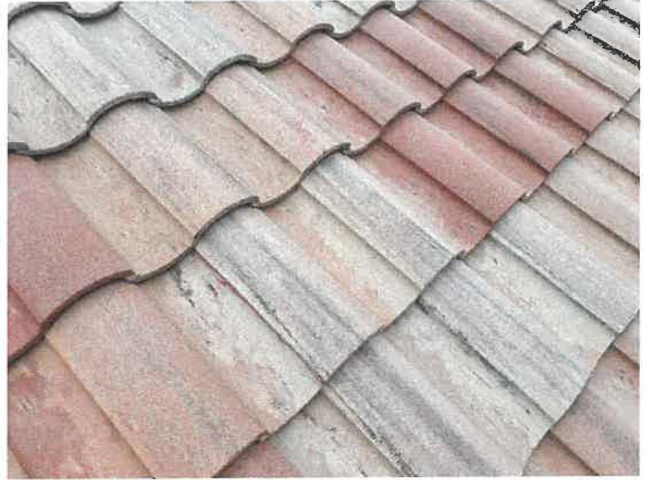
Building 15140: Repaired Cracked Roof Tiles
