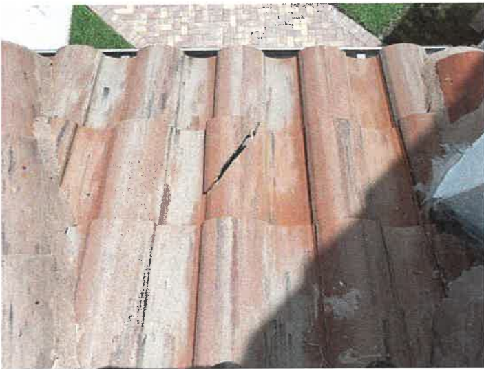
Building 15148: Identified Cracked Roof Tiles
