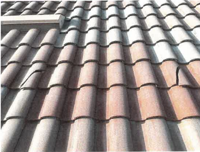
Building 15145: Identified Cracked Roof Tiles
