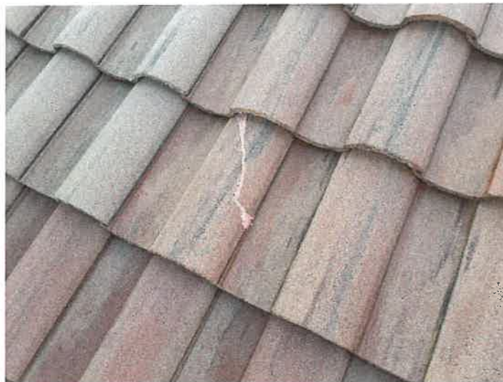
Building 15145: Repaired Cracked Roof Tiles
