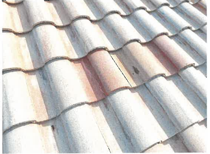
Building 15145: Repaired Cracked Roof Tiles
