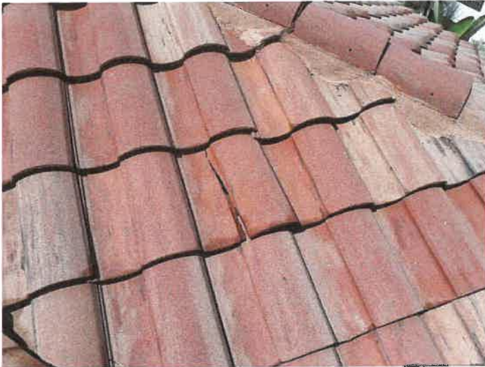
Building 15152: Identified Cracked Roof Tiles
