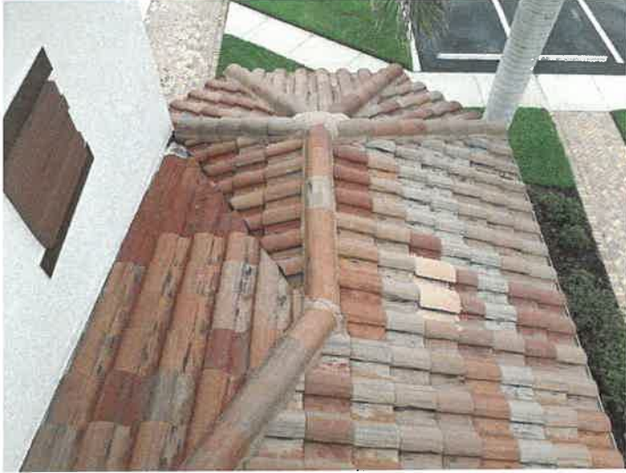
Building 15141: Surface Overview - Lower Roof The roof surface appears to be in good, maintainable condition at this time.
