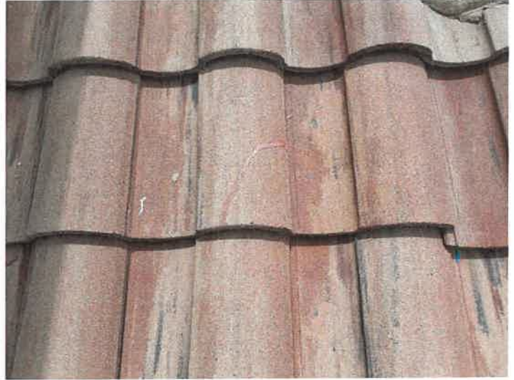
Building 15144: Repaired Cracked Roof Tiles
