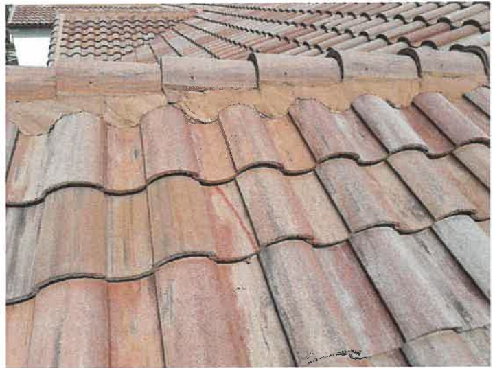
Building 15149: Repaired Cracked Roof Tiles
