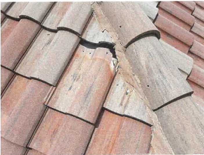
Building 15153: Displaced/Missing Roof Tile
