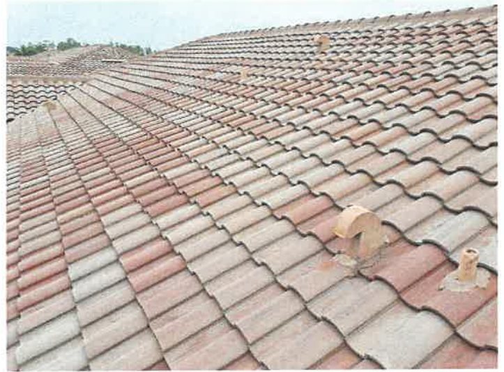
Building 15137: Roof Vents
