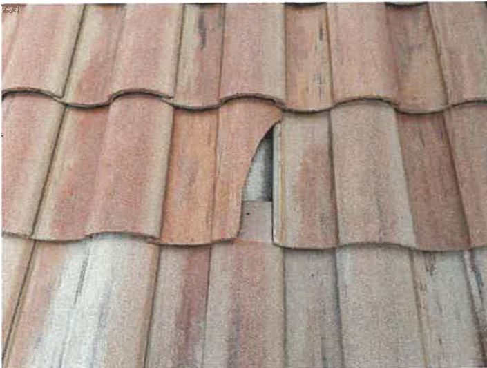
Building 15145: Broken Roof Tile
