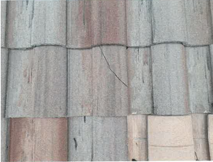
Building 15136: Identified Cracked Roof Tiles
