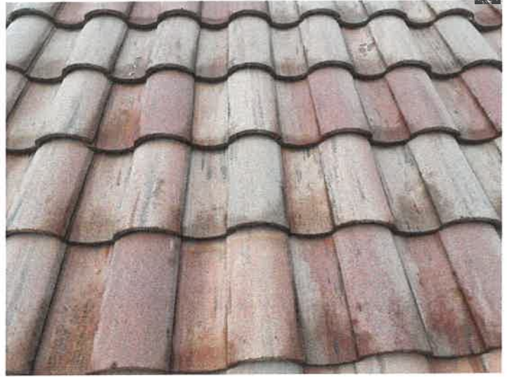
Building 15152: Repaired Displaced/Missing Roof Tile
