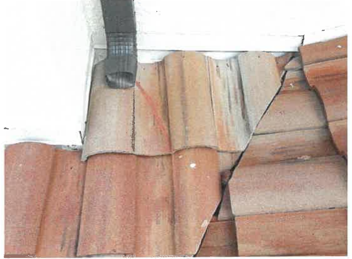
Building 15149: Repaired Cracked Roof Tiles
