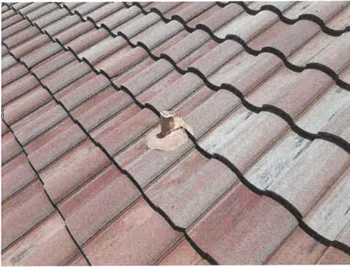
Building 15152: Lead Boots Lead boots appear to be in good condition.
