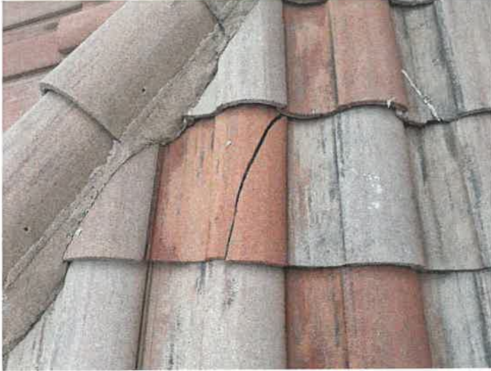
Building 15140: Identified Cracked Roof Tiles
