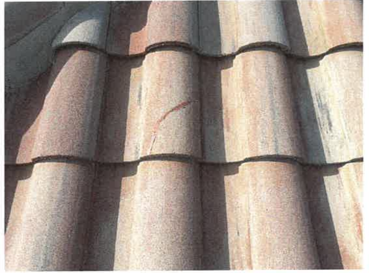
Building 15145: Repaired Cracked Roof Tiles
