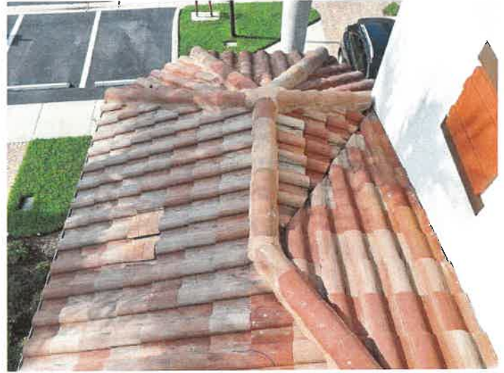
Building 15145: Surface Overview - Lower Roof The roof surface appears to be in good, maintainable condition at this time.
