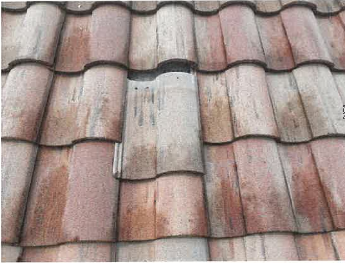
Building 15152: Displaced/Missing Roof Tile
