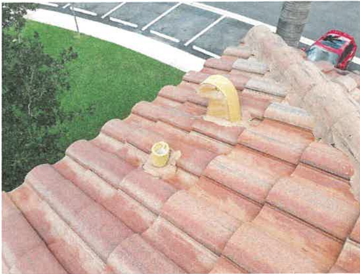
Building 15156: Lead Boots Lead boots appear to be in good condition.
