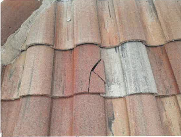
Building 15137: Identified Cracked Roof Tiles
