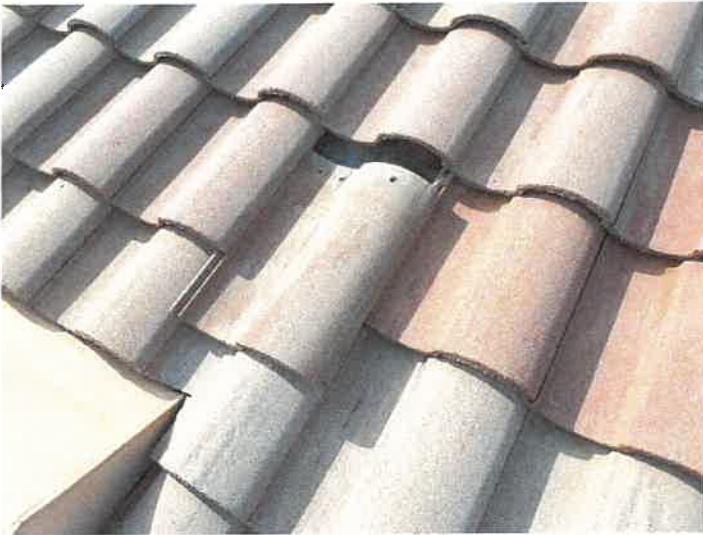
Building 15145: Displaced/Missing Roof Tile
