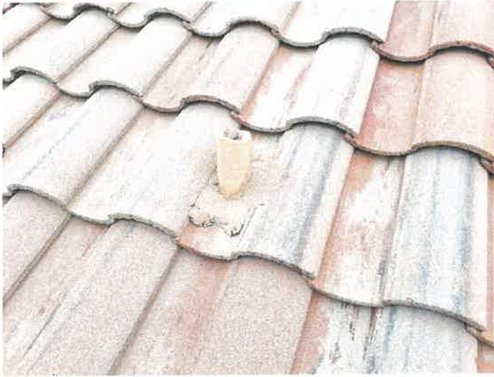
Building 15141: Lead Boots Lead boots appear to be in good condition.
