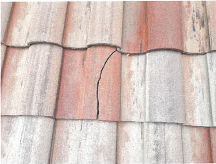
Building 15140: Identified Cracked Roof Tiles
