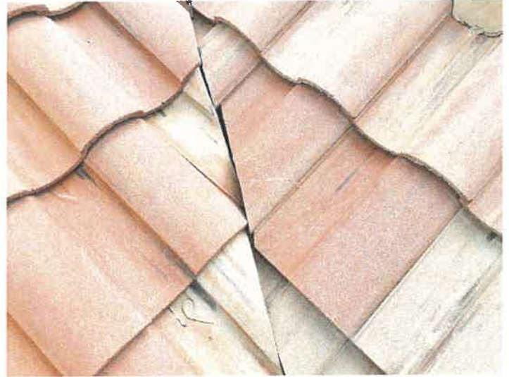
Building 15149: Repaired Cracked Roof Tiles
