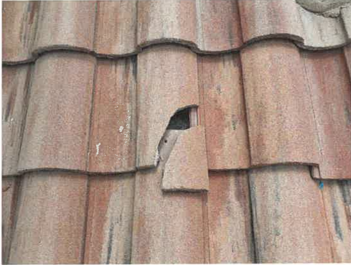
Building 15144: Identified Cracked Roof Tiles
