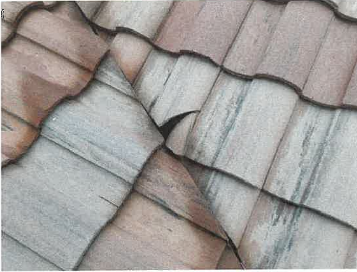
Building 15136: Identified Cracked Roof Tiles
