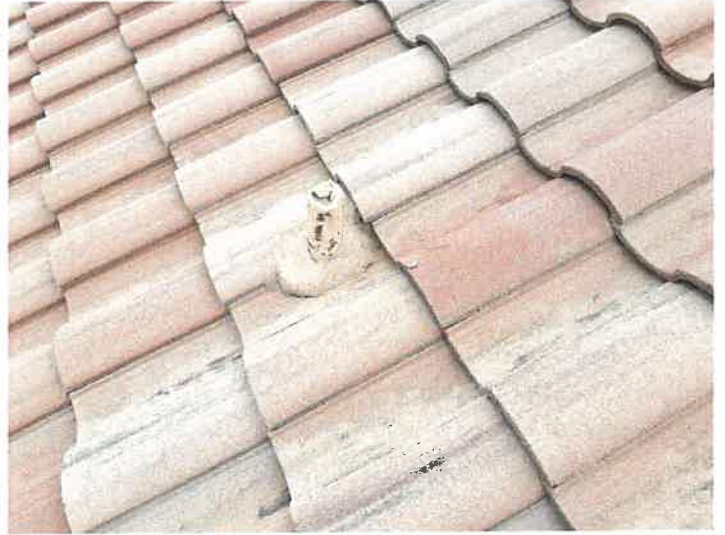
Building 15137: Lead Boots Lead boots appear to be in good condition.
