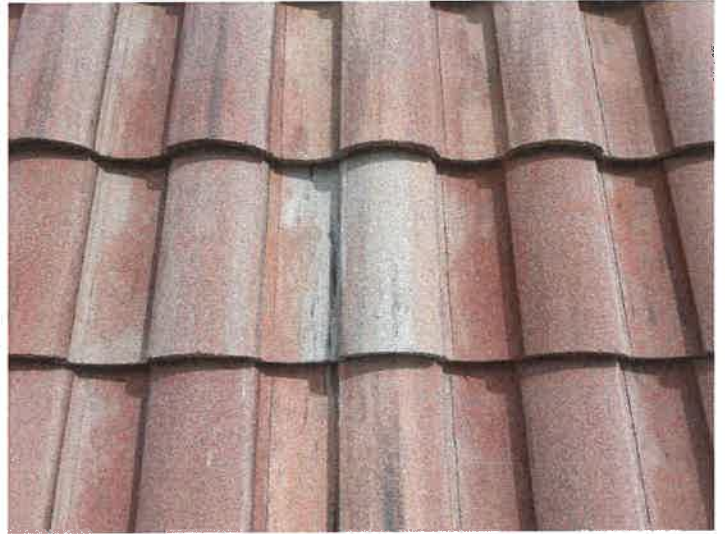
Building 15152: Repaired Displaced/Missing Roof Tile
