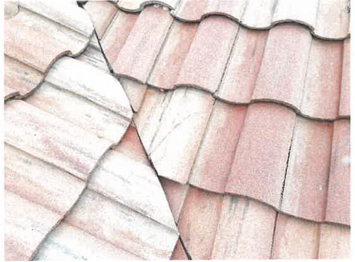
Building 15144: Repaired Cracked Roof Tiles
