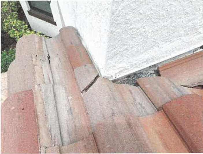
Building 15144: Identified Cracked Roof Tiles
