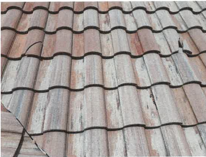
Building 15153: Identified Cracked Roof Tiles
