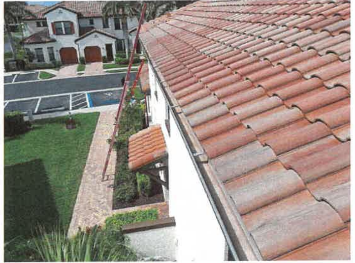
Building 15149: Gutters The gutters appear to be in good condition.
