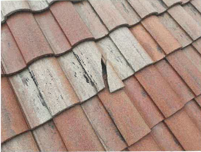
Building 15136: Identified Cracked Roof Tiles
