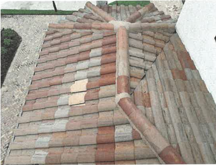
Building 15141: Appearance Overview - Lower Roof The roof appearance is in good, maintainable condition.
