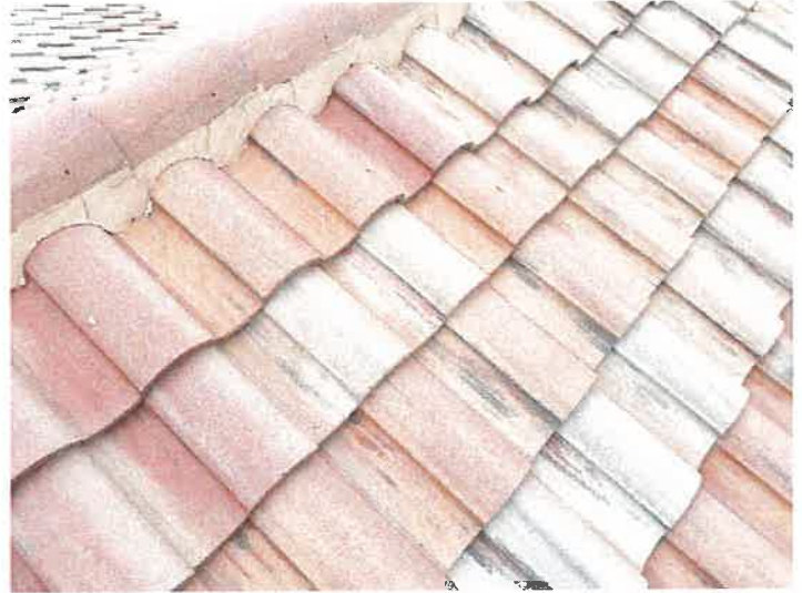
Building 15144: Repaired Cracked Roof Tiles
