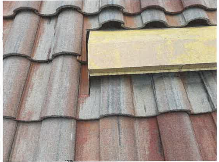
Building 15156: Repaired Cracked Roof Tiles The cracked roof tiles were repaired with Titebond sealant.
