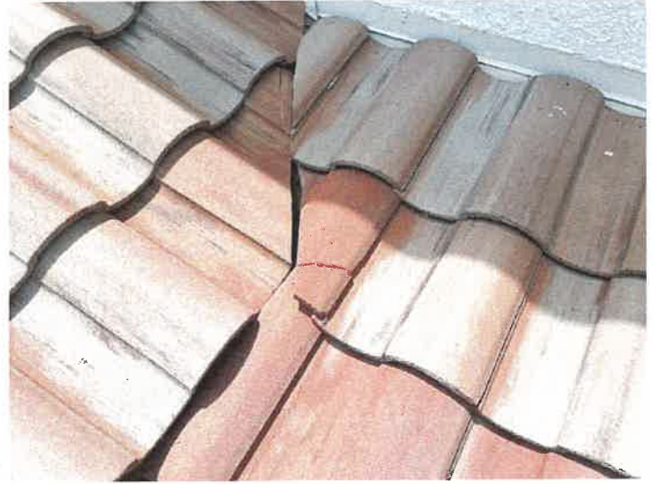
Building 15148: Repaired Cracked Roof Tiles
