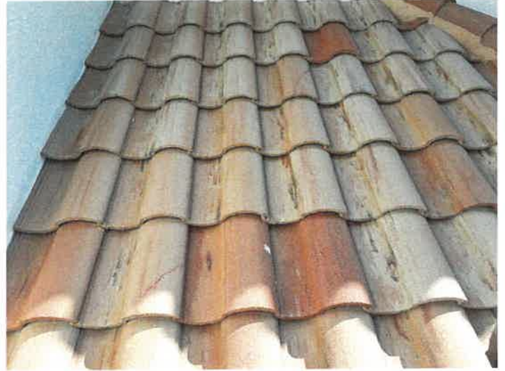
Building 15157: Repaired Cracked Roof Tiles
