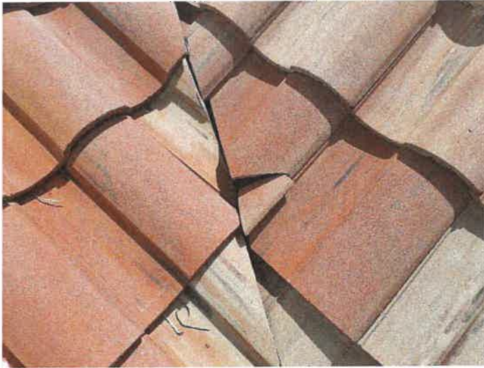
Building 15149: Identified Cracked Roof Tiles
