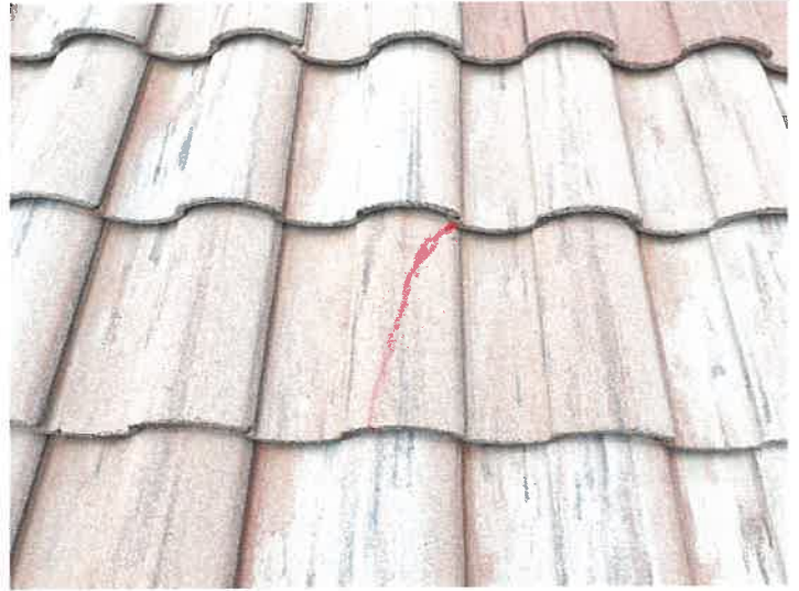
Building 15148: Repaired Cracked Roof Tiles
