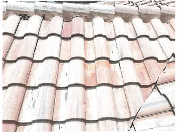
Repaired Cracked Roof Tiles
