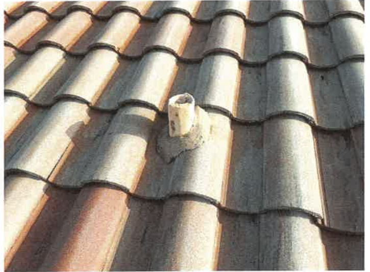
Building 15145: Lead Boots Lead boots appear to be in good condition.
