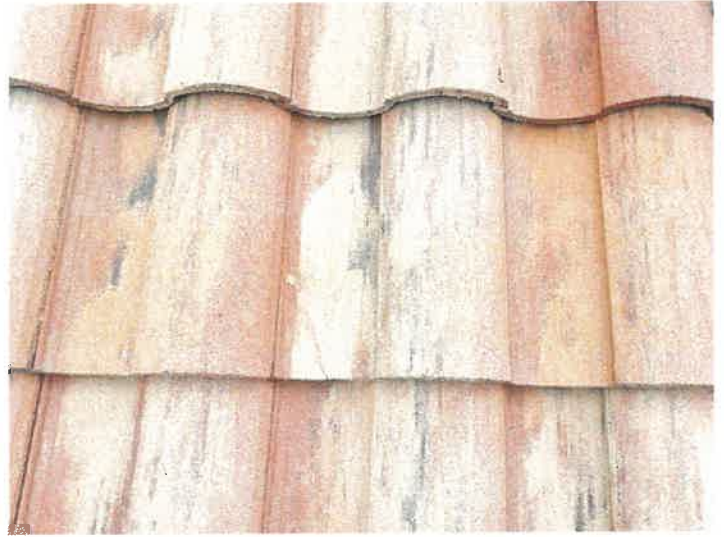
Building 15102: Repaired Cracked Roof Tiles
