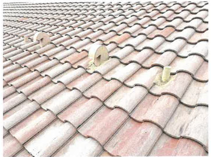
Building 15102: Lead Boots Lead boots appear to be in good condition.
