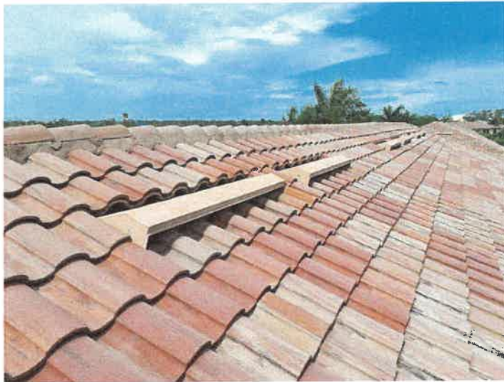
Building 15122: Identified Cracked Roof Tiles Cracked roof tiles can allow premature underlayment deterioration from excessive UV exposure.
