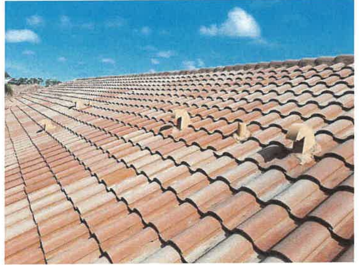
Building 15114: Roof Vents Roof vents appear to be in good condition.
