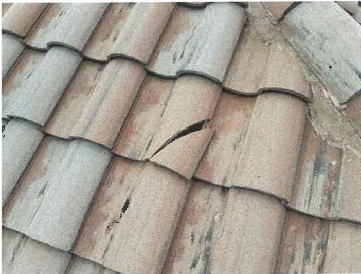
Building 15114: Identified Cracked Roof Tiles
