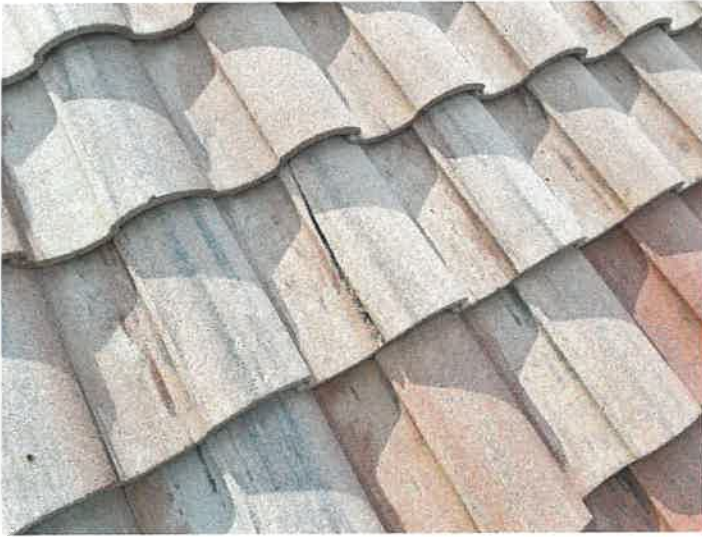
Building 15098: Identified Cracked Roof Tiles
