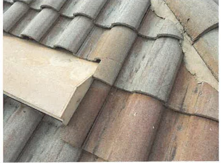
Building 15126: Repaired Cracked Roof Tiles
