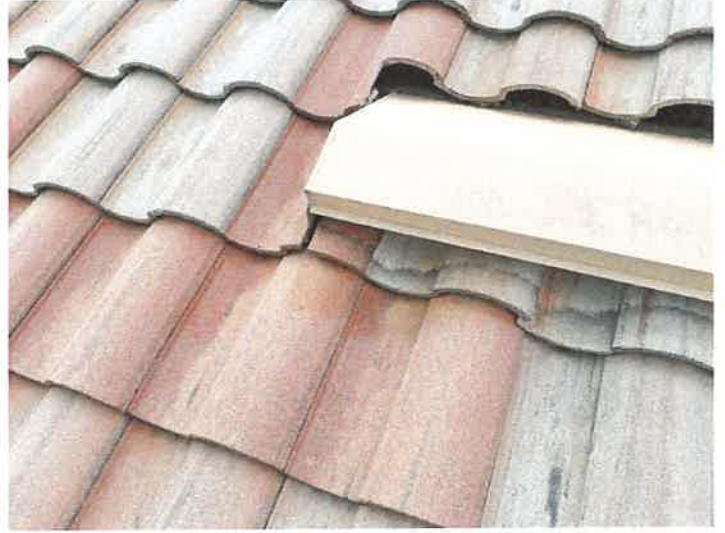
Building 15106: Repaired Displaced/Missing Roof Tile
