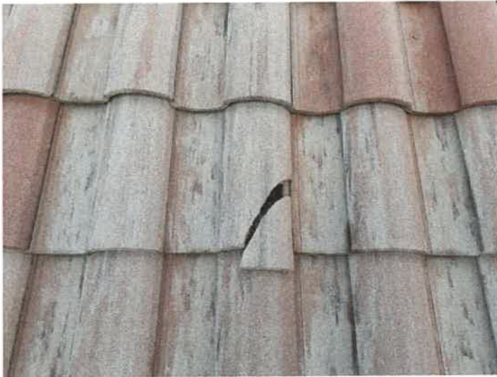
Building 15126: Identified Cracked Roof Tiles Cracked roof tiles can allow premature underlayment deterioration from excessive UV exposure.
