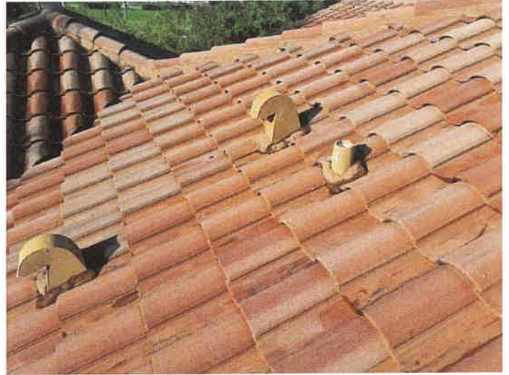
Building 15110: Lead Boots Lead boots appear to be in good condition.
