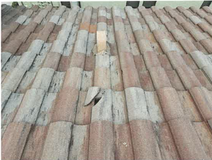
Building 15114: Identified Cracked Roof Tiles
