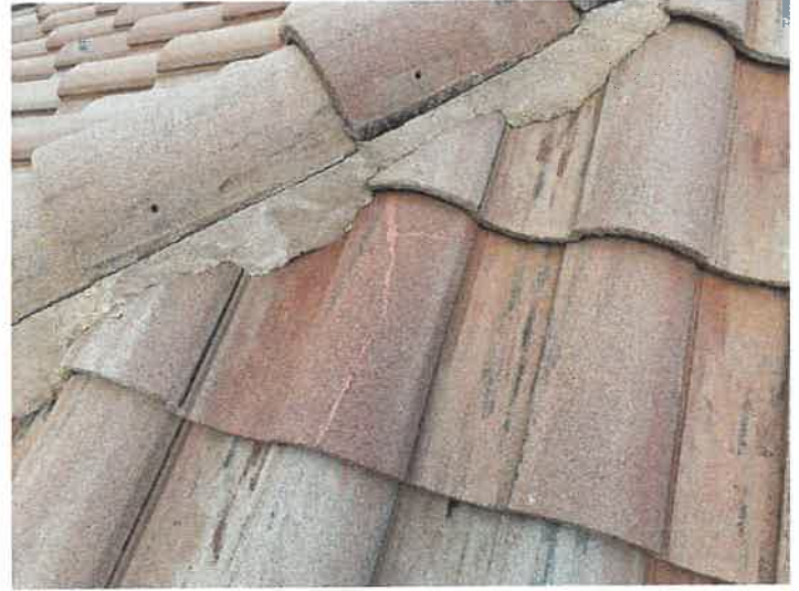
Building 15114: Repaired Cracked Roof Tiles
