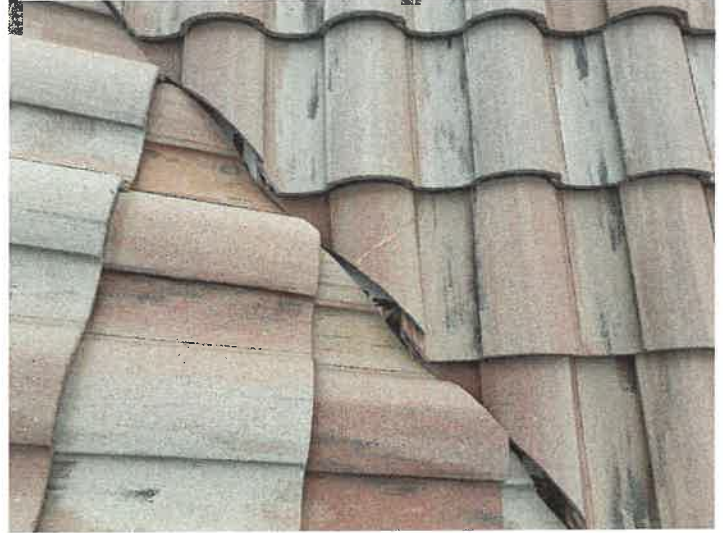
Building 15114: Repaired Cracked Roof Tiles
