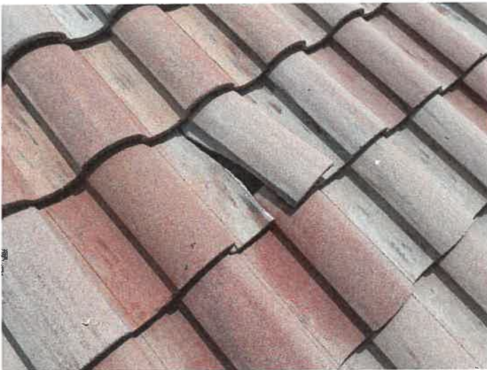
Building 15122: Identified Cracked Roof Tiles Cracked roof tiles can allow premature underlayment deterioration from excessive UV exposure.
