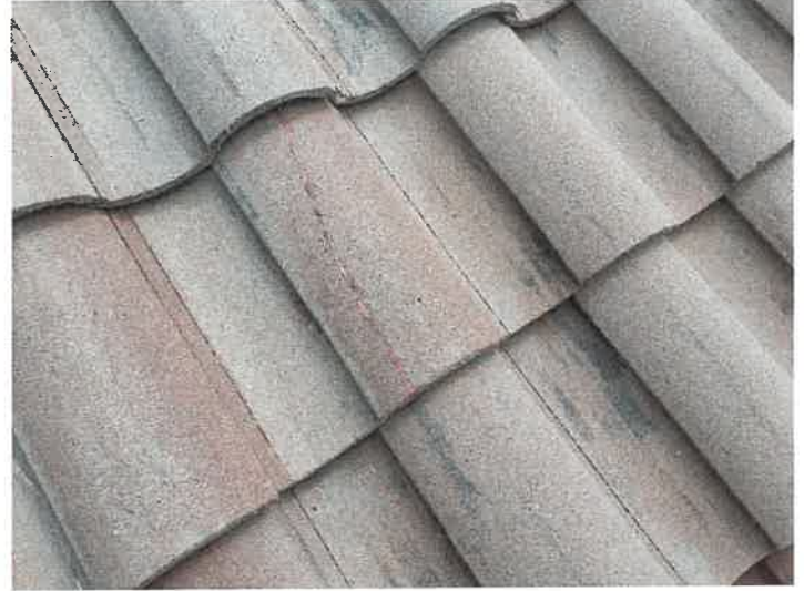
Building 15114: Repaired Cracked Roof Tiles
