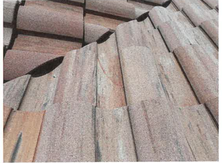
Building 15122: Repaired Cracked Roof Tiles
