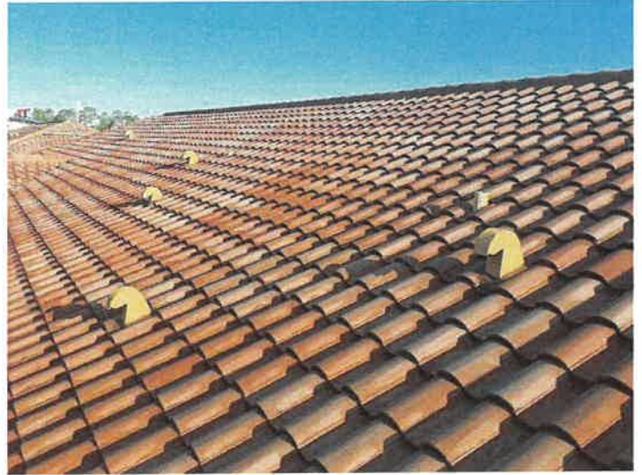
Building 15110: Roof Vents Roof vents appear to be in good condition.
