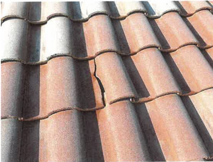
Building 15110: Identified Cracked Roof Tiles
