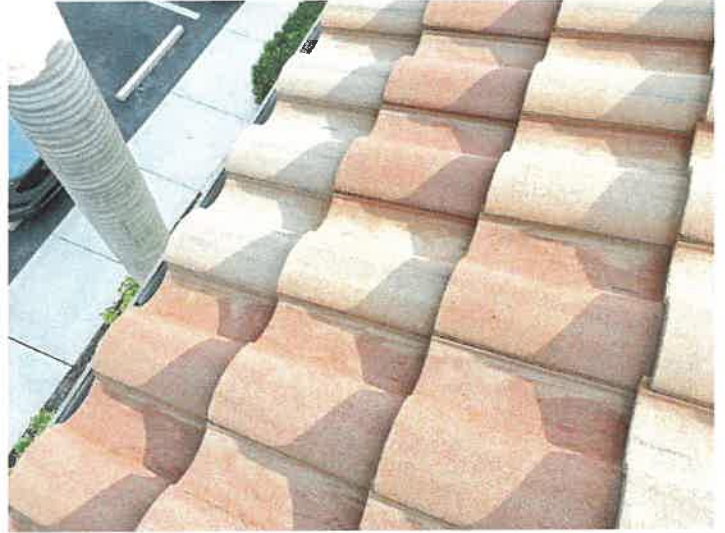
Building 15098: Repaired Displaced/Missing Roof Tile
