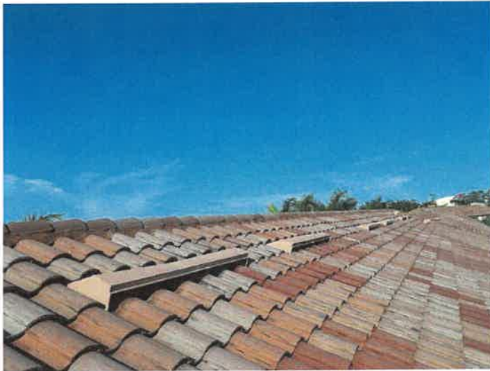
Building 15114: Roof Vents
