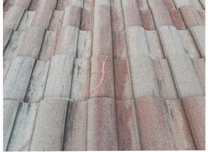
Building 15114: Repaired Cracked Roof Tiles The cracked roof tiles were repaired with Titebond sealant.
