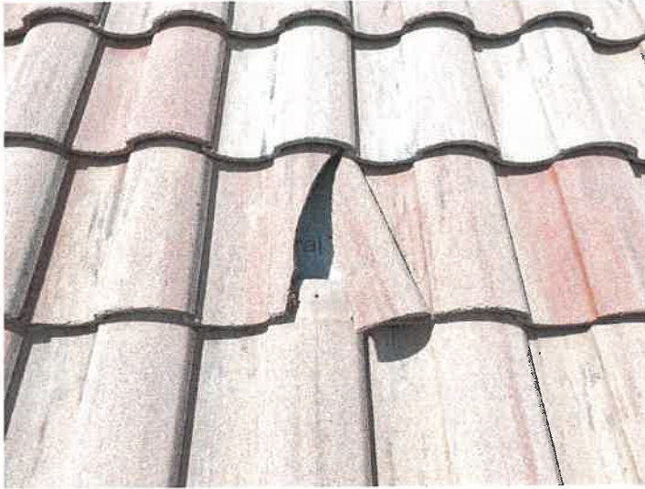
Building 15122: Identified Cracked Roof Tiles Cracked roof tiles can allow premature underlayment deterioration from excessive UV exposure.
