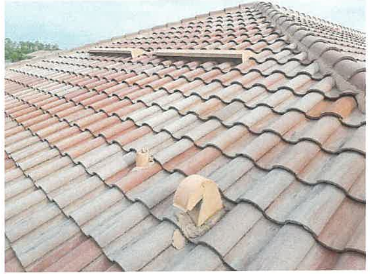
Building 15130: Roof Vents Roof vents appear to be in good condition.
