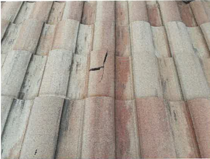
Building 15114: Identified Cracked Roof Tiles Cracked roof tiles can allow premature underlayment deterioration from excessive UV exposure.
