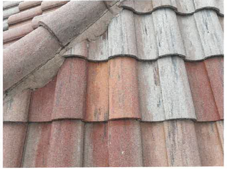
Building 15130: Repaired Displaced/Missing Roof Tile
