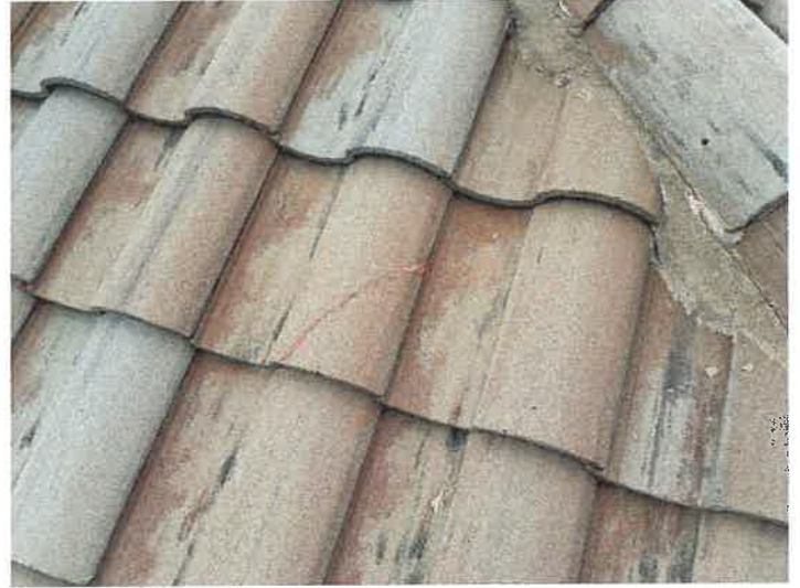
Building 15114: Repaired Cracked Roof Tiles
