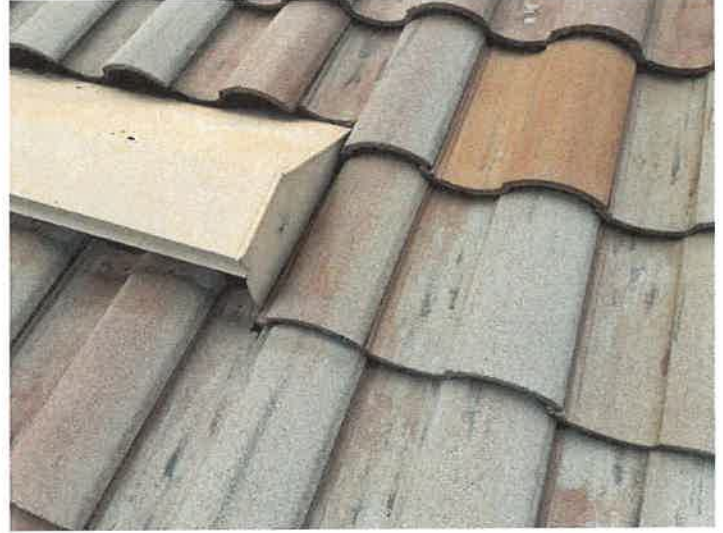
Building 15114: Repaired Displaced/Missing Roof Tile
