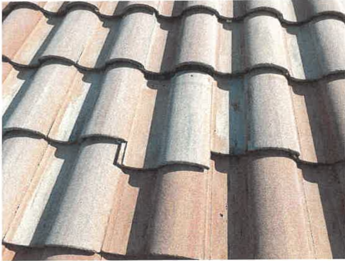
Building 15114: Displaced/Missing Roof Tile
