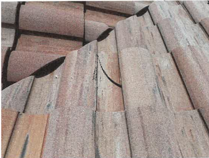
Building 15122: Identified Cracked Roof Tiles
