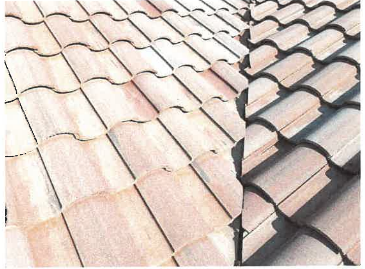
Building 15114: Repaired Displaced/Missing Roof Tile
