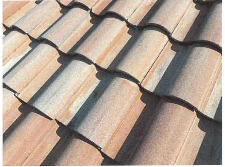
Building 15114: Repaired Displaced/Missing Roof Tile
