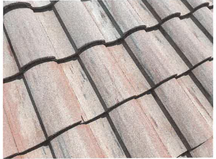
Building 15122: Repaired Cracked Roof Tiles
