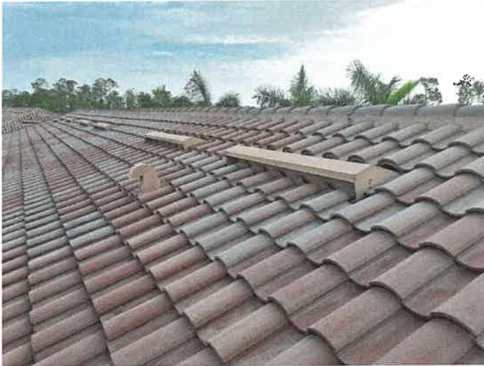
Building 15126: Roof Vents
