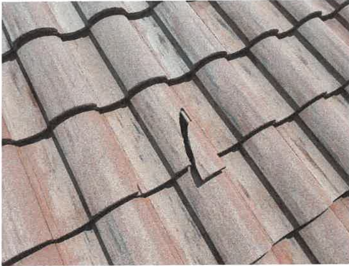
Building 15122: Identified Cracked Roof Tiles
