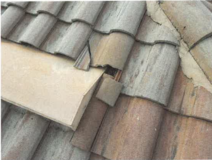
Building 15126: Identified Cracked Roof Tiles
