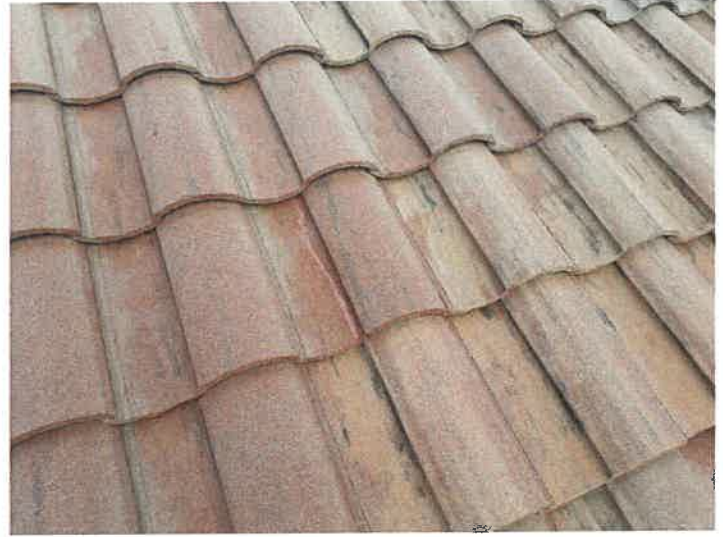
Building 15126: Repaired Cracked Roof Tiles
