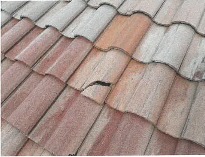
Building 15130: Identified Cracked Roof Tiles
