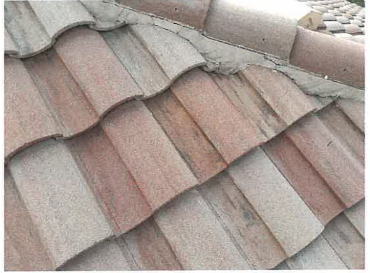
Building 15126: Repaired Displaced/Missing Roof Tile
