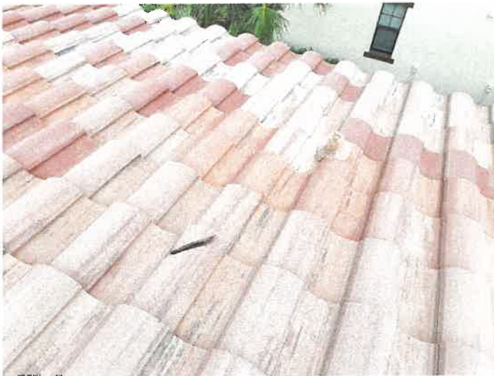
Building 15106: Identified Cracked Roof Tiles
