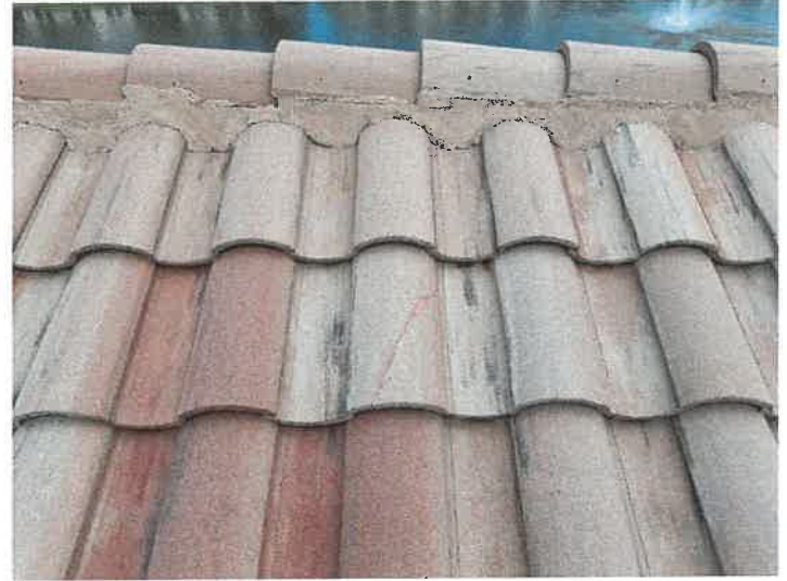
Building 15114: Repaired Cracked Roof Tiles
