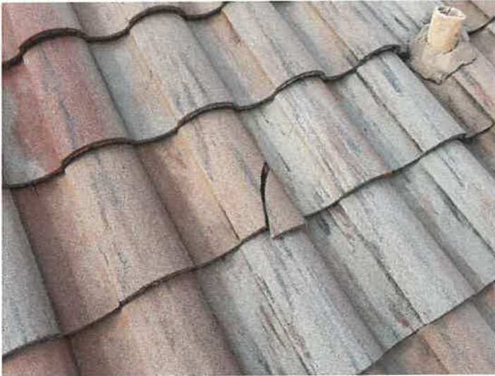
Building 15130: Identified Cracked Roof Tiles
