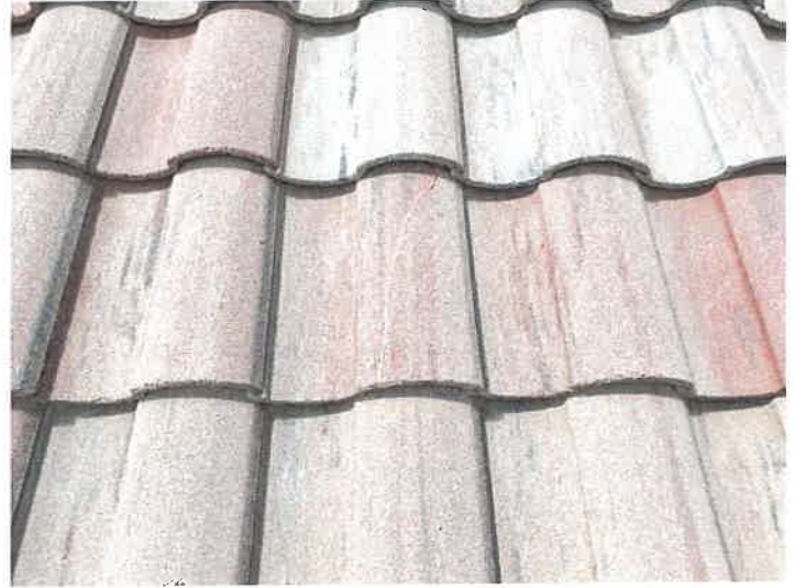
Building 15122: Repaired Cracked Roof Tiles The cracked roof tiles were repaired with Titebond sealant.
