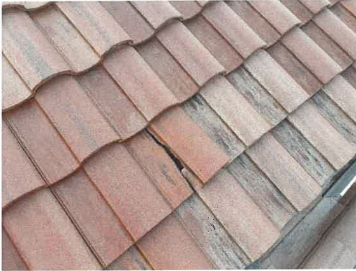
Building 15110: Identified Cracked Roof Tiles
