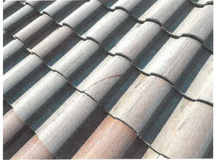
Building 15114: Repaired Cracked Roof Tiles
