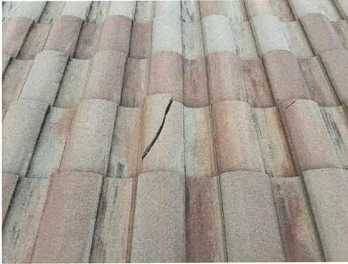
Building 15114: Identified Cracked Roof Tiles
