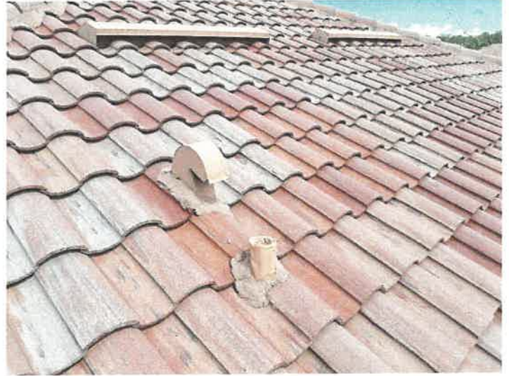
Building 15122: Lead Boots Lead boots appear to be in good condition.
