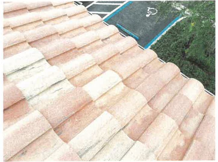
Building 15106: Repaired Displaced/Missing Roof Tile
