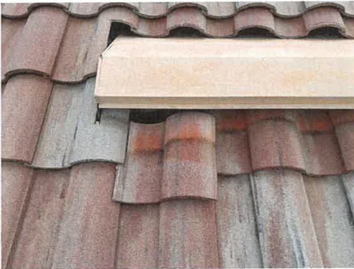
Building 15130: Displaced/Missing Roof Tile
