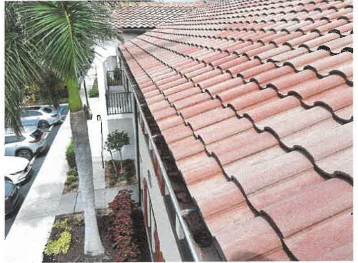
Building 15122: Gutters The gutters appear to be in good condition.
