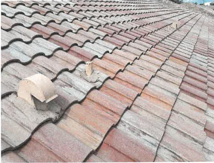
Building 15122: Lead Boots Lead boots appear to be in good condition.
