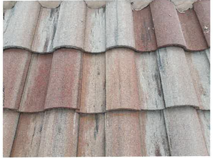
Building 15130: Repaired Displaced/Missing Roof Tile
