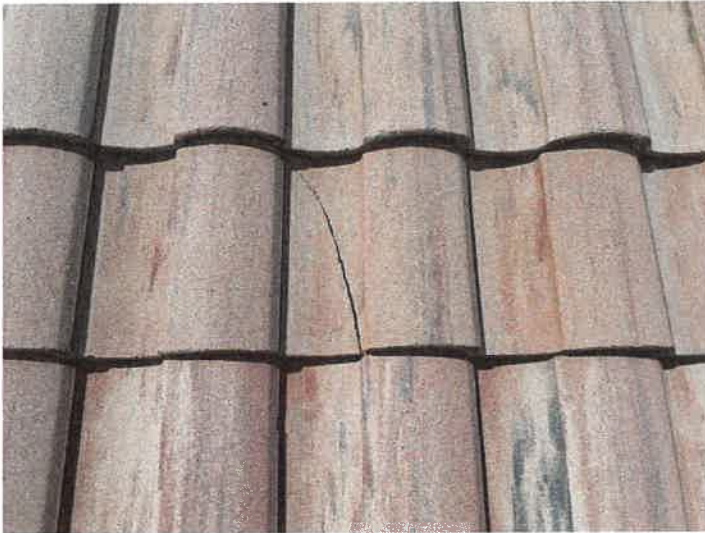
Building 15122: Identified Cracked Roof Tiles
