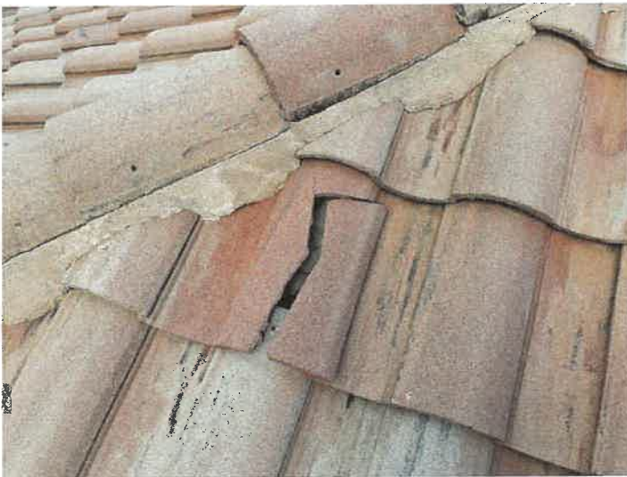
Building 15114: Identified Cracked Roof Tiles
