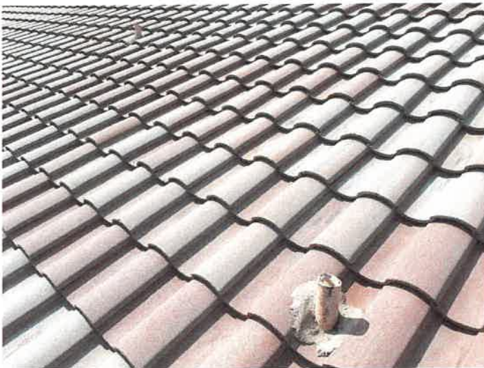
Building 15114: Lead Boots Lead boots appear to be in good condition.
