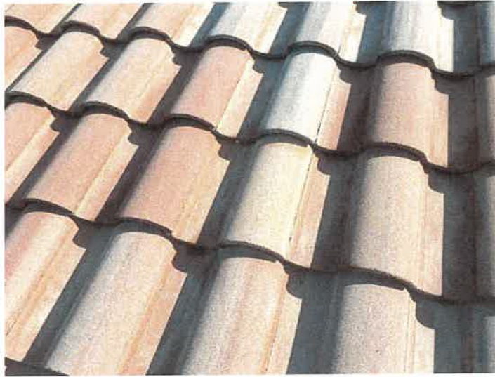
Building 15114: Repaired Displaced/Missing Roof Tile
