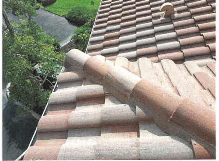
Building 15098: Repaired Cracked Roof Tiles
