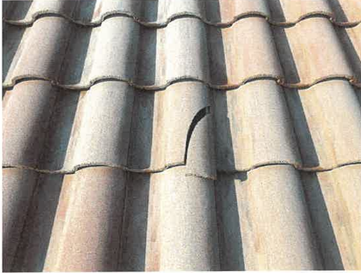
Building 15110: Identified Cracked Roof Tiles
