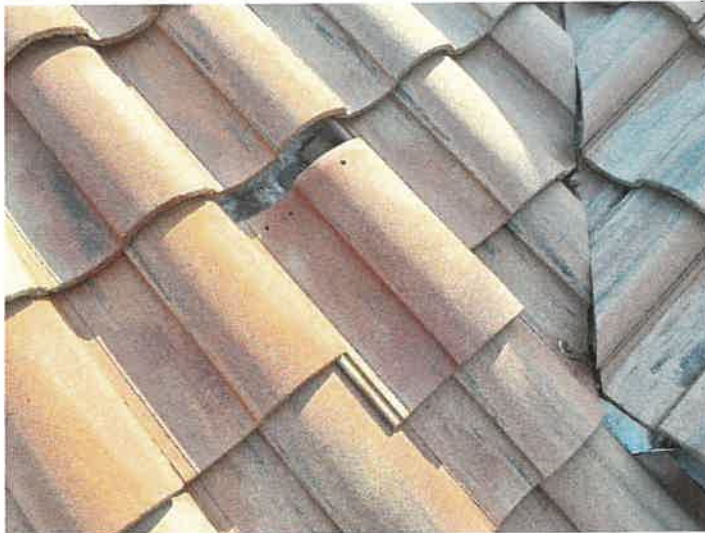
Building 15110: Displaced/Missing Roof Tile
