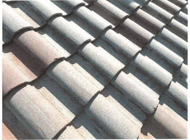
Building 15114: Repaired Cracked Roof Tiles
