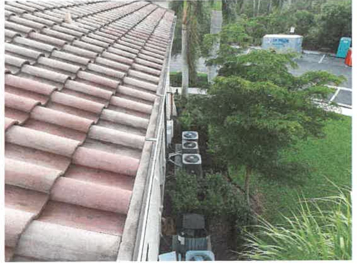
Building 15126: Gutters The gutters appear to be in good condition.
