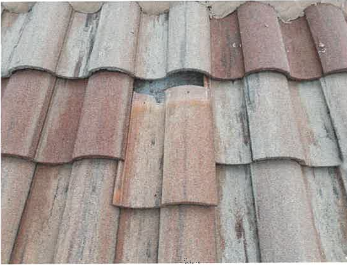
Building 15130: Displaced/Missing Roof Tile
