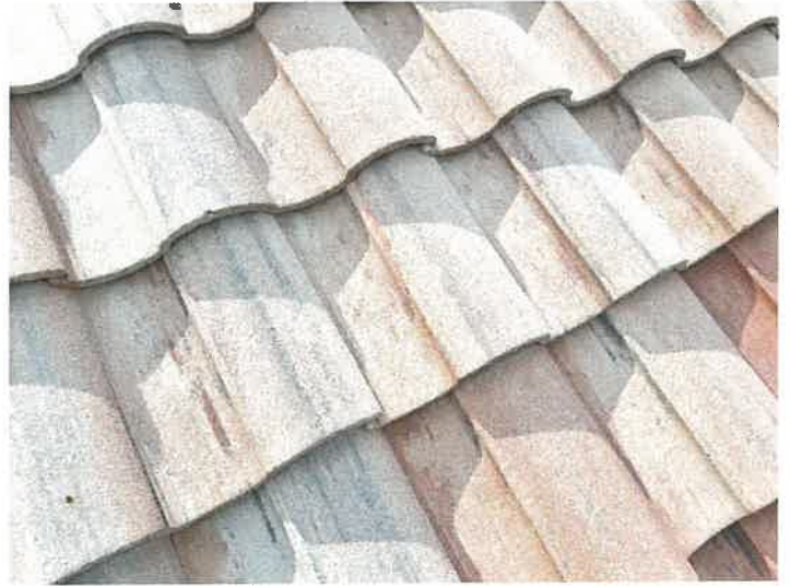
Building 15098: Repaired Cracked Roof Tiles
