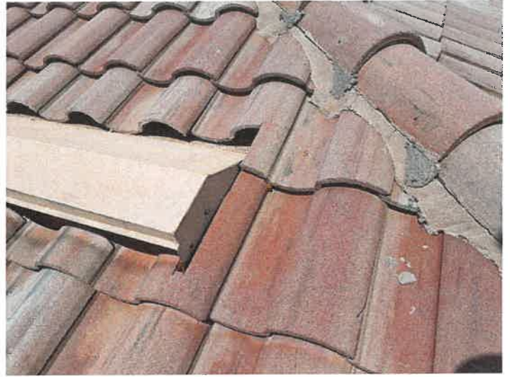
Building 15122: Repaired Cracked Roof Tiles
