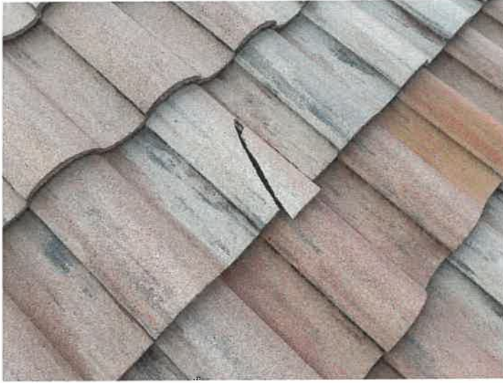
Building 15130: Identified Cracked Roof Tiles
