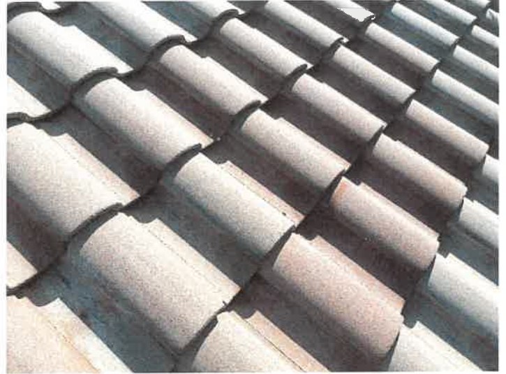
Building 15114: Repaired Displaced/Missing Roof Tile
