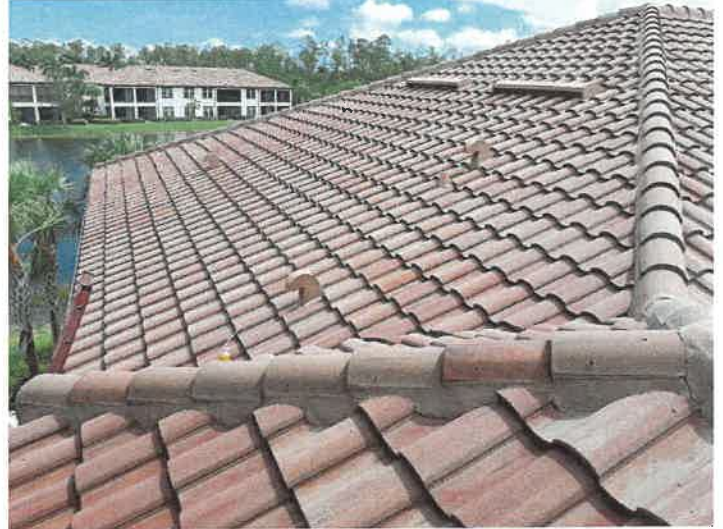
Building 15122: Surface Overview The roof surface appears to be in good, maintainable condition at this time.
