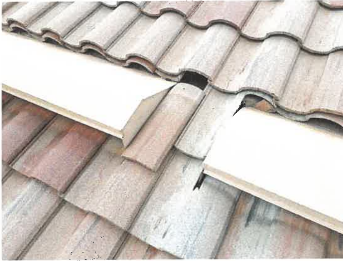
Building 15106: Displaced/Missing Roof Tile
