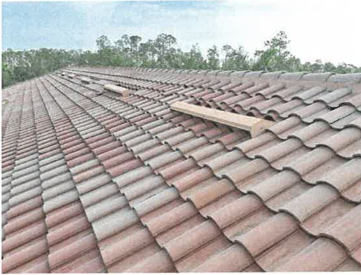
Building 15130: Roof Vents Roof vents appear to be in good condition.
