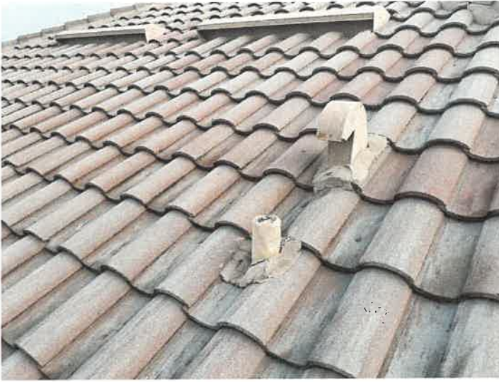
Building 15126: Lead Boots Lead boots appear to be in good condition.
