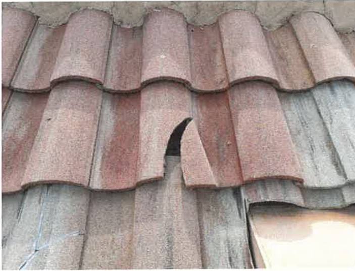
Building 15130: Identified Cracked Roof Tiles
