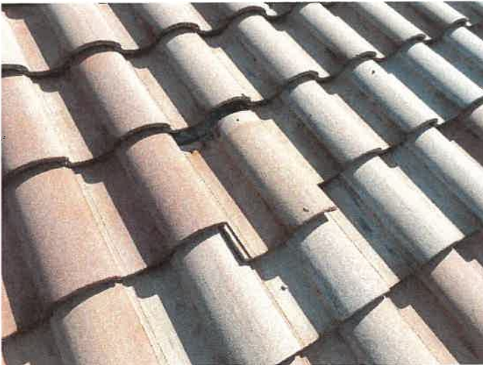
Building 15114: Displaced/Missing Roof Tile
