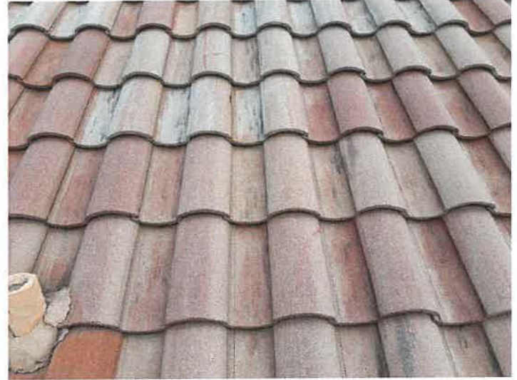
Building 15114: Repaired Cracked Roof Tiles
