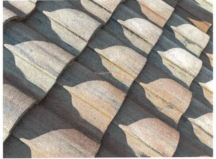
Building 15114: Repaired Cracked Roof Tiles
