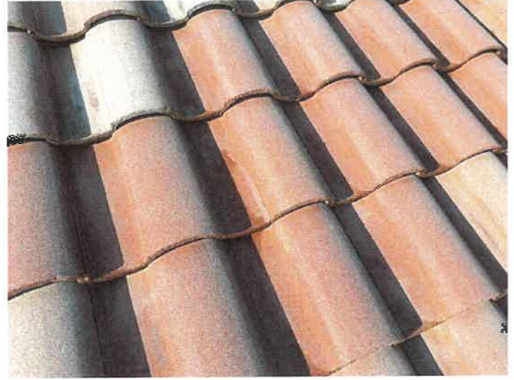
Building 15110: Repaired Cracked Roof Tiles
