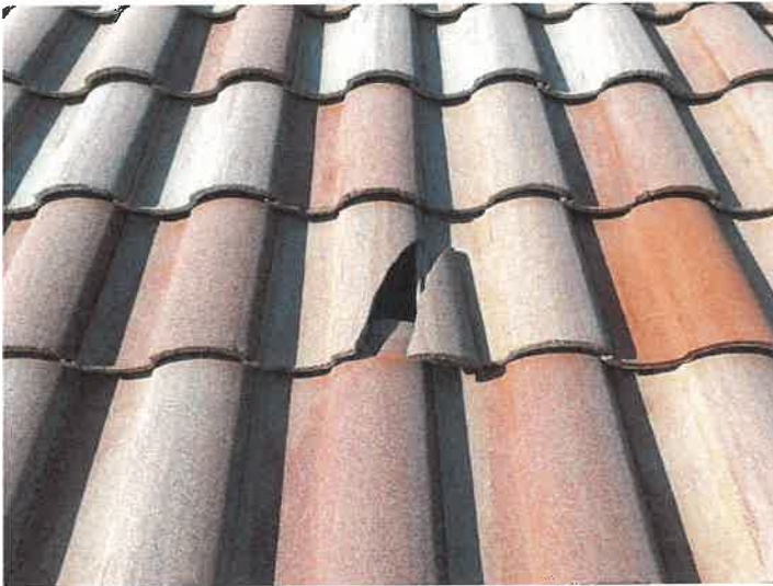
Building 15114: Identified Cracked Roof Tiles
