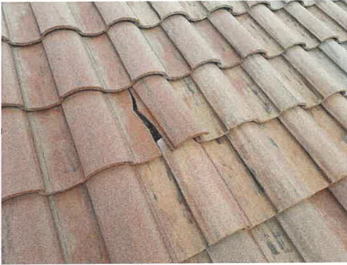
Building 15126: Identified Cracked Roof Tiles
