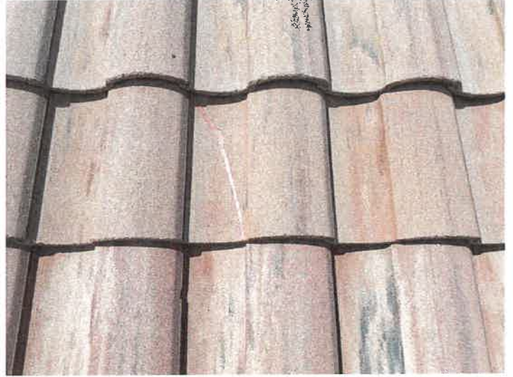
Building 15122: Repaired Cracked Roof Tiles
