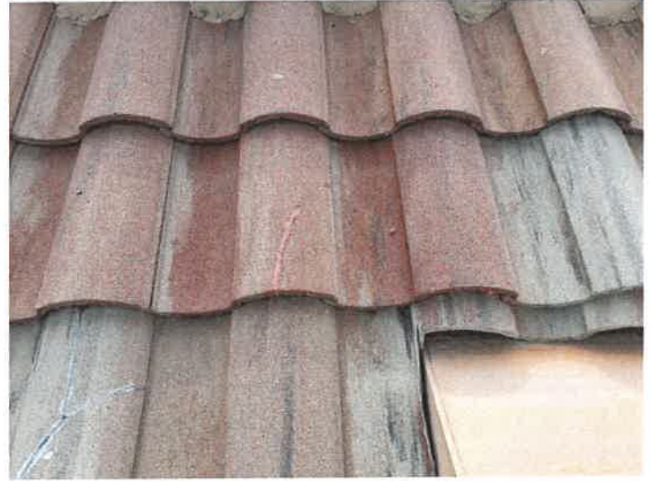
Building 15130: Repaired Cracked Roof Tiles
