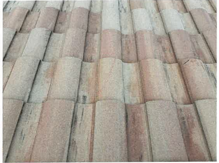
Building 15114: Repaired Cracked Roof Tiles
