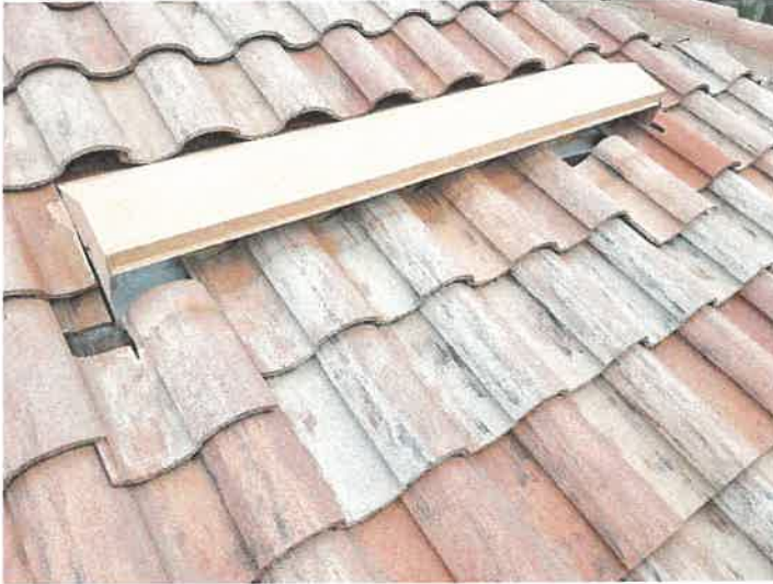
Building 15102: Displaced/Missing Roof Tile
