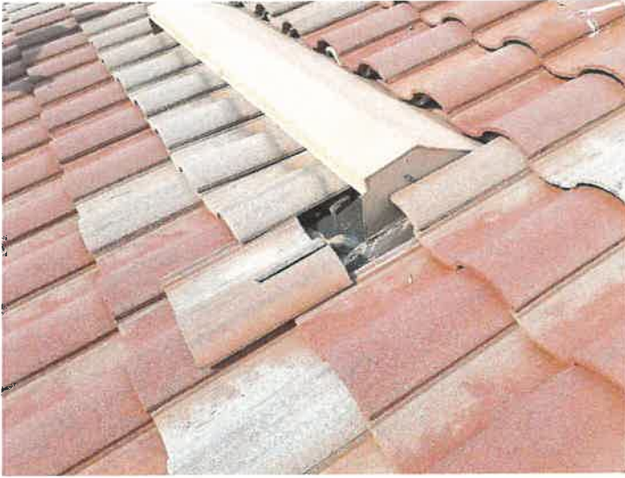
Building 15098: Displaced/Missing Roof Tile
