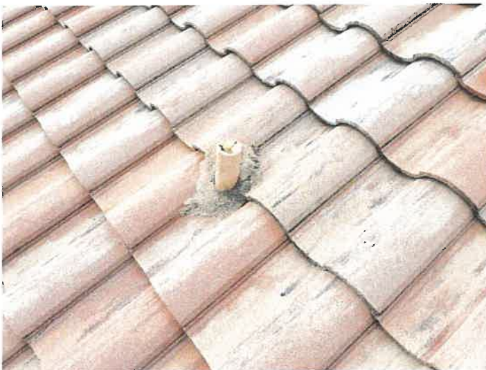
Building 15102: Lead Boots Lead boots appear to be in good condition.
