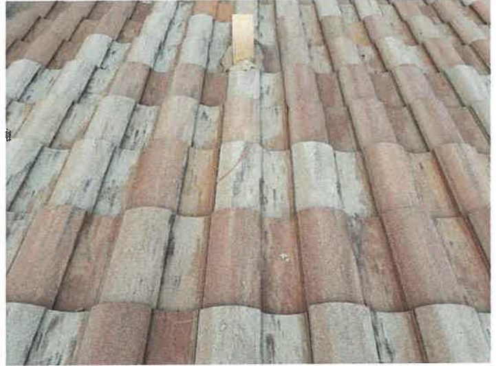
Building 15114: Repaired Cracked Roof Tiles
