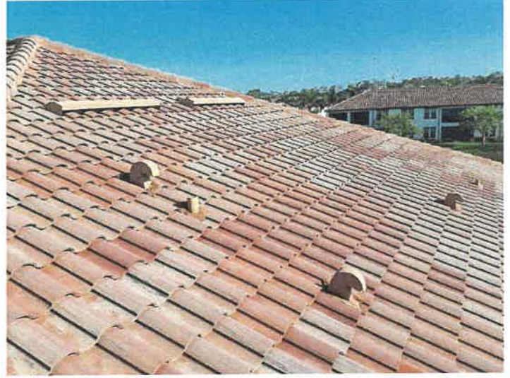
Building 15114: Roof Vents
