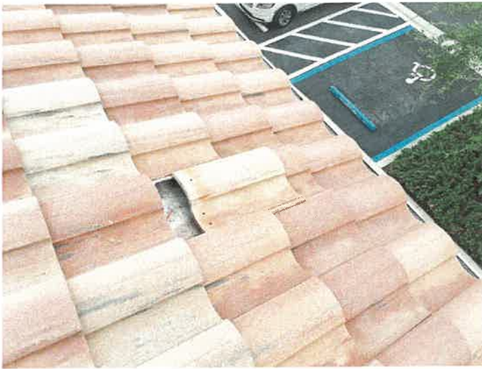
Building 15106: Displaced/Missing Roof Tile
