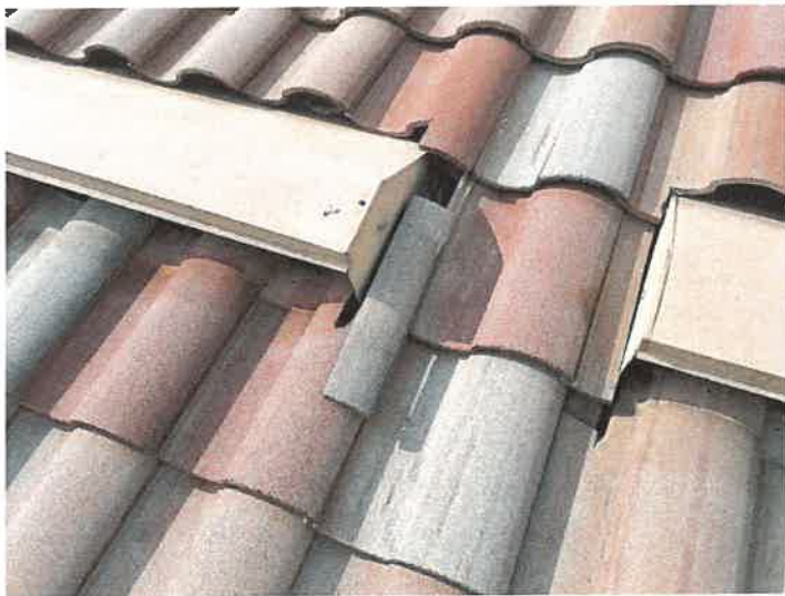
Building 15098: Displaced/Missing Roof Tile
