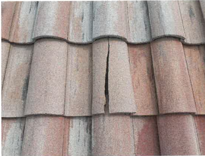
Building 15114: Identified Cracked Roof Tiles
