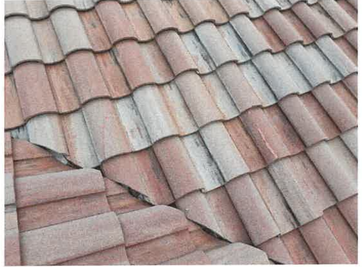
Building 15114: Repaired Cracked Roof Tiles
