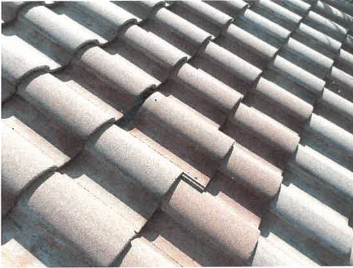
Building 15114: Displaced/Missing Roof Tile
