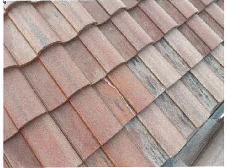
Building 15110: Repaired Cracked Roof Tiles
