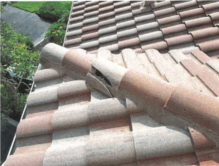
Building 15098: Identified Cracked Roof Tiles
