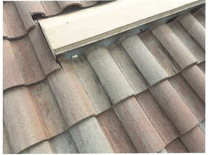
Building 15126: Repaired Displaced/Missing Roof Tile
