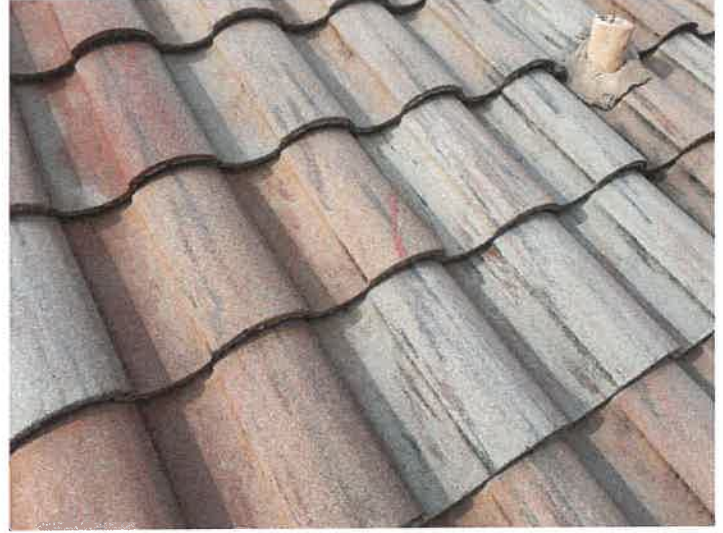
Building 15130: Repaired Cracked Roof Tiles
