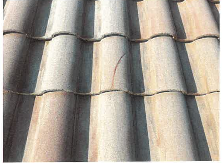
Building 15110: Repaired Cracked Roof Tiles
