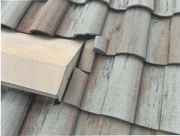
Building 15114: Identified Cracked Roof Tiles
