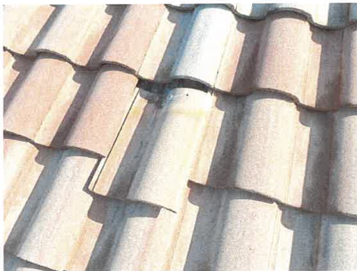
Building 15114: Displaced/Missing Roof Tile
