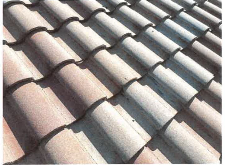
Building 15114: Repaired Displaced/Missing Roof Tile
