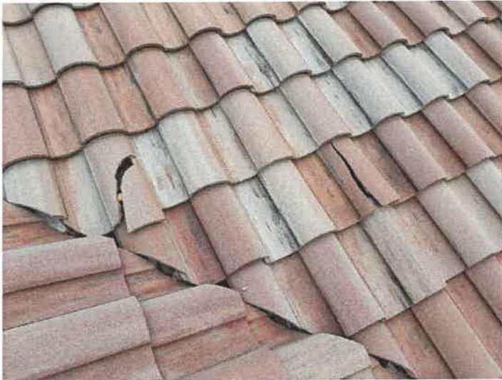
Building 15114: Identified Cracked Roof Tiles
