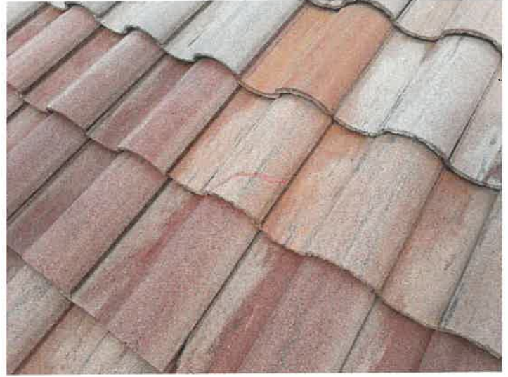
Building 15130: Repaired Cracked Roof Tiles
