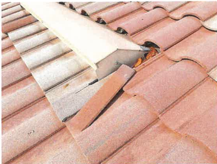
Building 15098: Displaced/Missing Roof Tile
