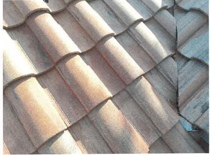
Building 15110: Repaired Displaced/Missing Roof Tile
