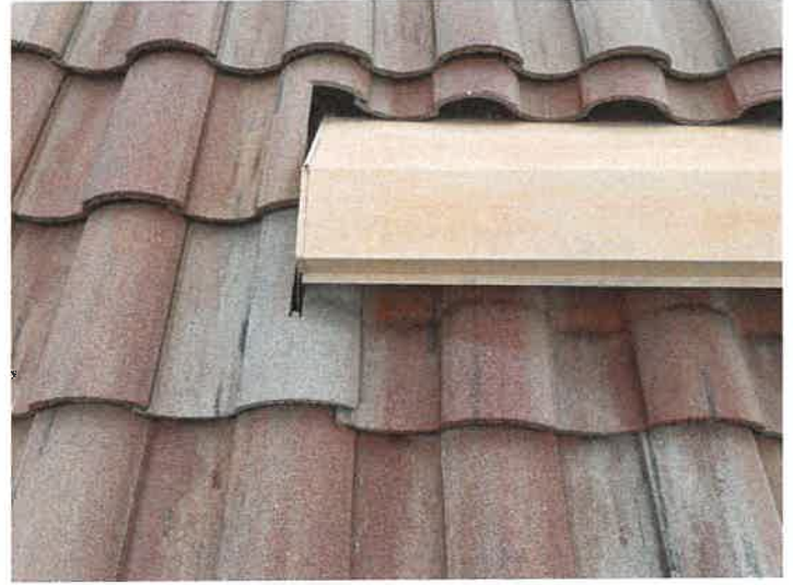
Building 15130: Repaired Displaced/Missing Roof Tile
