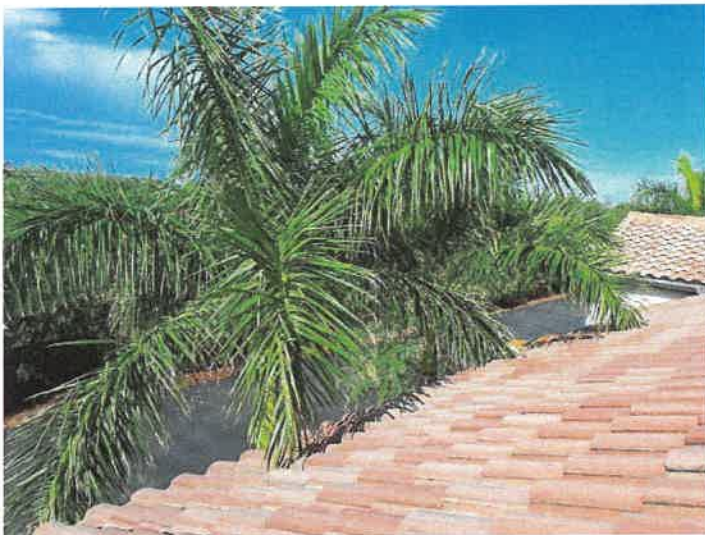
Building 15114: Tree Branches Identified tree branches hanging over the roof surface. Branches on the roof surface can cause deterioration of membrane, and act as an access for rodents and unwanted bugs/pests.
