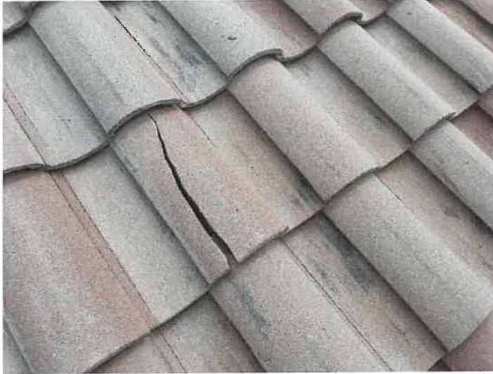
Building 15114: Identified Cracked Roof Tiles
