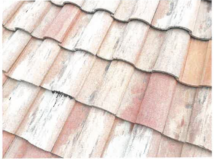
Building 15102: Repaired Displaced/Missing Roof Tile
