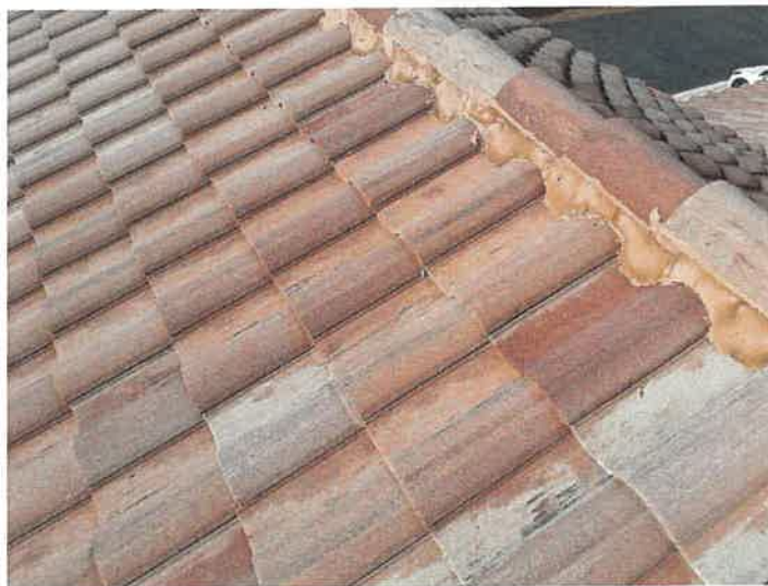
Building 15114: Repaired Displaced/Missing Roof Tile
