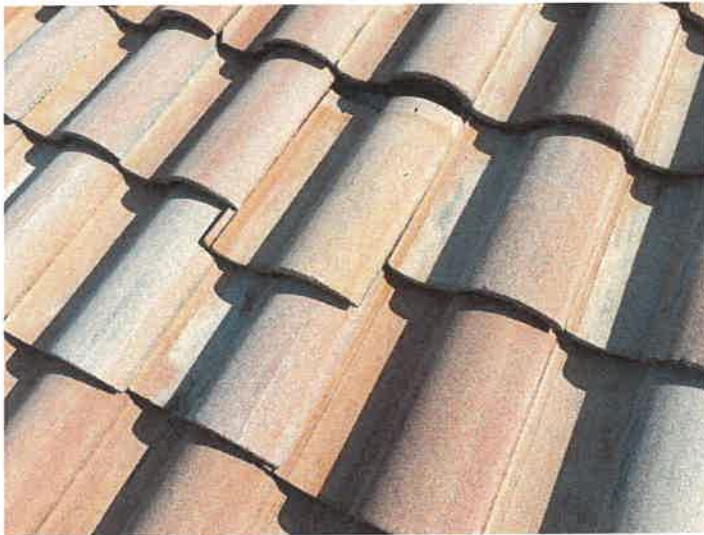
Building 15114: Displaced/Missing Roof Tile
