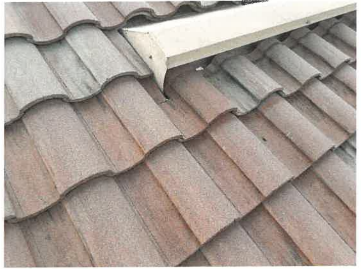
Building 15126: Repaired Displaced/Missing Roof Tile
