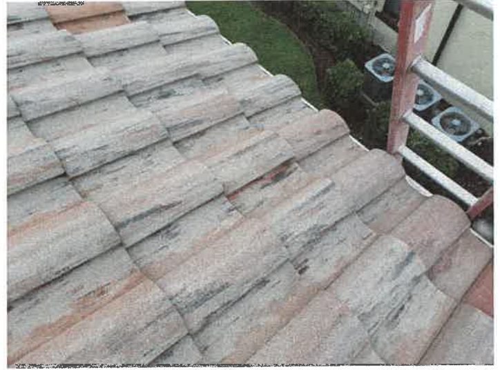
Building 15130: Repaired Cracked Roof Tiles The cracked roof tiles were repaired with Titebond sealant.
