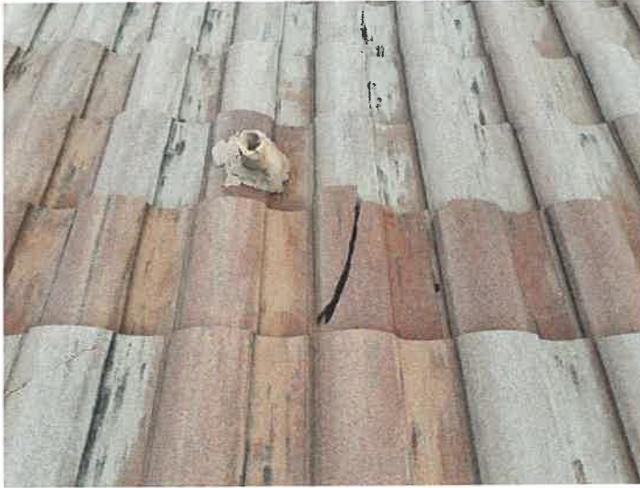
Building 15114: Identified Cracked Roof Tiles
