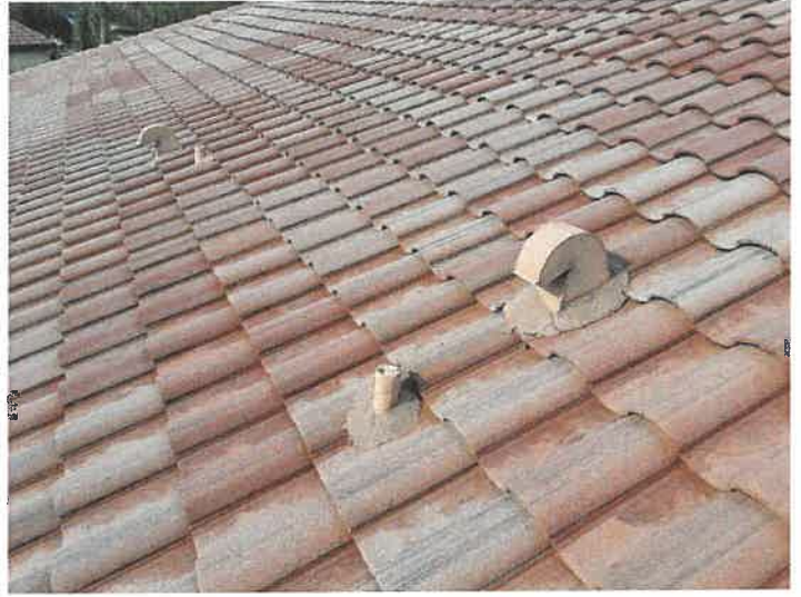
Building 15098: Lead Boots Lead boots appear to be in good condition.
