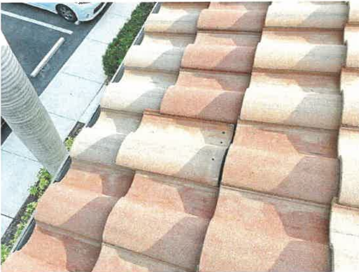
Building 15098: Displaced/Missing Roof Tile
