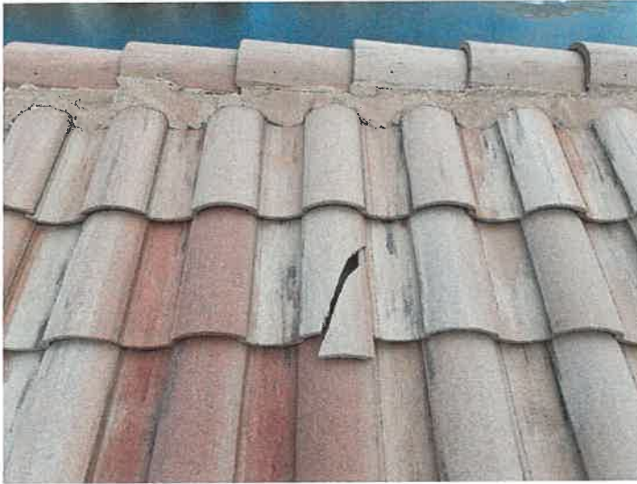
Building 15114: Identified Cracked Roof Tiles
