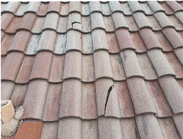
Building 15114: Identified Cracked Roof Tiles
