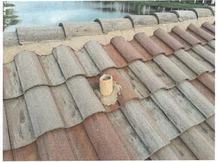
Building 15126: Lead Boots Lead boots appear to be in good condition.
