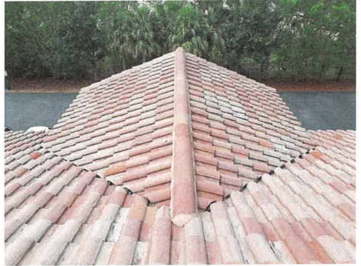
Building 15122: Valley The valley tiles appear to be in good condition.
