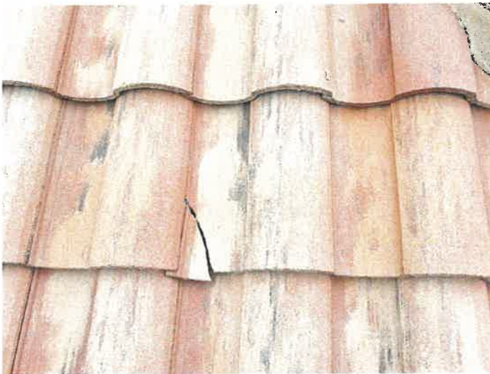
Building 15102: Identified Cracked Roof Tiles
