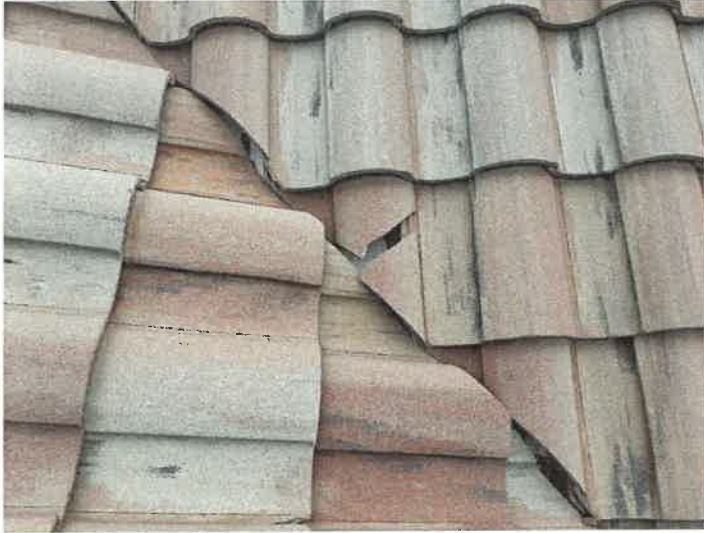
Building 15114: Identified Cracked Roof Tiles
