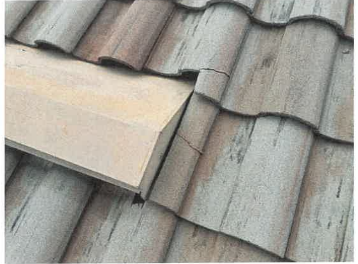
Building 15114: Repaired Cracked Roof Tiles
