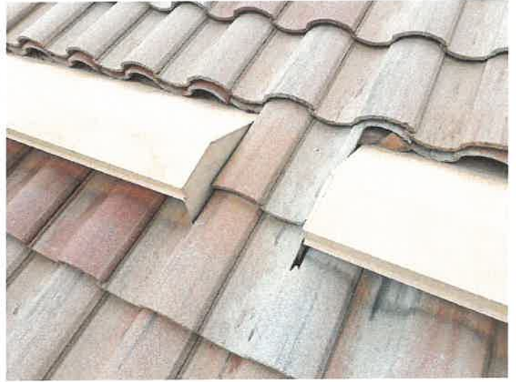
Building 15106: Repaired Displaced/Missing Roof Tile
