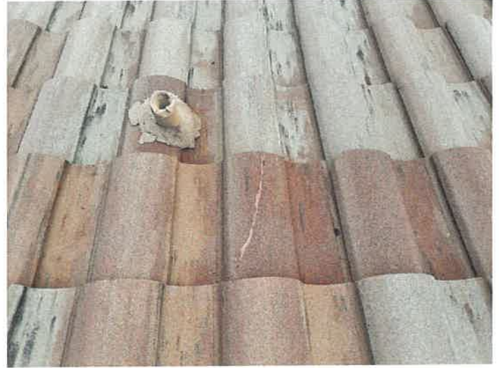
Building 15114: Repaired Cracked Roof Tiles
