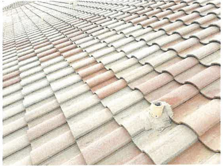
Building 15106: Lead Boots Lead boots appear to be in good condition.
