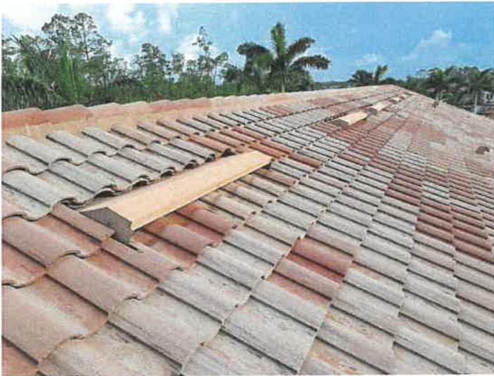
Building 15098: Roof Vents
