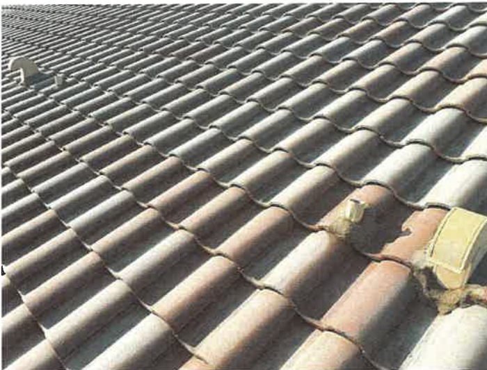
Building 15110: Lead Boots Lead boots appear to be in good condition.
