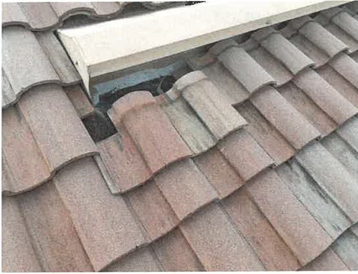
Building 15126: Displaced/Missing Roof Tile
