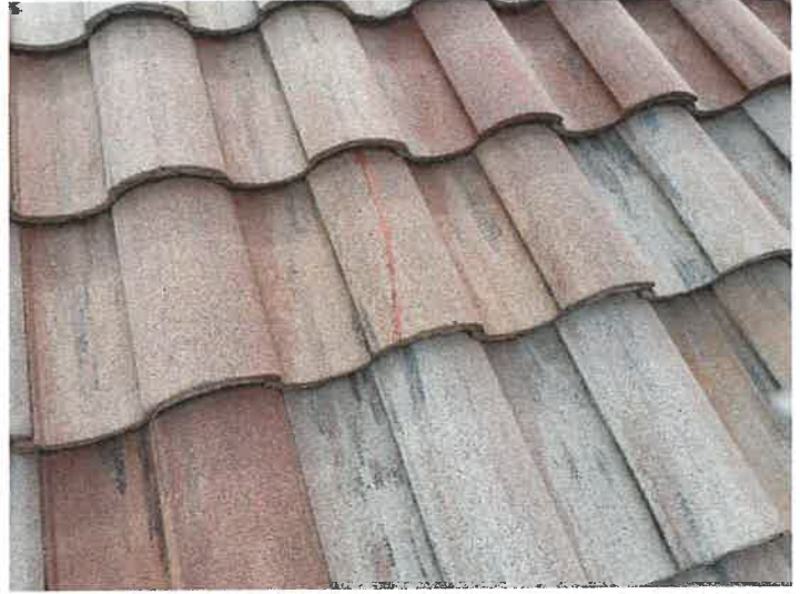
Building 15130: Repaired Cracked Roof Tiles
