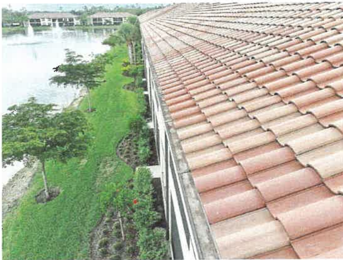
Building 15106: Gutters The gutters appear to be in good condition.
