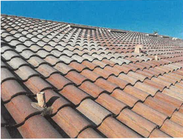
Building 15114: Lead Boots Lead boots appear to be in good condition.
