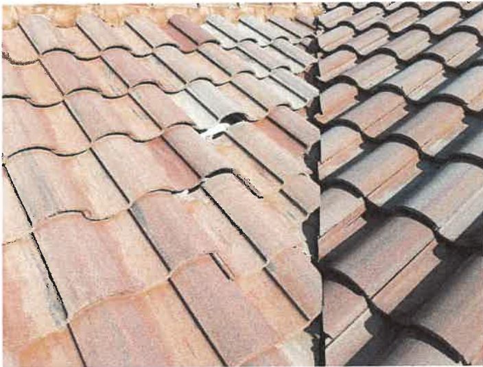
Building 15114: Displaced/Missing Roof Tile
