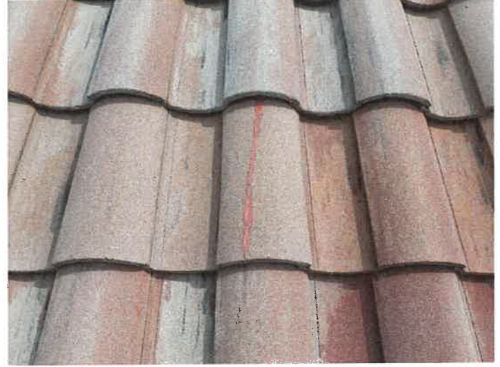
Building 15114: Repaired Cracked Roof Tiles
