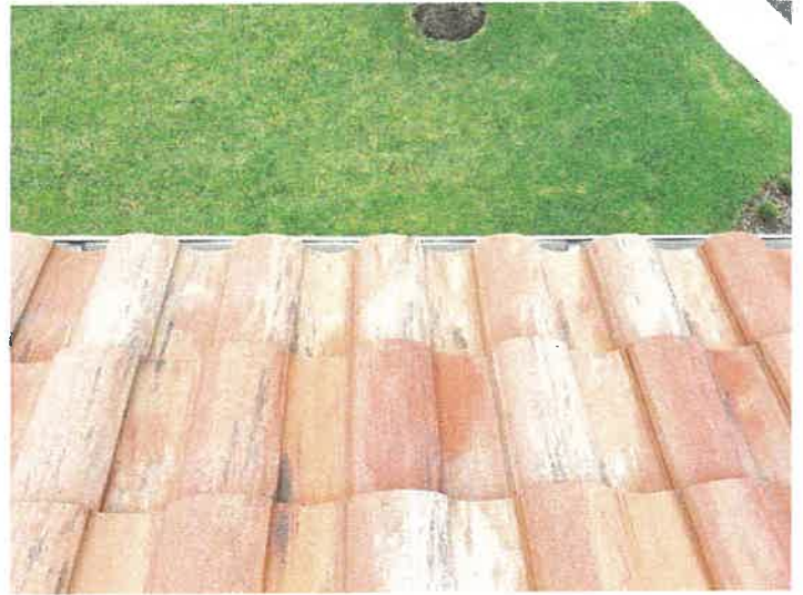
Building 15102: Repaired Cracked Roof Tiles
