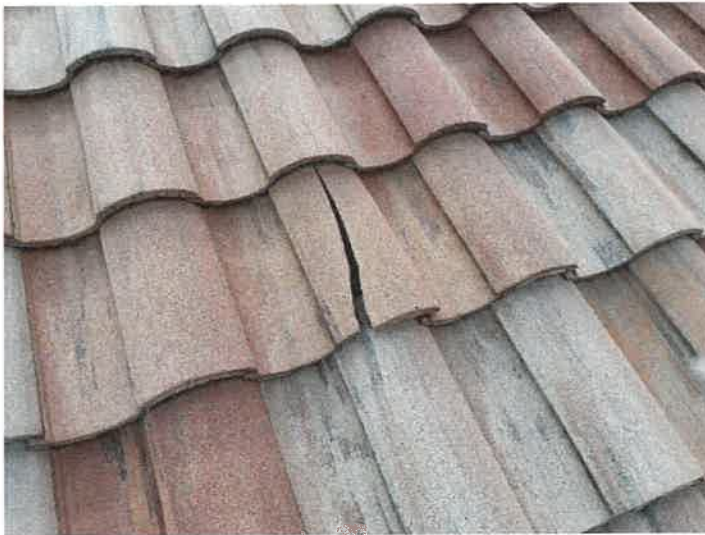
Building 15130: Identified Cracked Roof Tiles
