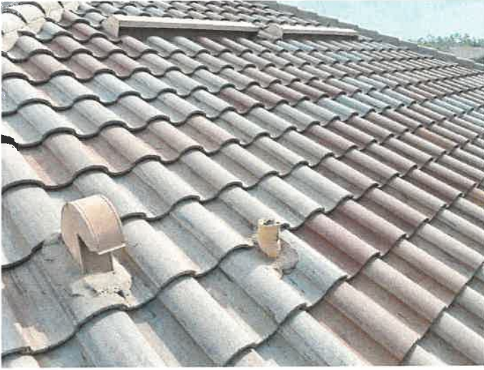
Building 15098: Lead Boots Lead boots appear to be in good condition.
