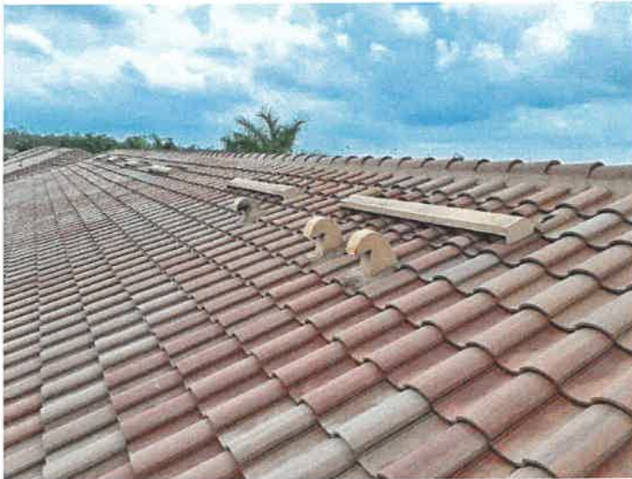
Building 15106: Identified Cracked Roof Tiles Cracked roof tiles can allow premature underlayment deterioration from excessive UV exposure.
