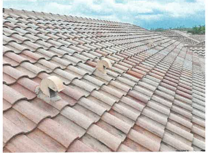
Building 15106: Roof Vents Roof vents appear to be in good condition.
