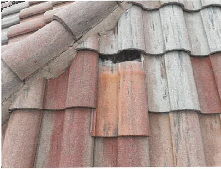
Building 15130: Displaced/Missing Roof Tile
