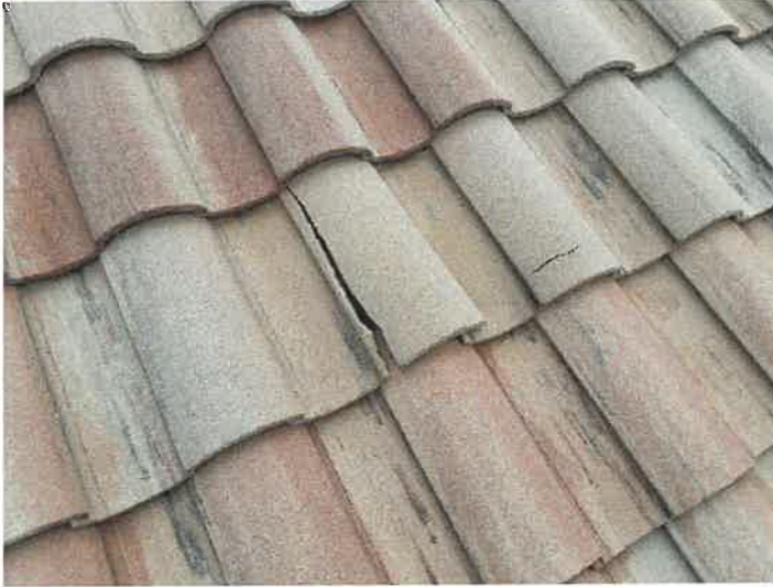
Building 15114: Identified Cracked Roof Tiles Cracked roof tiles can allow premature underlayment deterioration from excessive UV exposure.
