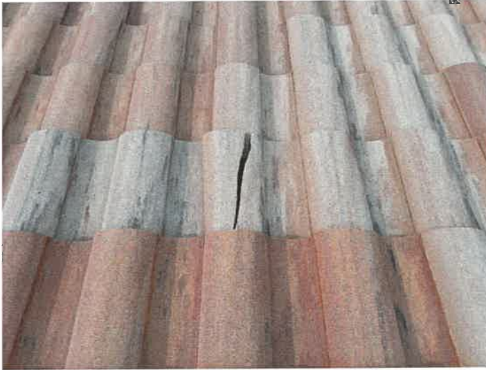
Building 15130: Identified Cracked Roof Tiles Cracked roof tiles can allow premature underlayment deterioration from excessive UV exposure.
