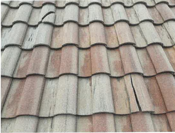
Building 15114: Identified Cracked Roof Tiles
