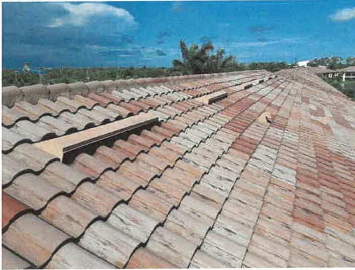
Building 15114: Roof Vents Roof vents appear to be in good condition.
