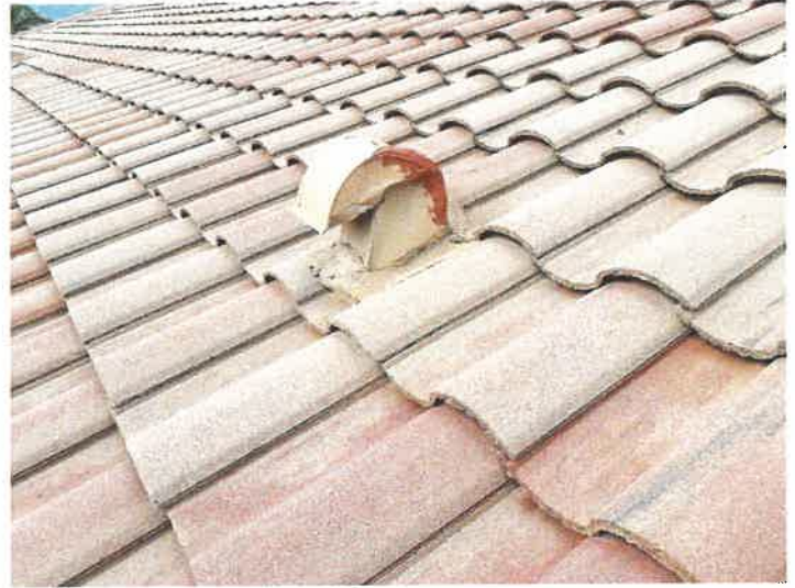
Building 15130: Temporary Repair A temporary repair was made, suggest replace gooseneck vent.
