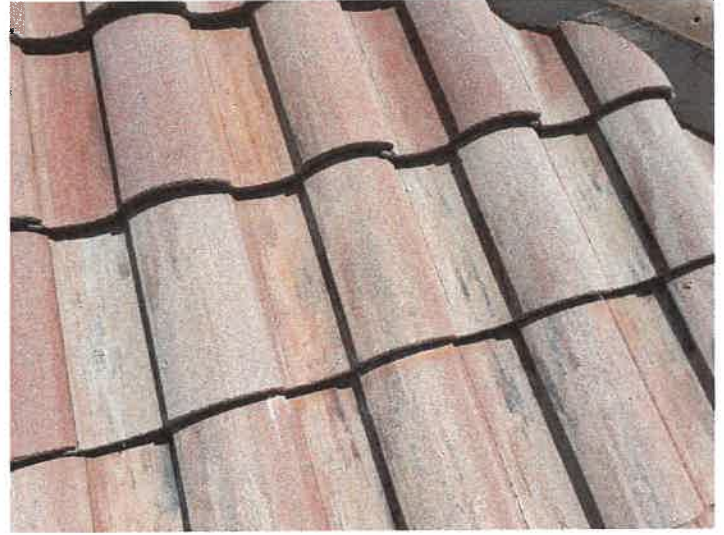
Building 15122: Repaired Displaced/Missing Roof Tile
