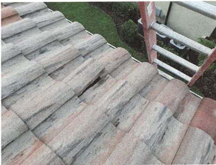
Building 15130: Identified Cracked Roof Tiles Cracked roof tiles can allow premature underlayment deterioration from excessive UV exposure.
