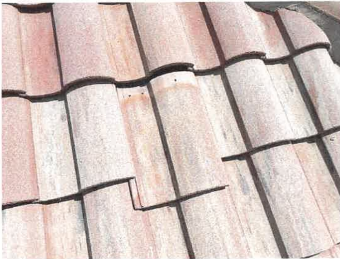
Building 15122: Displaced/Missing Roof Tile
