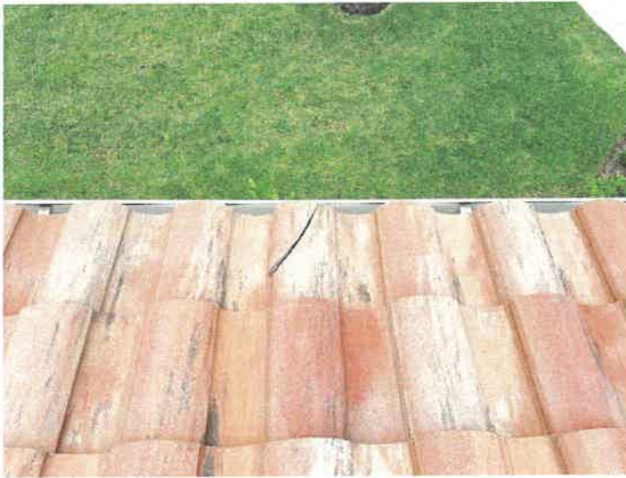
Building 15102: Identified Cracked Roof Tiles
