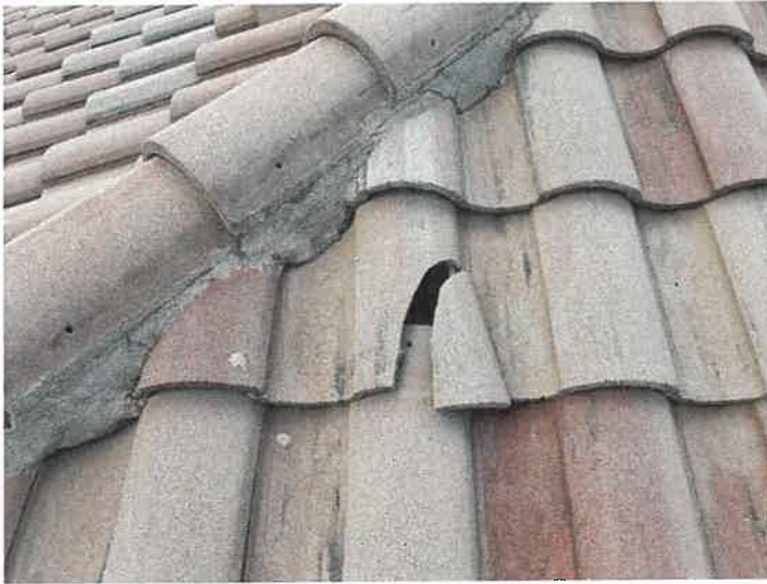
Building 15114: Identified Cracked Roof Tiles Cracked roof tiles can allow premature underlayment deterioration from excessive UV exposure.
