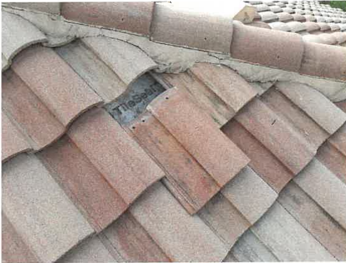
Building 15126: Displaced/Missing Roof Tile
