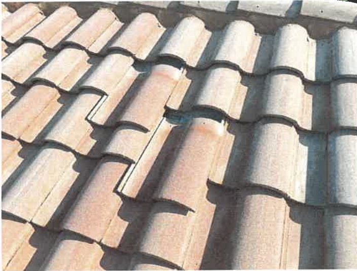
Building 15114: Displaced/Missing Roof Tile
