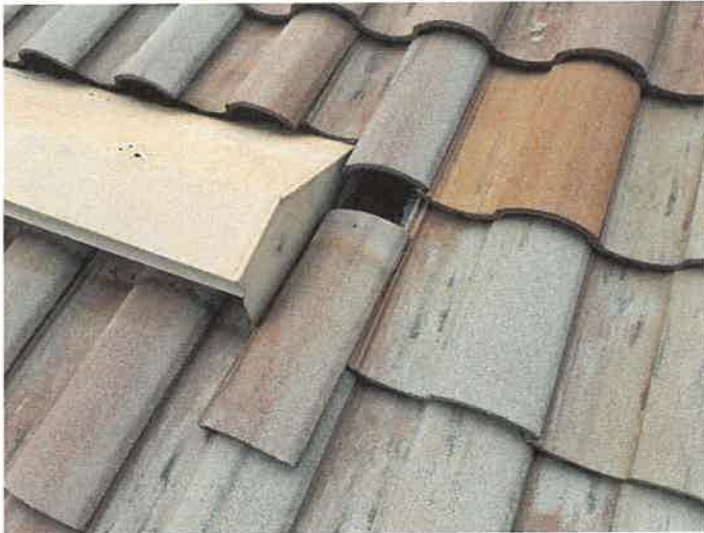
Building 15114: Displaced/Missing Roof Tile
