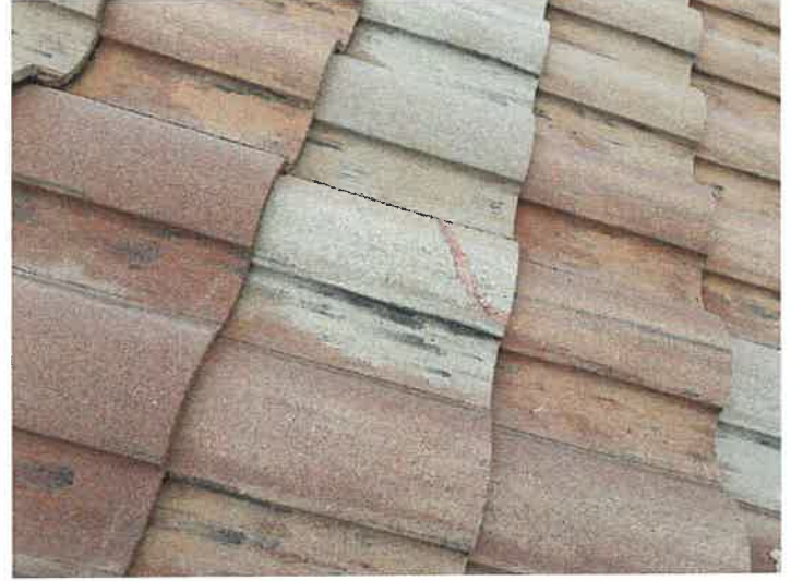
Building 15114: Repaired Cracked Roof Tiles
