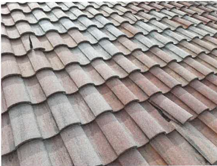
Building 15130: Identified Cracked Roof Tiles
