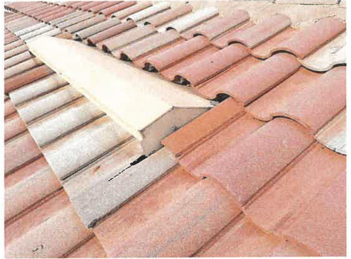
Building 15098: Repaired Displaced/Missing Roof Tile
