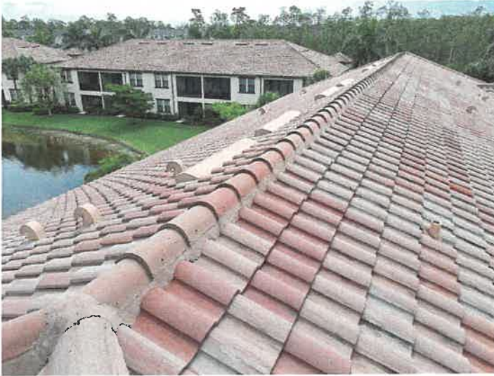
Building 15122: Ridge Tiles Ridge tiles appear to be in good condition.
