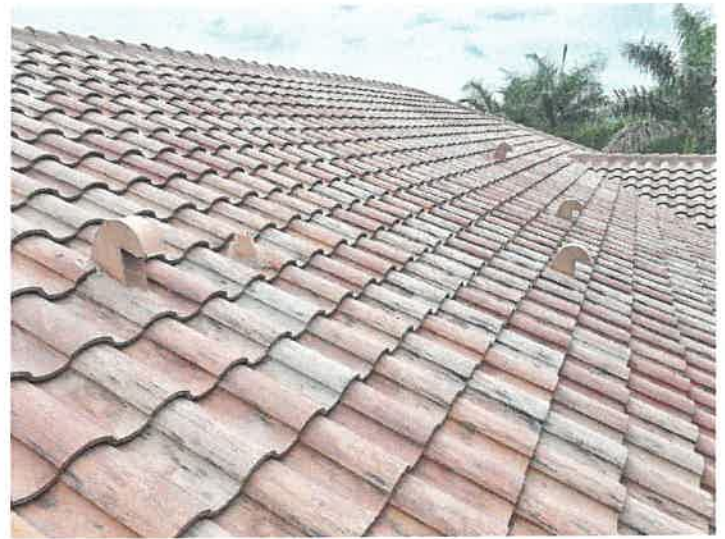
Building 15102: Roof Vents Roof vents appear to be in good condition.
