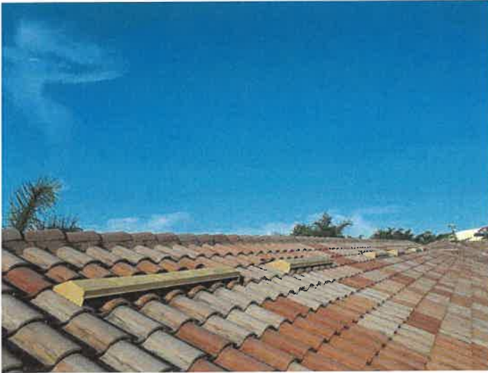
Building 15110: Roof Vents Roof vents appear to be in good condition.
