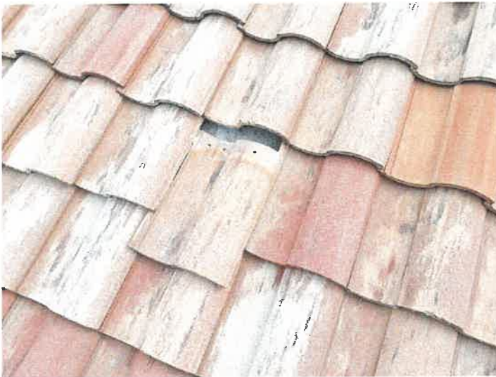
Building 15102: Displaced/Missing Roof Tile
