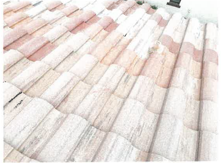
Building 15106: Repaired Cracked Roof Tiles
