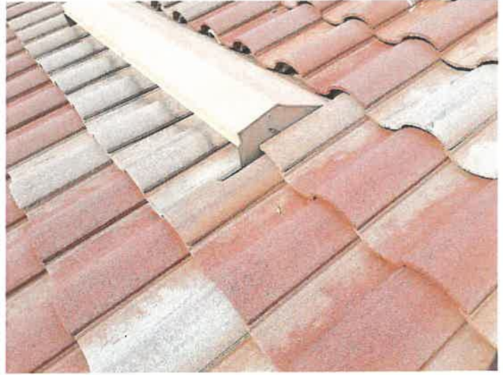
Building 15098: Repaired Displaced/Missing Roof Tile
