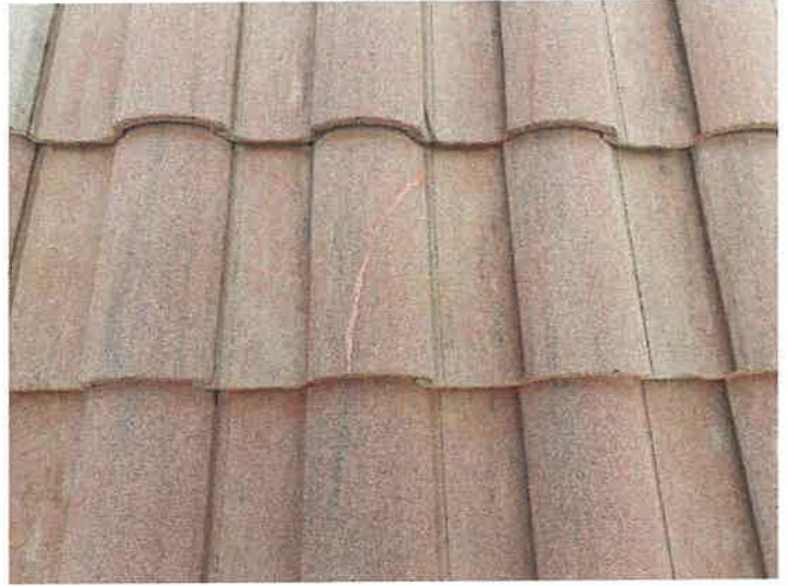
Building 15126: Repaired Cracked Roof Tiles The cracked roof tiles were repaired with Titebond sealant.
