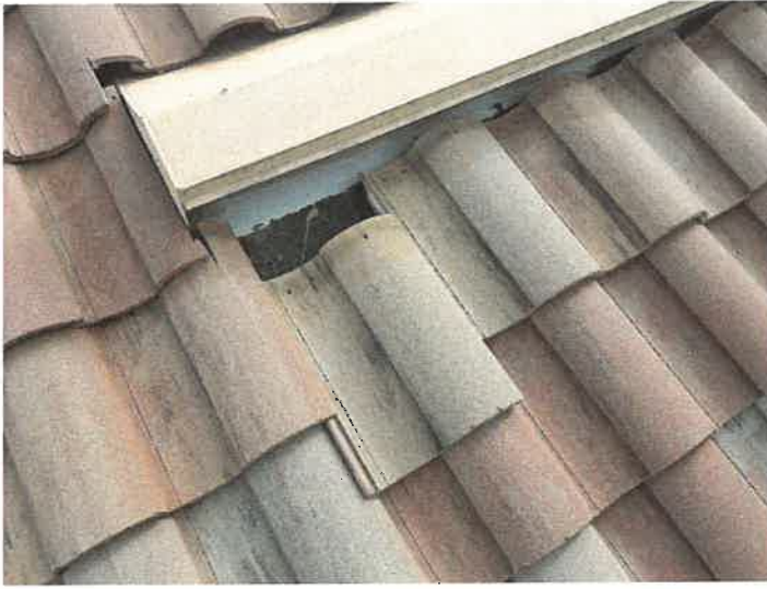
Building 15126: Displaced/Missing Roof Tile
