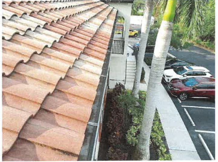
Building 15098: Gutters The gutters appear to be in good condition.
