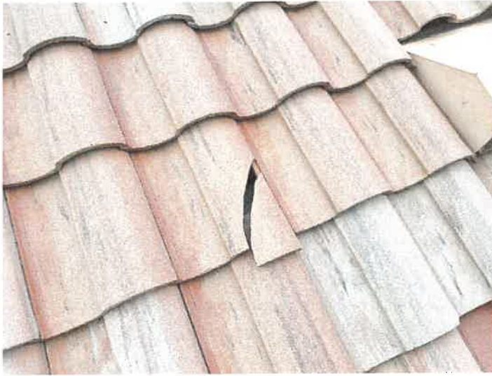
Building 15106: Identified Cracked Roof Tiles Cracked roof tiles can allow premature underlayment deterioration from excessive UV exposure.
