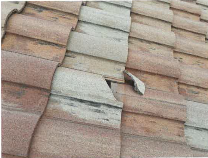
Building 15114: Identified Cracked Roof Tiles
