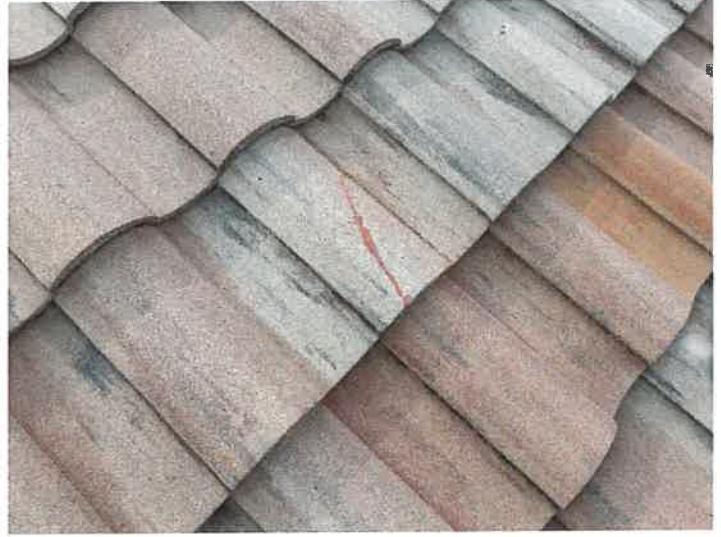
Building 15130: Repaired Cracked Roof Tiles
