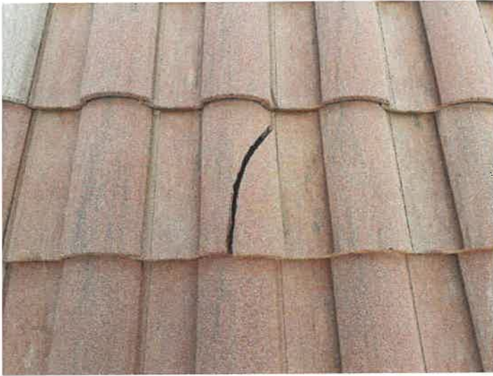
Building 15126: Identified Cracked Roof Tiles Cracked roof tiles can allow premature underlayment deterioration from excessive UV exposure.
