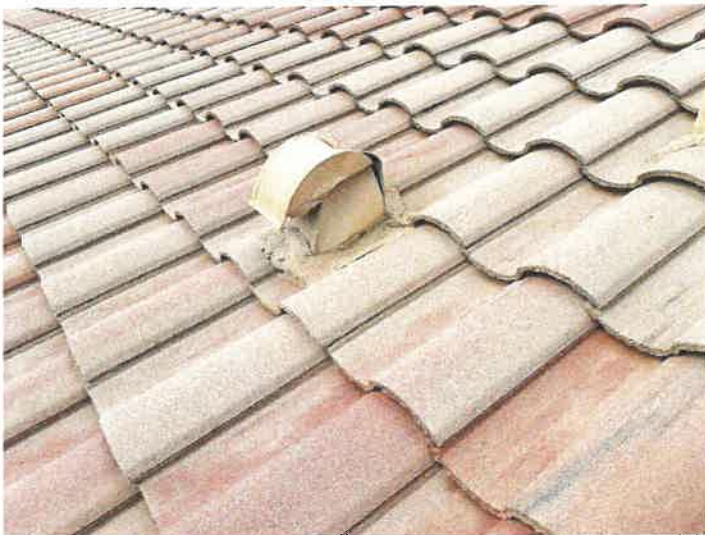
Building 15130: Gooseneck Vent Deformed Gooseneck vent is deformed and needs to be replaced.
