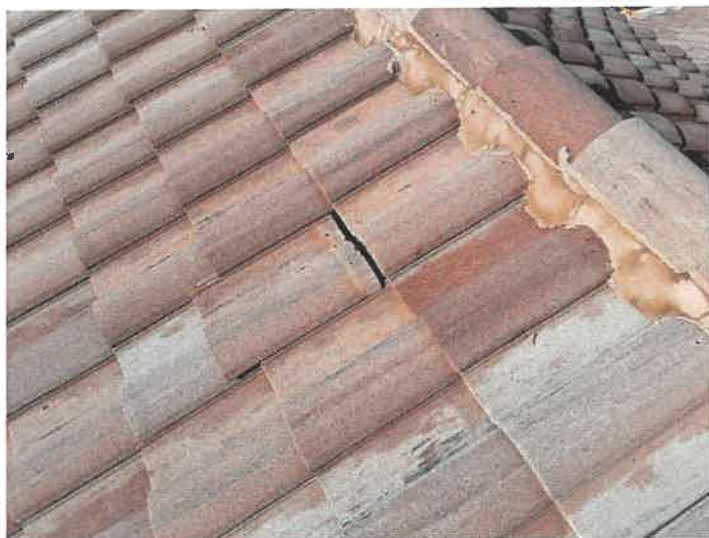
Building 15114: Displaced/Missing Roof Tile
