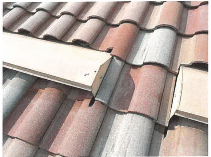
Building 15098: Repaired Displaced/Missing Roof Tile
