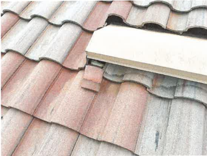
Building 15106: Displaced/Missing Roof Tile
