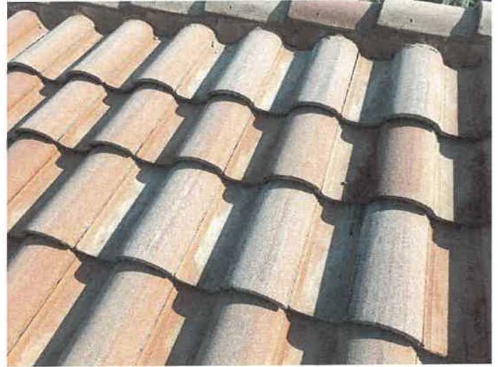
Building 15114: Repaired Displaced/Missing Roof Tile
