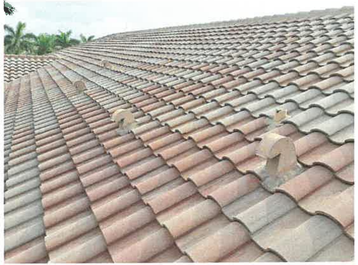
Building 15098: Roof Vents
