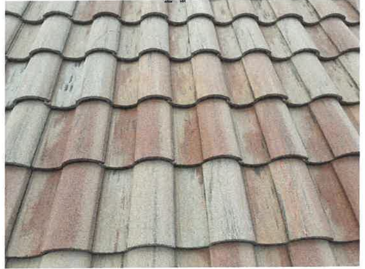
Building 15114: Repaired Cracked Roof Tiles
