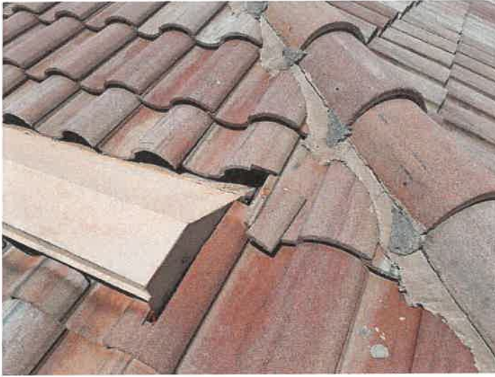
Building 15122: Identified Cracked Roof Tiles
