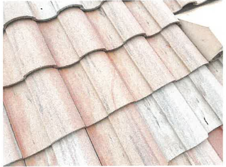
Building 15106: Repaired Cracked Roof Tiles The cracked roof tiles were repaired with Titebond sealant.
