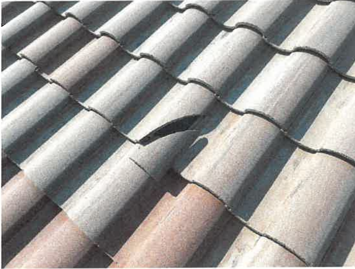
Building 15114: Identified Cracked Roof Tiles
